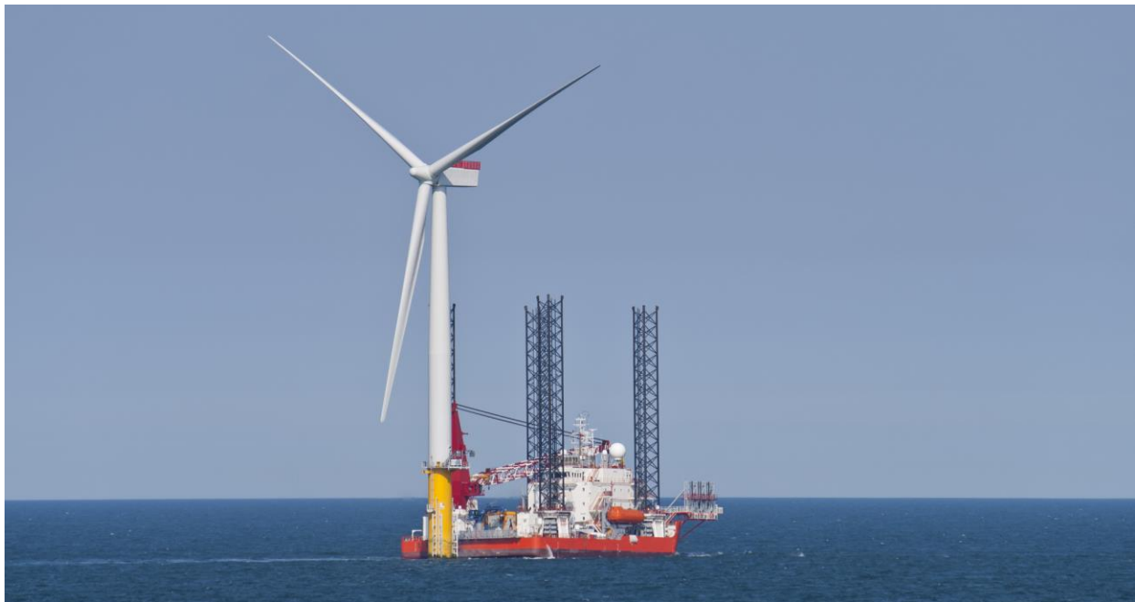
FIGURE 3-14. EXAMPLE OF A JACK-UP VESSEL INSTALLING A WTG
