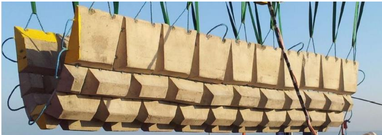
FIGURE 3-31. EXAMPLE OF CONCRETE CABLE PROTECTION MATTRESS
