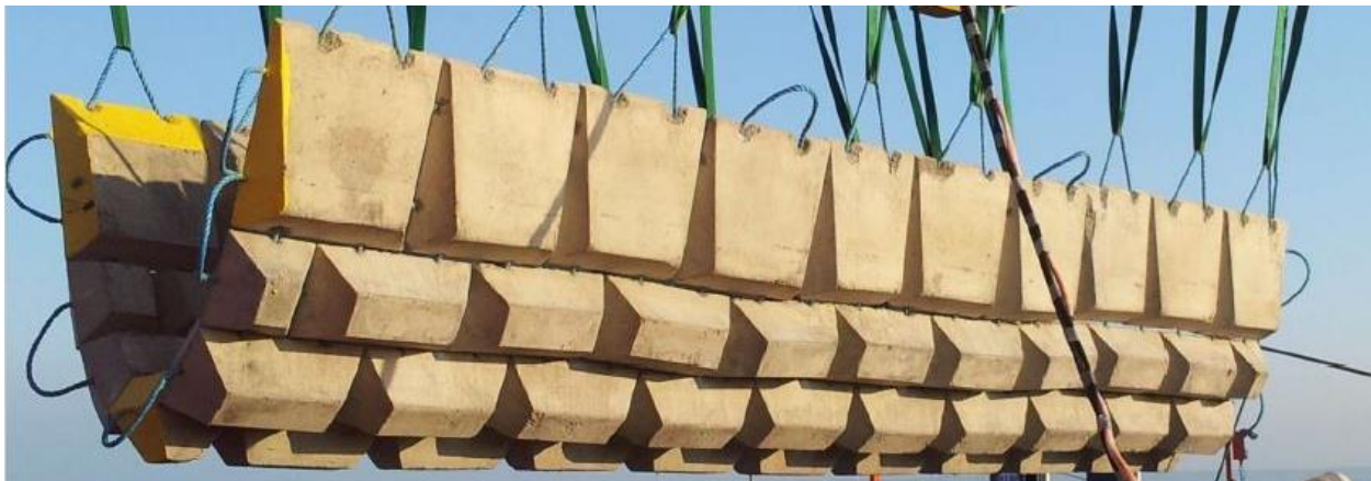
FIGURE 3-31. EXAMPLE OF CONCRETE CABLE PROTECTION MATTRESS
