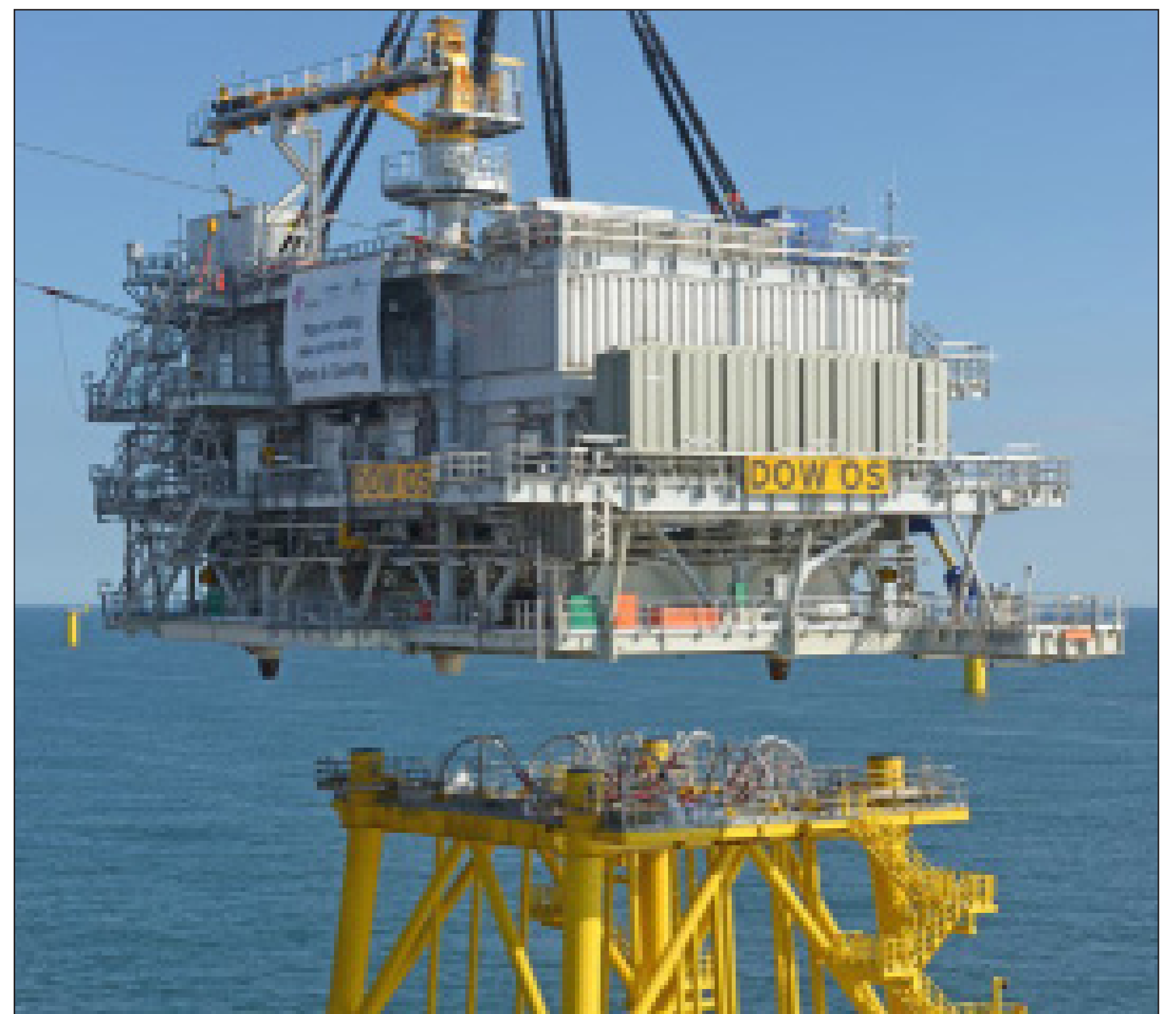
Installation of Offshore Substation
