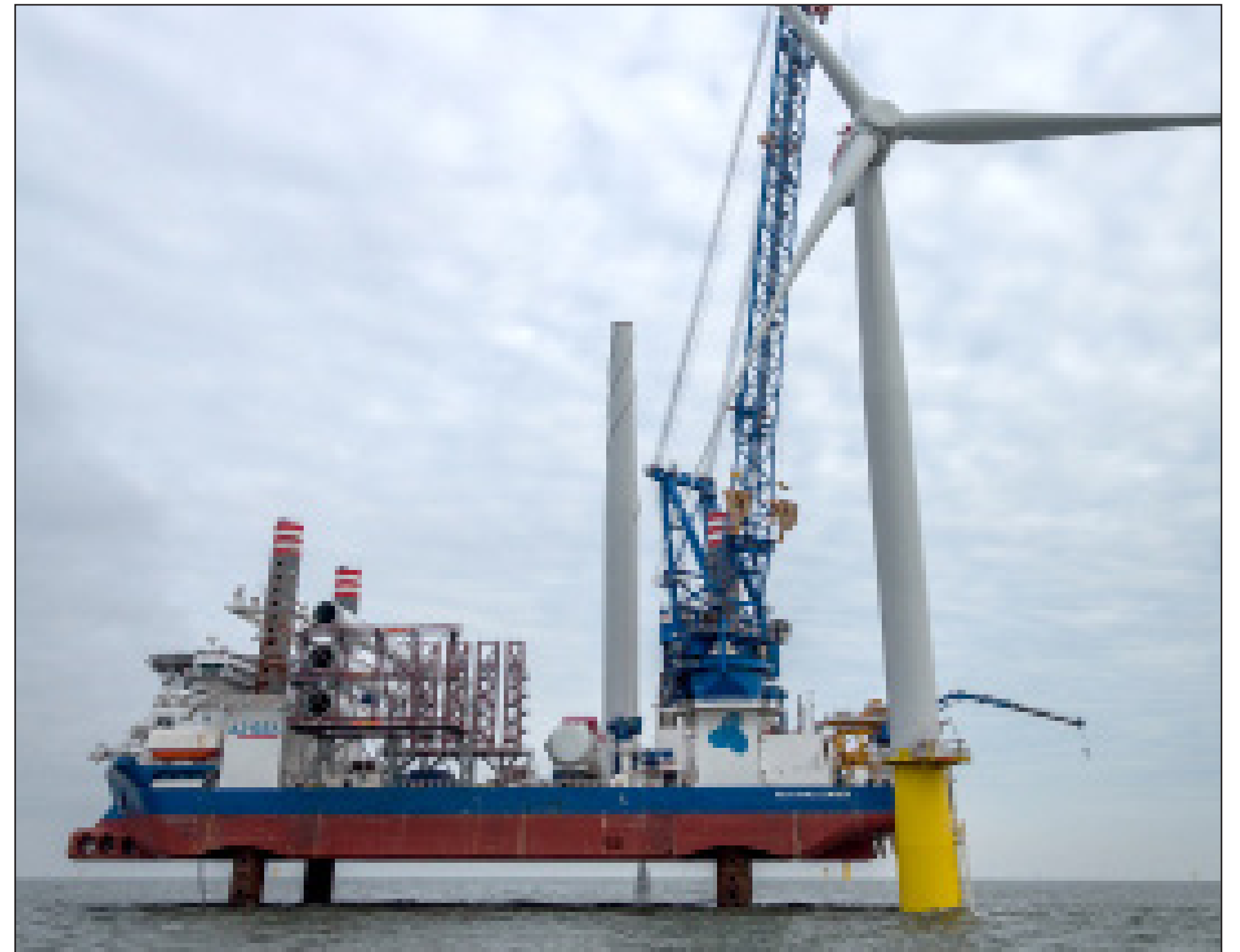
Wind Turbine Installation
