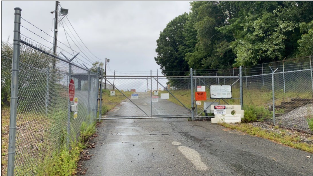
Figure 2.2-3. Overview of the potential Arthur Kill Road Substation and/or Converter Site at the Western Staten Island Substation entrance (no access). View to the northwest.
