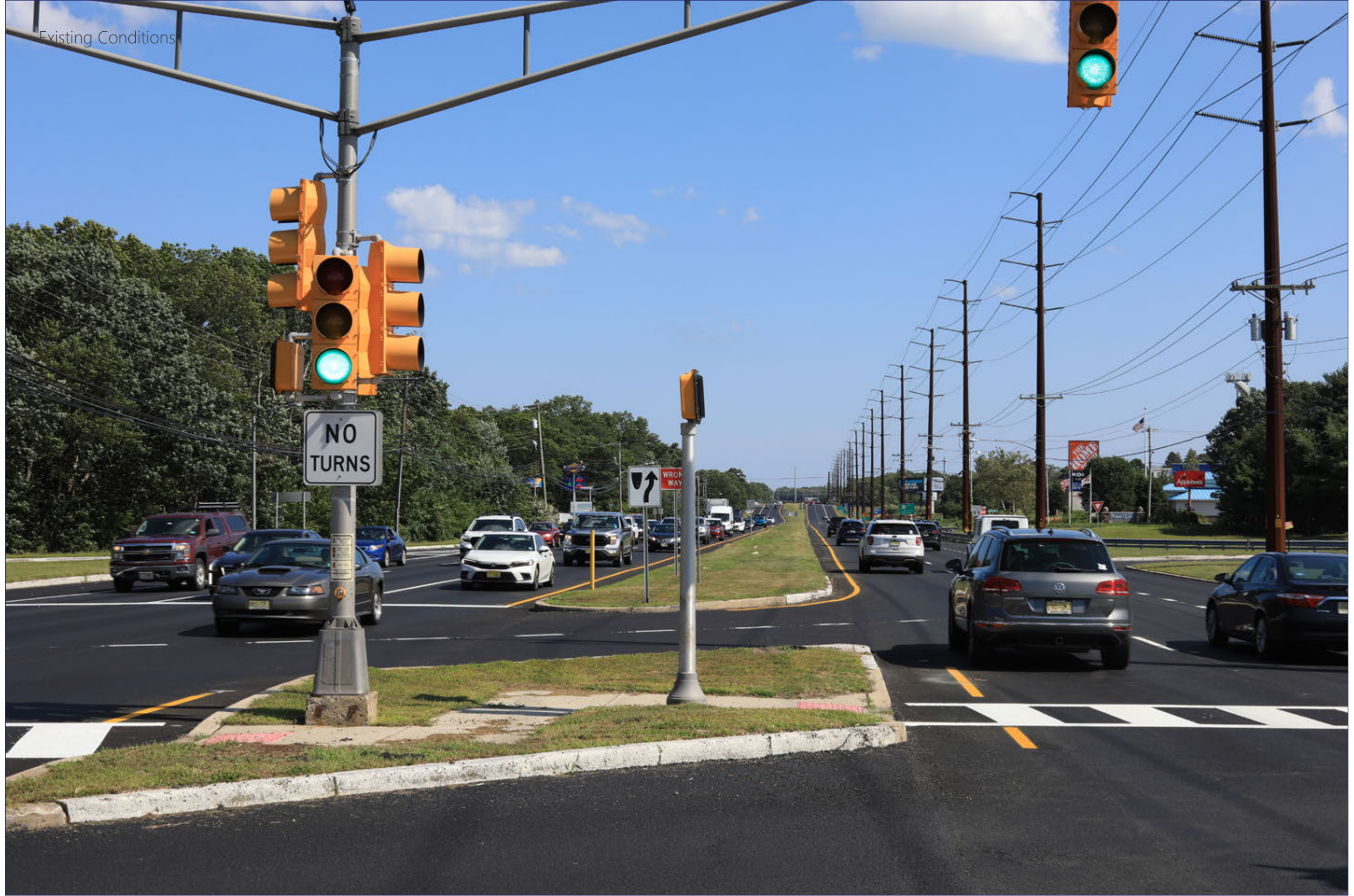
Atlantic Shores Offshore Wind: North (OCS-A 0549)
