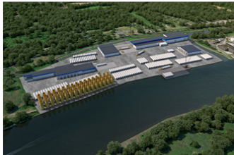
Port of Coeymans: Gravity Based Foundation Manufacturing
