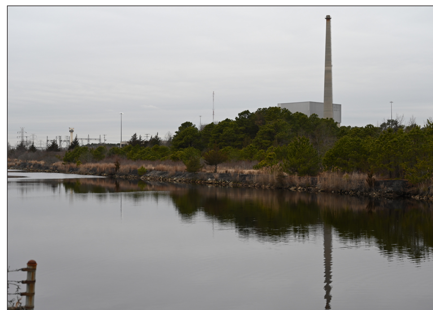
Oyster Creek Generating Station, adjacent to the proposed Oyster Creek Substation location
