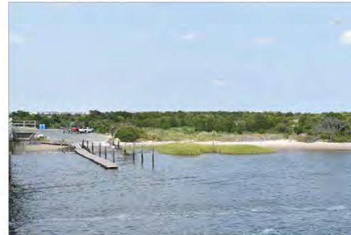
1. View looking northeast from Rush Chatten Bridge toward Corson's Inlet State Park.
