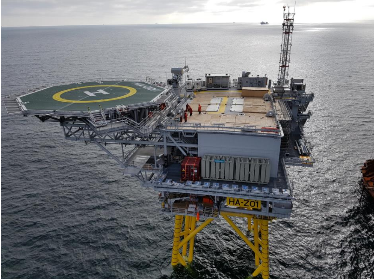
Figure C-3 Example of a Reactive Compensation Station (Hornsea I)
