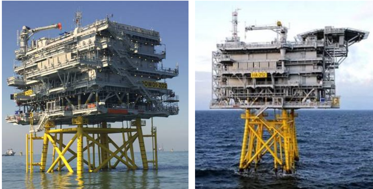
Figure 3.2 - Indicative Images of Offshore Substations.
