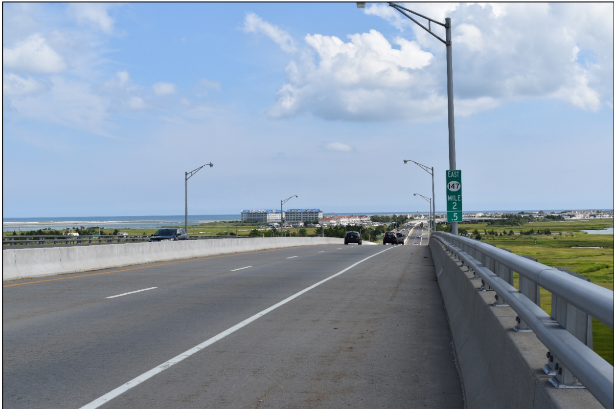
Figure 6.9 - Example of a Bridge (Route 147 towards Wildwood, NJ).
