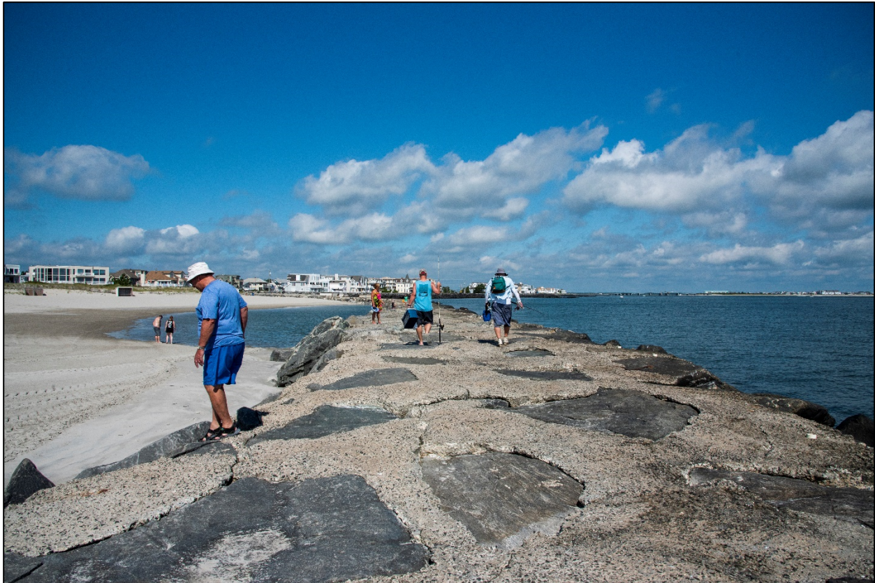
Figure 6.2 - Example of Jetty/Seawall (Avalon, NJ).
