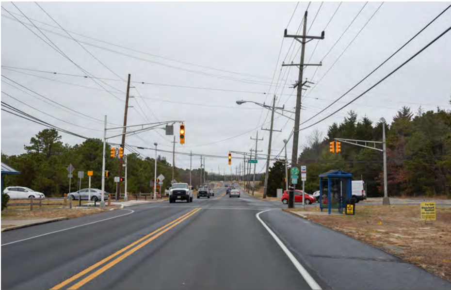
011 Ocean Township - Proposed Underground Cable Route to Oyster Creek, Bay Parkway N
