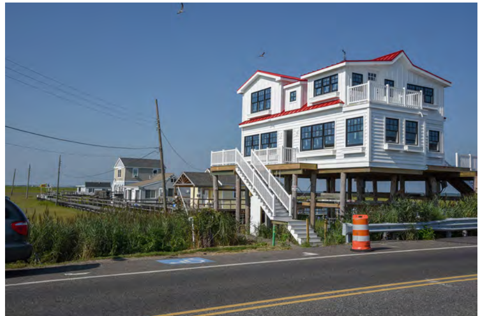
390 Middle Township - Atlantic City Railroad Cape May Division Historic District SW
