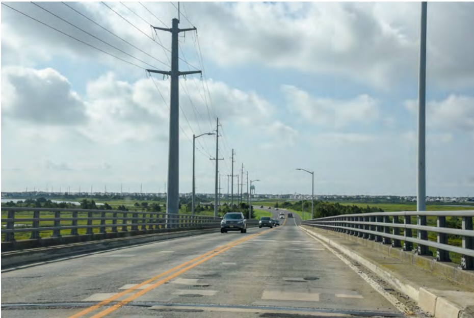
377 Avalon - Route 201 Bridge, Avalon Boulevard SE
