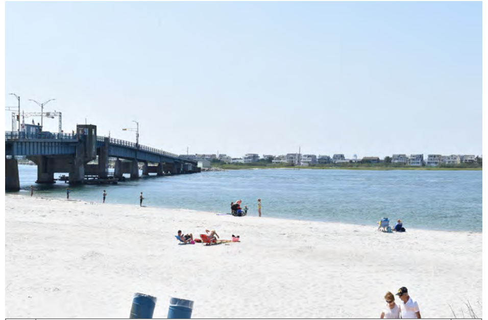
349 Sea Isle City - Townsend Inlet Park, Townsend Inlet Bridge S
