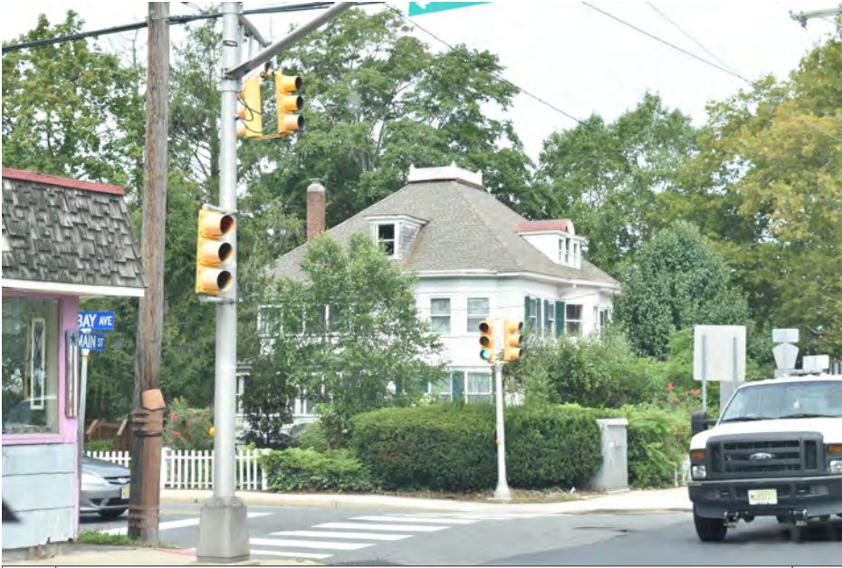
032 | Barnegat Township - Barnegat Historic District, Main Street at Bay Avenue | N
