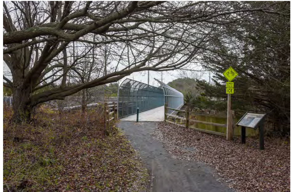
004 | Lacey Township - Barnegat Trail Pedestrian Bridge over Forked River | S
