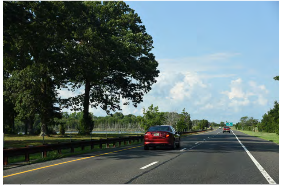
458 Lower Township - Garden State Parkway, Historic Resource N
