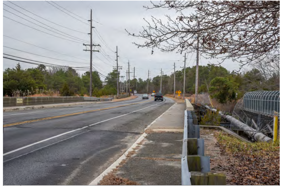
006 | Lacey Township - Oyster Creek Route, Route 9 Bridge over Forked River | S
