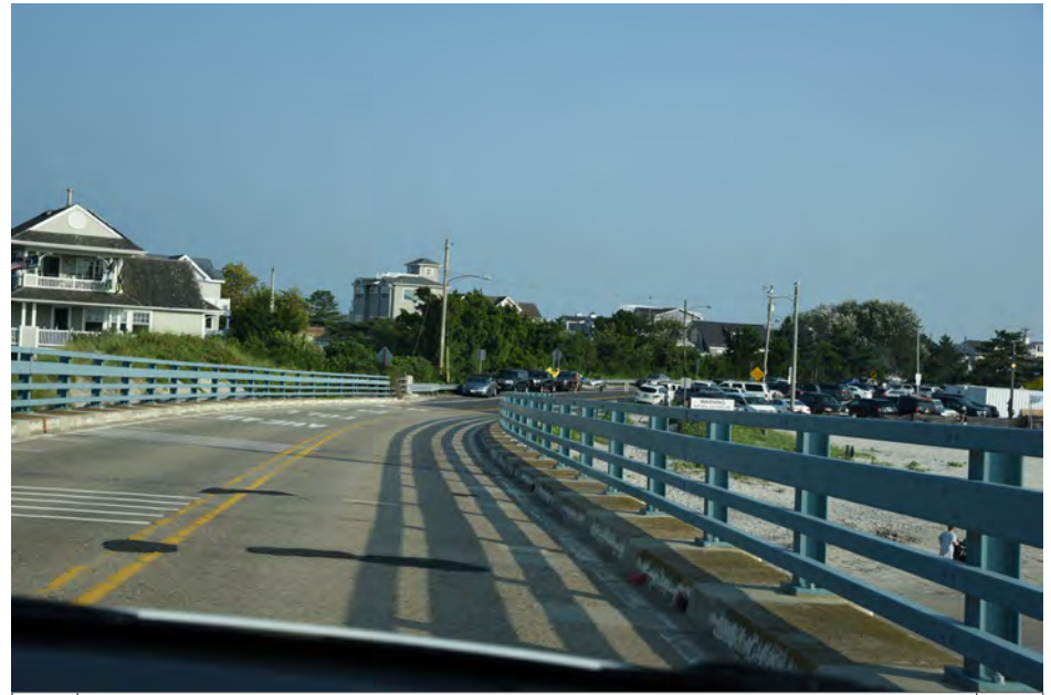
316 Upper Township - Corson's Inlet Bridge, toward Deauville Inn, Bay Avenue S
