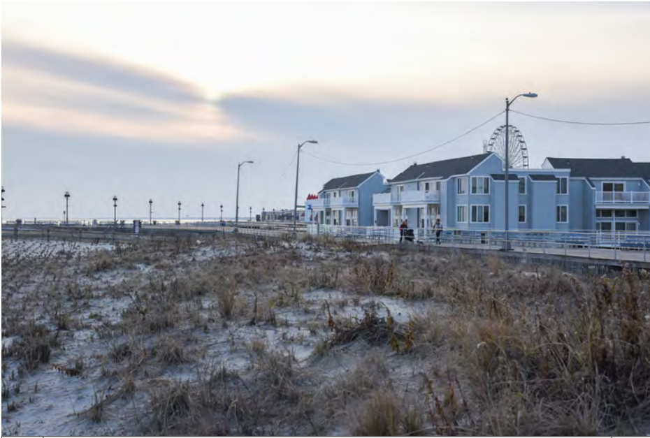
264 Ocean City - Beach Access, 4th Street SW
