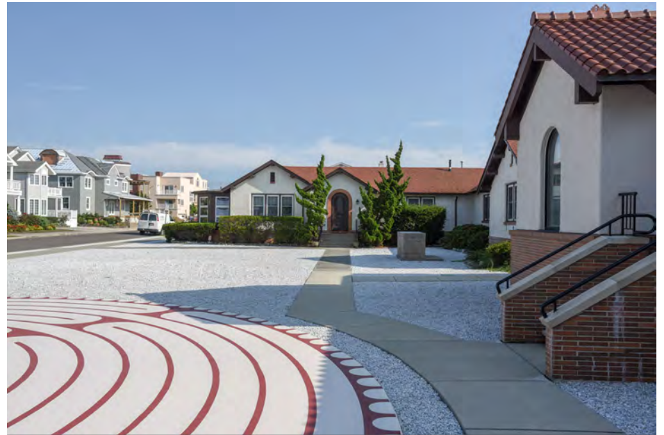
236 Longport - Church of the Redeemer SE
