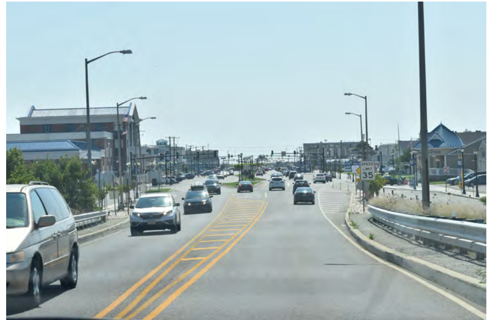
355 Sea Isle City - John F. Kennedy Boulevard entering Sea Isle City SE
