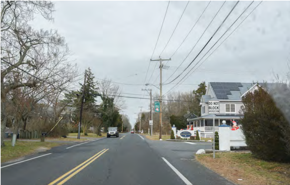
017 Ocean Township - Proposed Underground Cable Route to Oyster Creek, Main Street, Route 613 N
