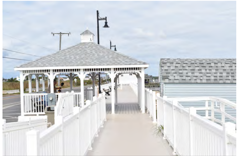
035 | Barnegat Township - Barnegat Beach | N
