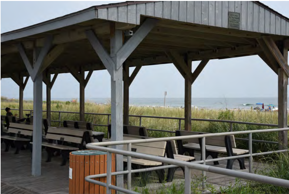
208 Ventnor City - Boardwalk Pavilion, at South Cambridge Avenue E
