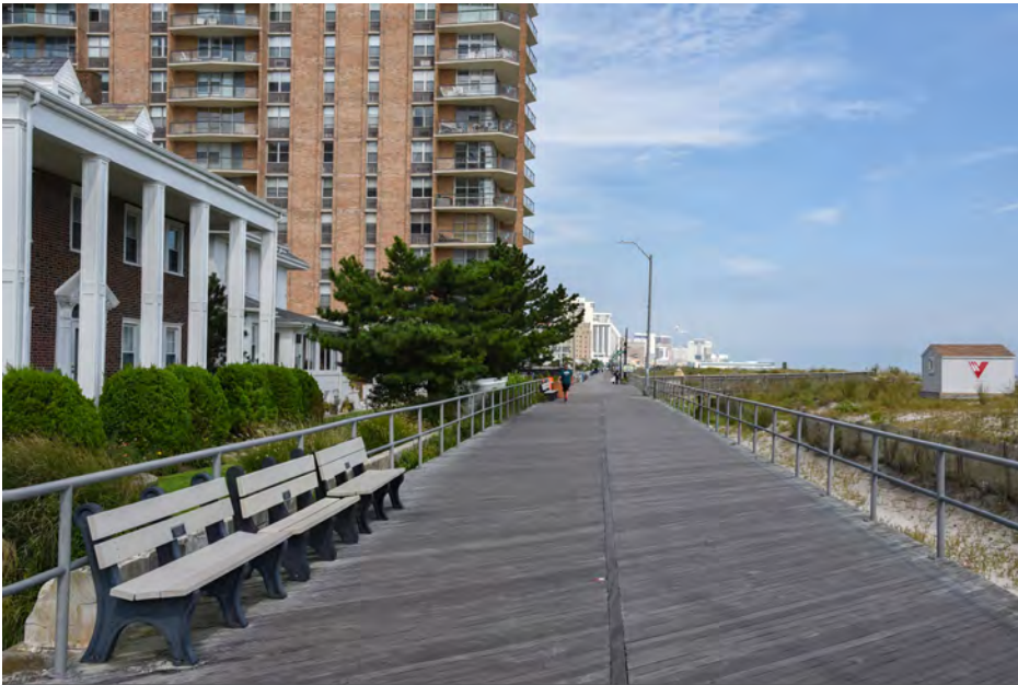
201 | Ventnor City - Boardwalk, at South Marion Avenue | NE
