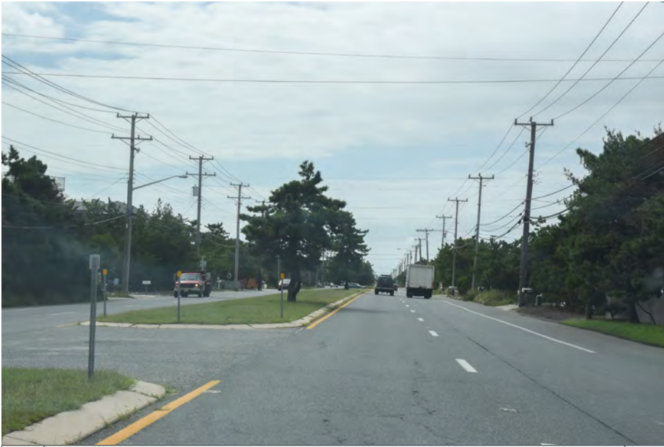
048 Long Beach Township (North Beach) - Long Beach Boulevard SW
