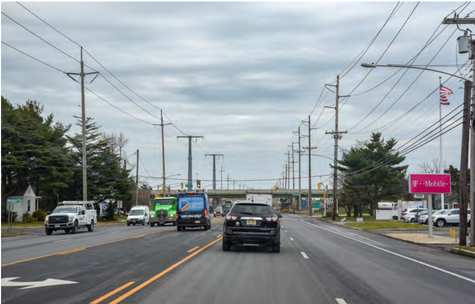
302 Upper Township - Proposed Underground Cable Route to BL England, Roosevelt Boulevard SE
