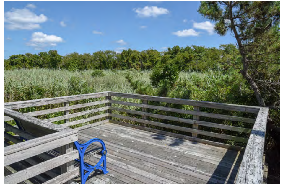
378 Avalon - Armacost Community Wildlife Observation Platform W
