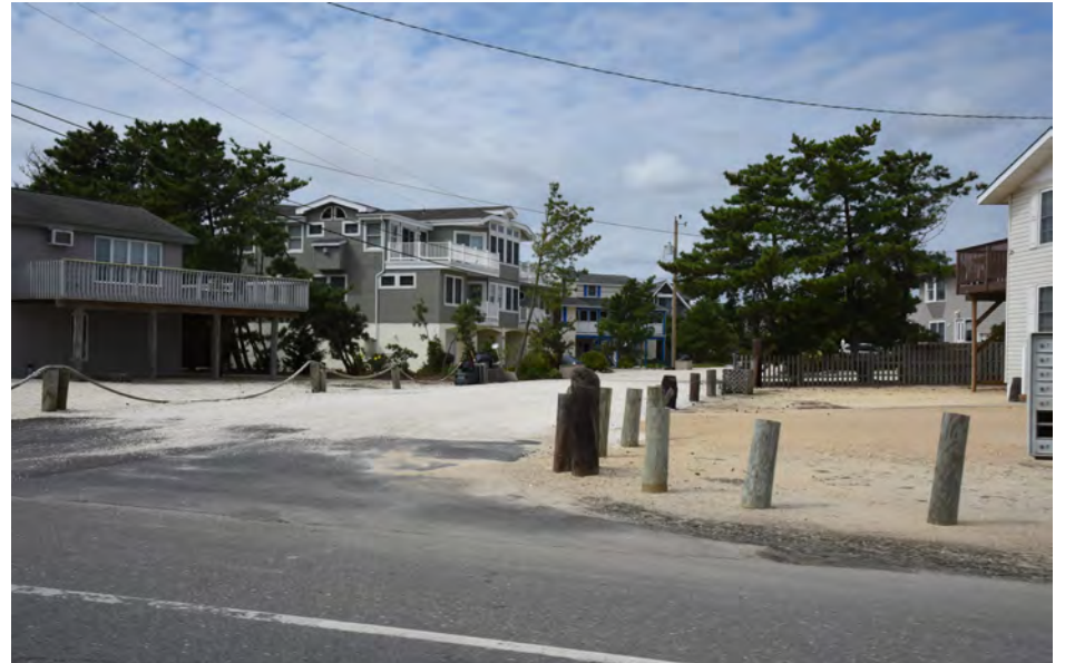
049 Long Beach Township (North Beach) - Long Beach Boulevard at Terrapin Lane W
