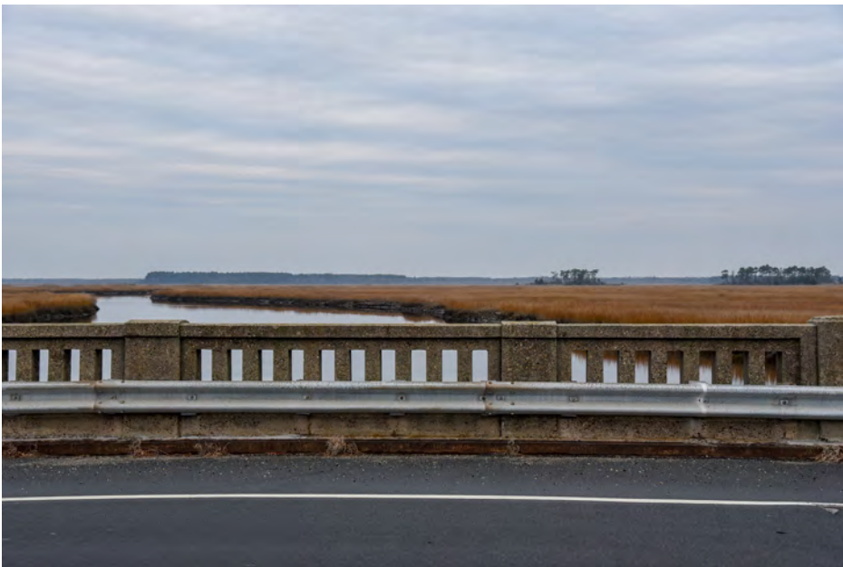
389 Middle Township - Route 47 Bridge SE
