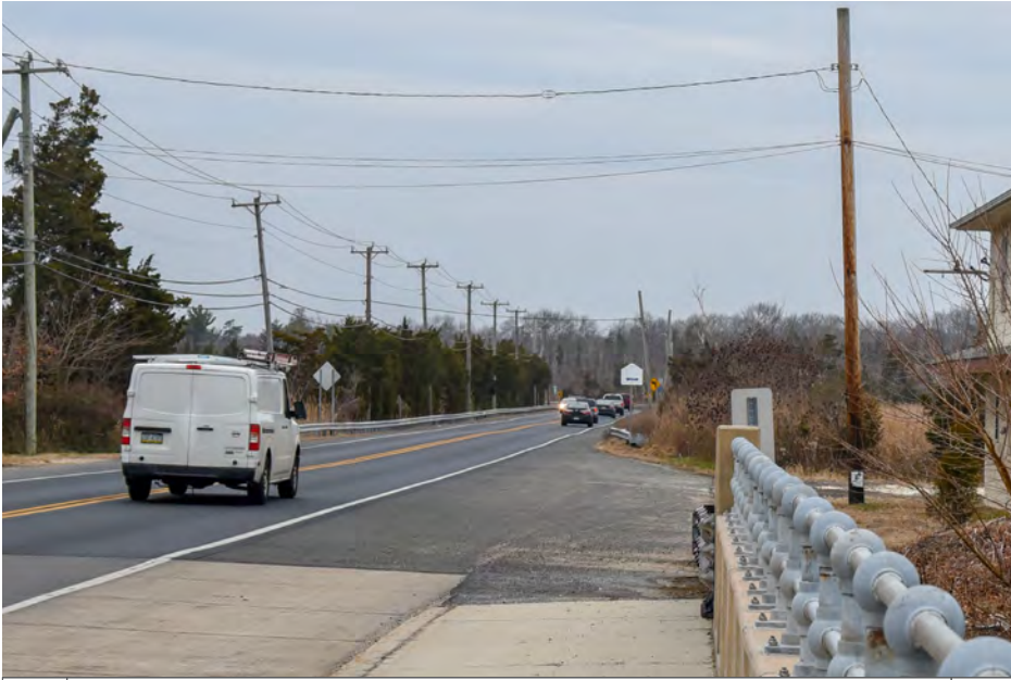
326 Dennis Township - Bridge over Dennis Creek, Route 47 N
