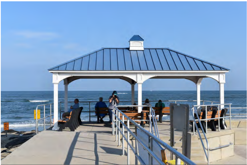
450 North Wildwood - John F. Kennedy Boulevard Pavilion SE
