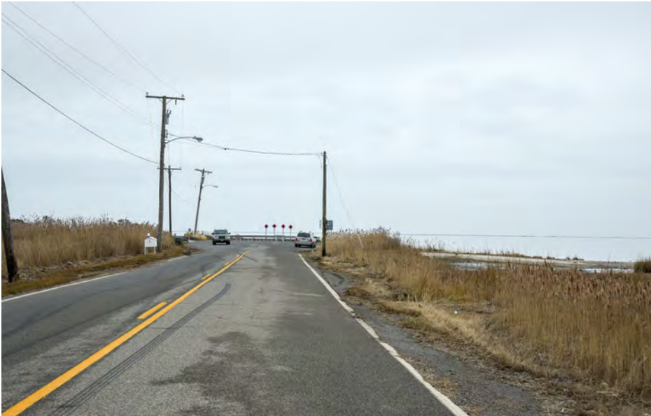
013 Ocean Township - Proposed Underground Cable Route to Oyster Creek, Bay Parkway, End of Road N
