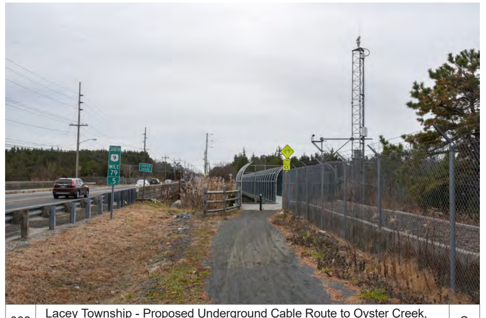
008 | Lacey Township - Proposed Underground Cable Route to Oyster Creek, Barnegat Branch Trail, Route 9, South Branch Forked River | S
