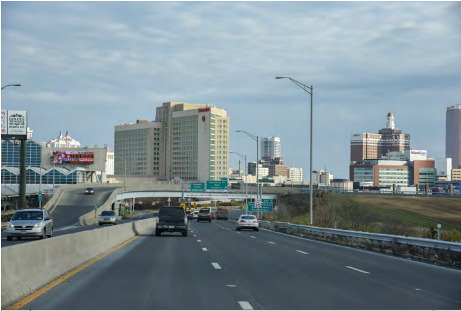
152 Atlantic City - Atlantic City Expressway E
