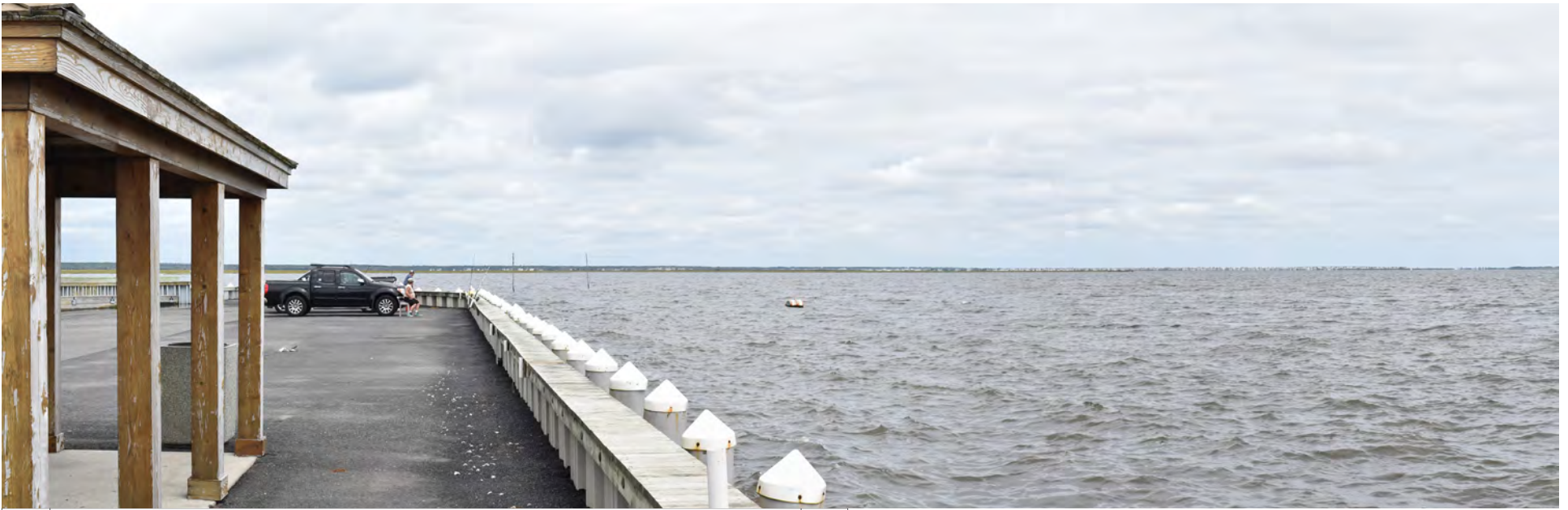
064 Eagleswood Township - Dock Road Pavilion, Edwin B. Forsythe Conservation Area N
