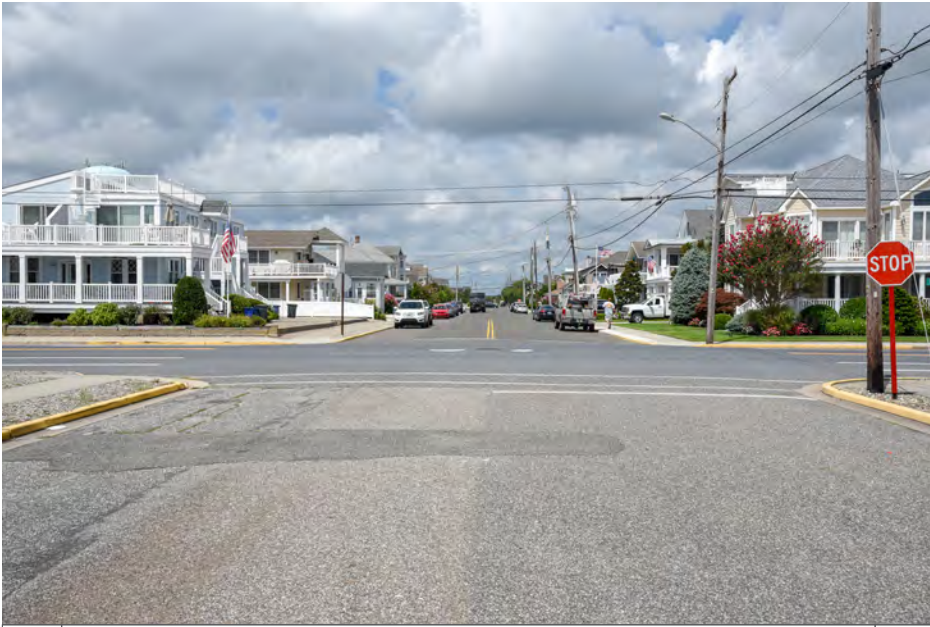
360 Avalon - 37th Street at First Avenue, toward bay NW
