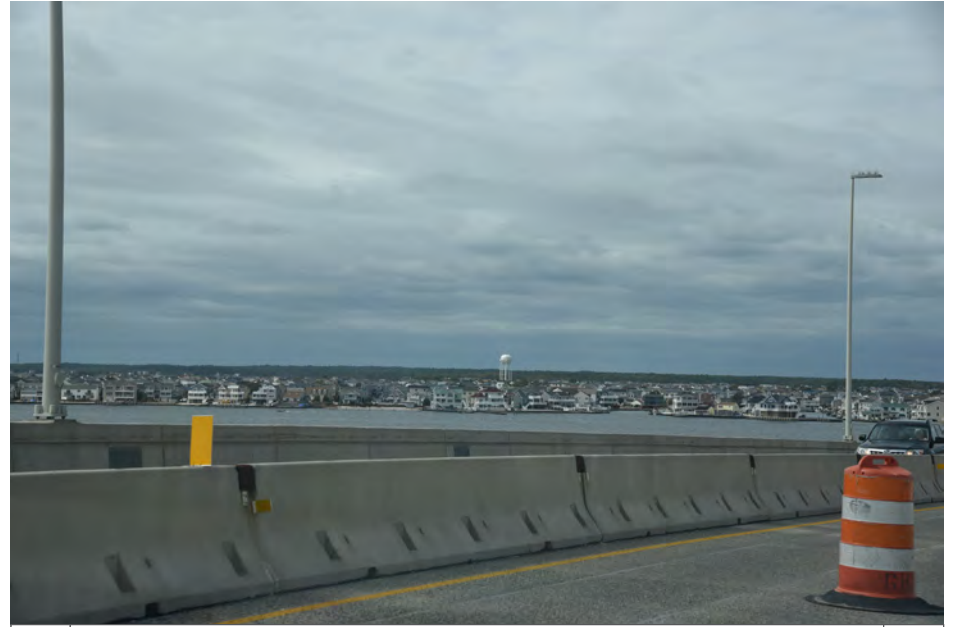
045 Stafford Township - Dorland J. Henderson Memorial Bridge SE
