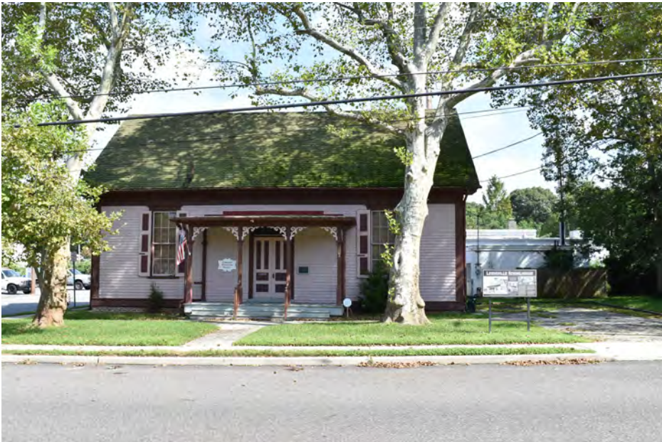
216 Linwood - Leedsville Schoolhouse, Historic Resource SE
