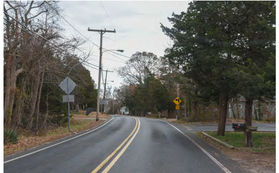
014 Ocean Township - Proposed Underground Cable Route to Oyster Creek, Bryant Road S
