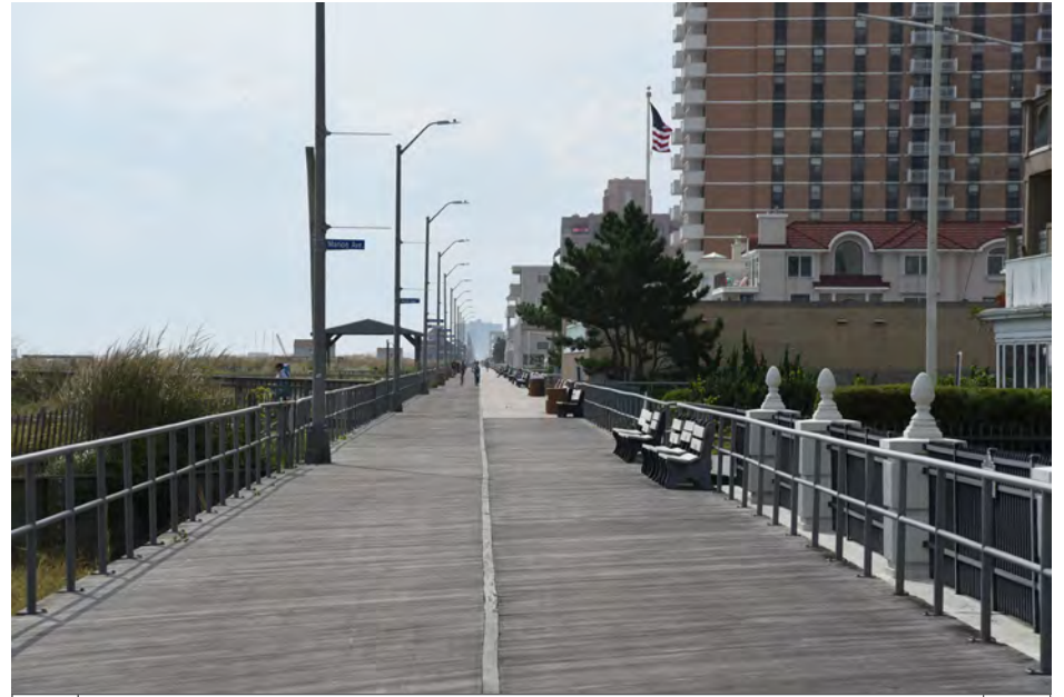
200 | Ventnor City - Boardwalk, at South Baton Rouge Avenue | SW
