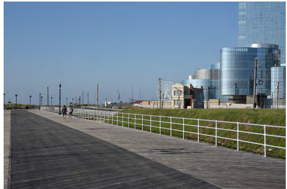
163 Atlantic City - Atlantic City Boardwalk at New Hampshire Street | SW
