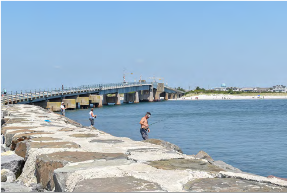
371 Avalon - Townsend Inlet Bridge, Ocean Drive N
