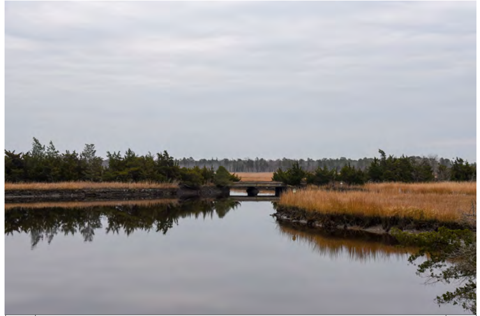
327 Dennis Township - Bridge over Dennis Creek, Route 47 E
