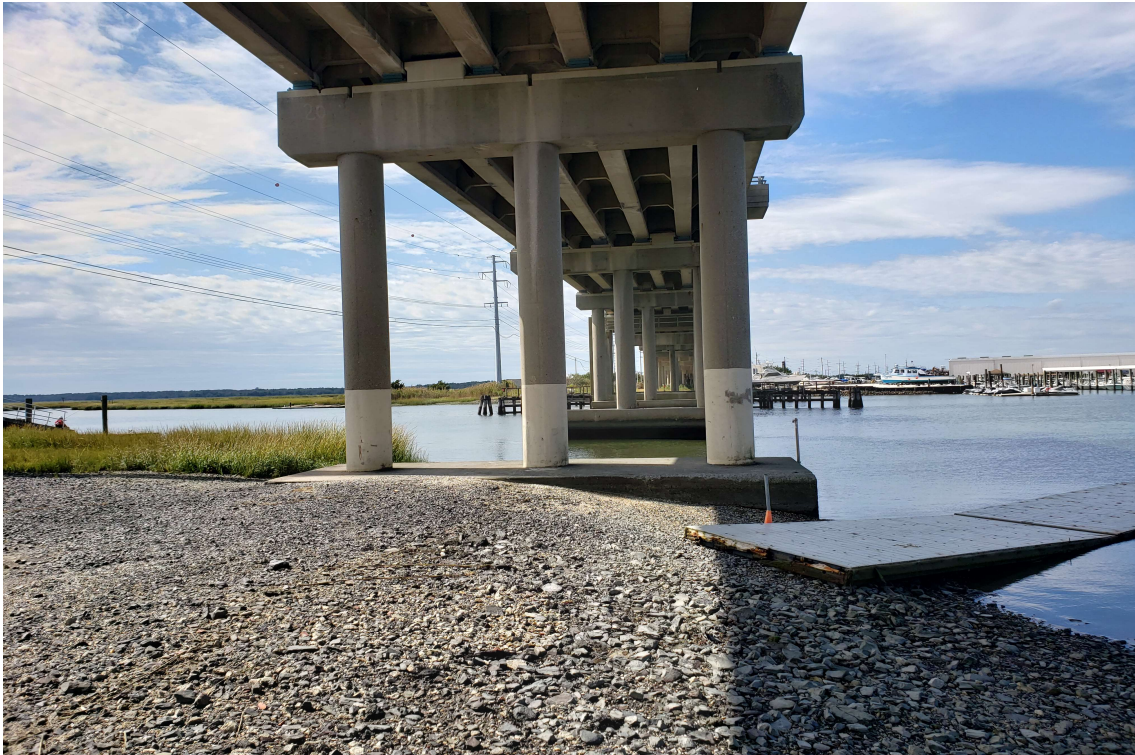
Photo 9: Viewing northwest at the proposed HDD crossing area of Crook Horn Creek, marina in background, public fishing access in foreground right.
