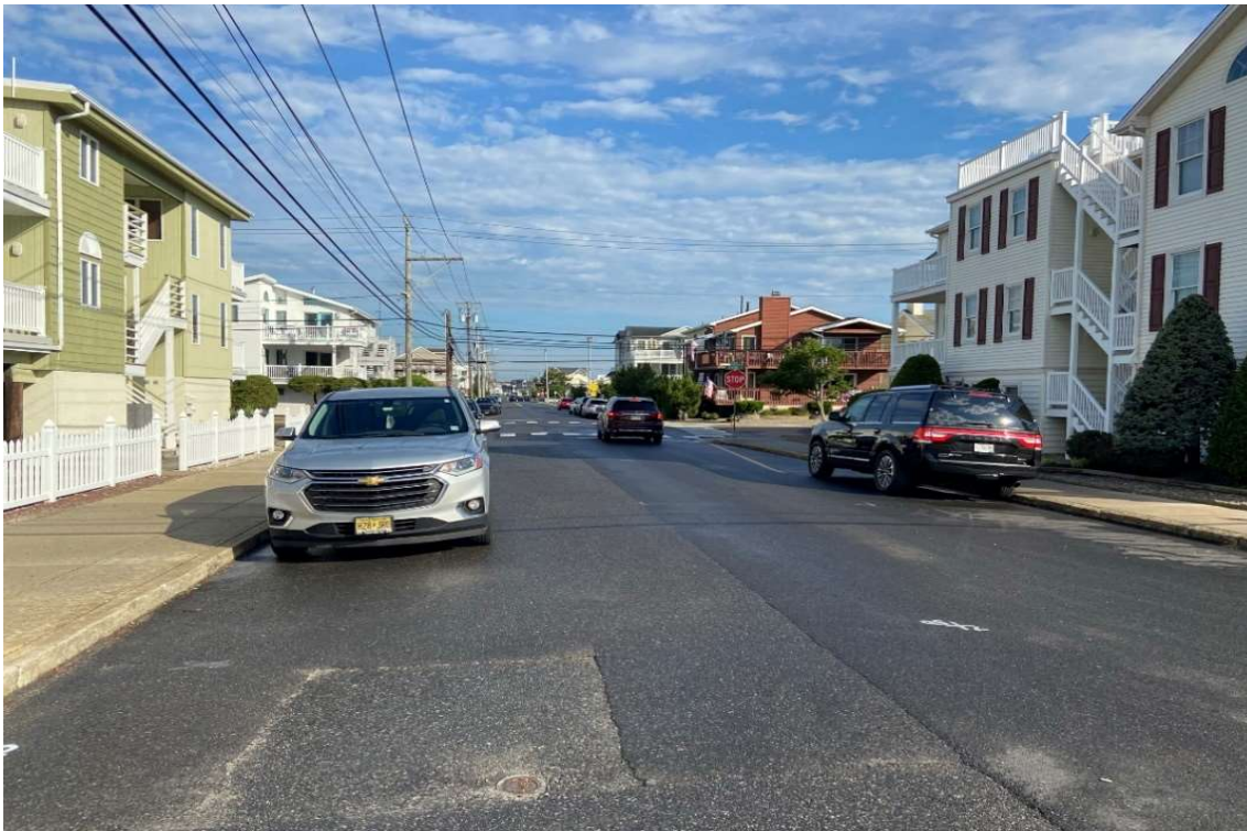
Photo 2: Viewing west northwest at the proposed transition joint bay HDD landing area of 35th Street from the beach access area
