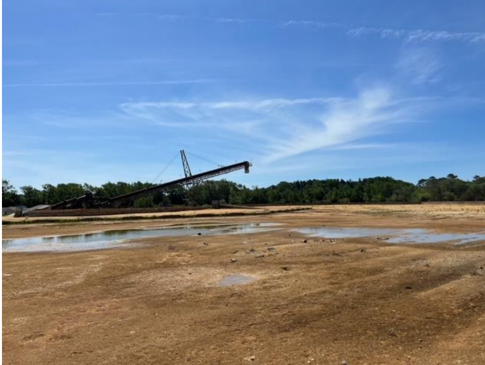
Photo 5 – Former coal storage area with portion of old conveyor system.
