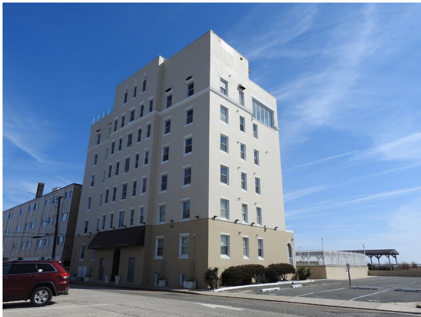
Photo Description: Northwest and southwest elevations, facing east.
