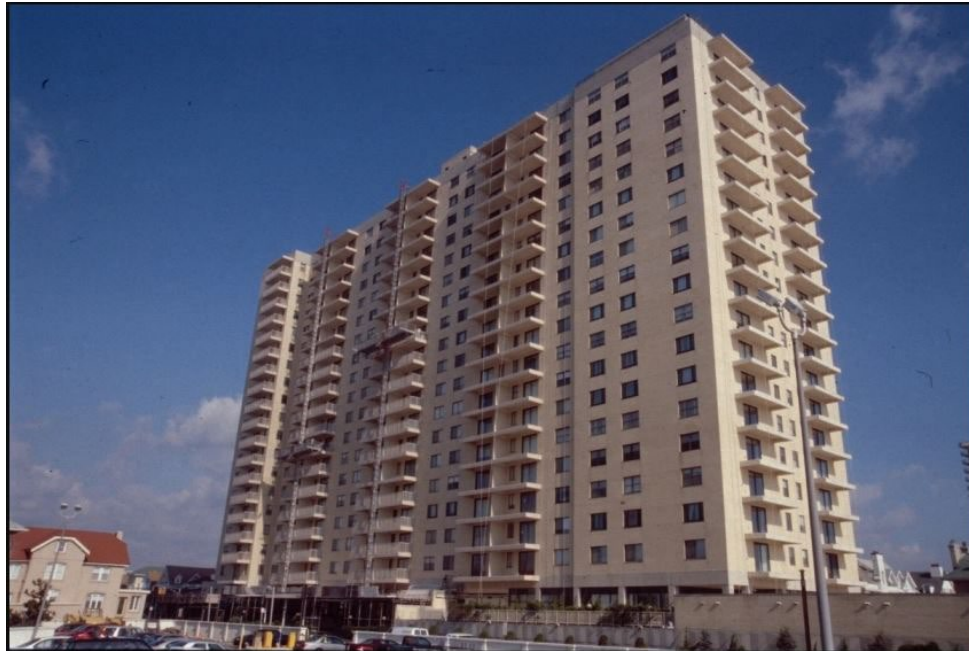
Figure 3. Undated image of 5000 Boardwalk during balcony replacement (Becica & Associates LLC n.d.)
