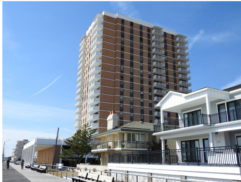
Photo Description: Regency Towers, 5200 Boardwalk, view to the southwest.
