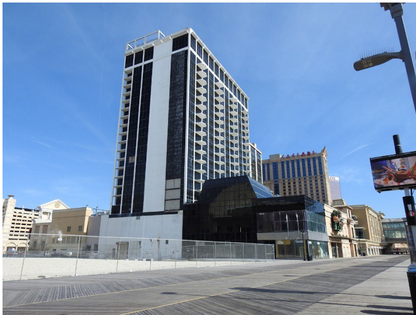
Photo Description: Holiday Inn of Atlantic City, 2201 Boardwalk, view to the northeast.
