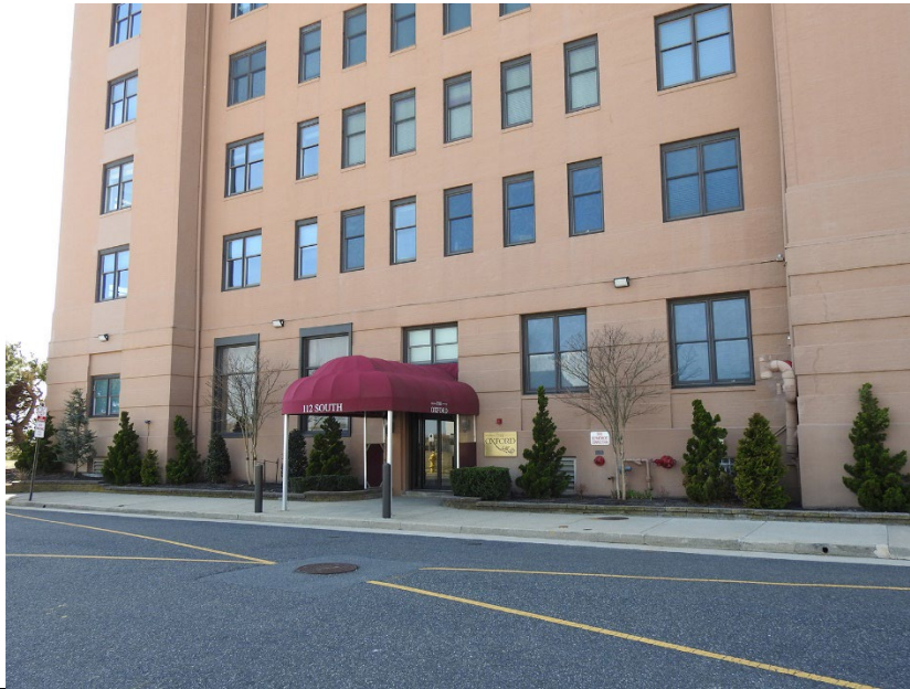
Photo Description: Entry on northeast elevation, facing south.
