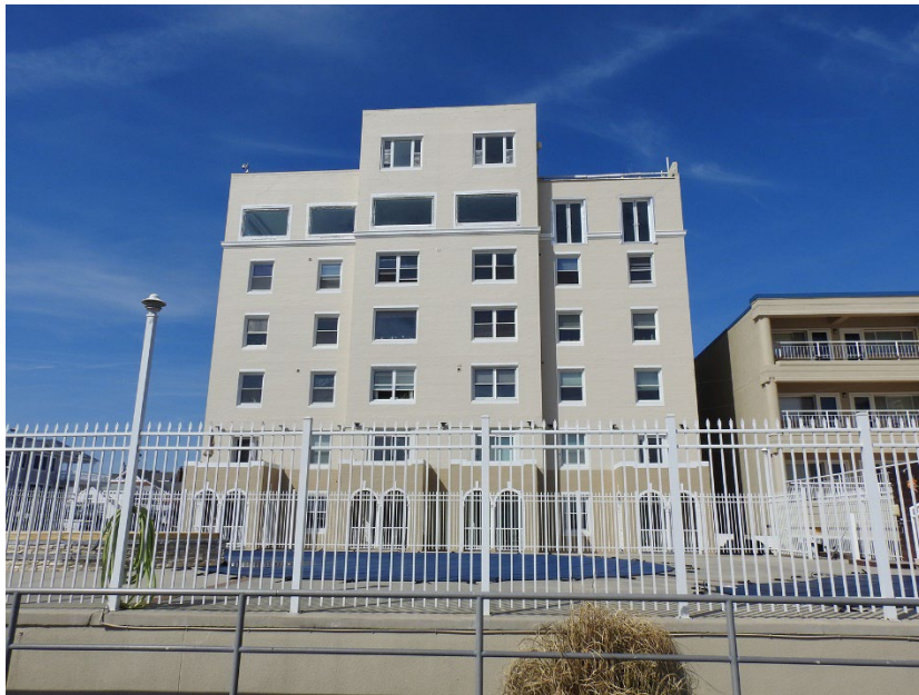
Photo Description: Southeast elevation, facing northwest.
