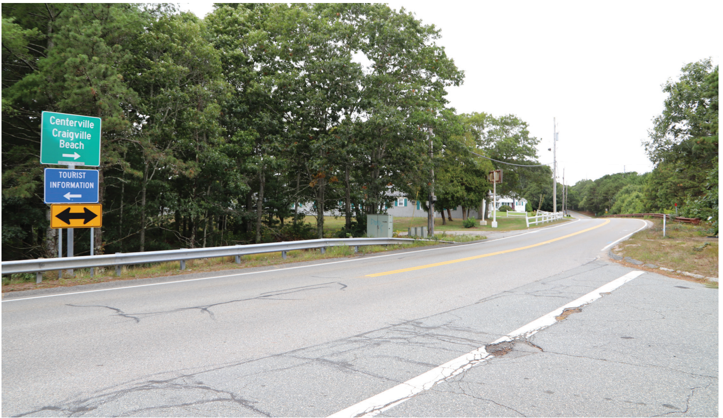
VP1 - Shootflying Hill Road at Route 6 Eastbound Exit Ramp
