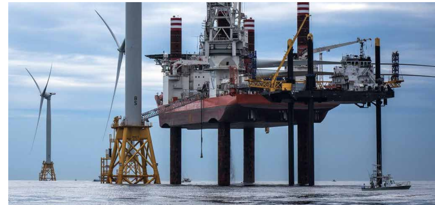
Offshore WTG installation Vessel (Source: ESS Group, Inc)
