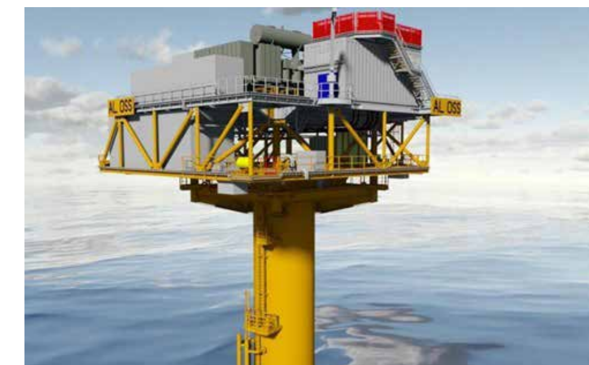
Conceptual OSS atop a Monopile Foundation
