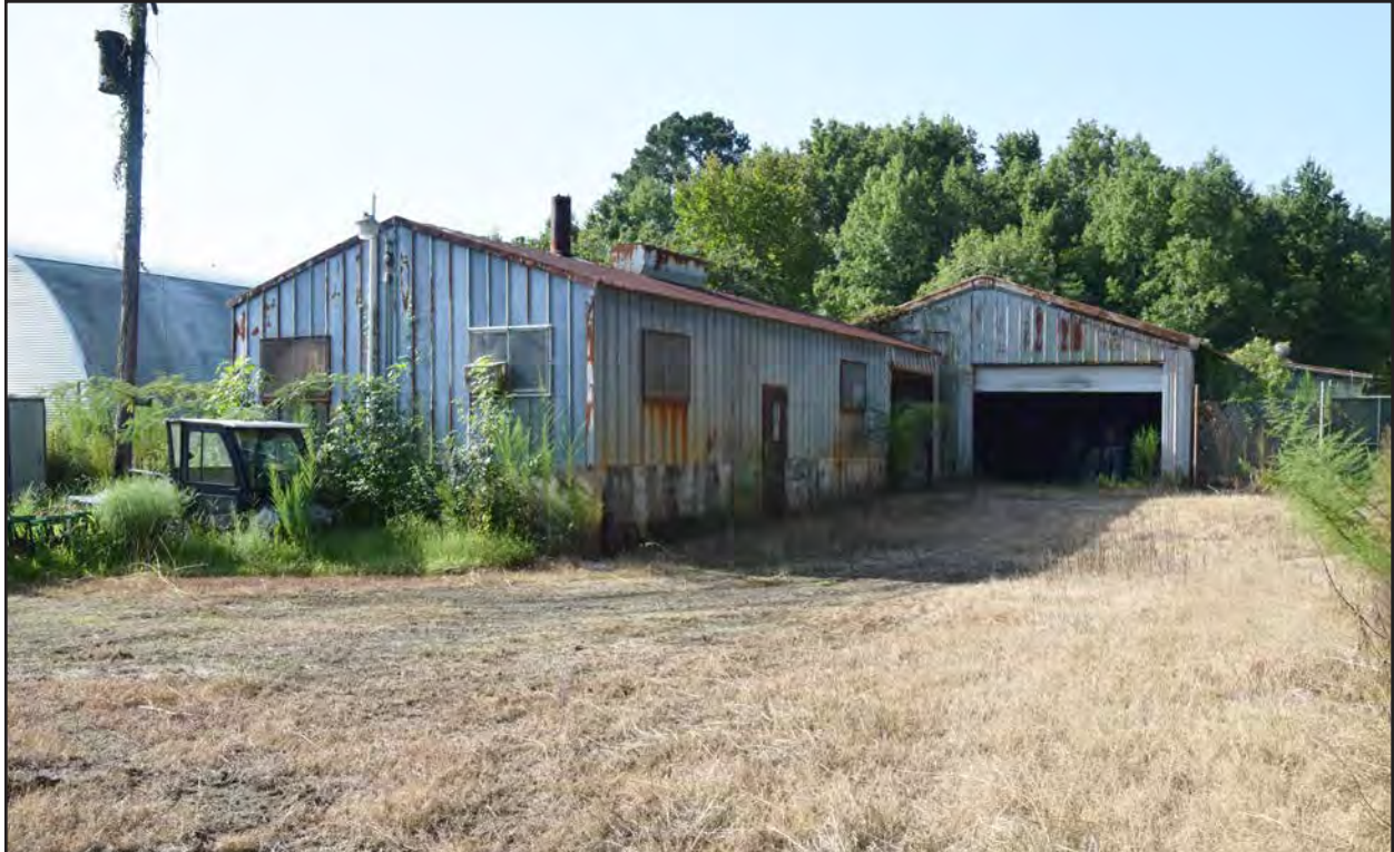
Figure 176. 134-5937, equipment shed, northeast and northwest elevations, view to the south.
