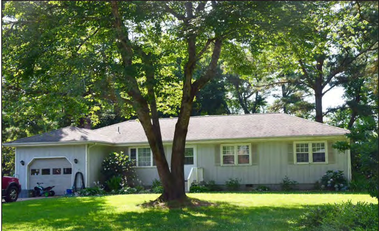
Figure 82. 131-6199, linear Ranch, northwest elevation, view to the southeast.
