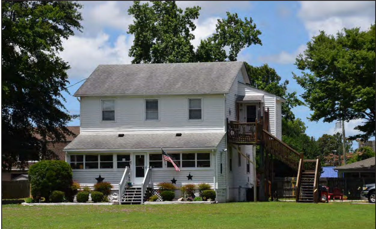
Figure 168. 134-0162, dwelling, south and east elevations, view to the northwest.
