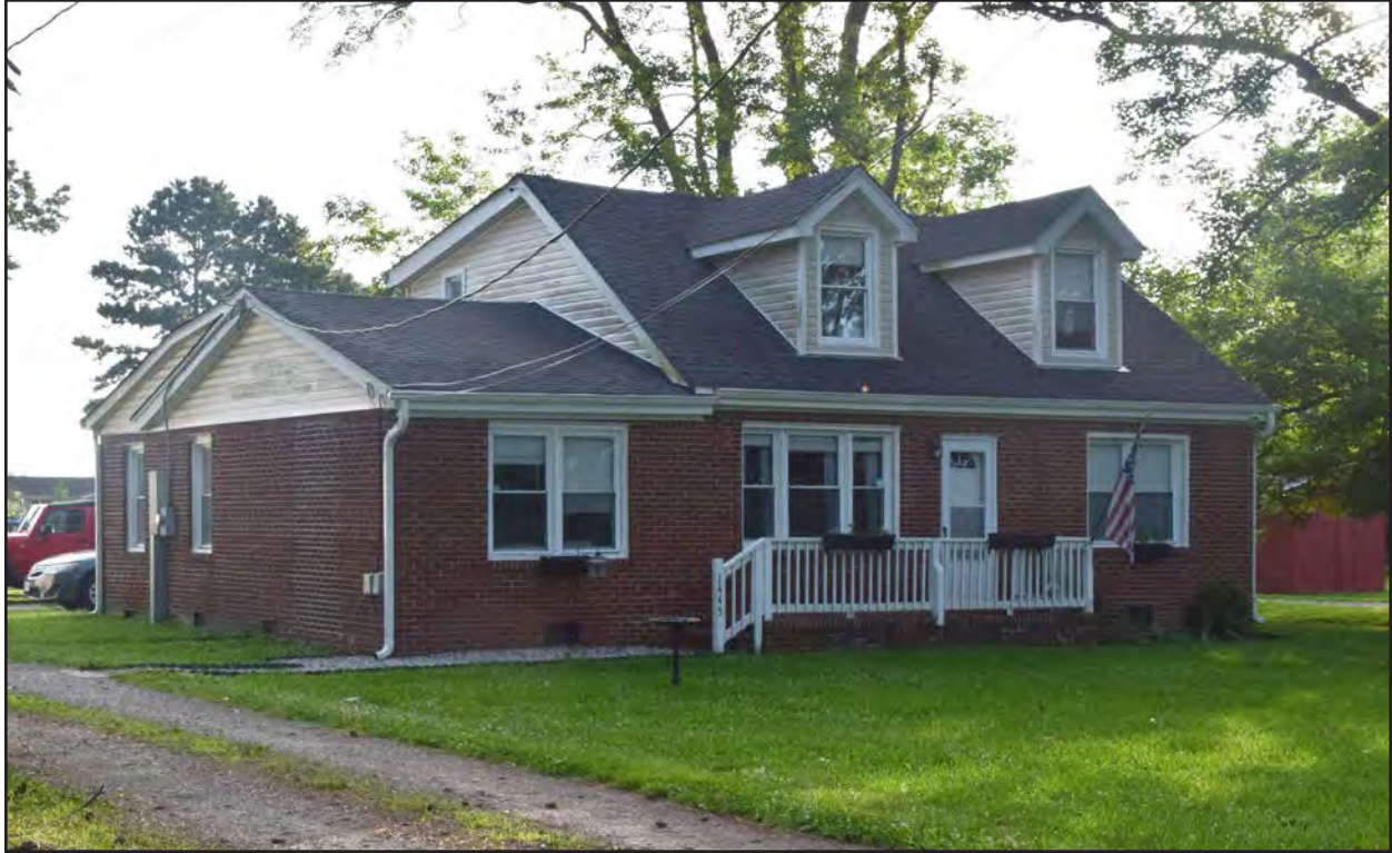
Figure 37. 131-5985, Cape Cod dwelling, southwest and northwest elevations, view to the east.
