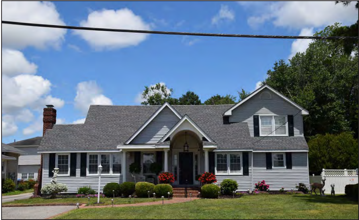
Figure 223. 134-5882, linear Ranch, south elevation, view to the north.
