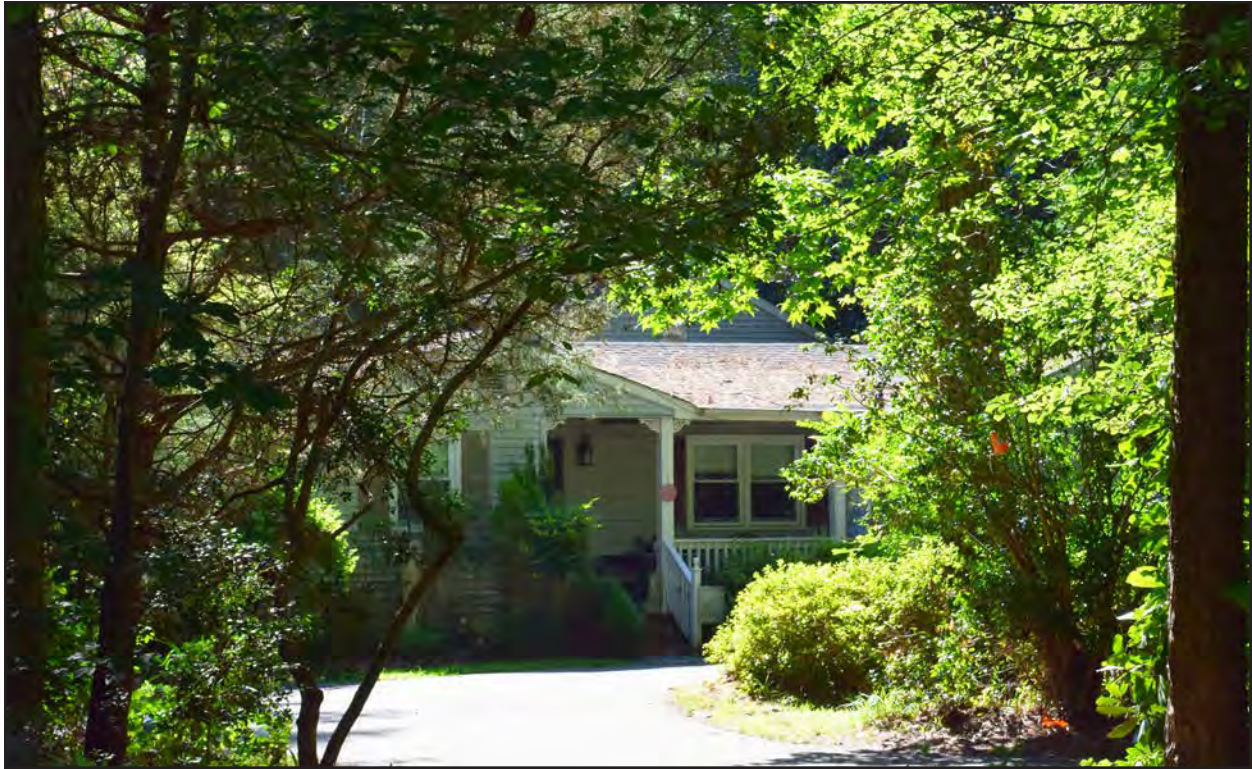
Figure 229. 134-5888, compact Ranch, west elevation, view to the east.
