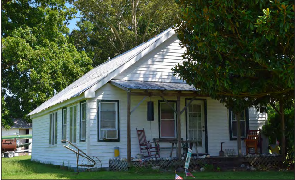
Figure 55. 131-6005, vernacular secondary dwelling, southeast elevation, view to the northwest
