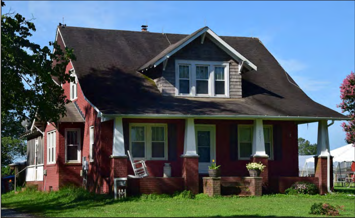
Figure 19. 131-5435, Mount Pleasant Farms, Craftsman Bungalow, northeast and southeast elevations,
