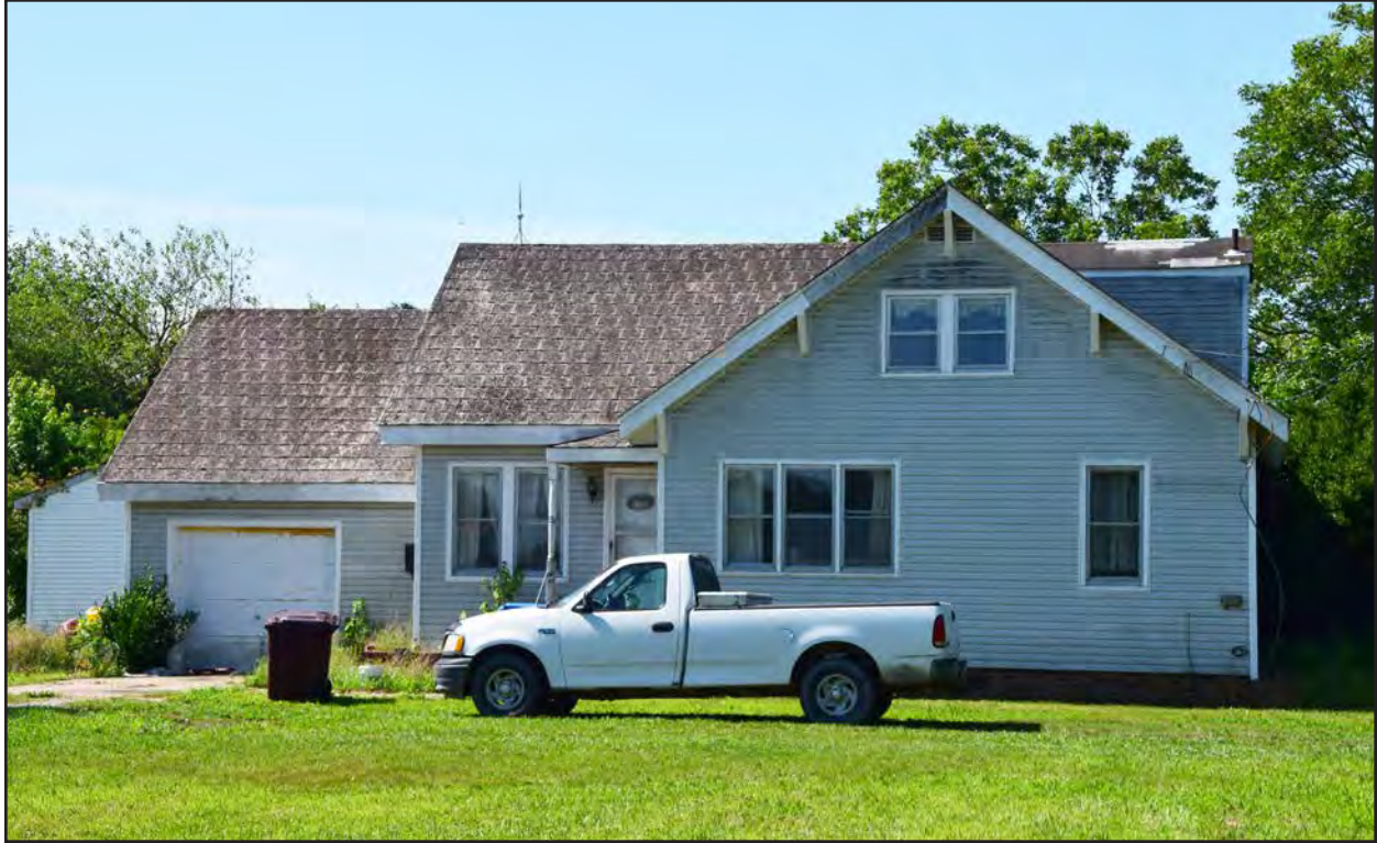
Figure 133. 131-6251, dwelling, north elevation, view to the south.
