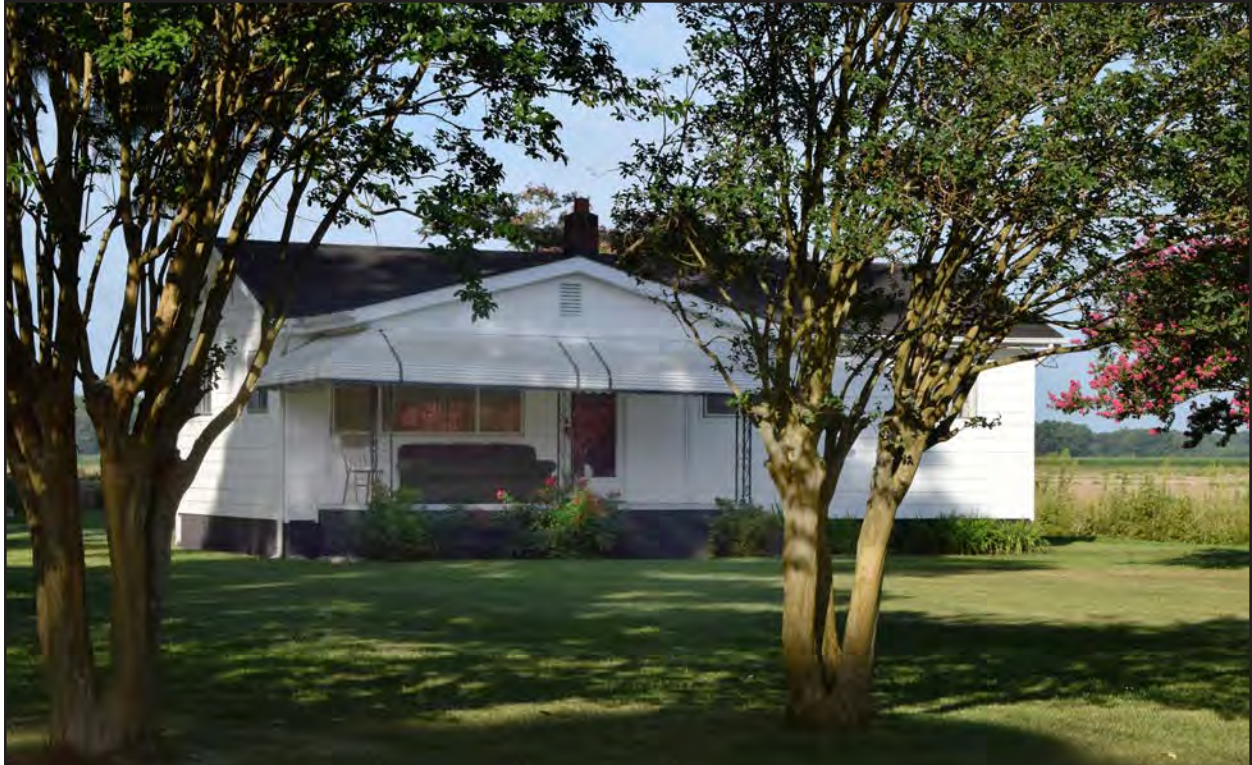
Figure 96. 131-6213, compact Ranch, northeast and southeast elevations, view to the west.
