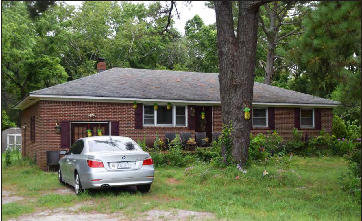
Figure 98. 131-6215, compact Ranch, southwest and northwest elevations, view to the east.
