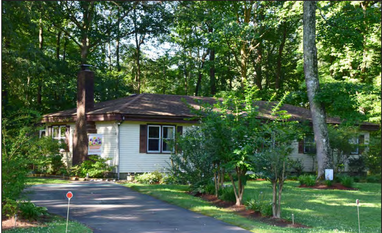
Figure 264. 134-5924, dwelling, east elevation.
