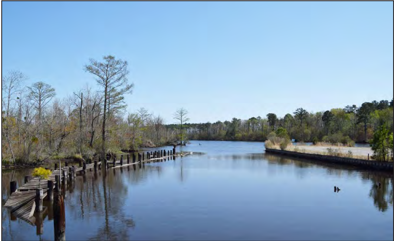
Figure 1. 131-0044/131-5333-0002, Albemarle & Chesapeake Canal, view from North Landing Road to the southeast.
