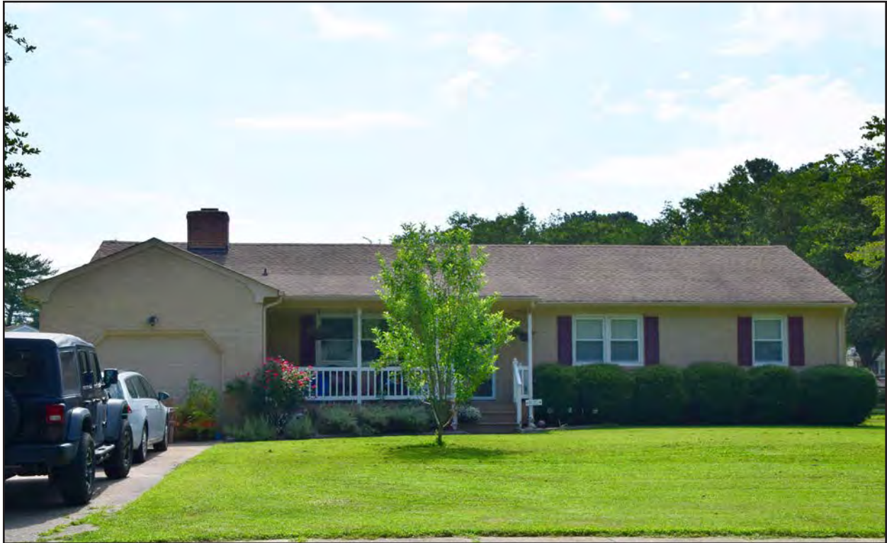
Figure 89. 131-6206, linear Ranch, west elevation, view to the east.
