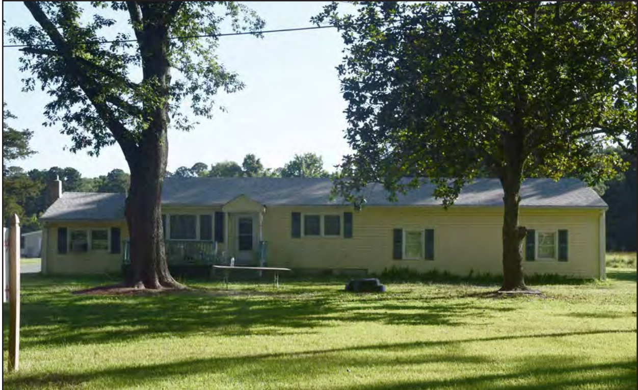
Figure 286. 134-5950, modified compact Ranch dwelling, southeast elevation, view to the northwest.
