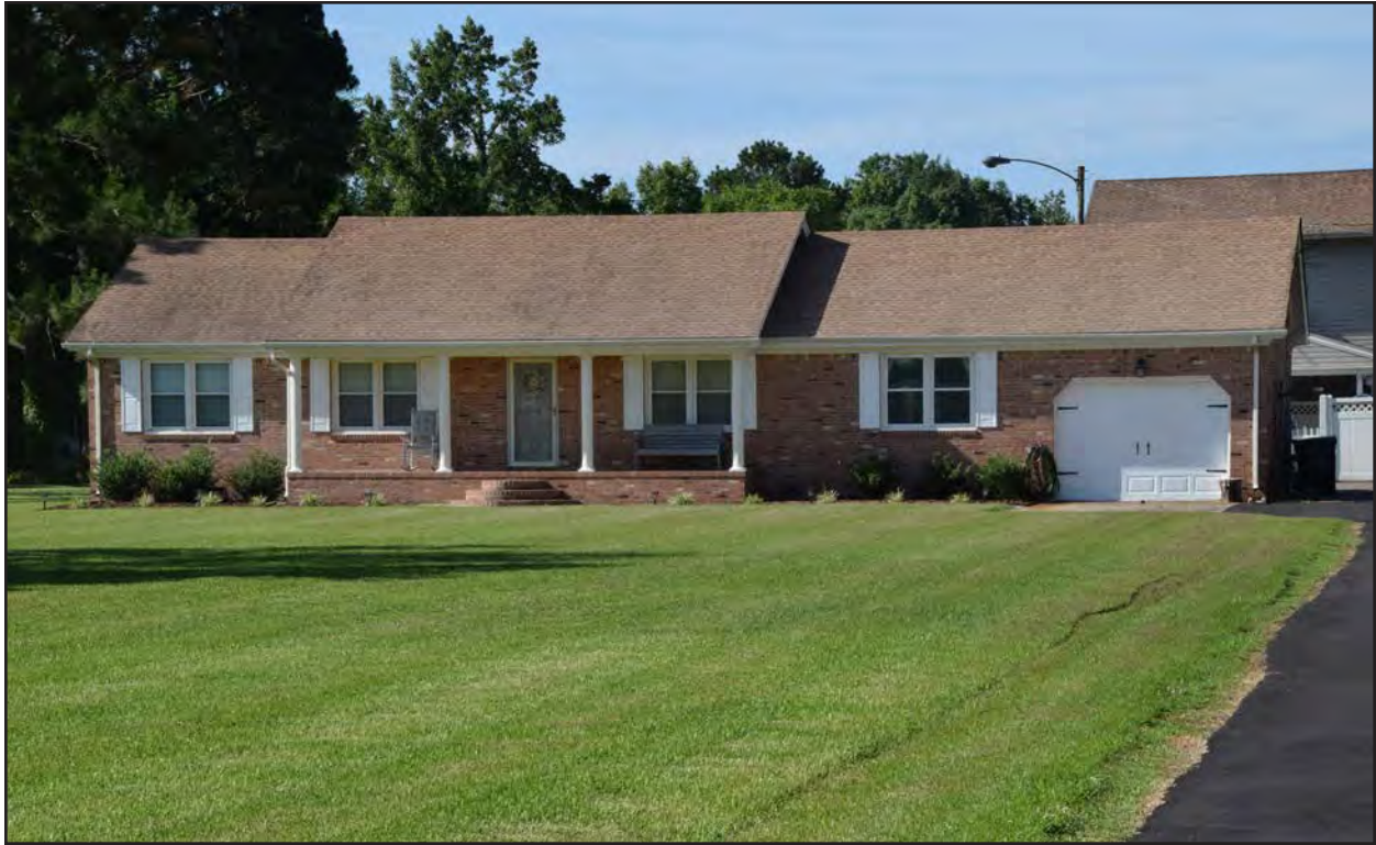
Figure 91. 131-6208, linear Ranch, north elevation, view to the south.
