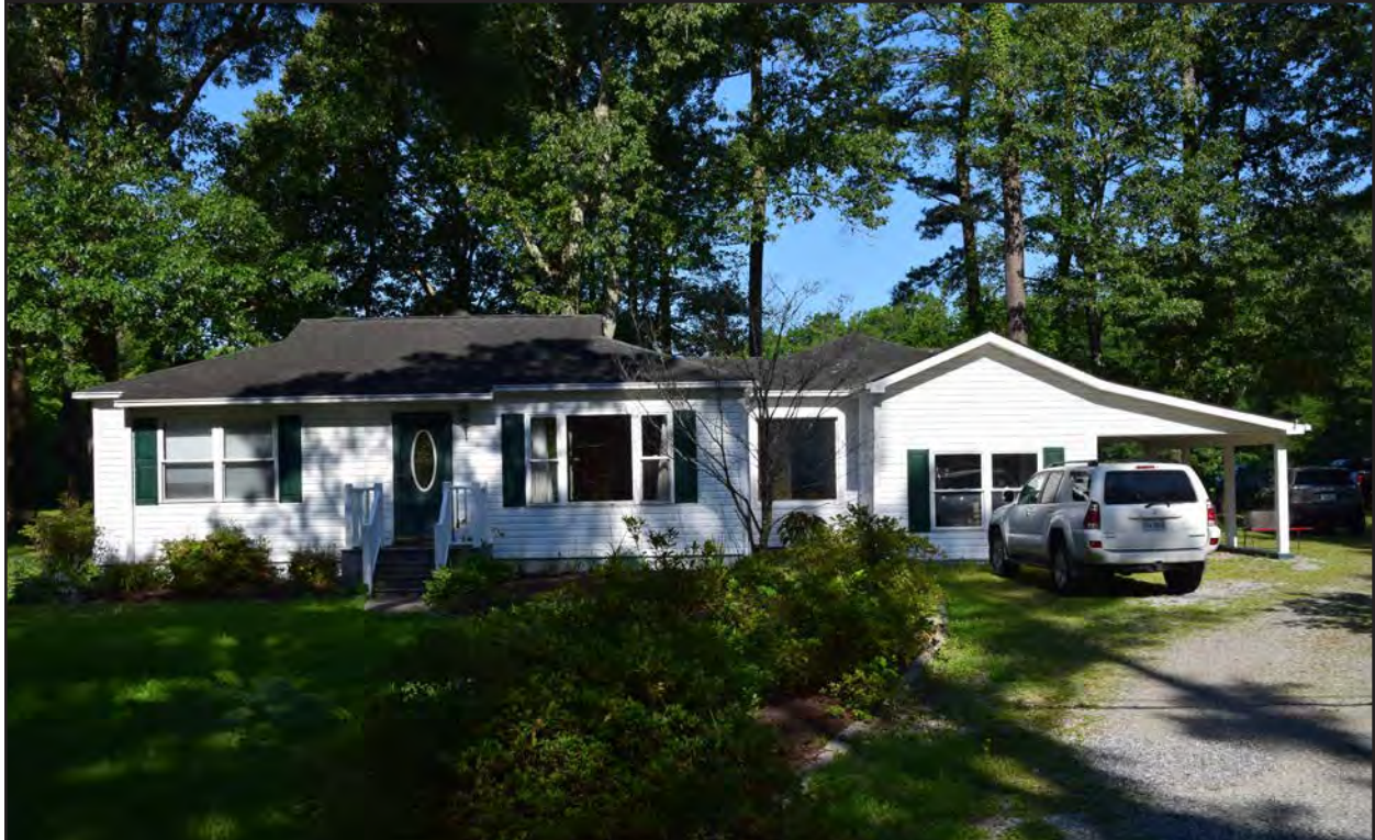
Figure 246. 134-5906, dwelling, east elevation, view to the west.
