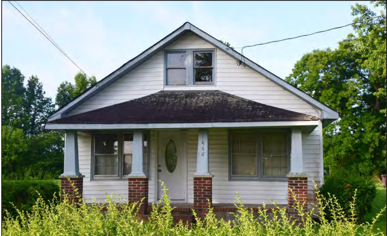
Figure 52. 131-6000, Craftsman dwelling, northeast elevation, view to the southwest.
