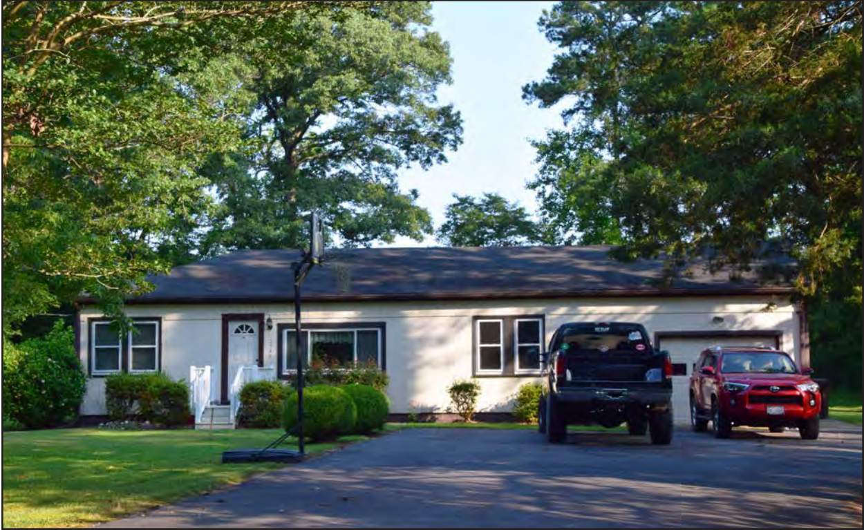
Figure 143. 131-6262, compact Ranch, southeast elevation, view to the northwest.
