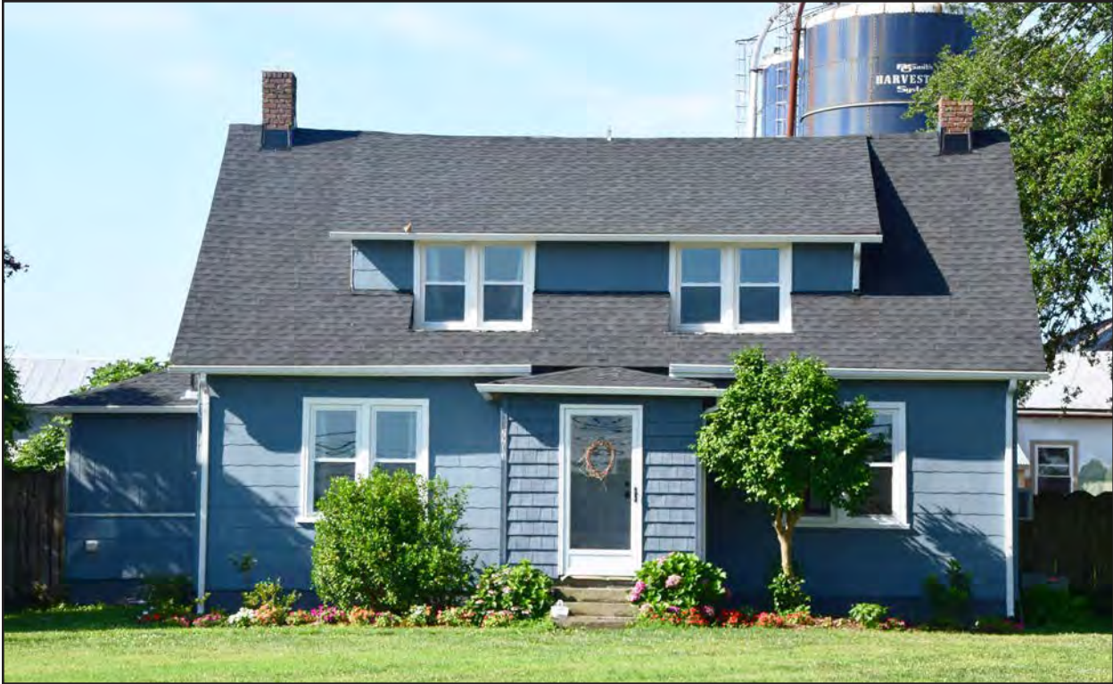
Figure 132. 131-6249, Colonial Revival dwelling, northeast elevation, view to the southwest.
