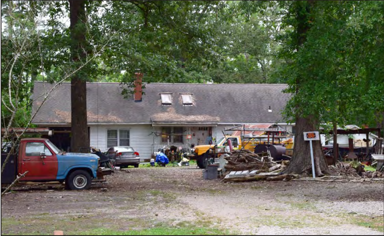
Figure 211. 134-5677, dwelling, east elevation, view to the west.
