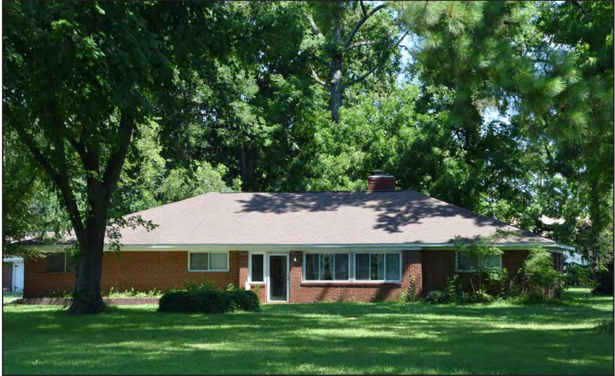
Figure 233. 134-5892, dwelling, south elevation, view to the north.
