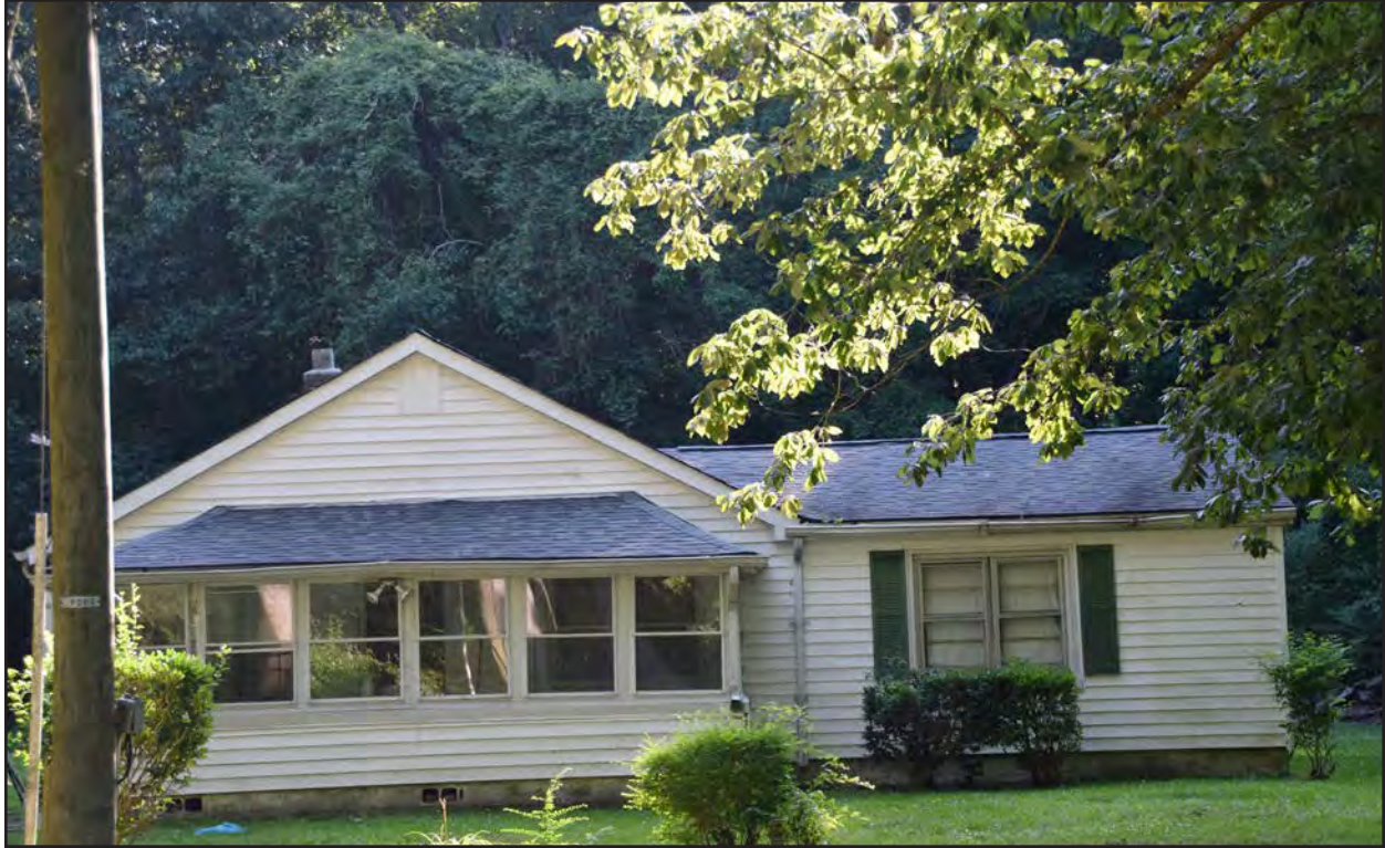
Figure 283. 134-5947, dwelling, southwest elevation, view to the northeast.
