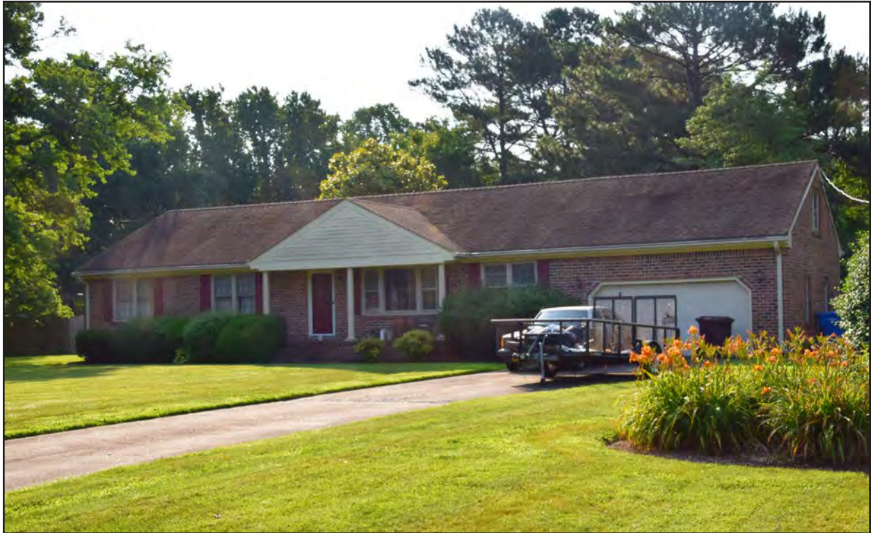
Figure 119. 131-6236, linear Ranch, northwest and southwest elevations, view to the east.
