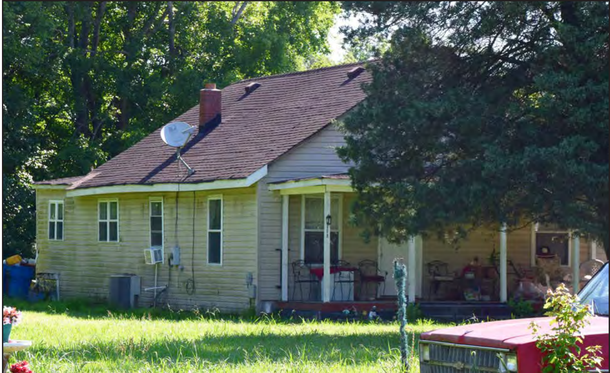
Figure 166. 134-0158, vernacular dwelling, southwest and northwest elevations, view to the east
