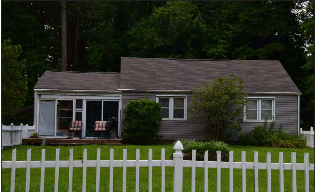
Figure 278. 134-5942, American Small House, north elevation, view to the south.
