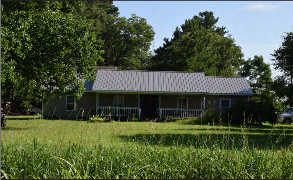
Figure 28. 131-5891, dwelling, south elevation, view to the north.
