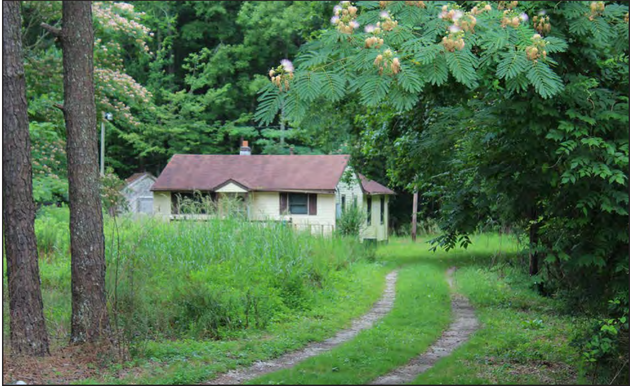
Figure 73. 131-6189, dwelling, northeast and northwest elevations, view to the south.
