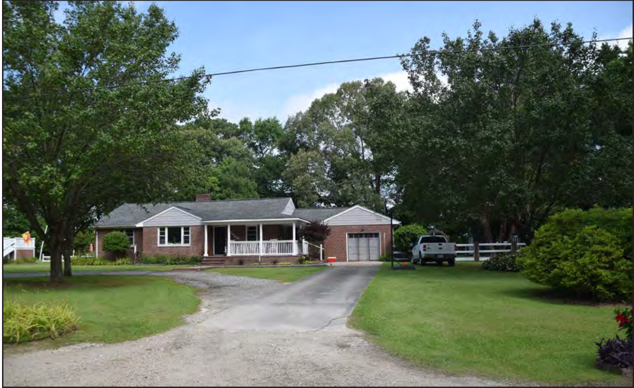
Figure 291. 134-5955, dwelling, southeast elevation, view to the northwest.
