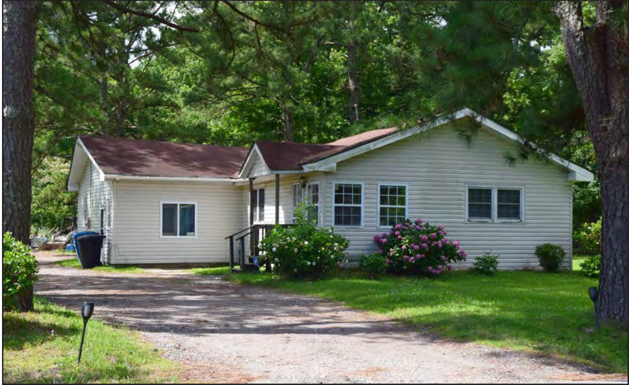
Figure 163. 131-0105, north and east elevations, view to the southwest
