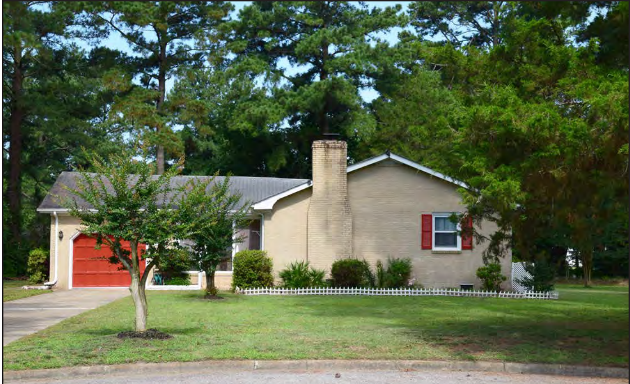
Figure 66: 131-6182, half-courtyard Ranch, east elevation, view to the west.
