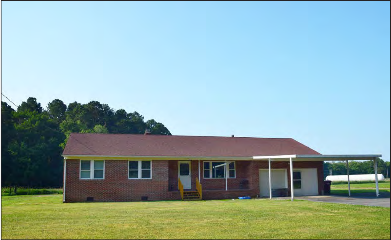
Figure 116. 131-6233, linear Ranch, northwest elevation, view to the southeast.
