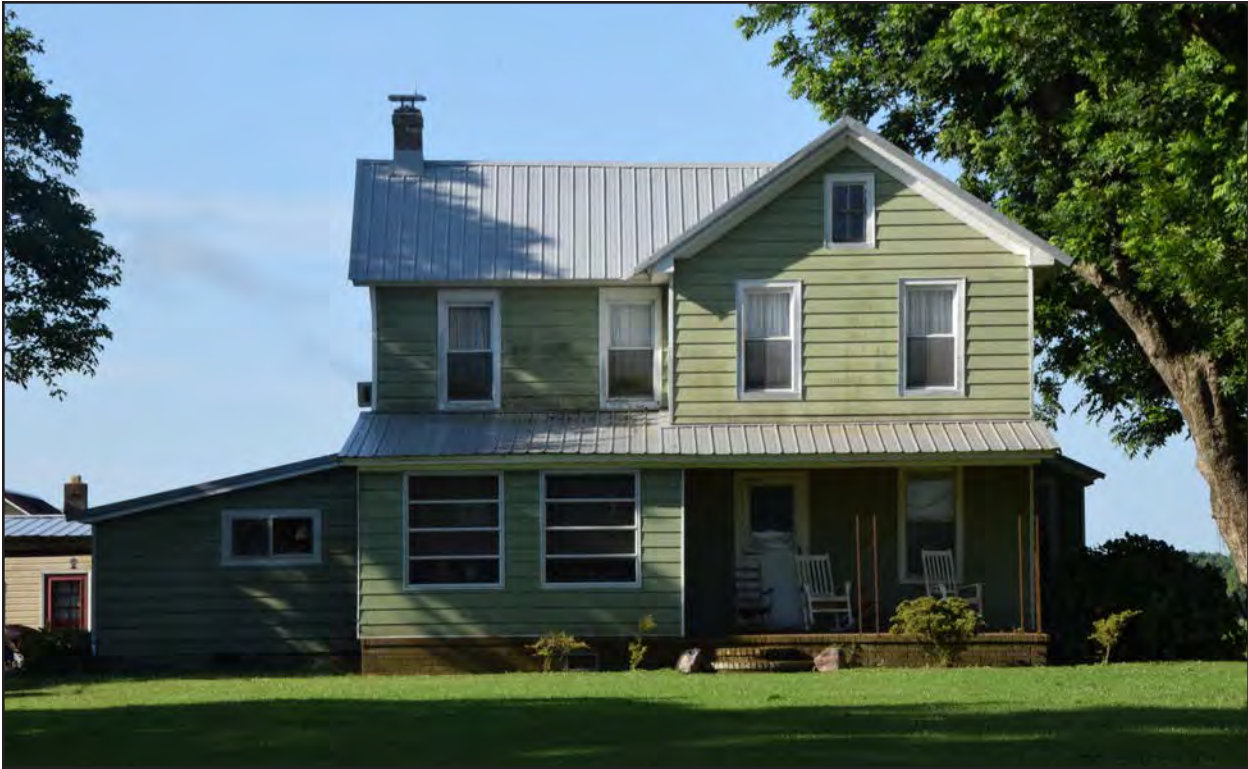
Figure 21. 131-5442, Dwelling, north elevation, view to the south.
