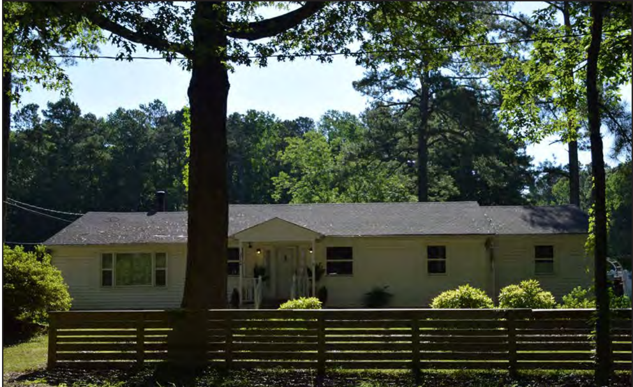
Figure 222. 134-5881, linear Ranch, west elevation, view to the east.
