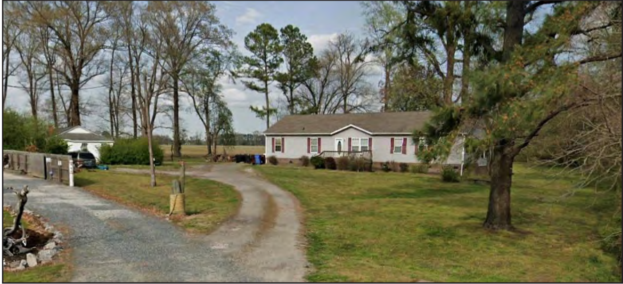
Figure 19. 131-5978, Minimal Traditional house, no longer extant, view to the northeast.
