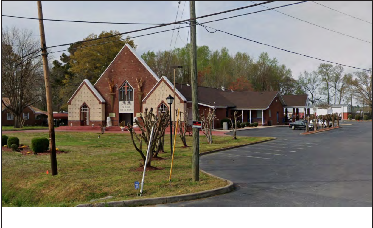
Figure 60. 131-6014, The United House of Prayer for All People Church, south and east elevations, view to the northwest.
