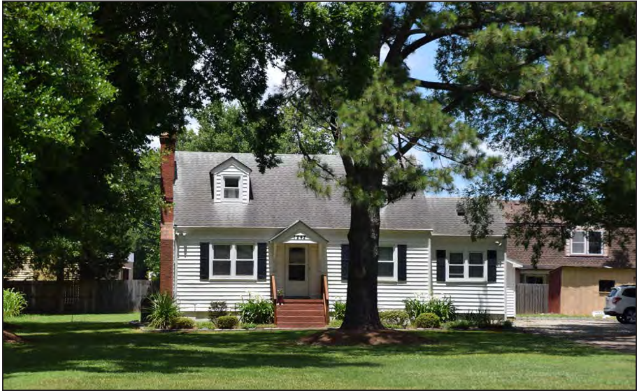
Figure 167. 134-0161, dwelling, south elevation, view to the north
