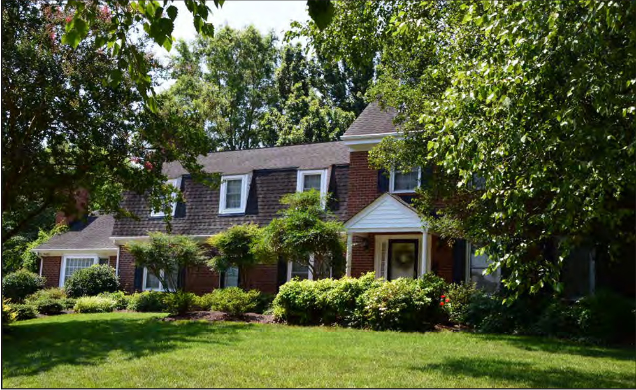
Figure 294. 134-5958, dwelling, northeast elevation.
