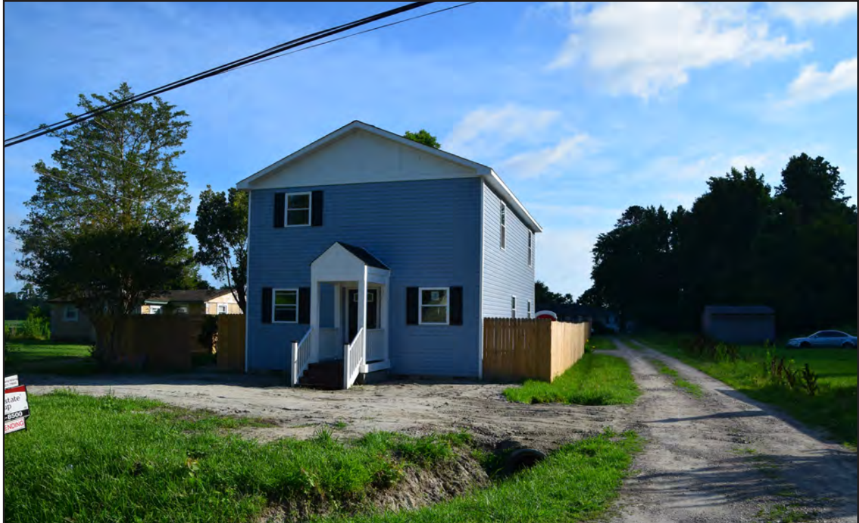
Figure 20. 131-5993, Minimal Traditional house, no longer extant, view to the northeast.
