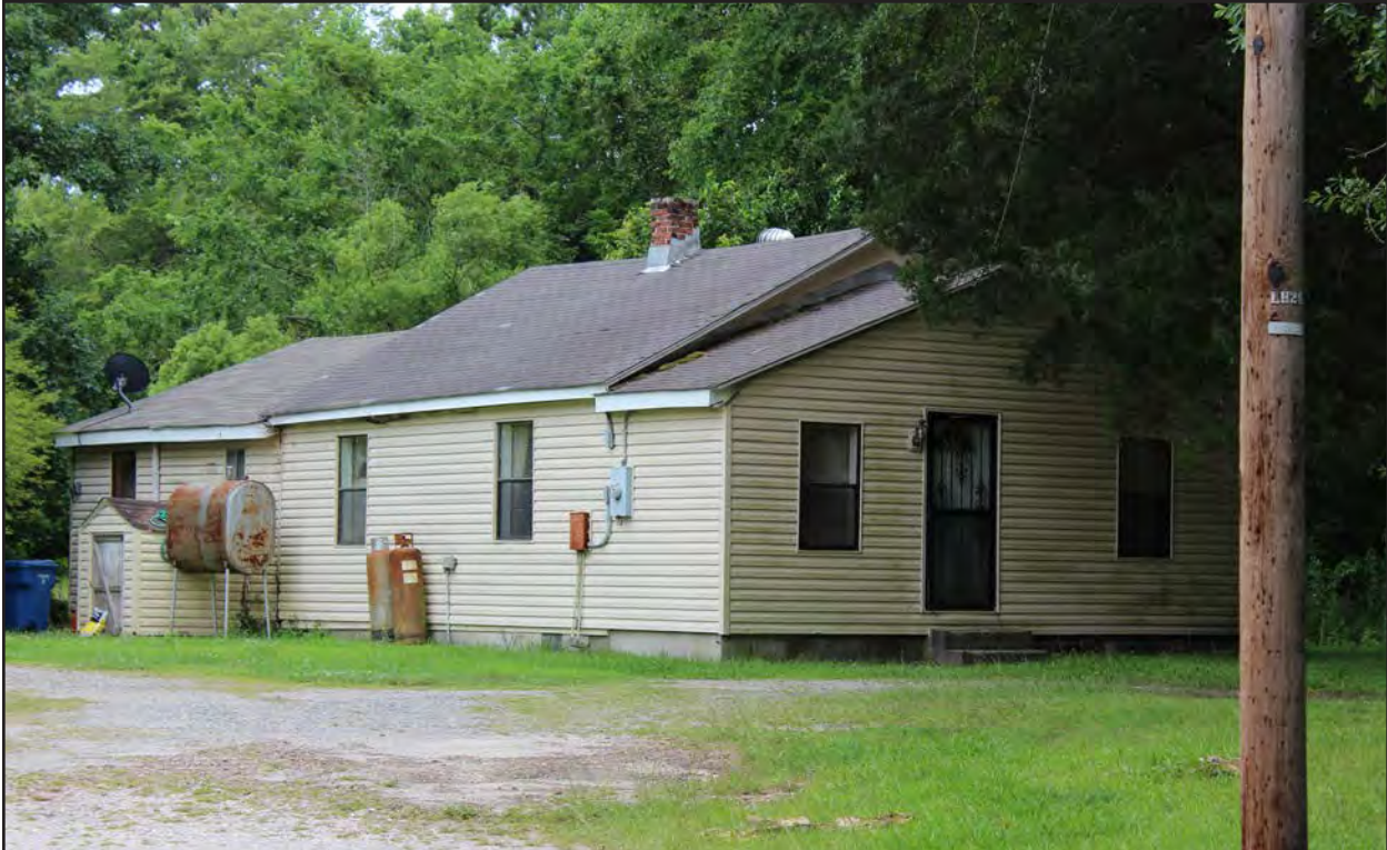
Figure 76. 131-6193, dwelling, northeast and southeast elevations, view to the west.
