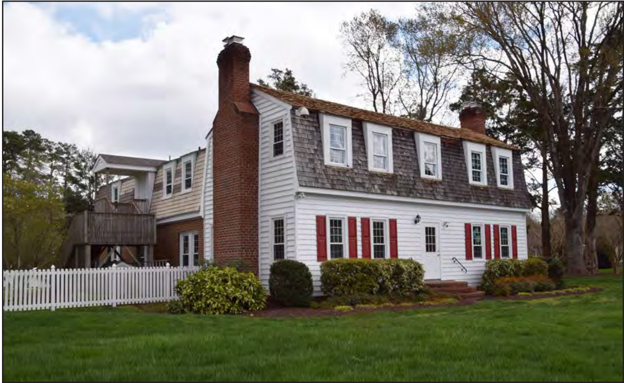
Figure 161. 134-0072, Thomas Lovett House/Rollingwood Academy, southwest and northwest elevations, view to the east.
