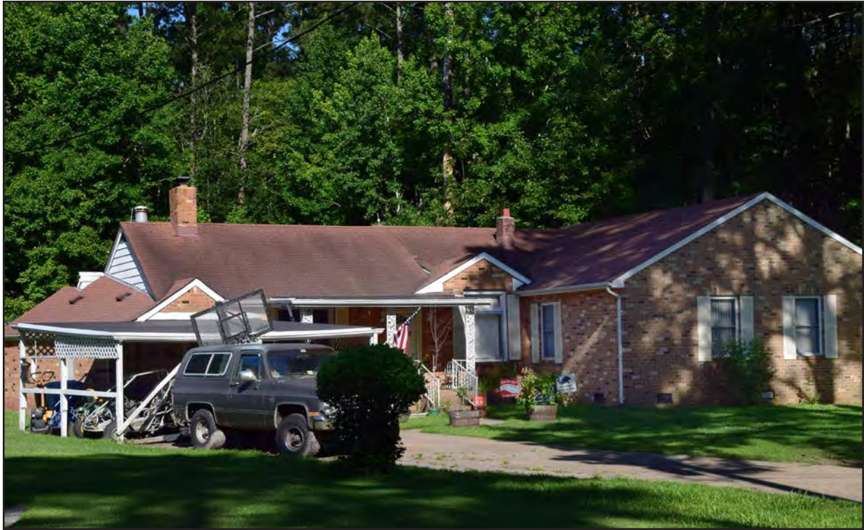
Figure 225. 134-5884, dwelling, south and east elevations, view to the northwest.
