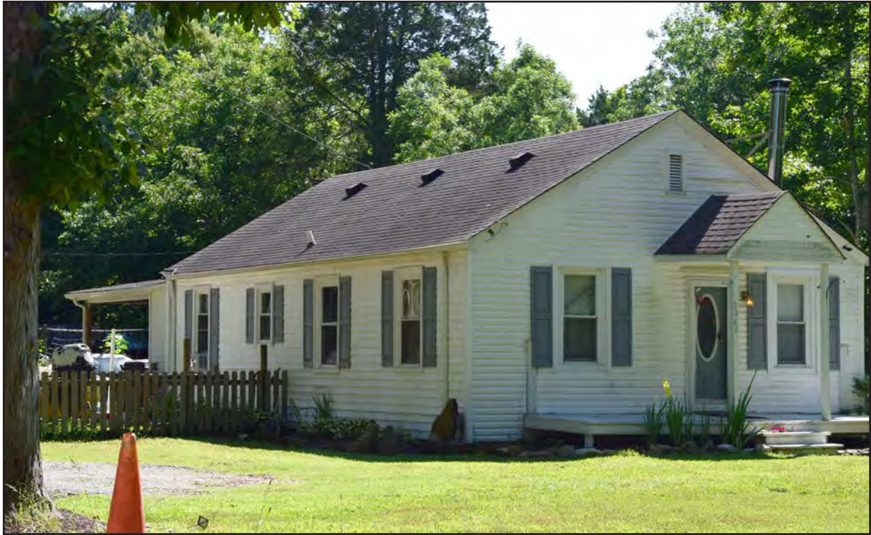
Figure 271. 134-5932, dwelling, southwest elevation, view to the northeast.
