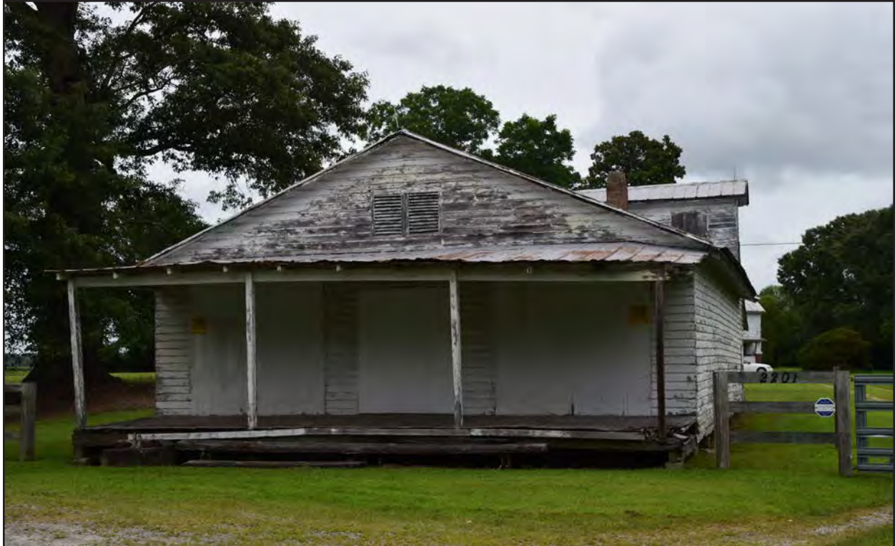
Figure 6: 131-0158, Eddie Hudgins Store, southwest and southeast elevations, view to the north.
