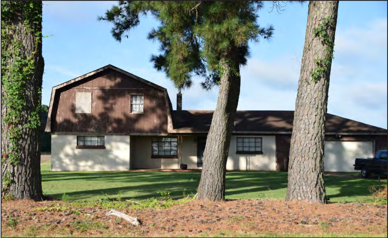
Figure 146. 131-6265, linear Ranch, northeast elevation, view to the southwest.
