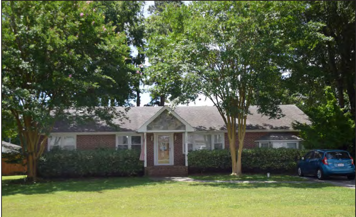
Figure 198. 134-5218, linear Ranch, north elevation, view to the south.
