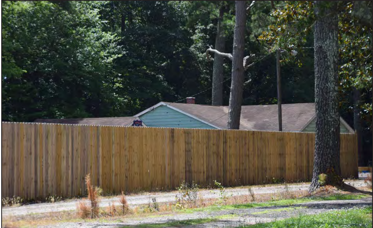
Figure 254. 134-5914, dwelling, north and west elevations, view to the southeast.
