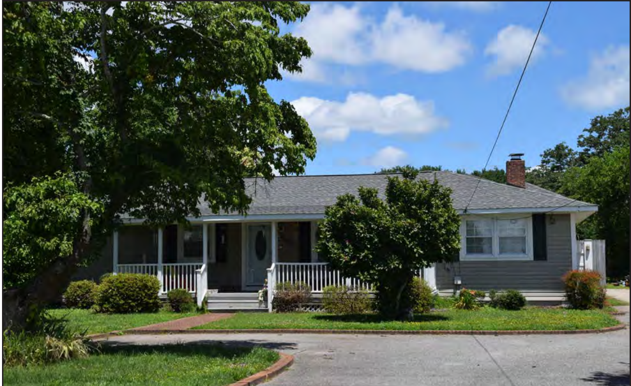
Figure 250. 134-5910, linear Ranch, south elevation, view to the north.
