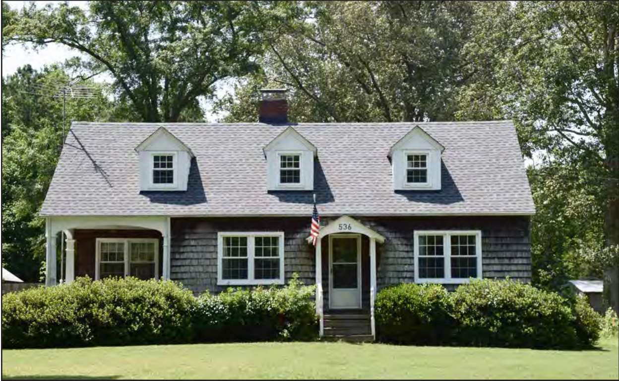
Figure 131. 131-6248, Colonial Revival dwelling, northeast elevation.
