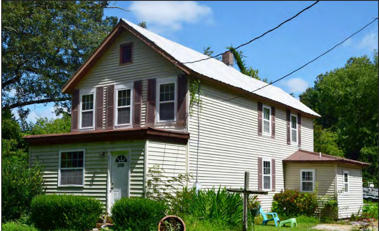
Figure 102. 131-6219, vernacular dwelling, south and east elevations, view to the northwest.
