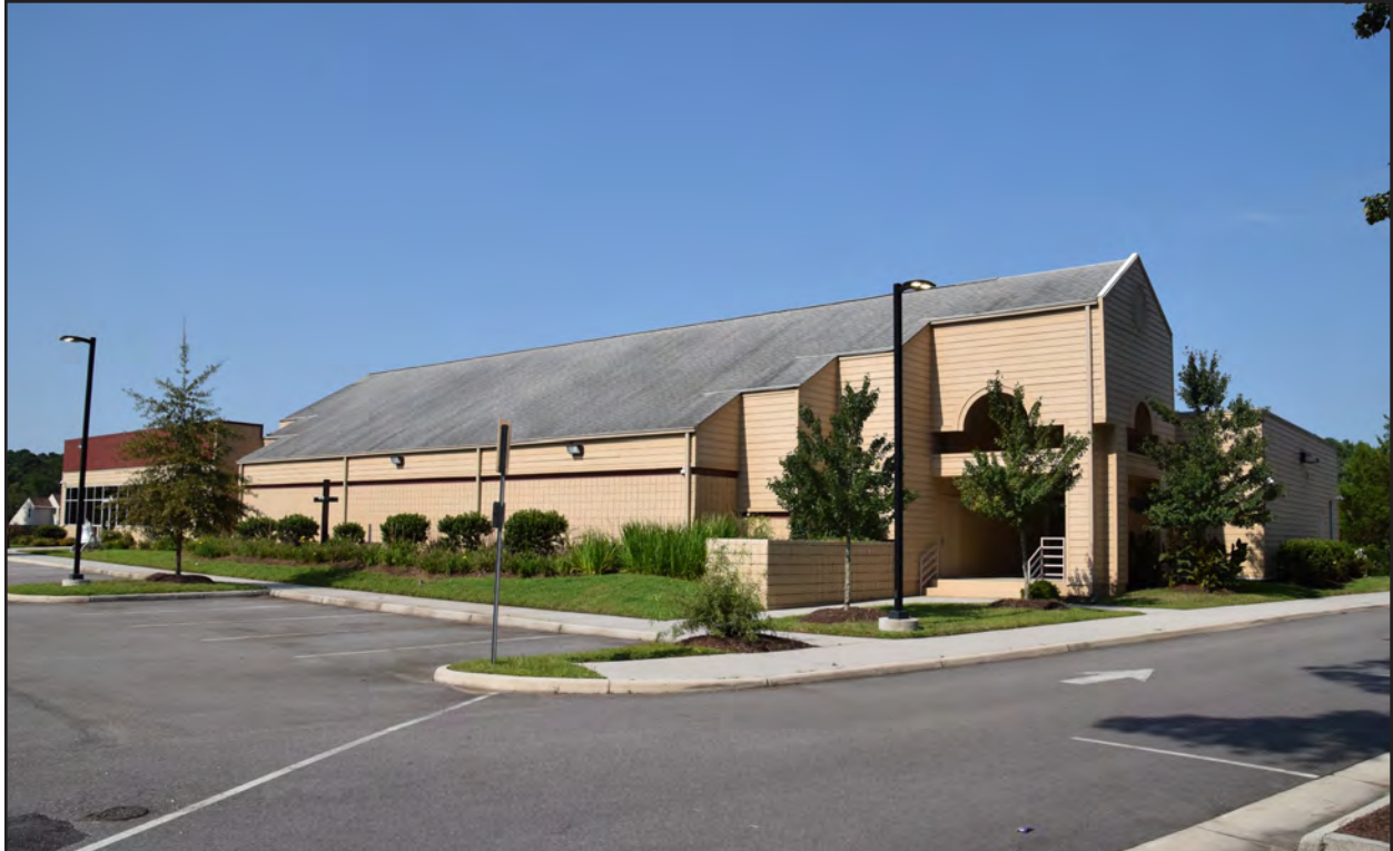
Figure 30. 134-0152, Piney Grove Church Hall, no longer extant, replacement church, view to the north.
