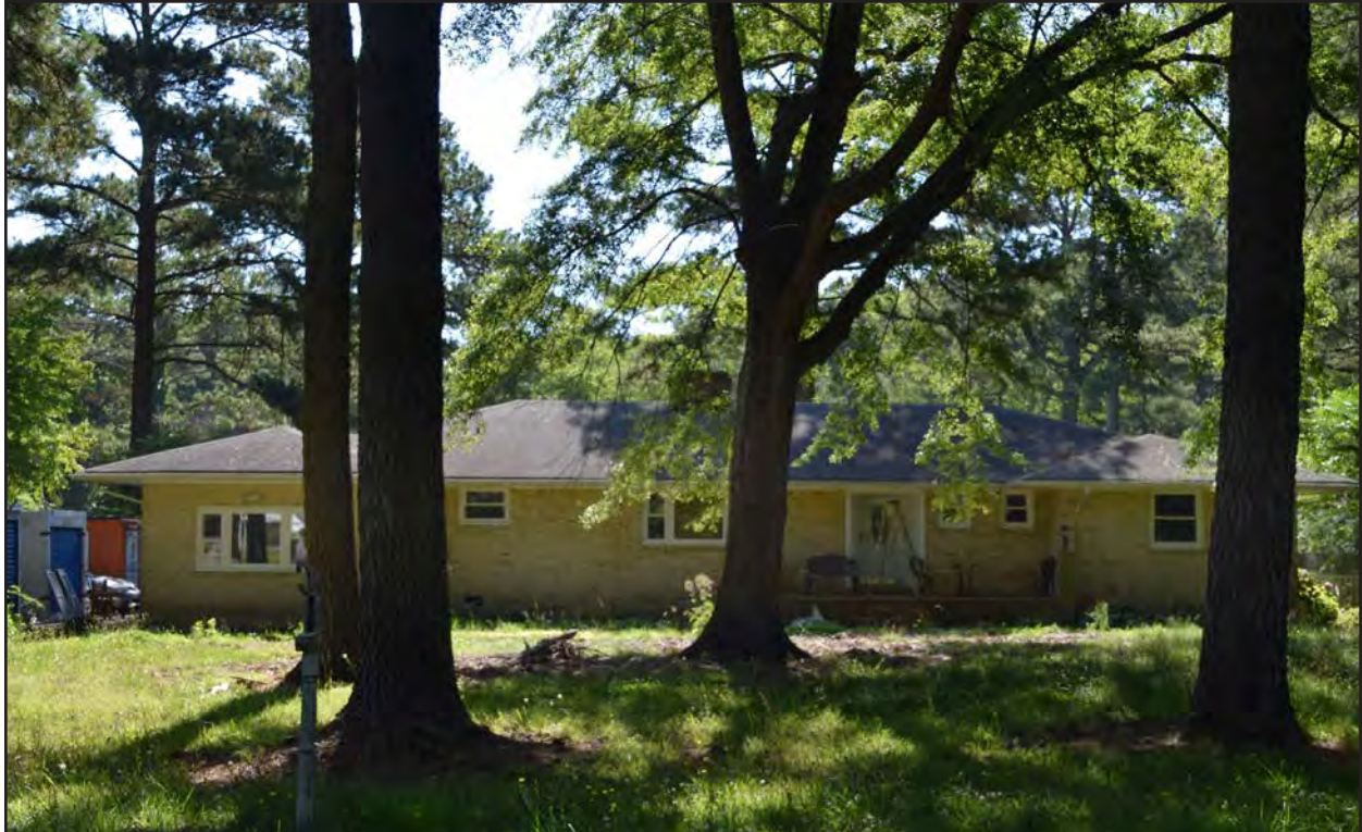
Figure 236. 134-5896, dwelling, west elevation, view to the east.
