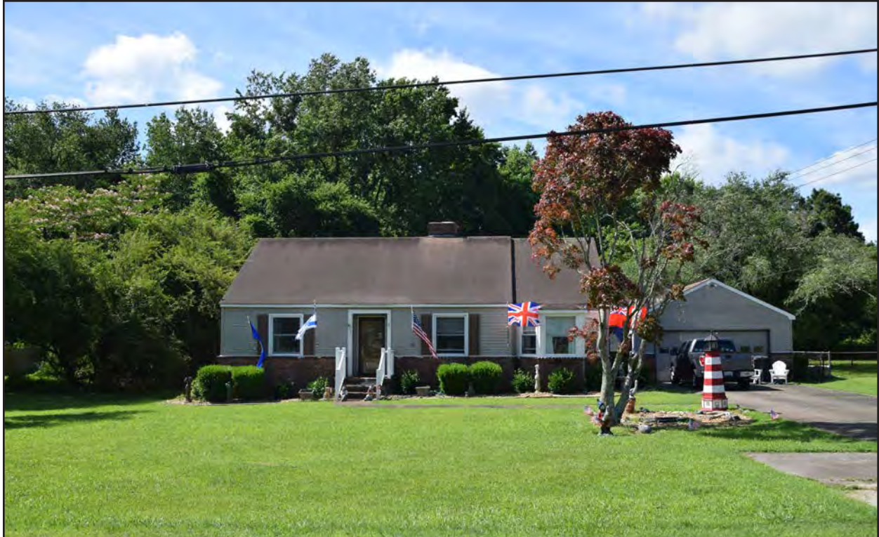
Figure 202. 134-5222, dwelling, north elevation, view to the south.
