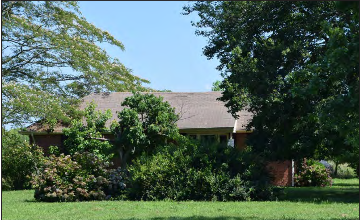
Figure 232. 134-5891, dwelling, south elevation, view to the north.
