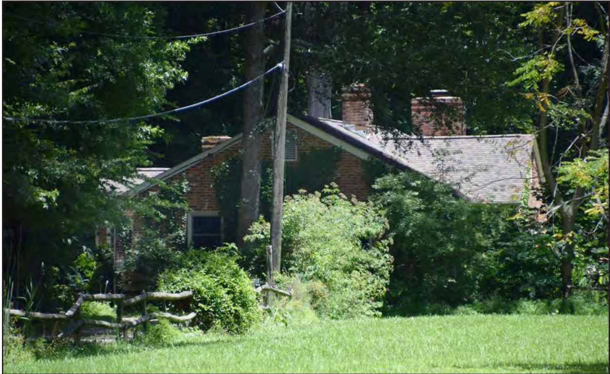
Figure 281. 134-5945, linear-with-clusters Ranch dwelling, southeast and southwest elevations, view to the north.
