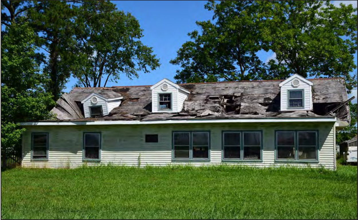
Figure 53. 131-6004, vernacular dwelling, southeast elevation, view to the northwest.
