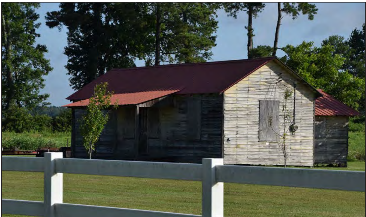
Figure 2. 131-0150, saddlebag, southwest and southeast elevations, view to the north.
