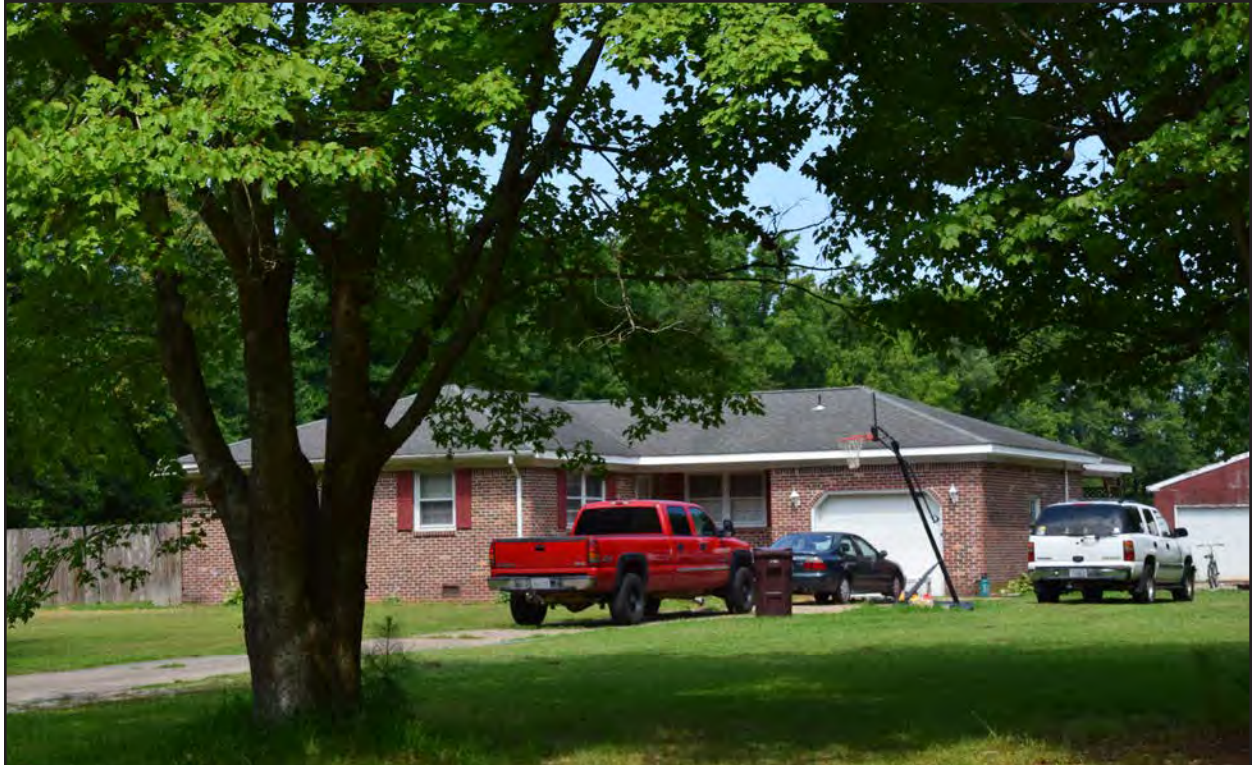
Figure 122. 131-6239, half-courtyard Ranch, north and east elevations, view to the northwest.
