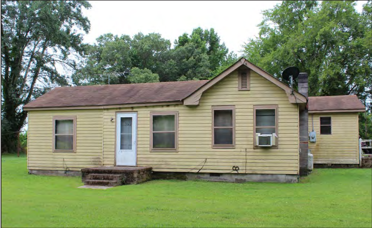
Figure 75. 131-6192, dwelling and additions, northeast and northwest elevations, view to the south.
