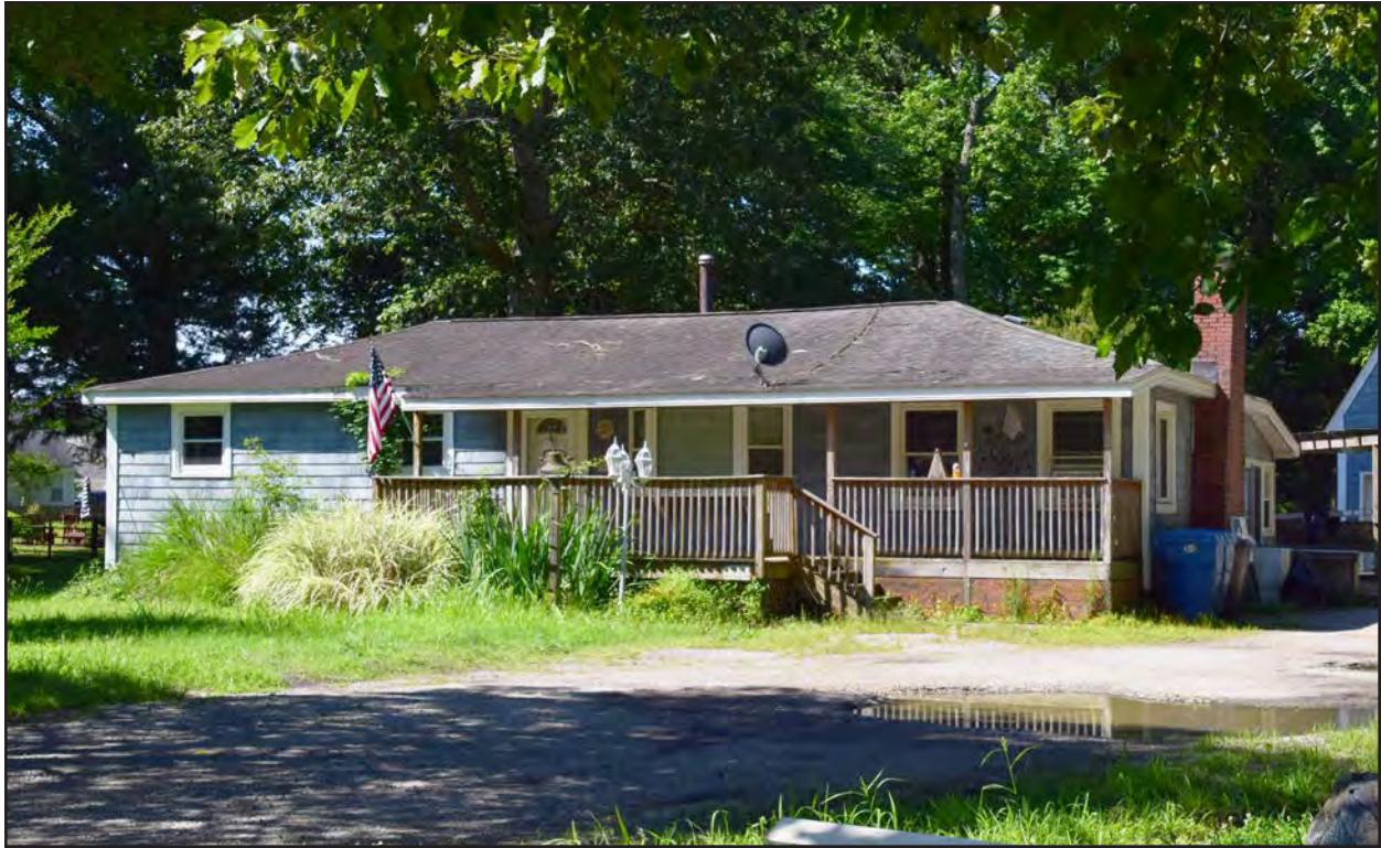
Figure 265. 134-5925, dwelling, North and East elevations.
