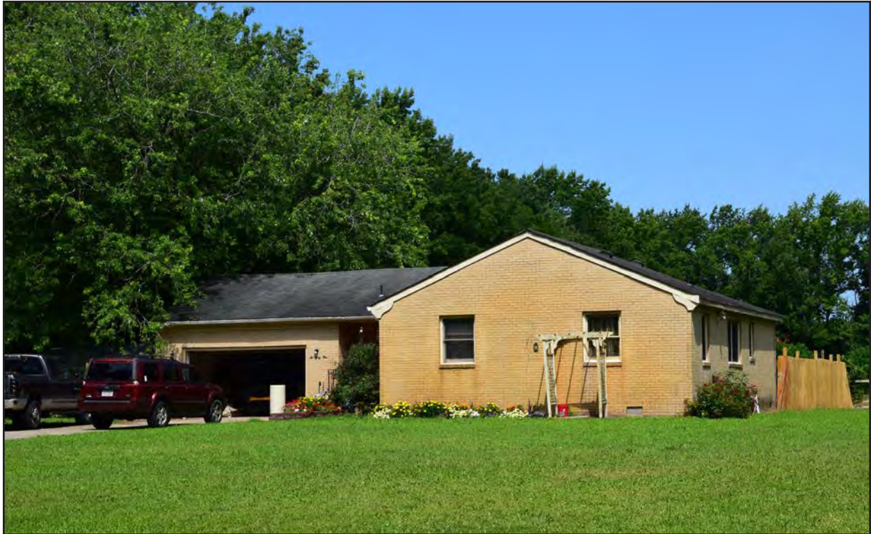
Figure 121. 131-6238, half-courtyard Ranch, east elevation, view to the west.
