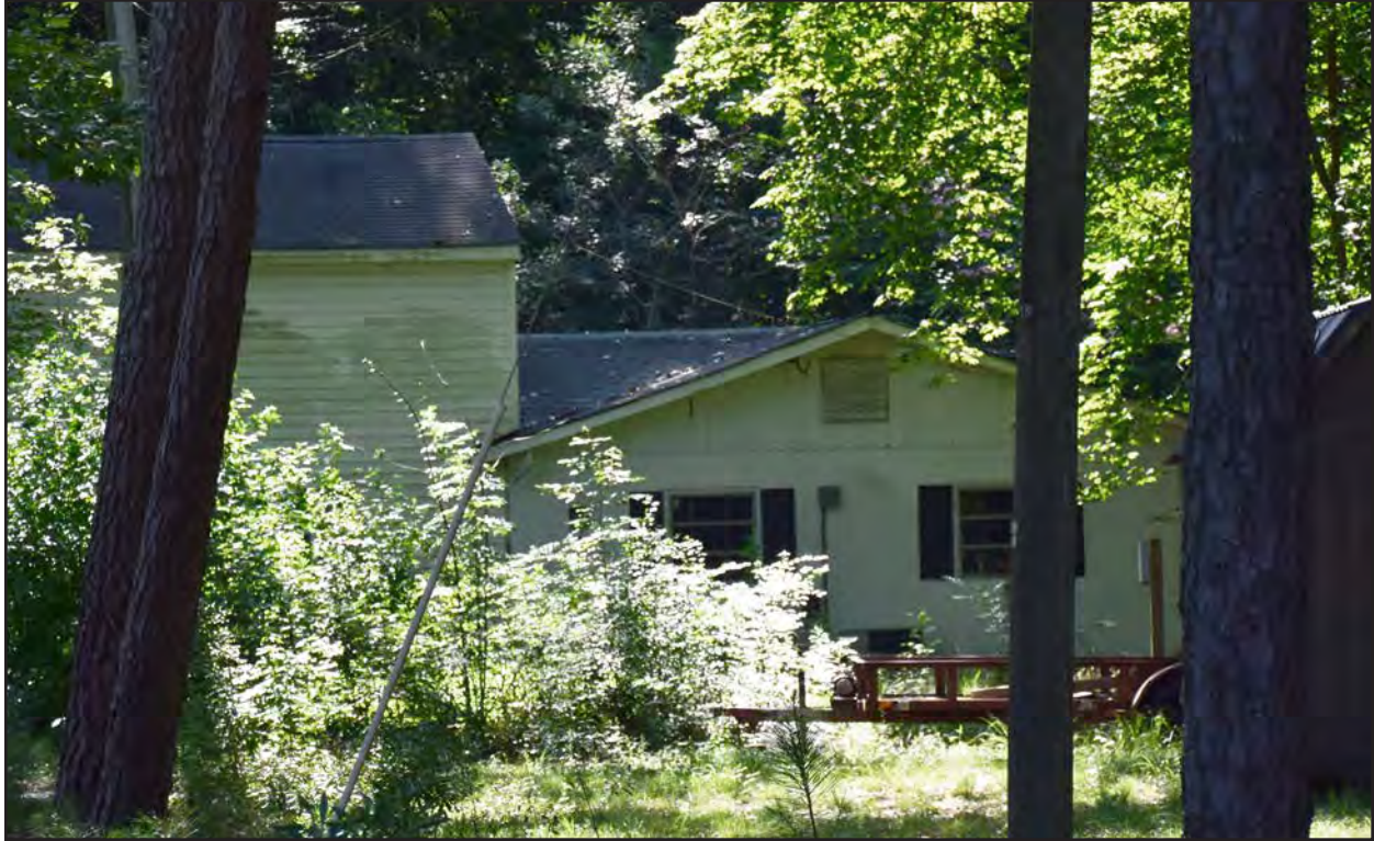
Figure 289. 134-5952, secondary vernacular dwelling, west elevation, view to the east.
