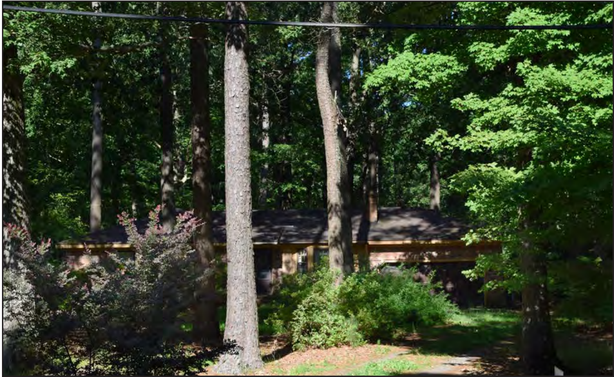
Figure 227. 134-5886, dwelling, east elevation, view to the west.
