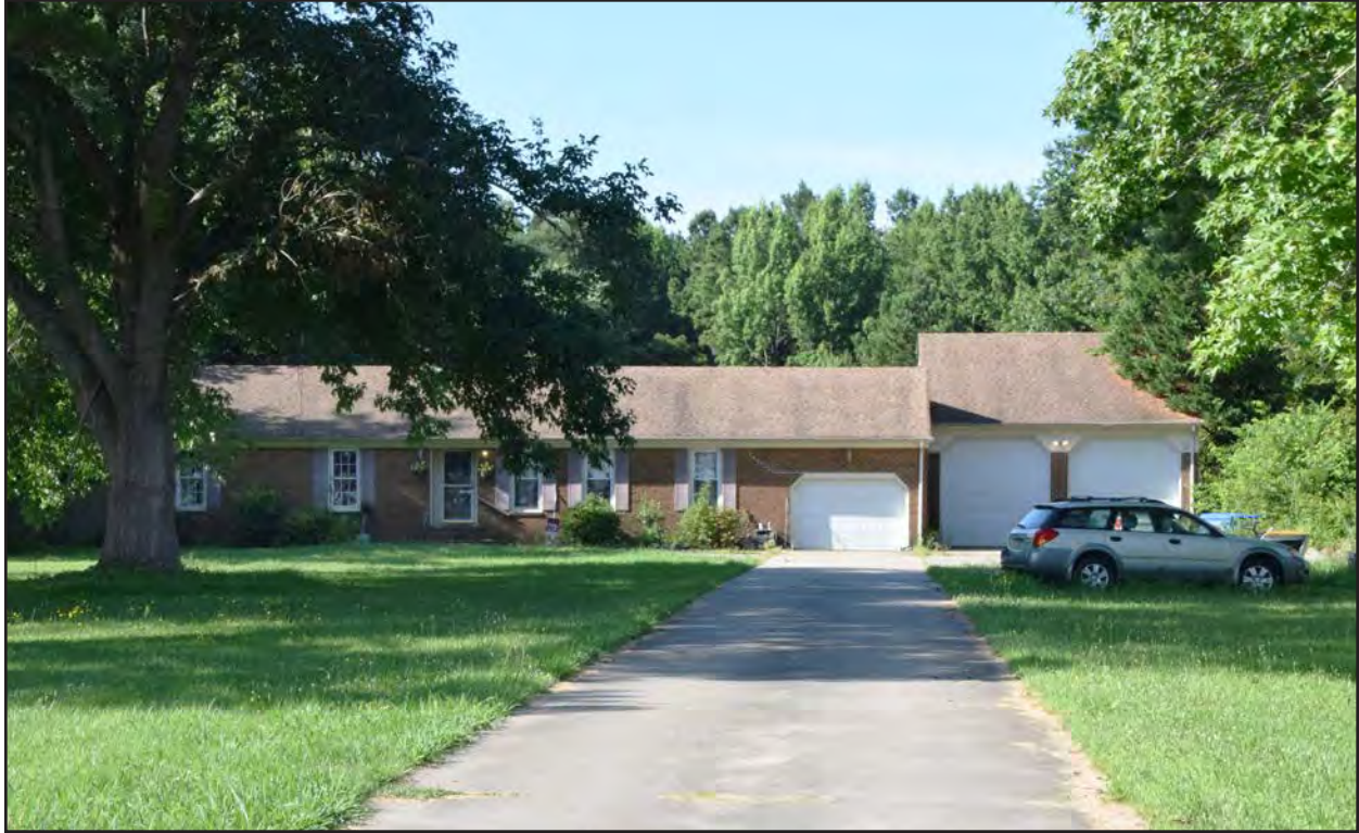
Figure 149. 131-6268, linear Ranch, north elevation, view to the south.
