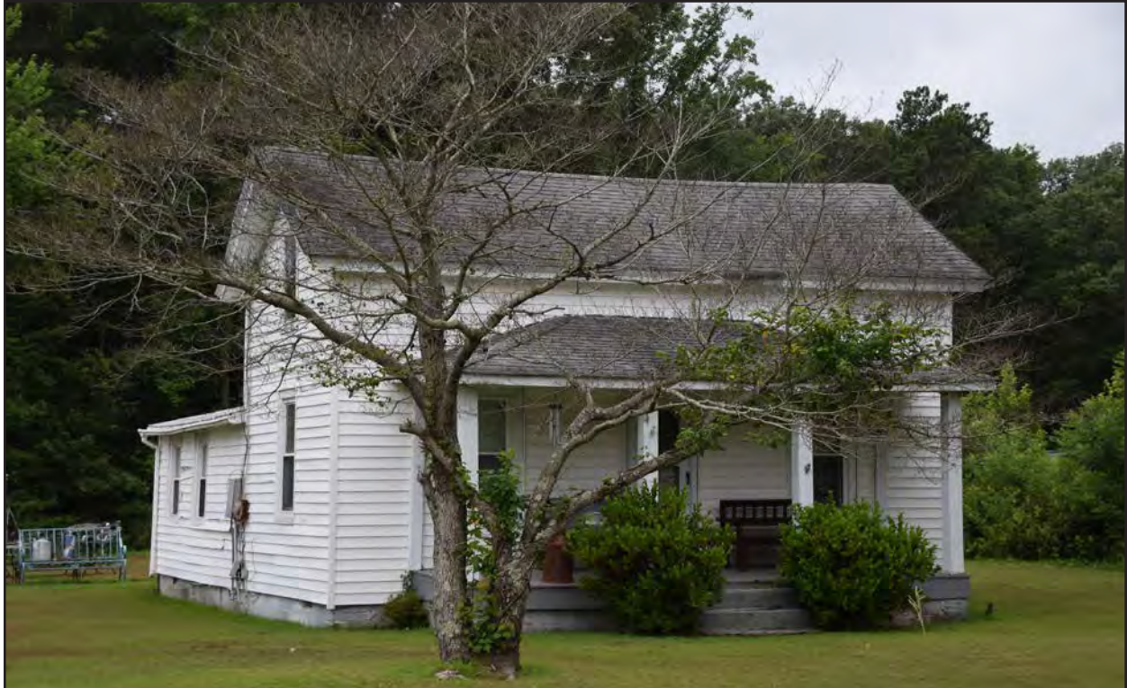
Figure 4. 131-0152, vernacular dwelling, northeast and southeast elevations, view to the west.
