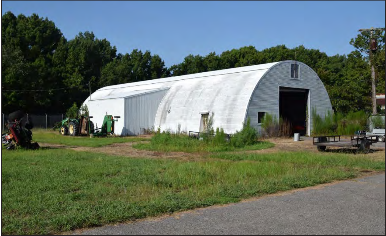
Figure 175. 134-5937, Quonset Hut, northeast and southeast elevations, view to west.
