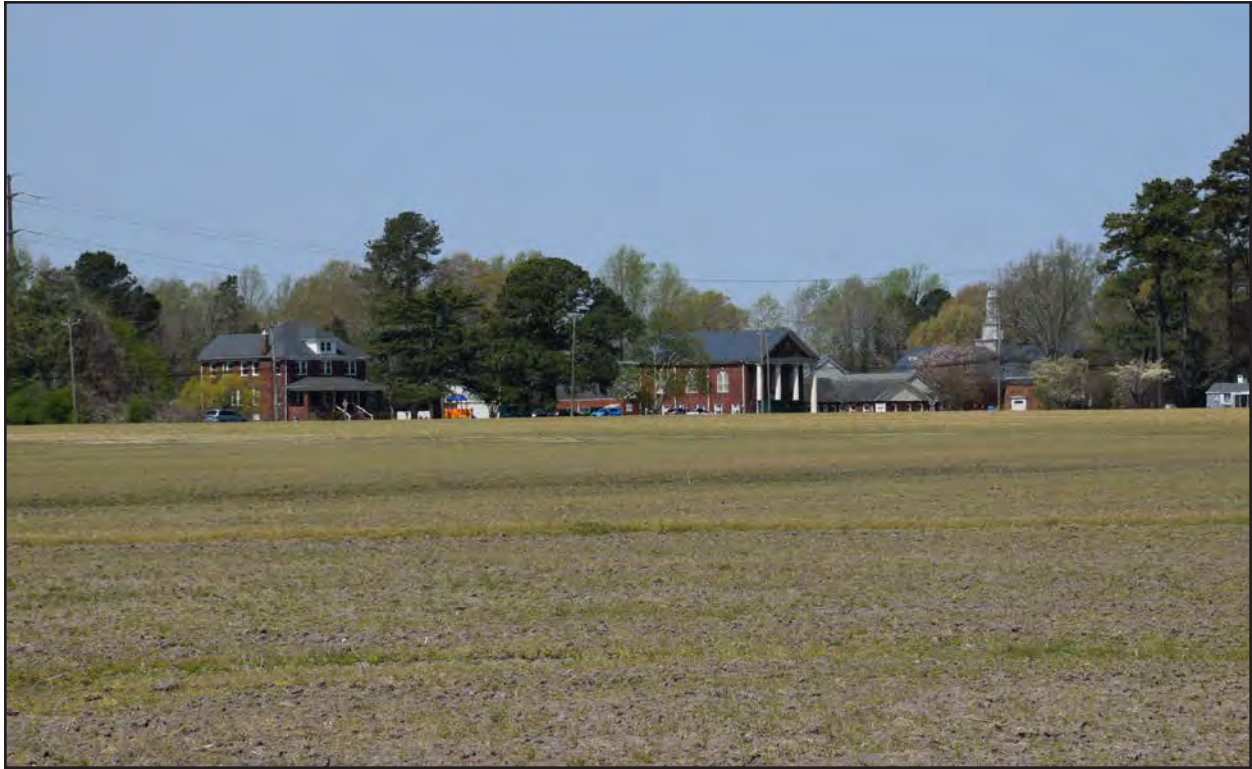
Figure 13. 131-5071, Centreville-Fentress Historic District, view to the northwest.
