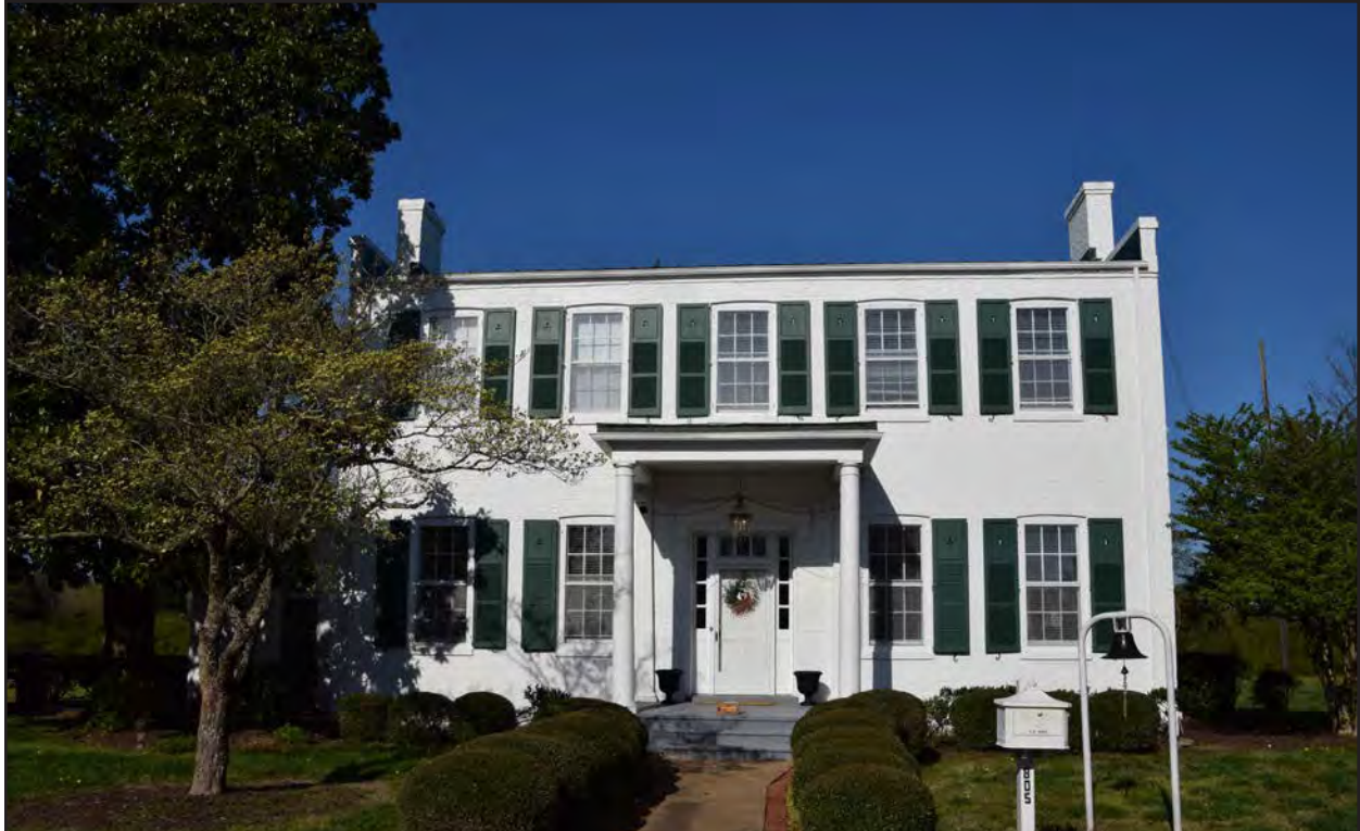
Figure 156. 134-0003, James Bell House, east elevation, view to the west.
