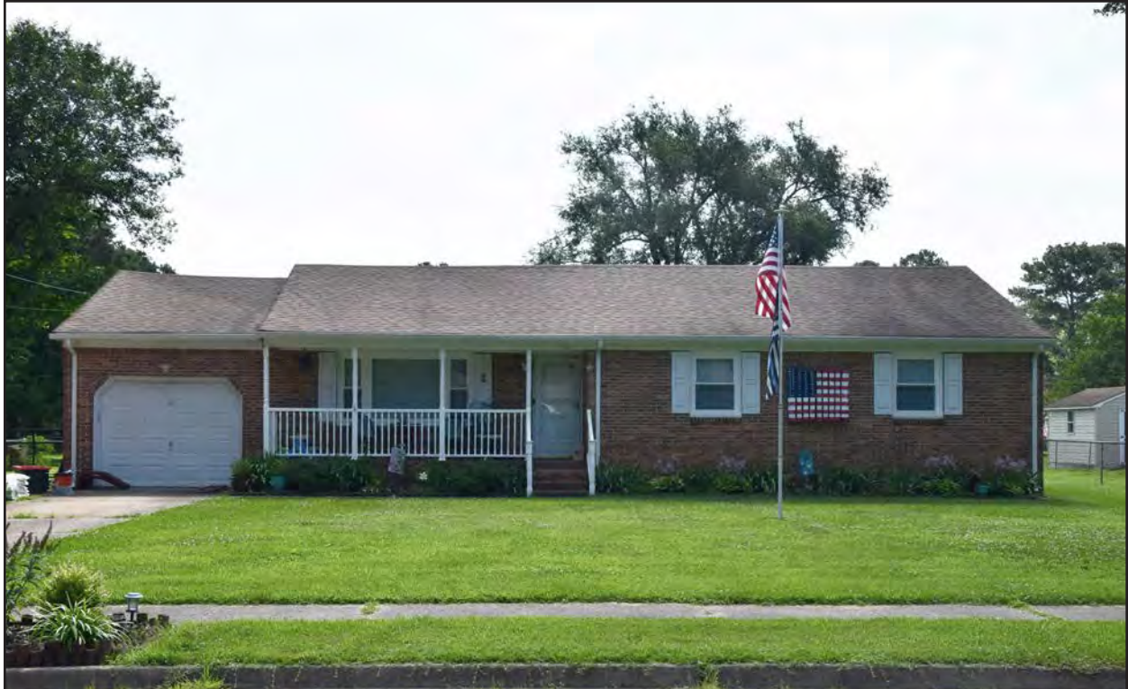
Figure 88. 131-6205, linear Ranch, west elevation, view to the east.
