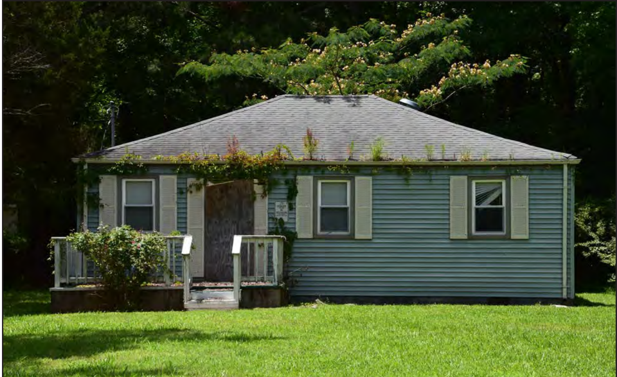
Figure 276. 134-5940, dwelling, east elevation, view to the west.
