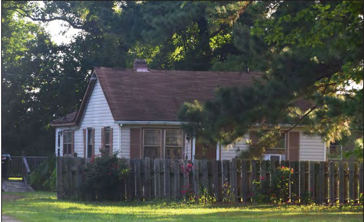
Figure 40. 131-5988, dwelling, southwest and northwest elevations, view to the east.
