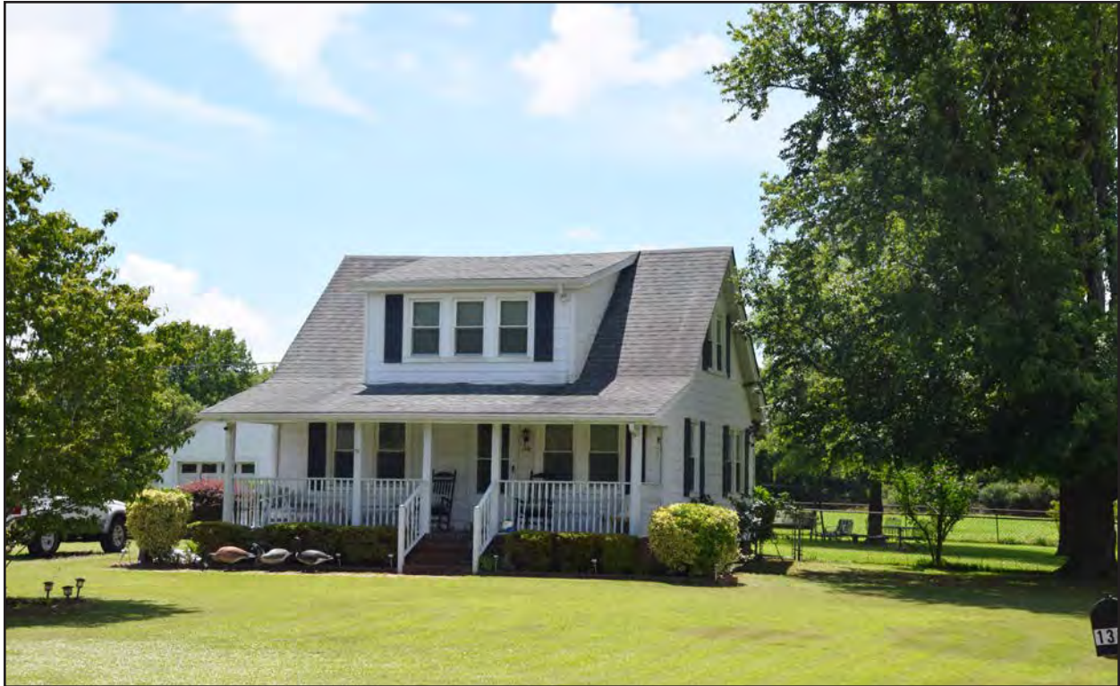
Figure 165. 134-0112, Craftsman dwelling, north and west elevations, view to the southeast.
