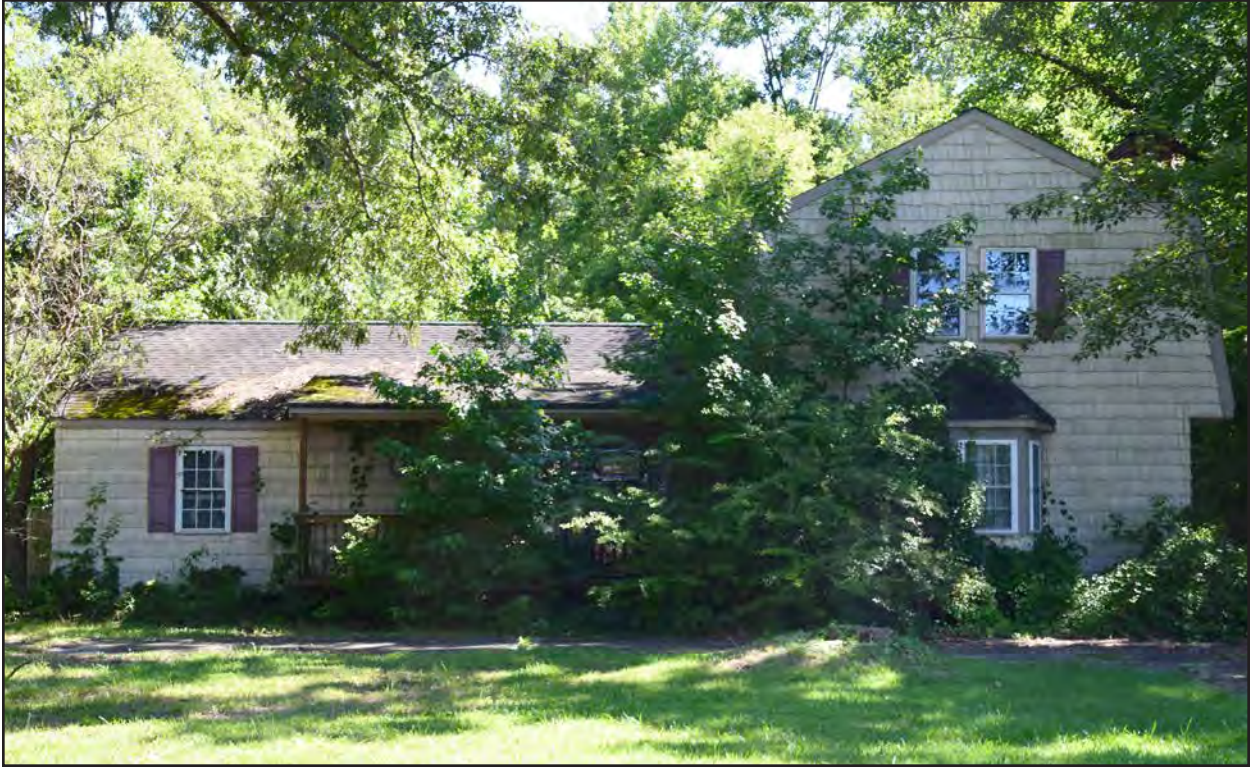
Figure 273. 134-5934, dwelling, southwest elevation, view to the northeast.
