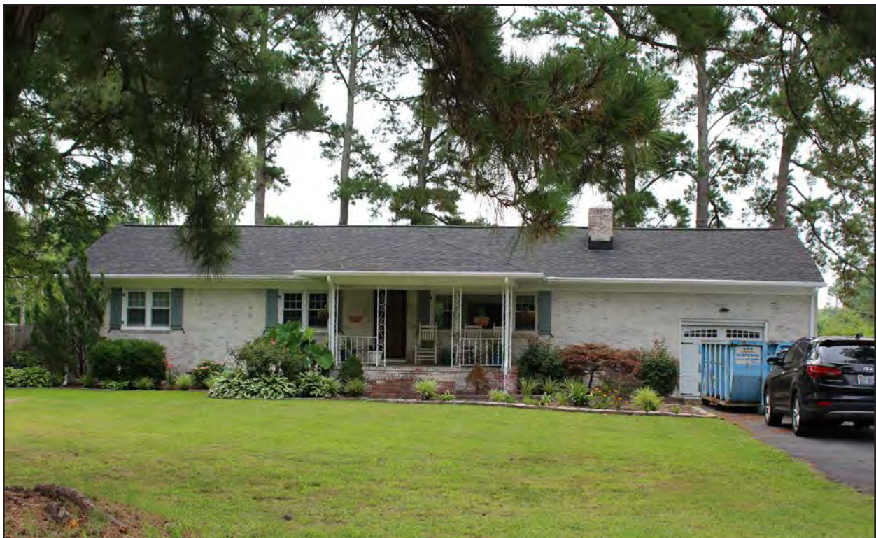
Figure 138. 131-6257, linear Ranch dwelling, west elevation, view to the east.
