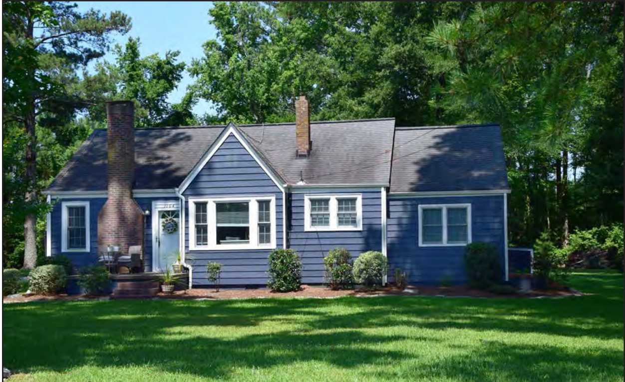
Figure 128. 131-6245, Tudor Revival dwelling, southeast elevation, view to the northwest.
