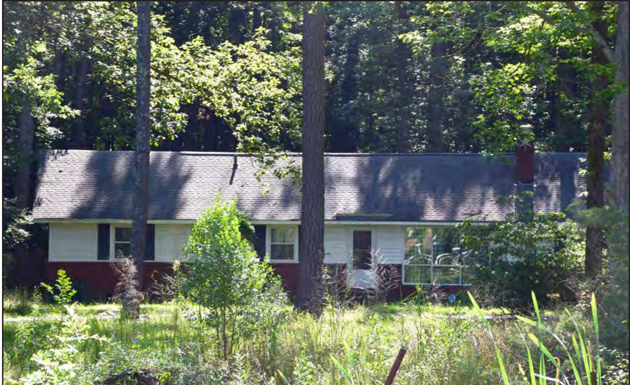
Figure 288. 134-5952, linear Ranch dwelling, west elevation, view to the east.
