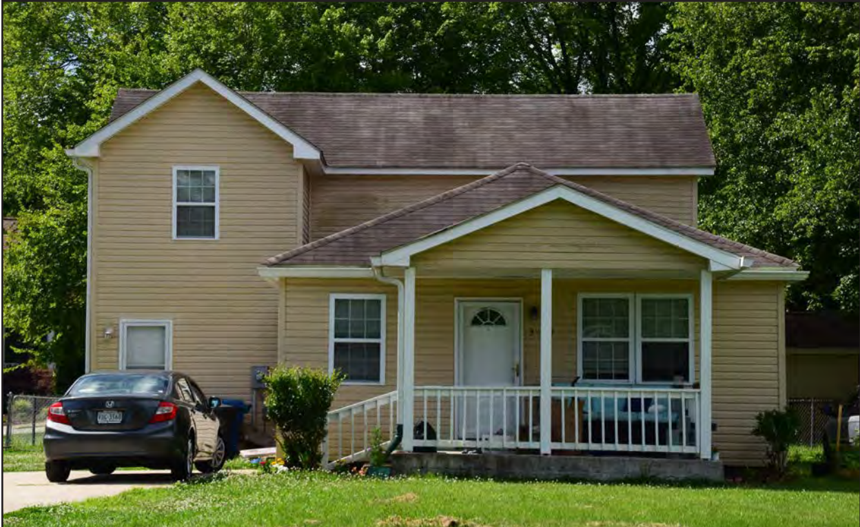
Figure 242. 134-5901, dwelling, north elevation, view to the south.
