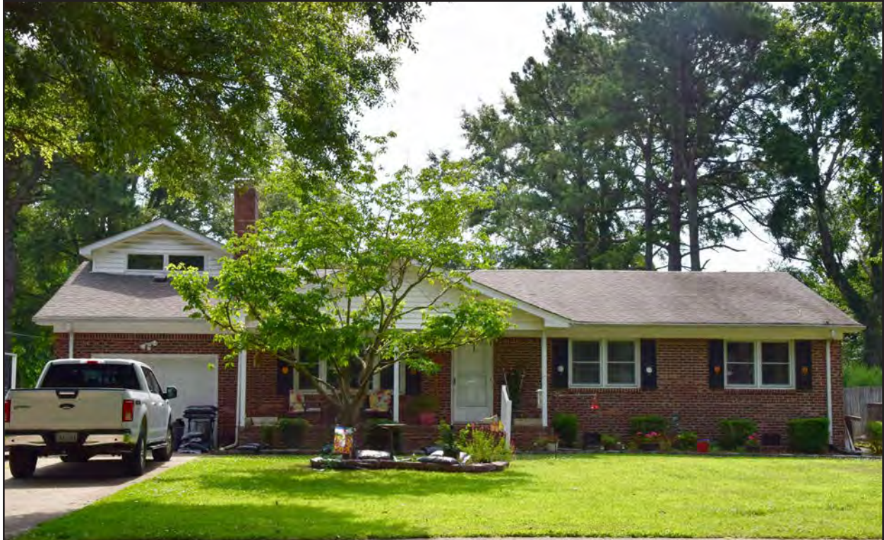
Figure 80. 131-6197, linear Ranch, west elevation, view to the east.
