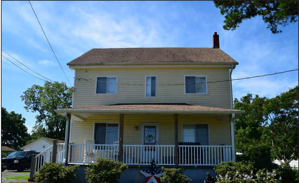
Figure 10. 131-0178, vernacular dwelling, north elevation, view to the south.
