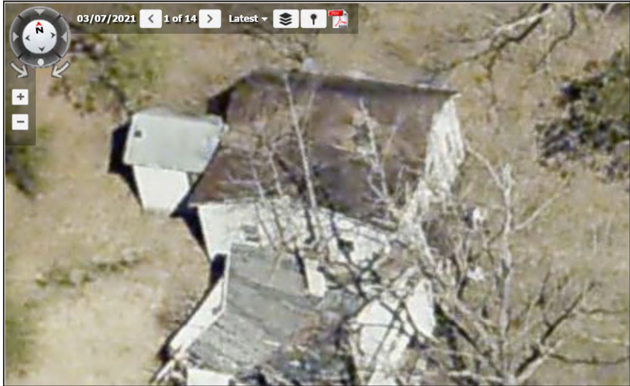
Figure 239. 134-5899, dwelling, aerial photograph.
