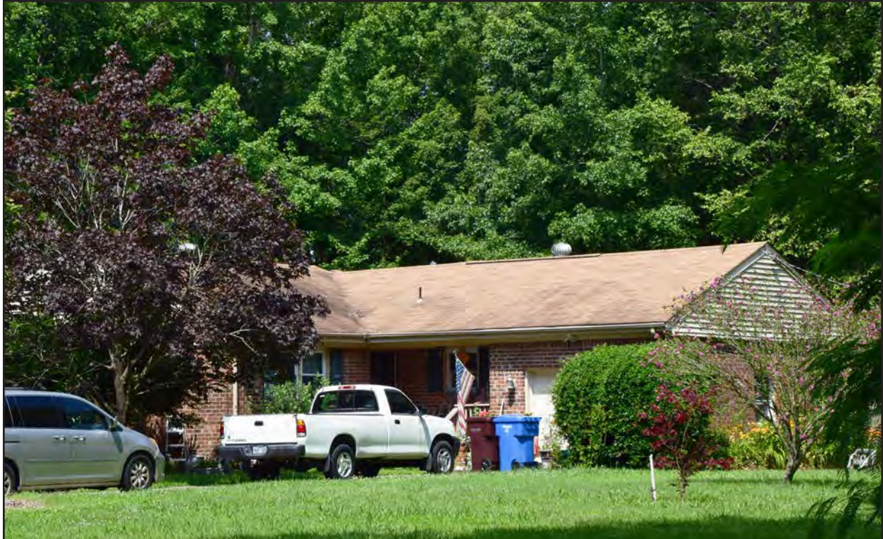
Figure 120. 131-6237, half-courtyard Ranch, north and east elevations, view to the northwest.
