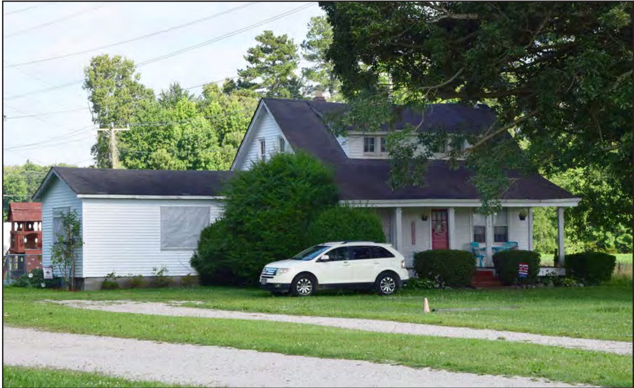
Figure 151. 131-6269, Murray Farms, secondary dwelling, east and south elevations, view to the northwest.
