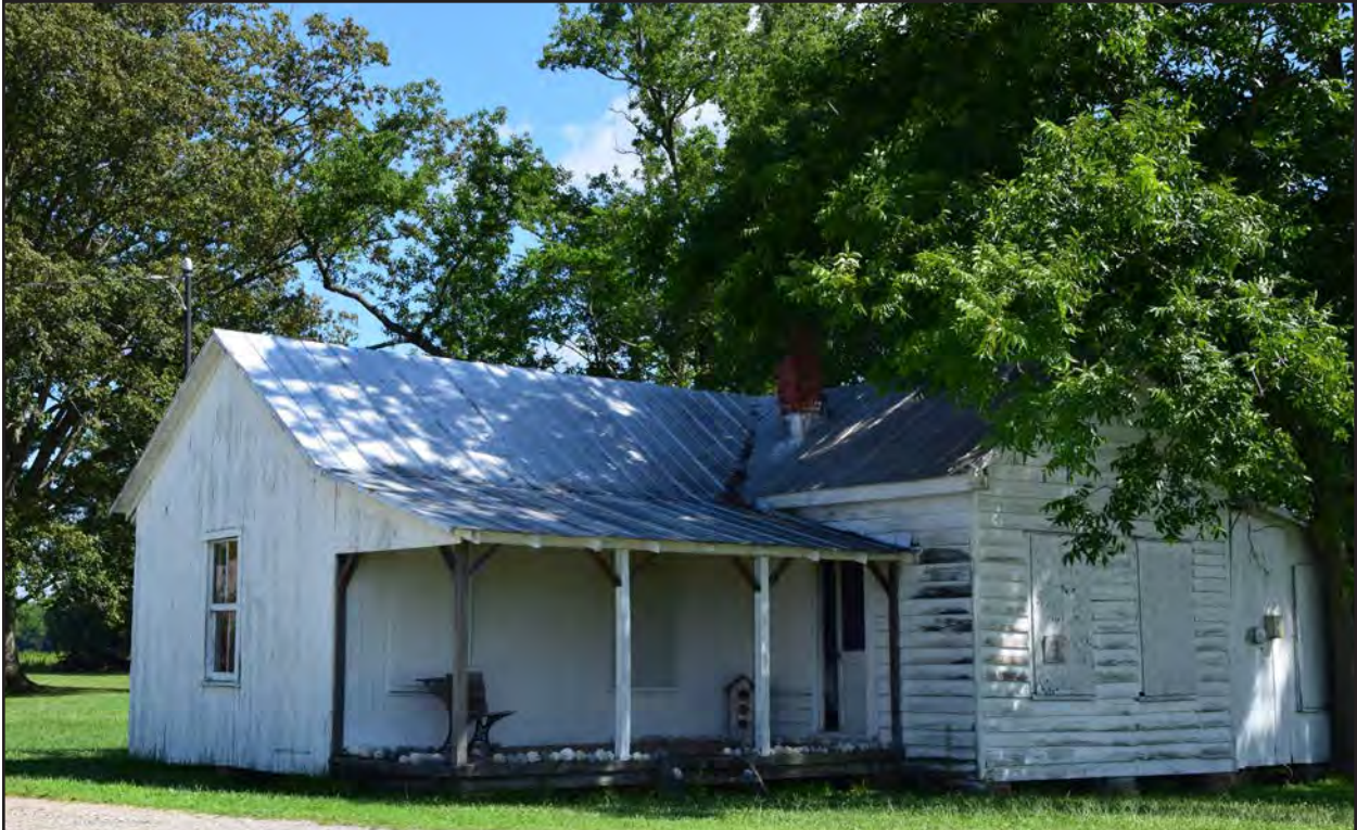
Figure 54. 131-6005, vernacular primary dwelling, southeast and southwest elevations, view to the north.
