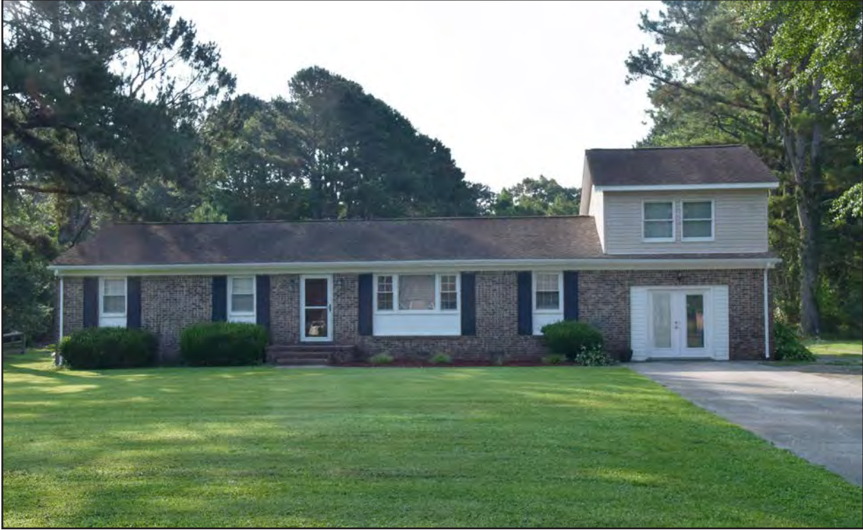
Figure 118. 131-6235, linear Ranch, northwest elevation, view to the southeast.
