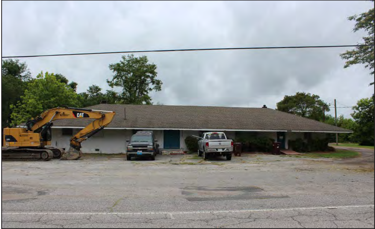
Figure 99. 131-6216, Deal's Grocery, northeast elevation, view to the southwest.
