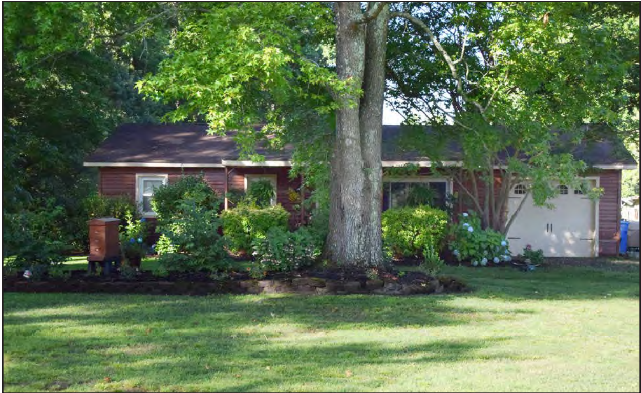
Figure 95. 131-6212, linear Ranch, northeast elevation, view to the southwest.
