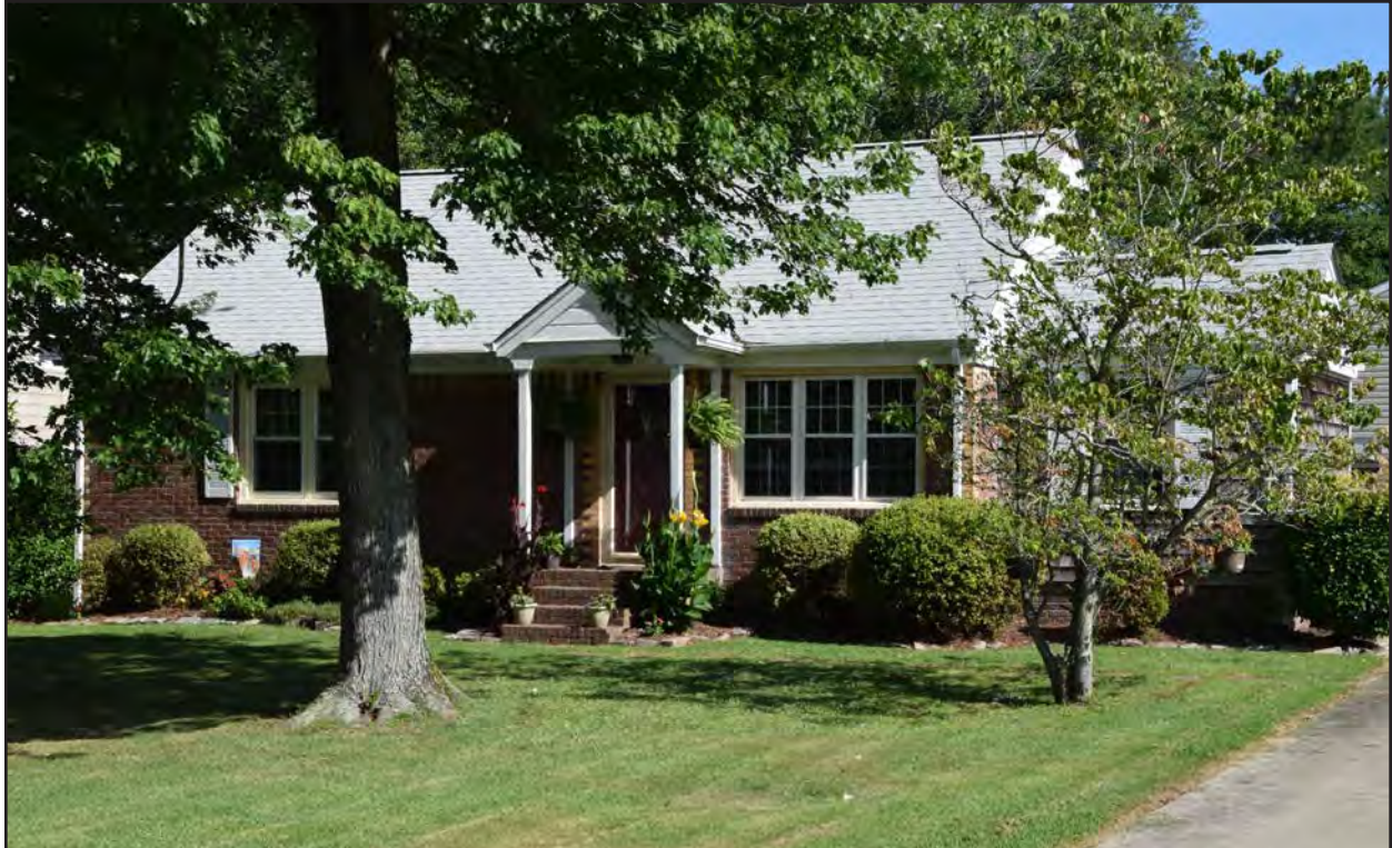
Figure 204. 134-5224, dwelling, south and east elevations, view to the northwest. 134
