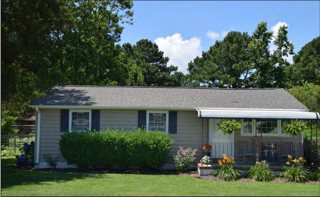
Figure 293. 134-5957, dwelling, northeast elevation.
