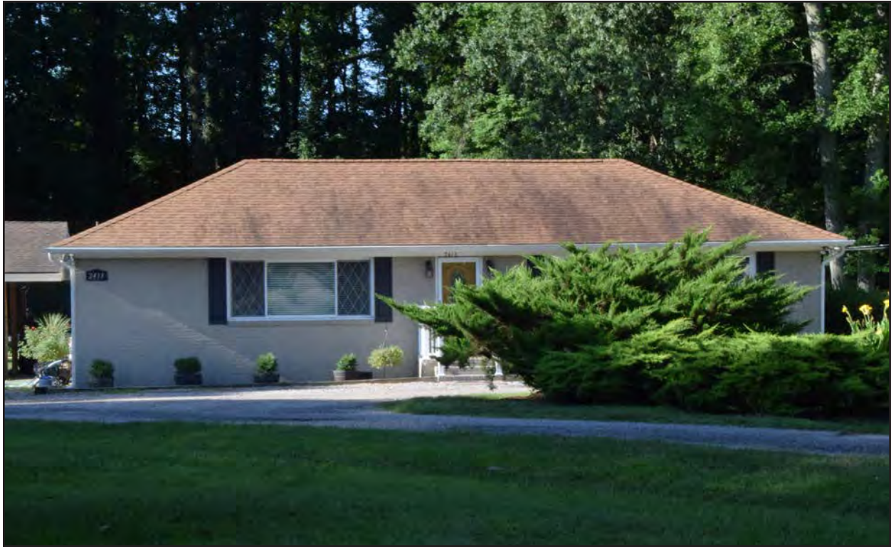
Figure 261. 134-5921, dwelling, north elevation, view to the south.
