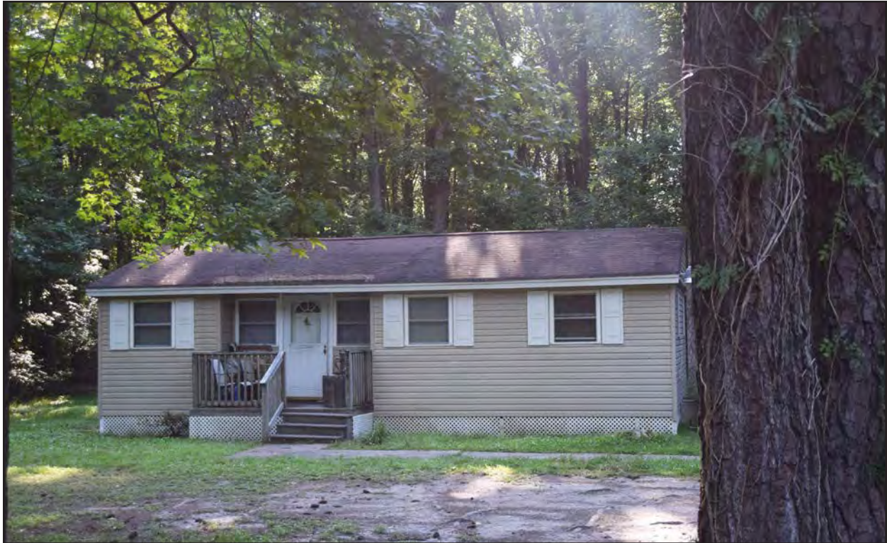
Figure 237. 134-5897, compact Ranch, west elevation, view to the east.
