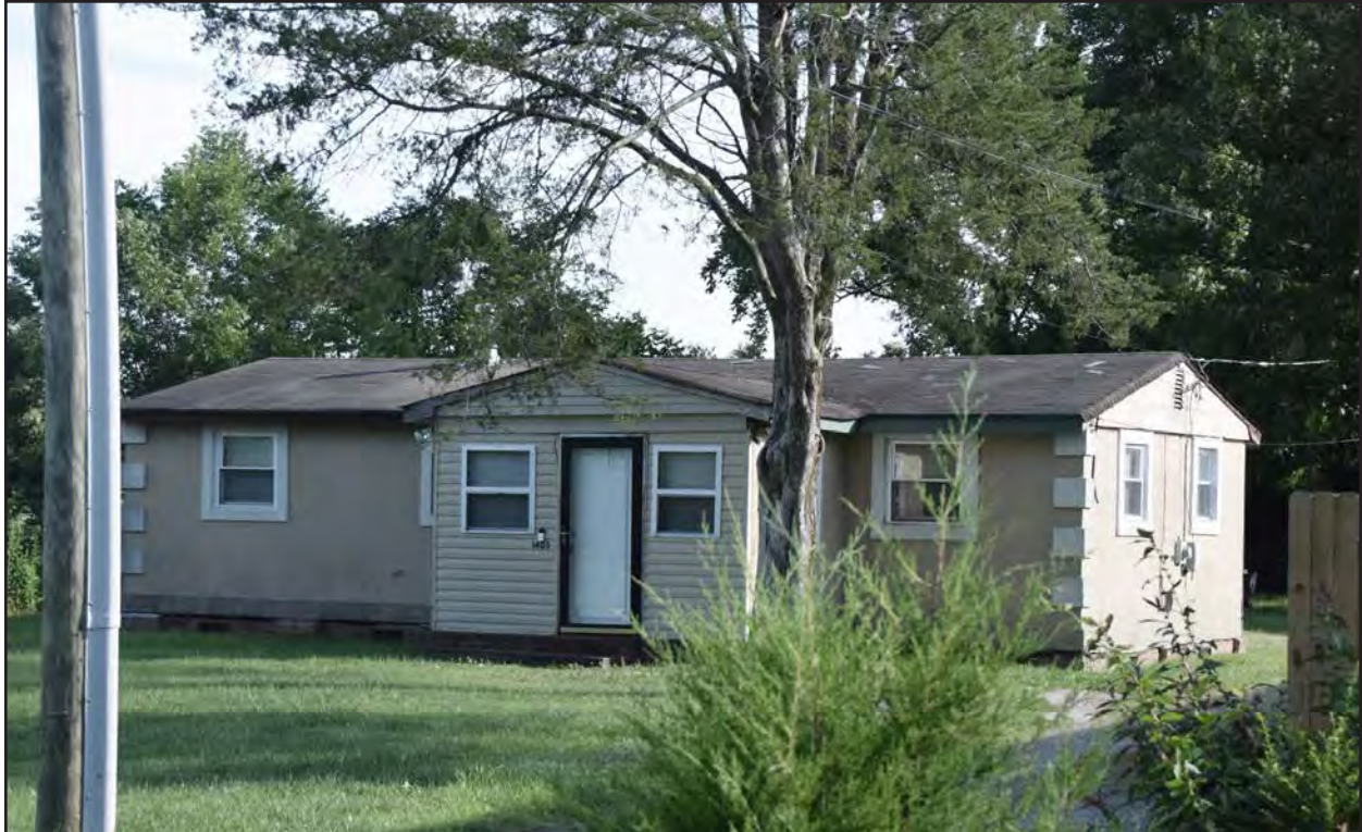
Figure 46. 131-5994, Ranch, southwest and southeast elevations, view to the north.
