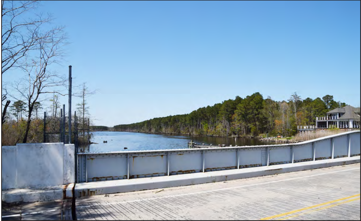
Figure 3: 131-5333, Albemarle & Chesapeake Canal Historic District, view to the northwest.
