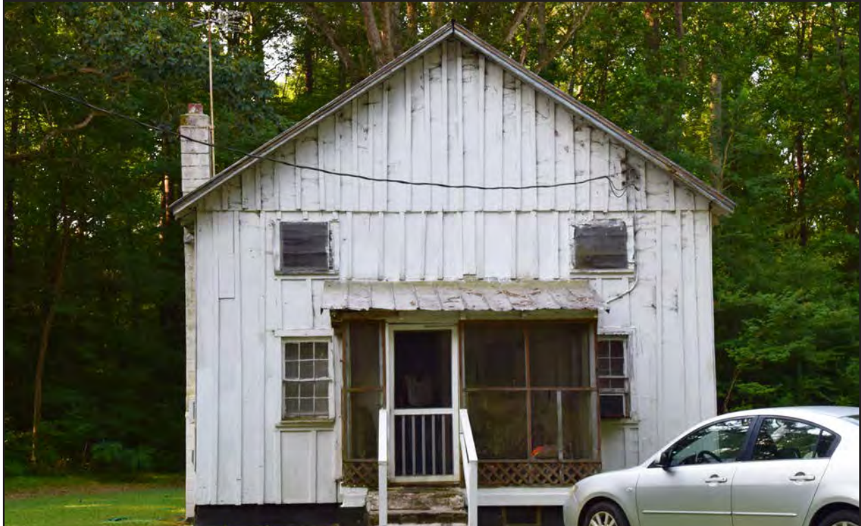
Figure 140. 131-6259, vernacular dwelling, north elevation, view to the south.
