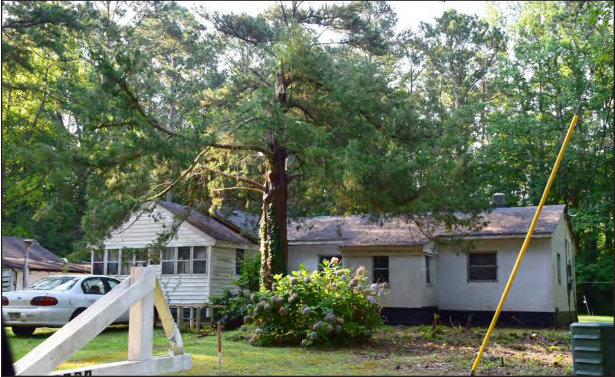
Figure 115. 131-6232, dwelling, northwest and southwest elevations.
