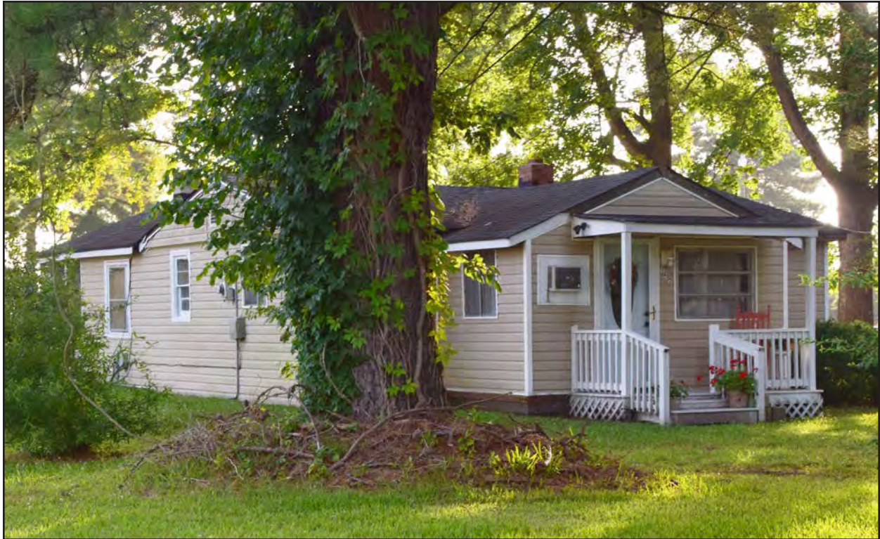
Figure 39. 131-5987, dwelling, southwest and northwest elevations, view to the east.
