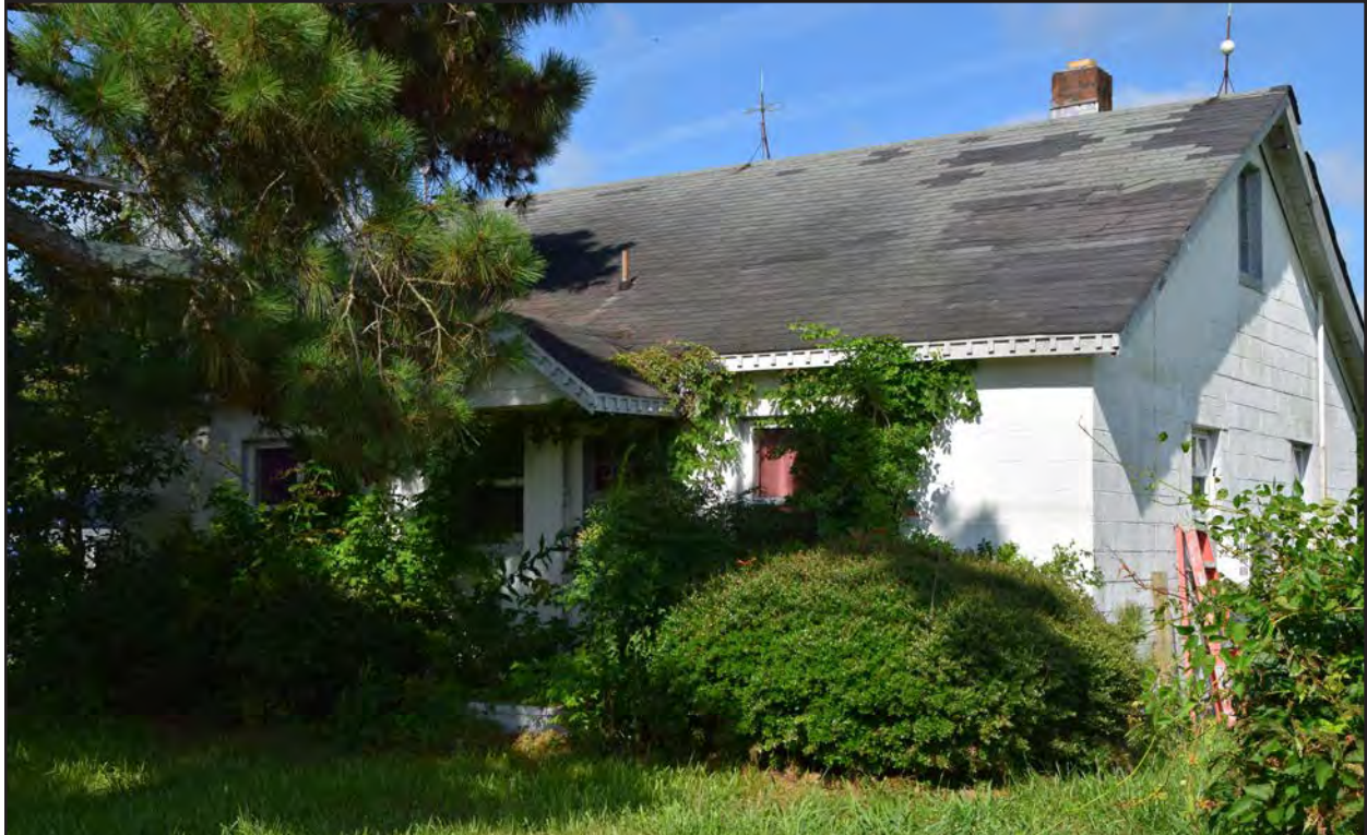
Figure 24. 131-5886, worker house, east and north elevations, view to the southwest.
