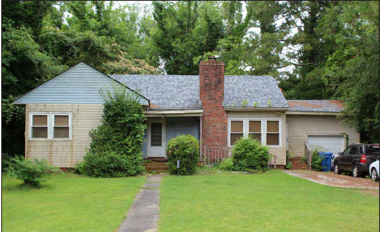
Figure 74. 131-6191, Minimal Traditional dwelling, northeast elevation, view to the southwest.
