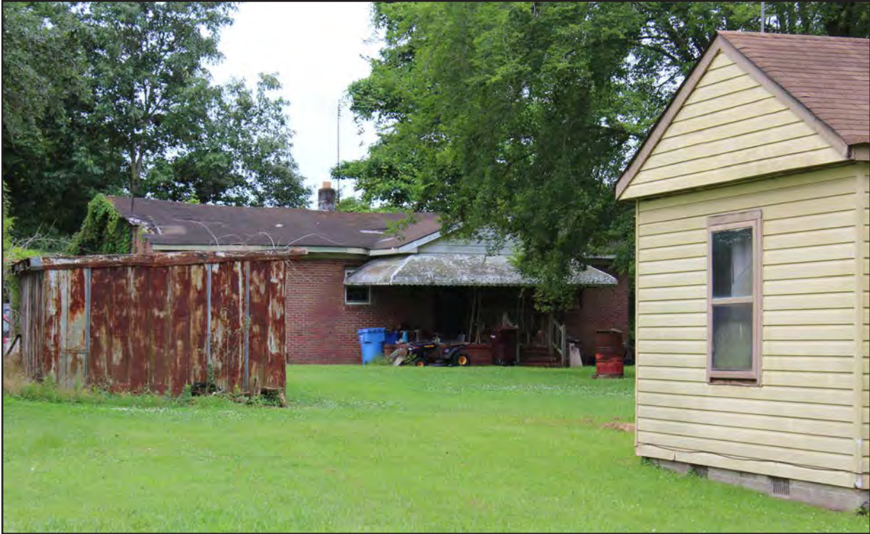
Figure 72. 131-6188, northeast and southeast elevations, view to the south.
