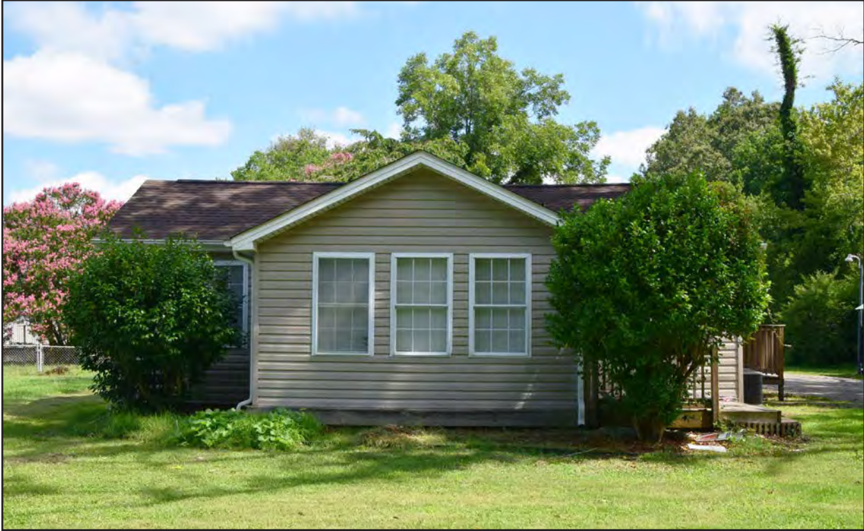
Figure 103: 131-6220, vernacular dwelling, south elevations, view to the north.
