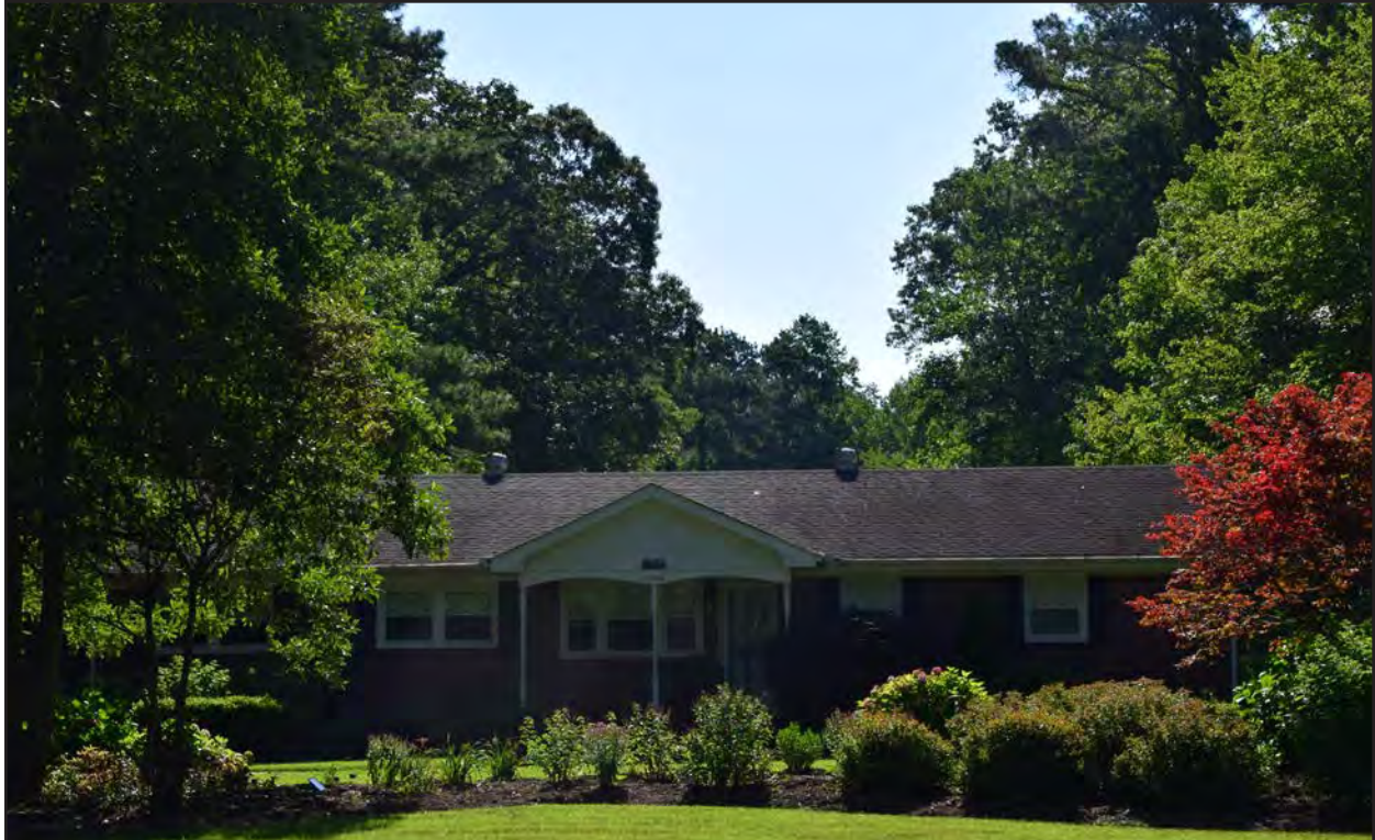
Figure 226. 134-5885, linear Ranch dwelling, west elevation, view to the east.
