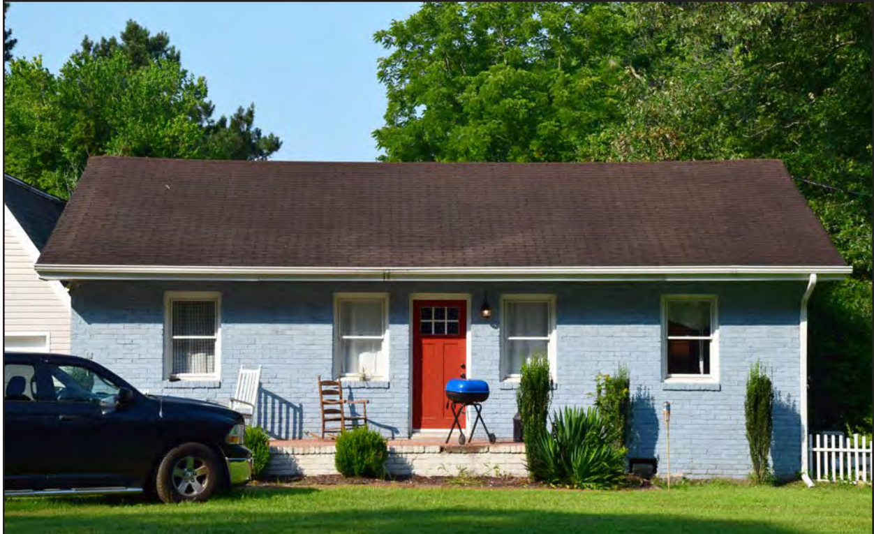
Figure 126. 131-6243, compact Ranch, northeast elevation, view to the southwest.
