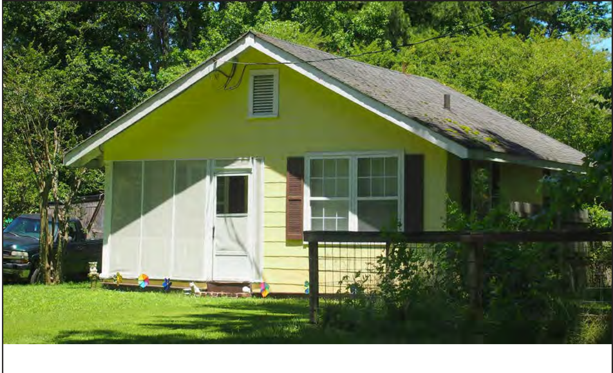
Figure 172. 134-0920, Craftsman dwelling, south and east elevations, view to the northwest.
