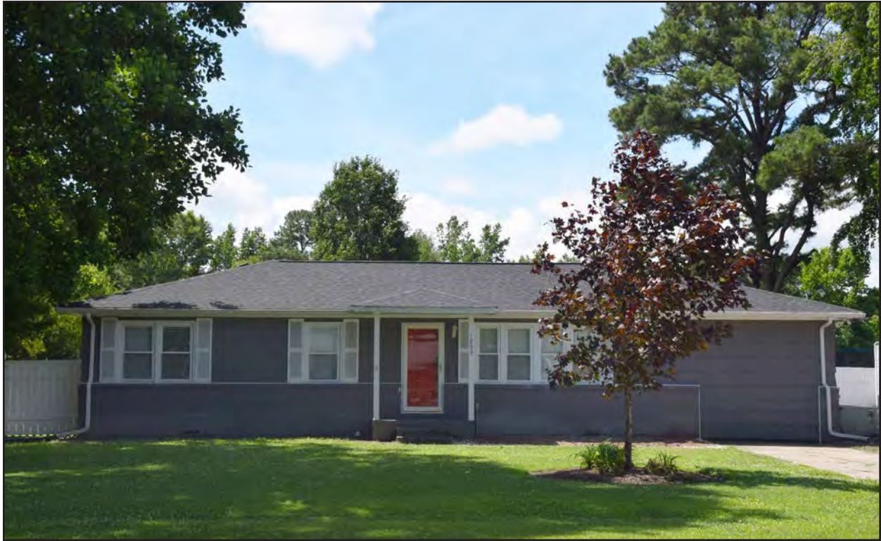
Figure 199. 134-5219, linear Ranch, north elevation, view to the south.
