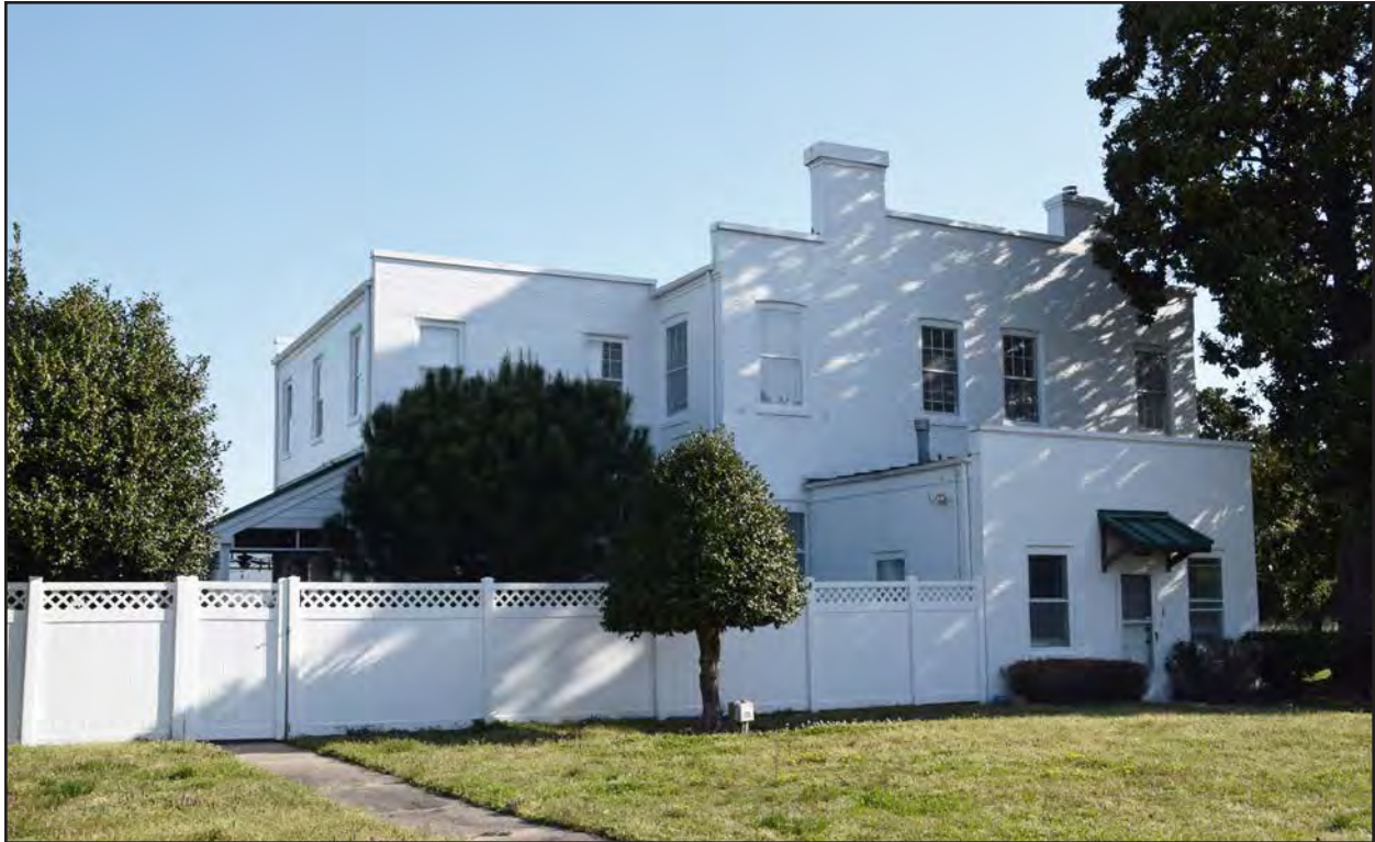
Figure 157. 134-0003, James Bell House showing additions, south and west elevations, view to the northeast.
