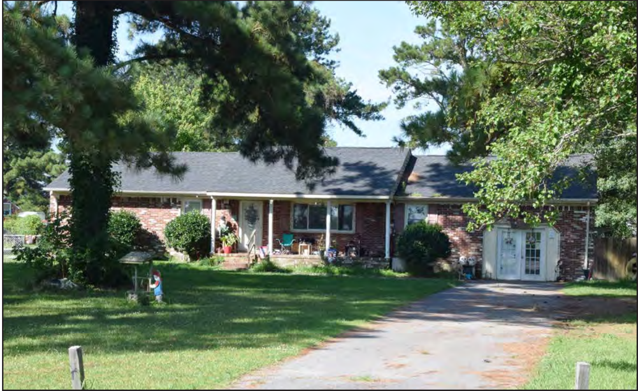
Figure 153. 131-6271, linear Ranch, northeast elevation, view to the southwest.
