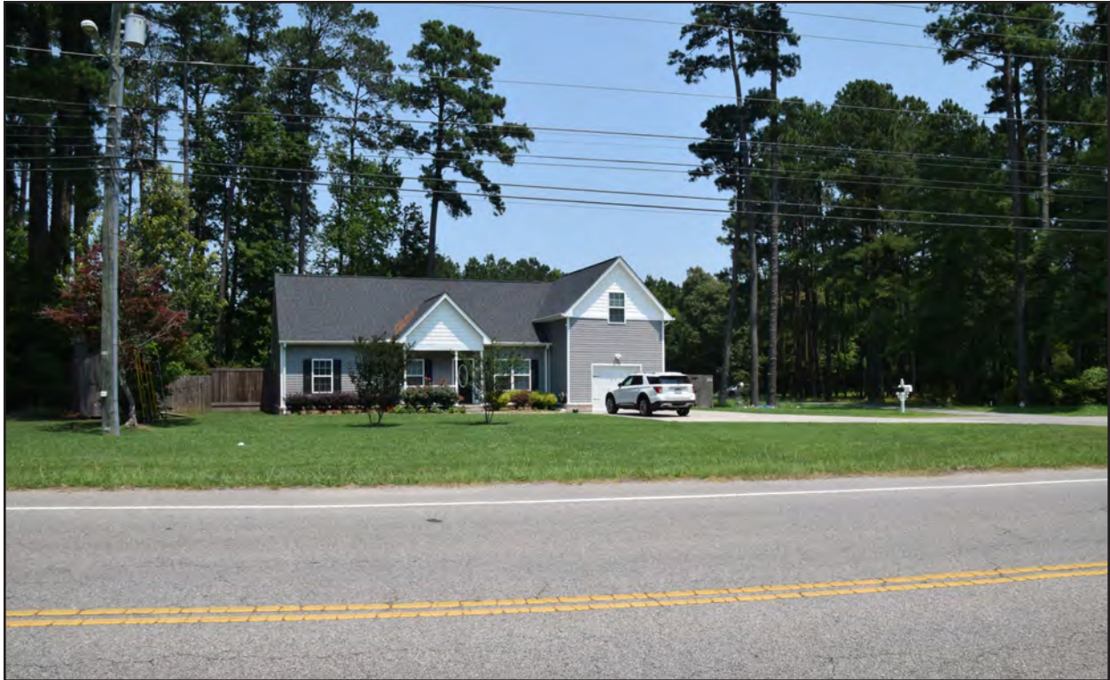
Figure 17. 131-5378, Colonial Revival dwelling, no longer extant, view to the northwest.
