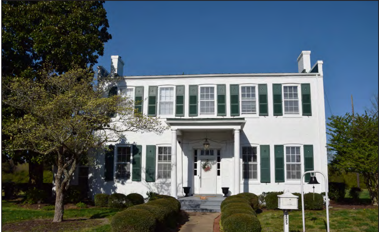
Figure 4: 134-0003/134-5027-0004, James Bell House, east elevation, view to the west.
