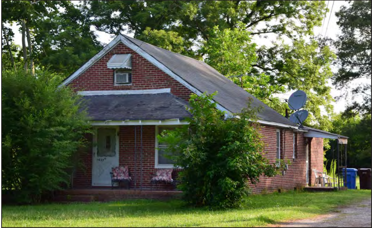
Figure 33. 131-5981, vernacular dwelling, southwest and southeast elevations, view to the north.
