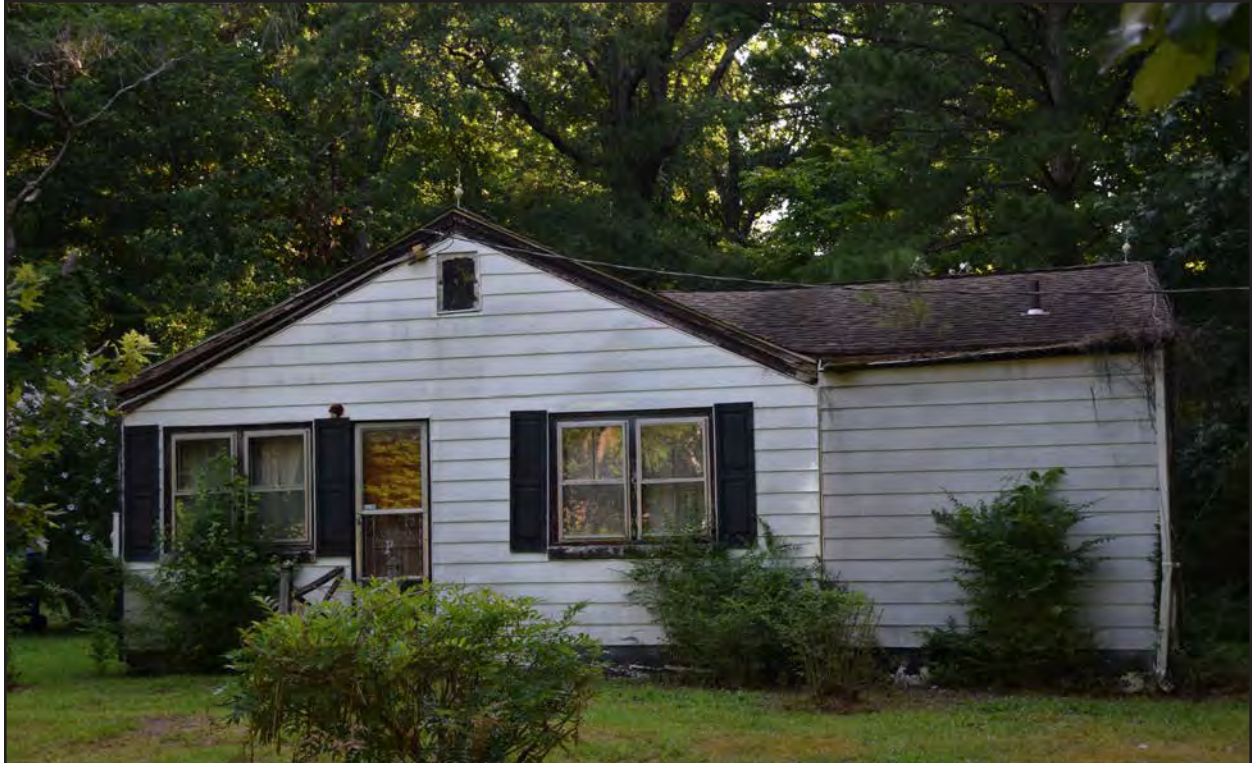
Figure 270. 134-5930, dwelling, southwest elevation, view to the northeast.
