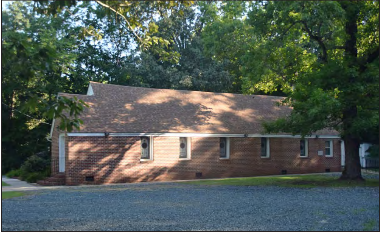
Figure 217. 134-5848, Campbell's Chapel AME Church, southeast elevation, view to the northwest.
