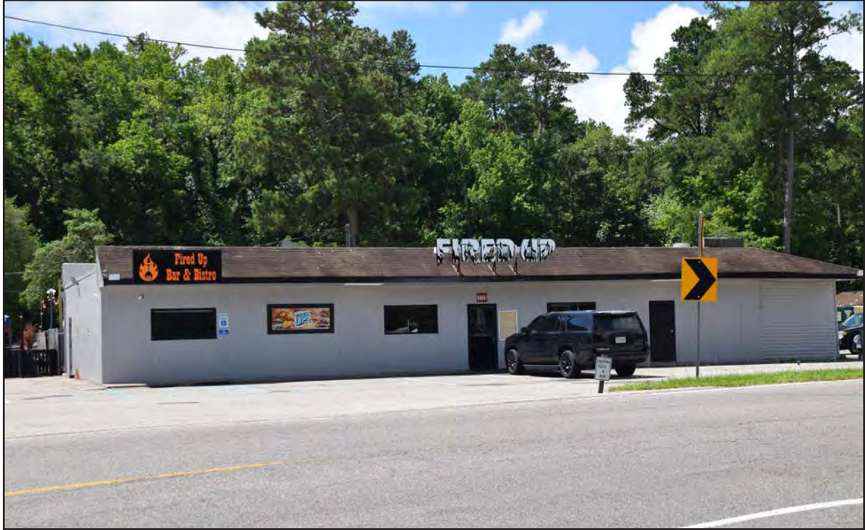
Figure 277. 134-5941, commercial structure, north and east elevations, view to the southwest.
