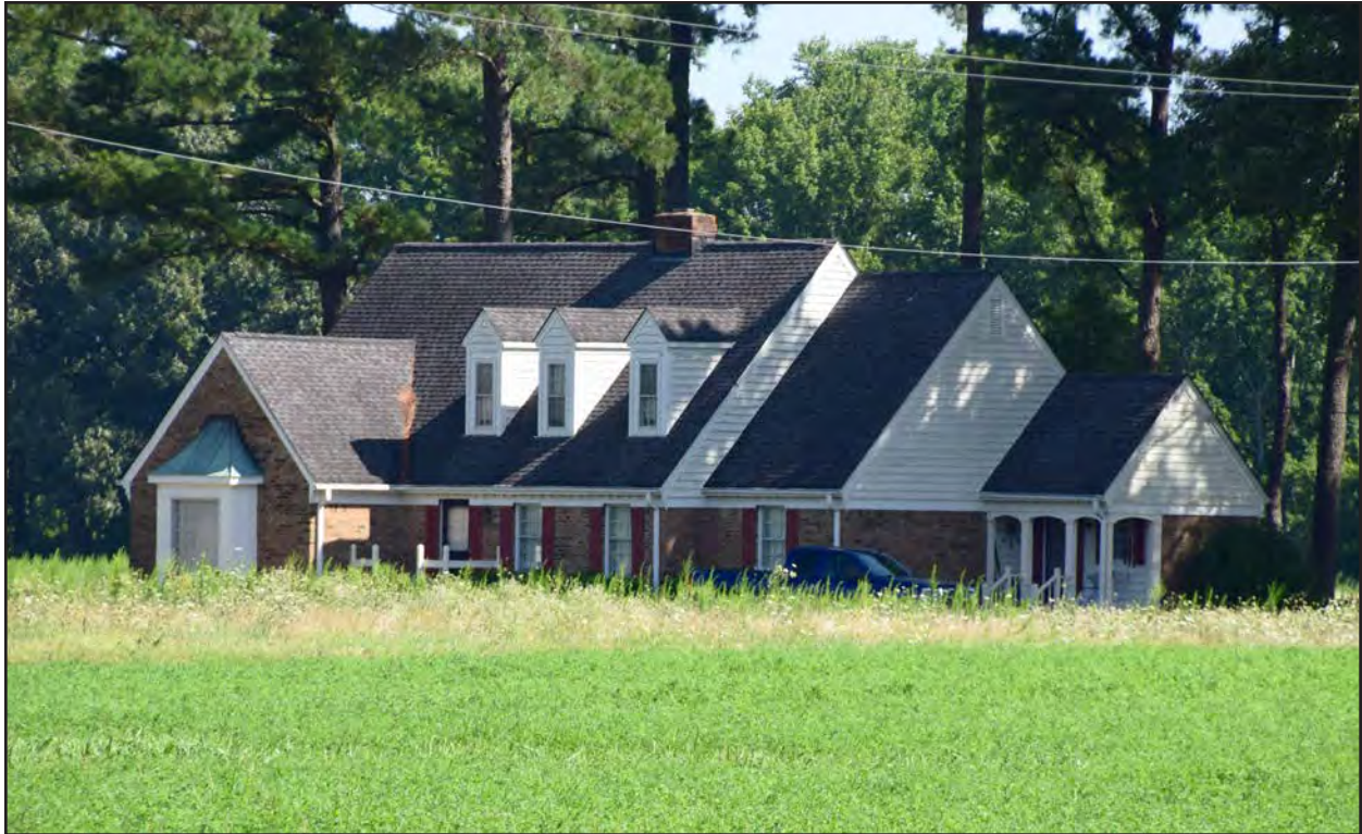
Figure 123. 131-6240, Neo-eclectic dwelling, southwest and southeast elevations, view to the north.
