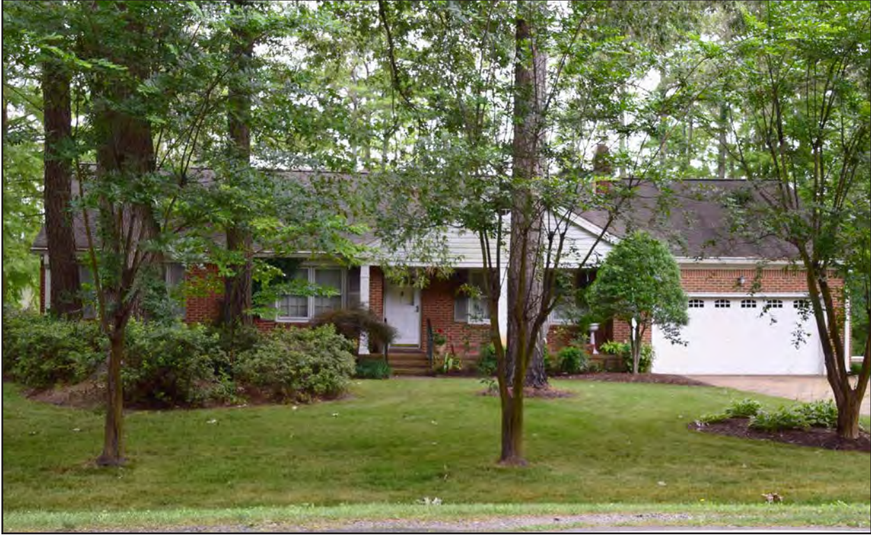
Figure 212. 134-5678, dwelling, east elevation, view to the west.
