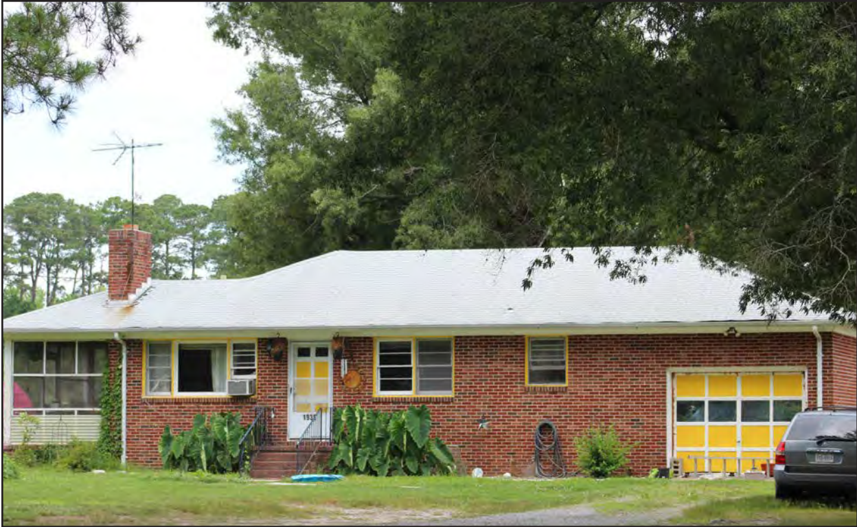
Figure 220. 134-5879, linear ranch, west and south elevations, view to the northeast.
