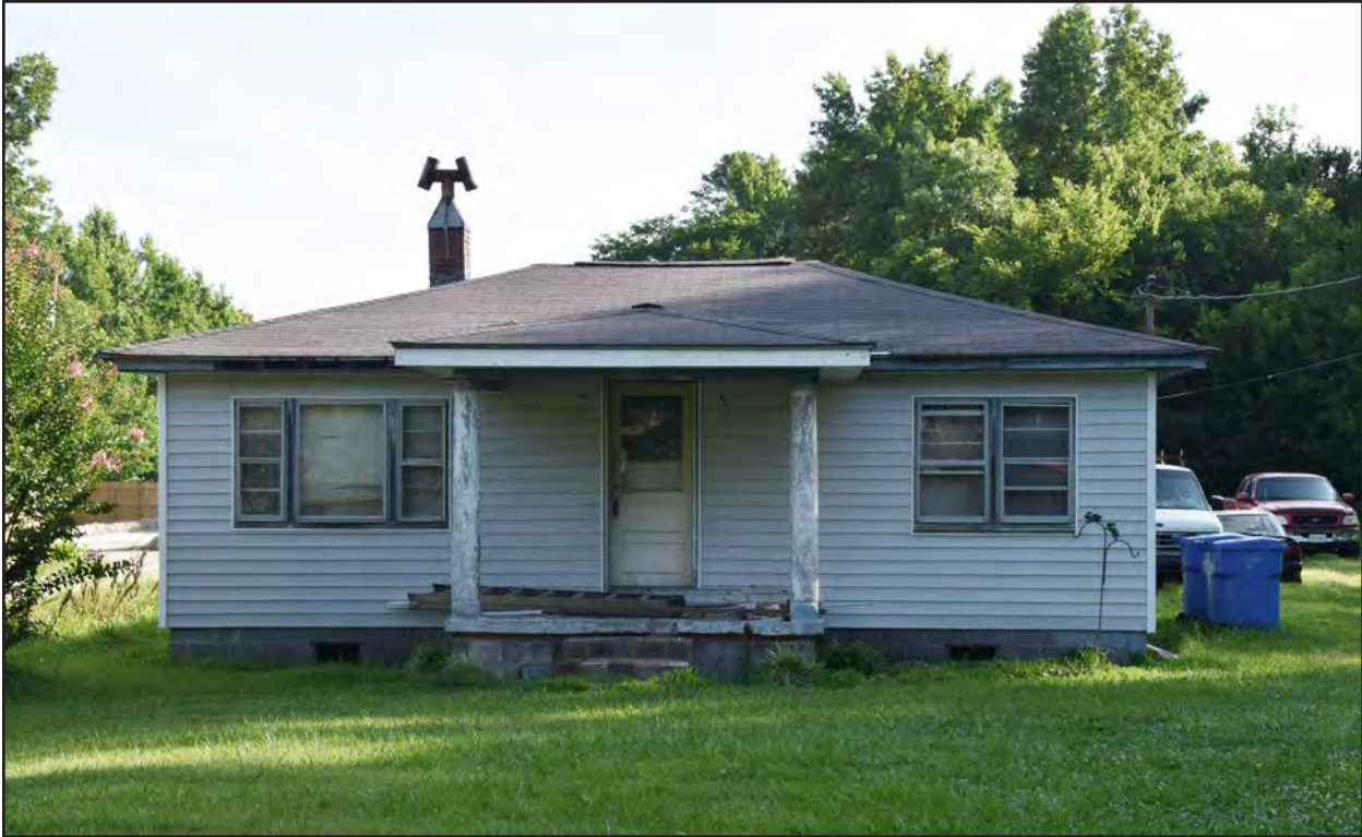
Figure 44. 131-5992, primary dwelling, southwest elevation, view to the northeast
