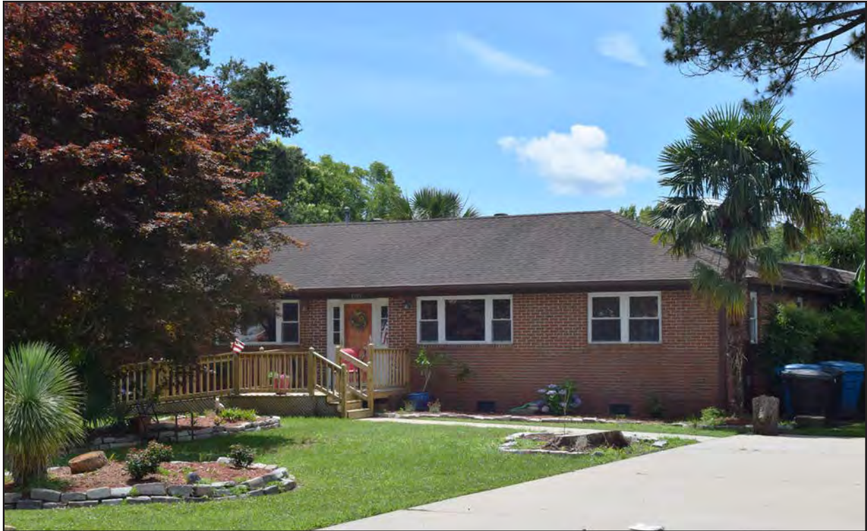
Figure 197. 134-5216, linear Ranch dwelling, north and west elevations, view to the southeast.
