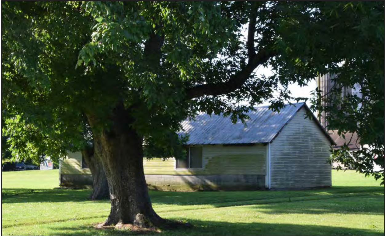
Figure 23. 131-6190, Kurtz Farm, Structure 2, north elevation, view to the south.
