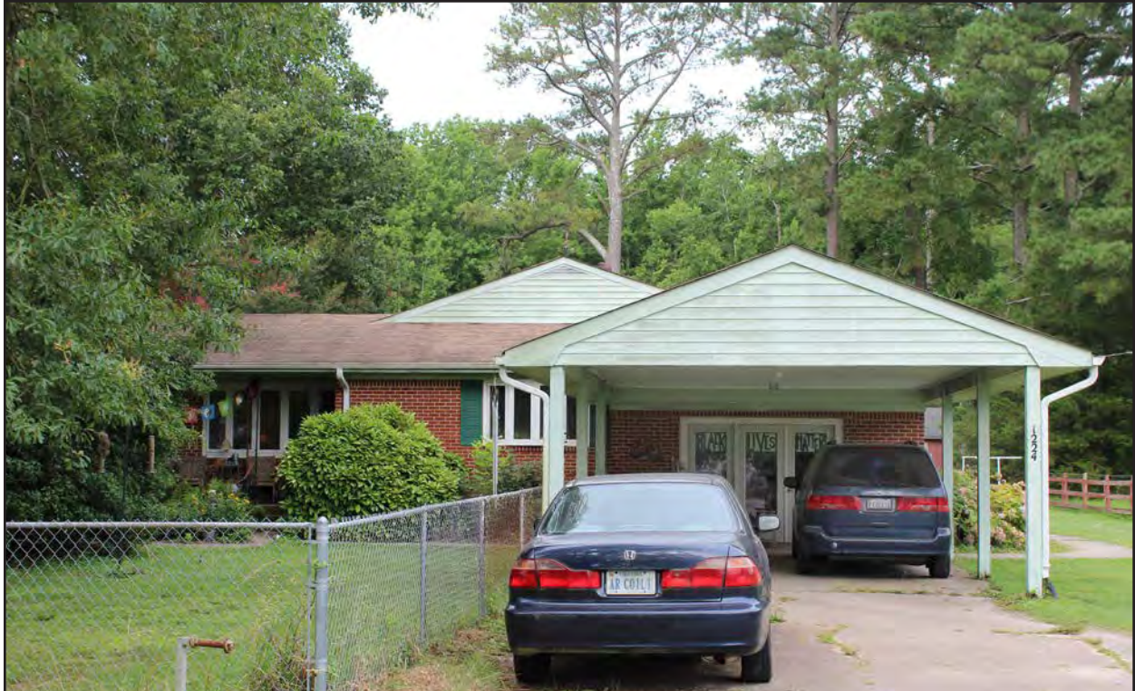
Figure 106. 131-6223, Ranch, east elevation, view to the west.
