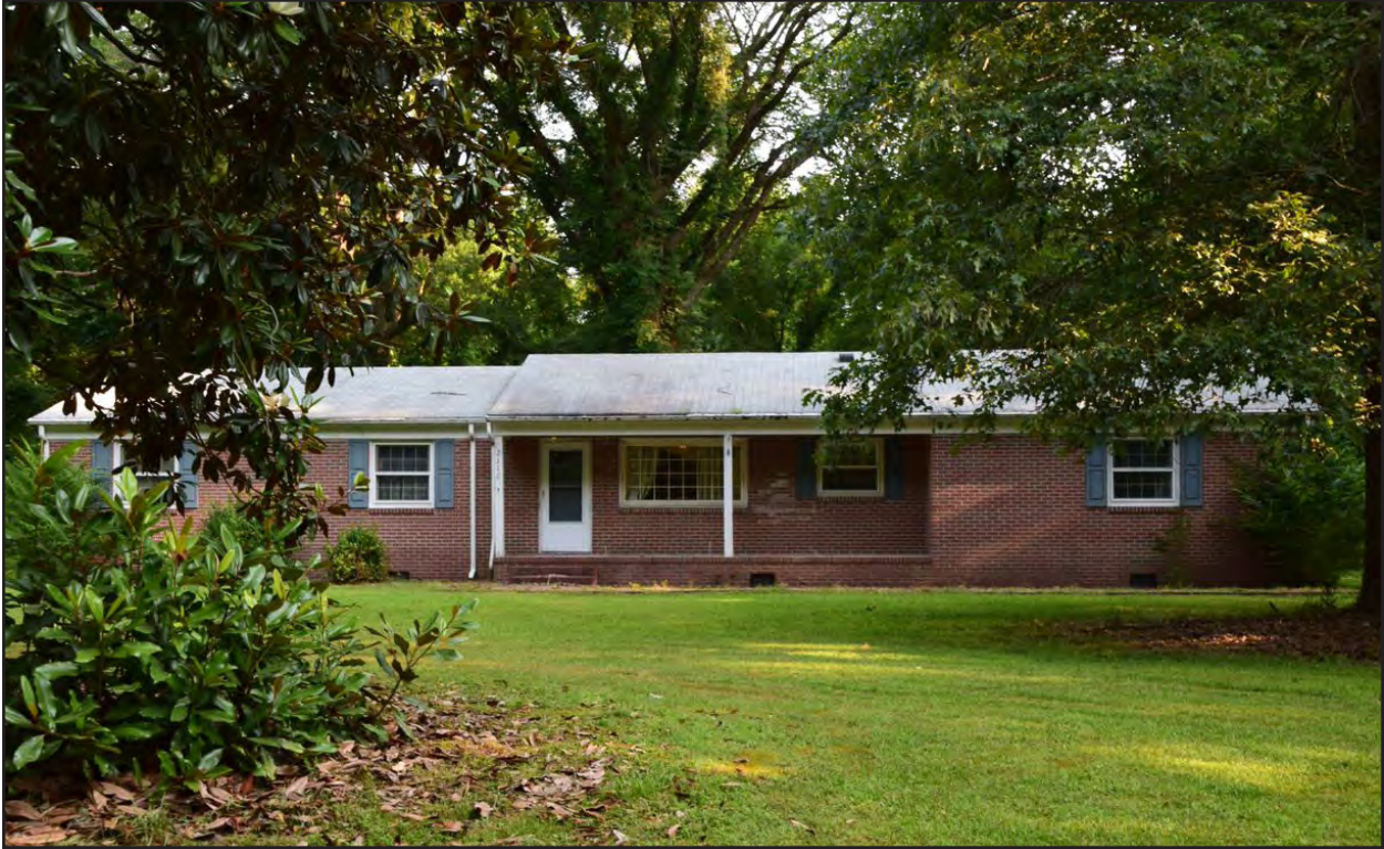
Figure 141. 131-6260, linear Ranch, south elevation, view to the north.
