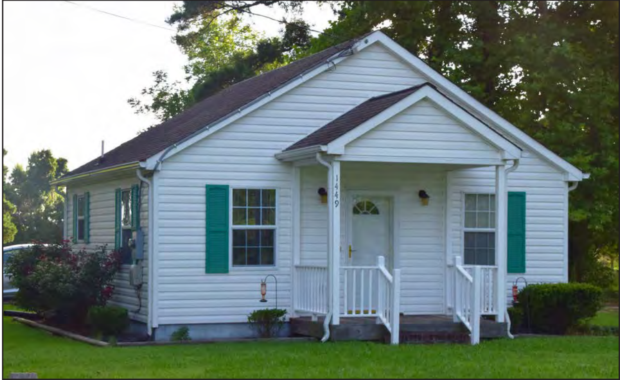
Figure 35. 131-5983, Minimal Traditional dwelling, southwest and northwest elevations, view to the east.
