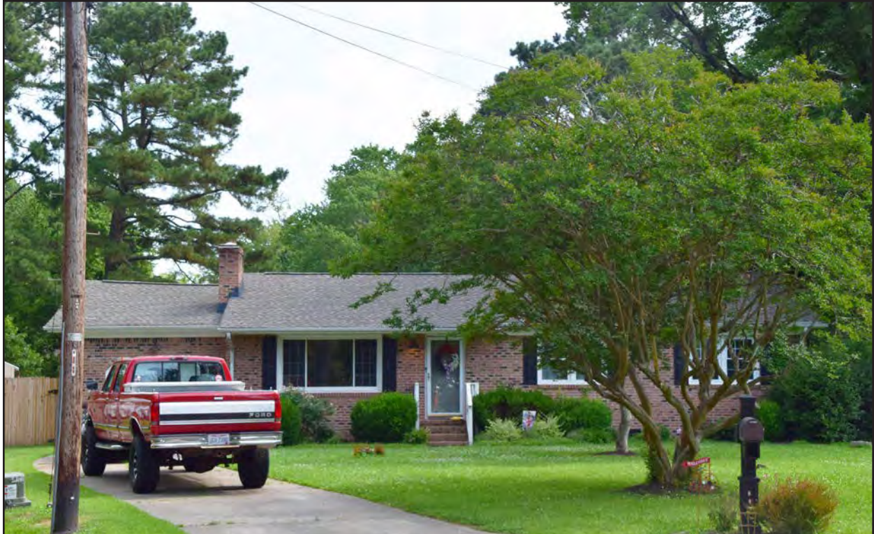
Figure 78. 131-6195, linear ranch, south elevation, view to the north.
