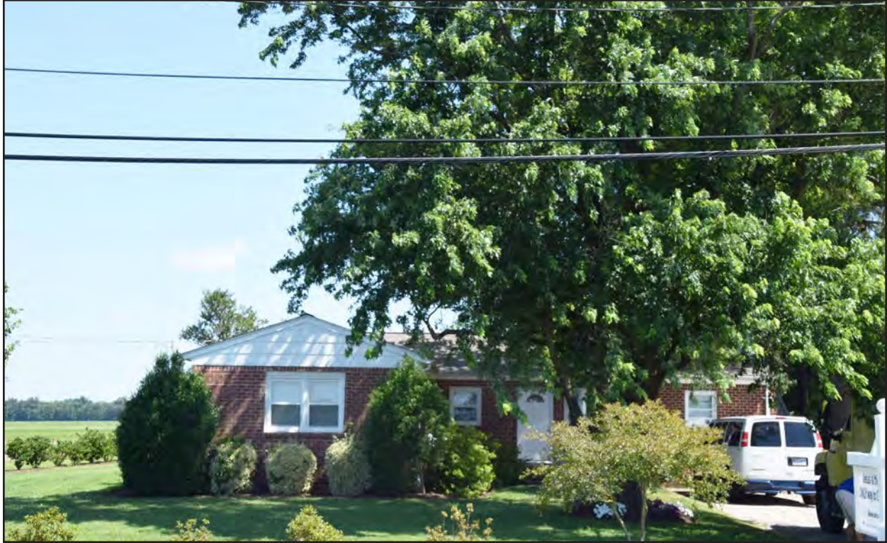
Figure 231. 134-5890, dwelling, south elevation, view to the north.
