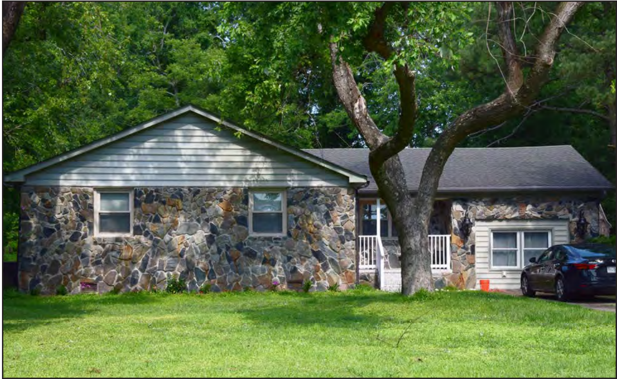
Figure 85. 131-6202, half-courtyard Ranch, east elevation, view to the west.
