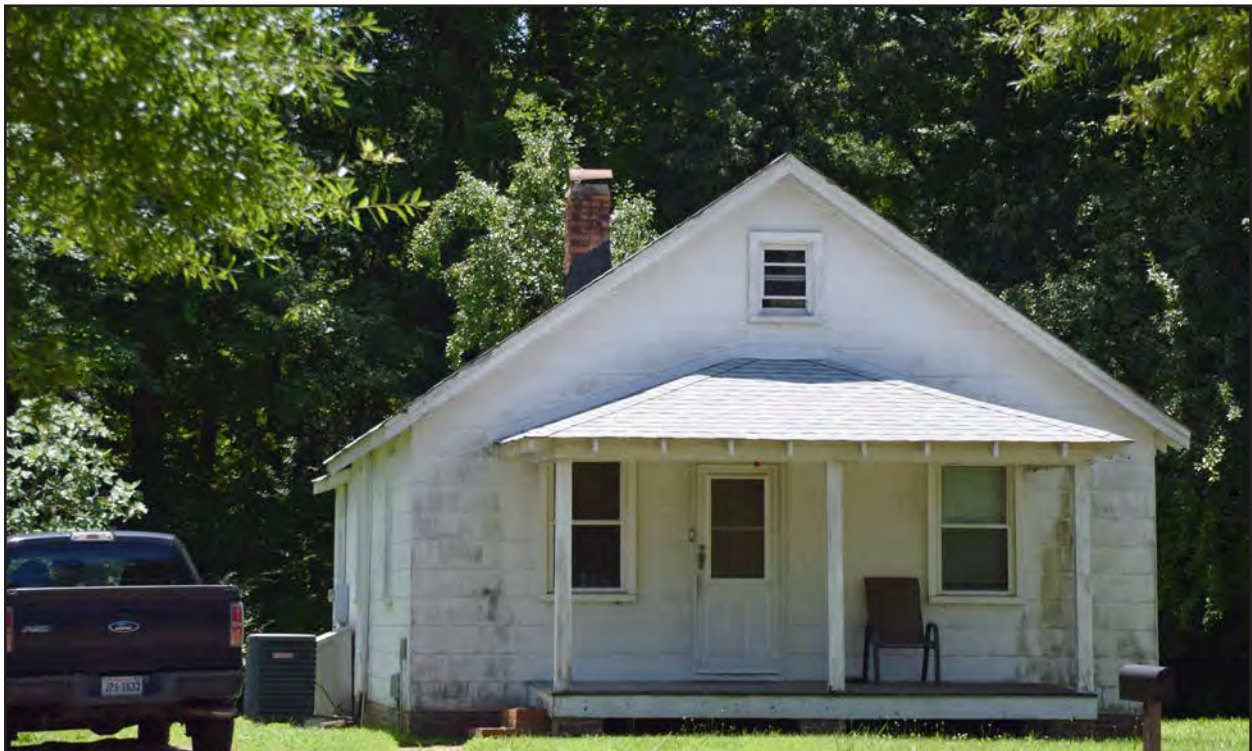
Figure 162. 134-0101, Craftsman dwelling, north elevation, view to the south.
