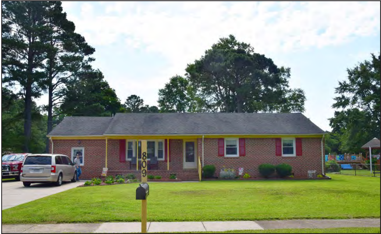
Figure 79. 131-6196, linear Ranch, west elevation, view to the east.
