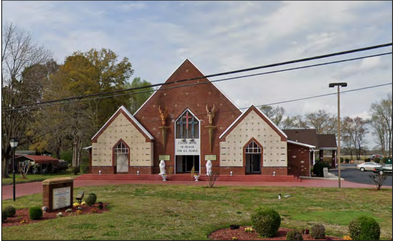
Figure 59. 131-6014, The United House of Prayer for All People Church, south elevation, view to the north.
