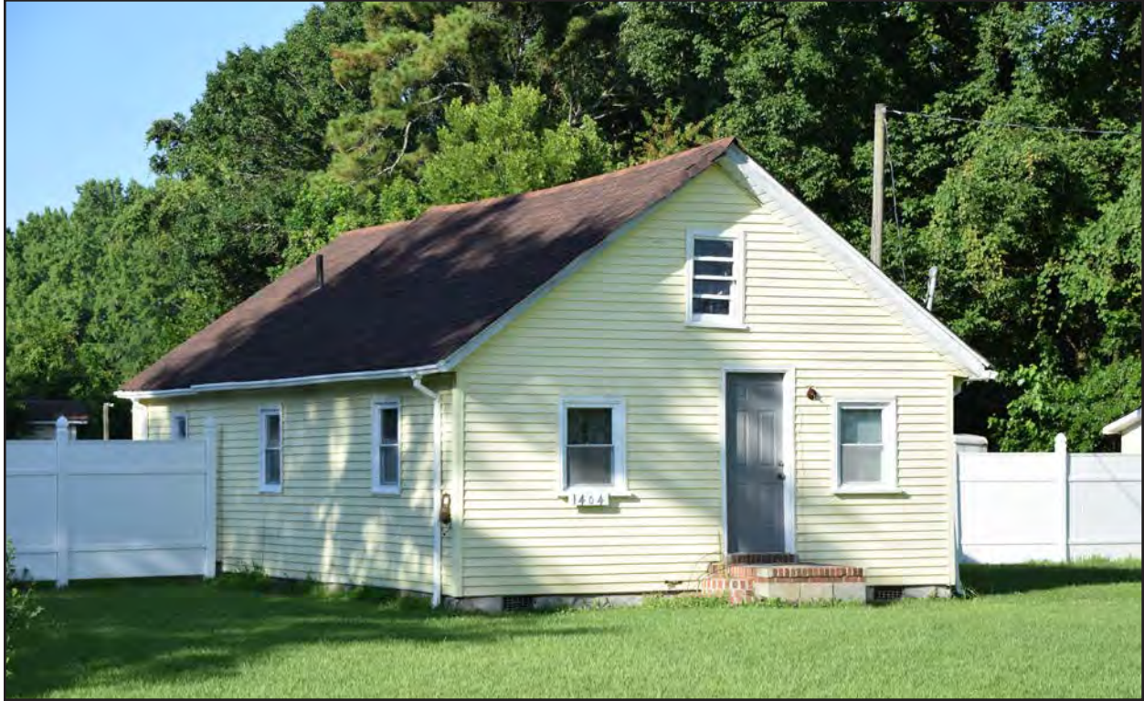
Figure 47. 131-5995, vernacular dwelling, northeast and southeast elevations, view to the west.
