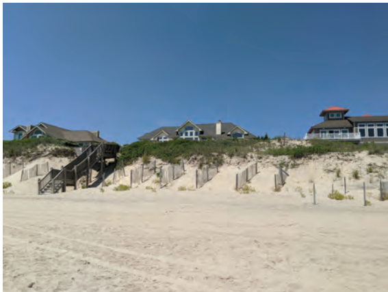
1: West-facing view toward foredune and beach front residences
