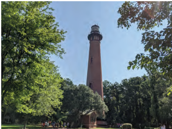
1: Exterior view of Currituck Beach Lighthouse, facing east
