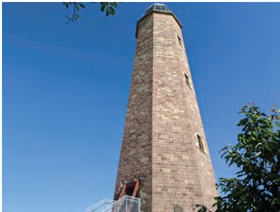
1: Exterior View of Old Cape Henry Lighthouse
