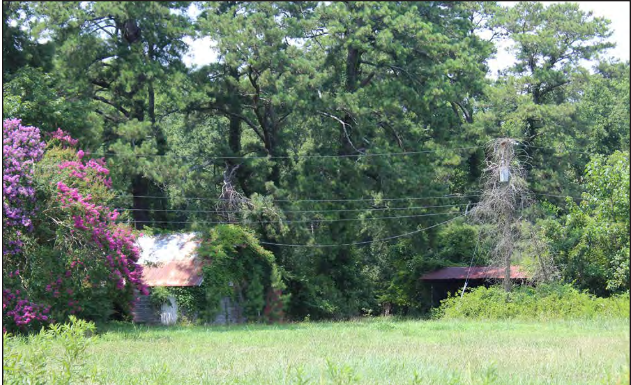
Figure 292. 134-5956, workshop, south and east elevations, view to the northwest.
