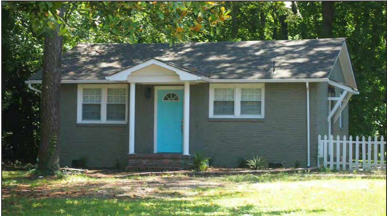
Figure 249. 134-5909, American Small House, north and west elevations, view to the southeast.
