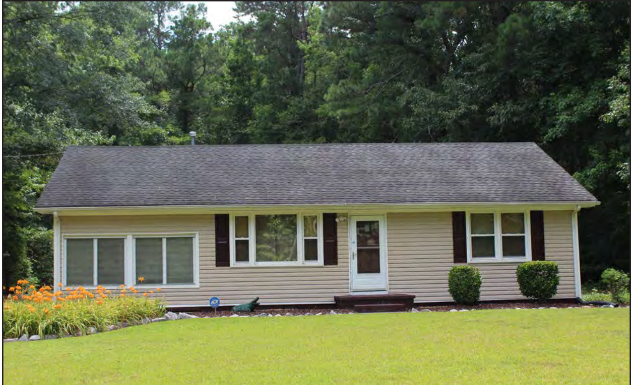
Figure 284. 134-5948, compact Ranch dwelling, northeast elevation, view to the southwest.
