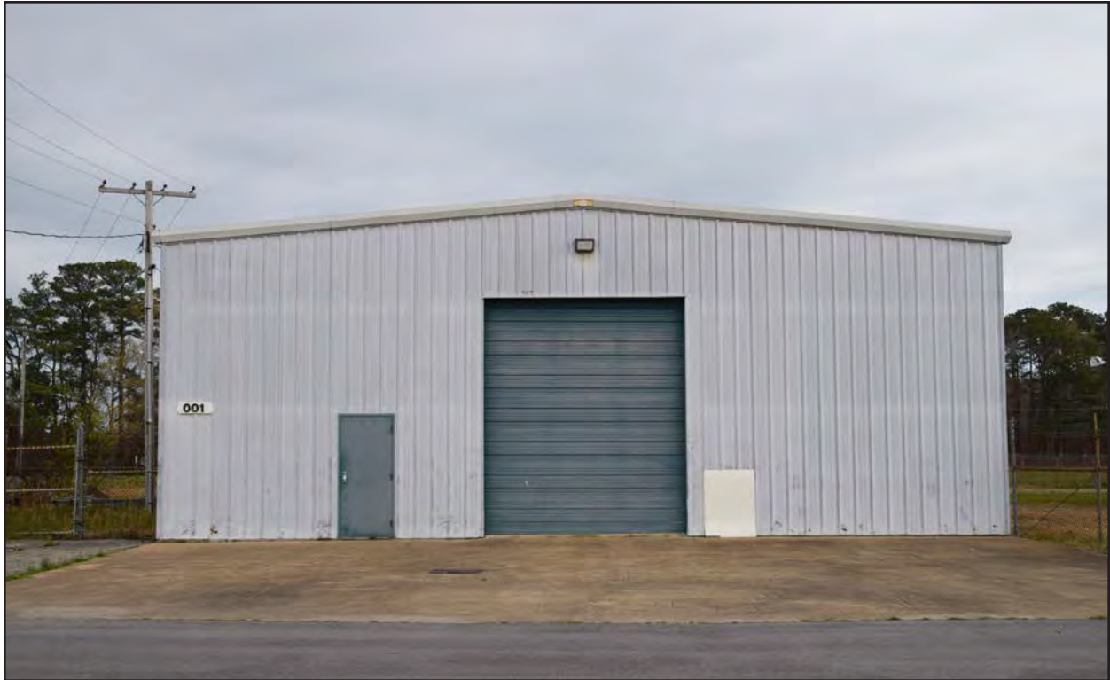
Figure 171. 134-0413-0110, Building 1, south elevation, view to the north
