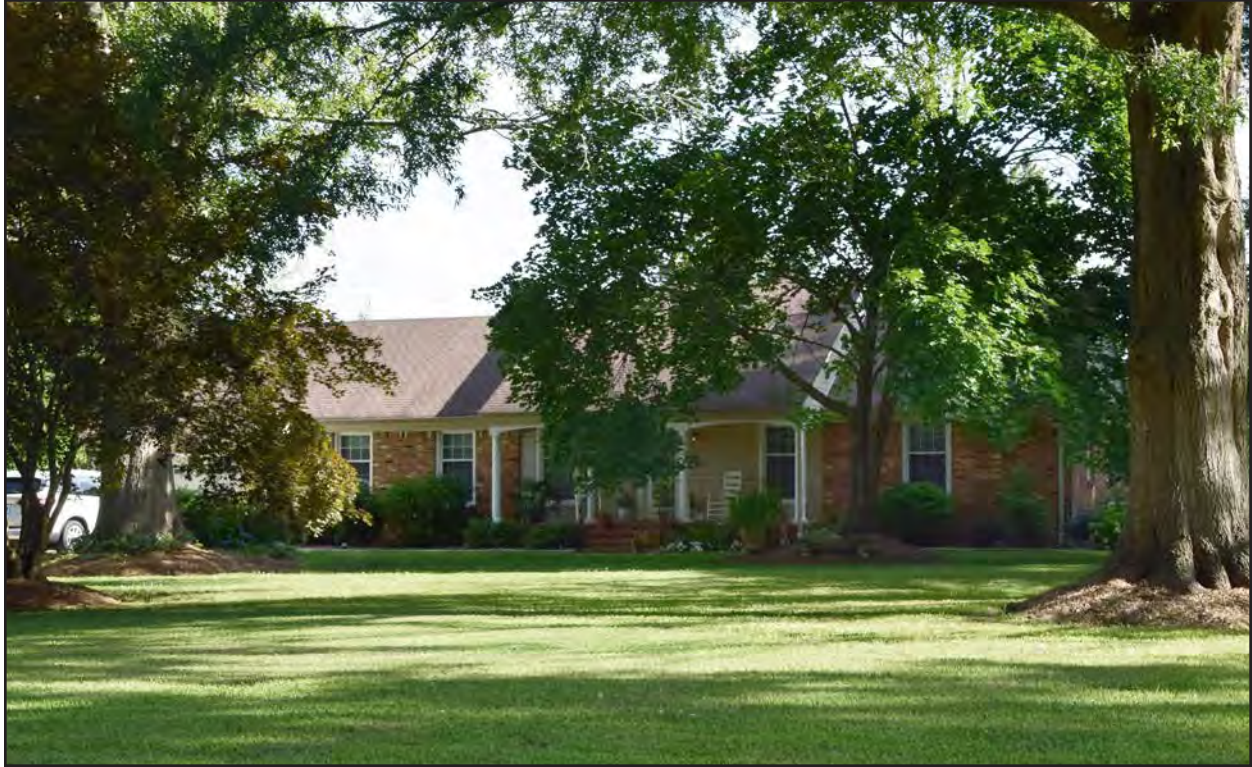
Figure 93. 131-6210, linear Ranch dwelling, south elevation, view to the north-northeast.
