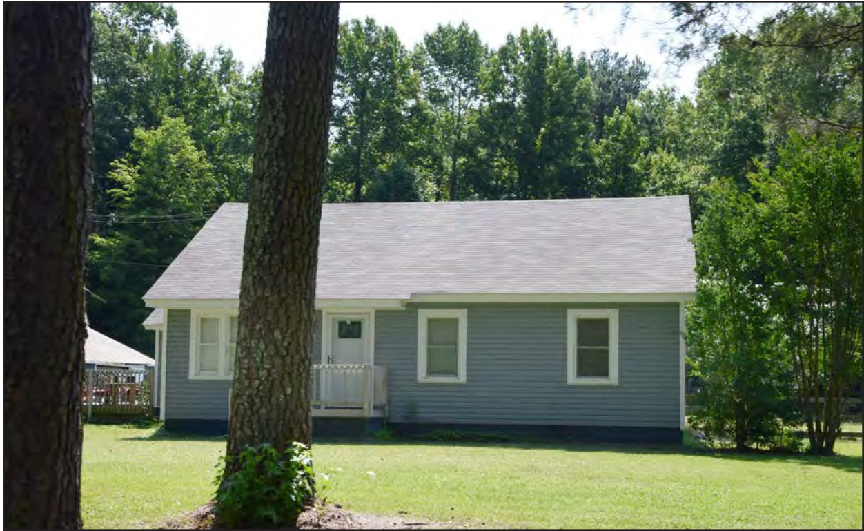
Figure 127. 131-6244, American Small House, northwest elevation, view to the southeast.
