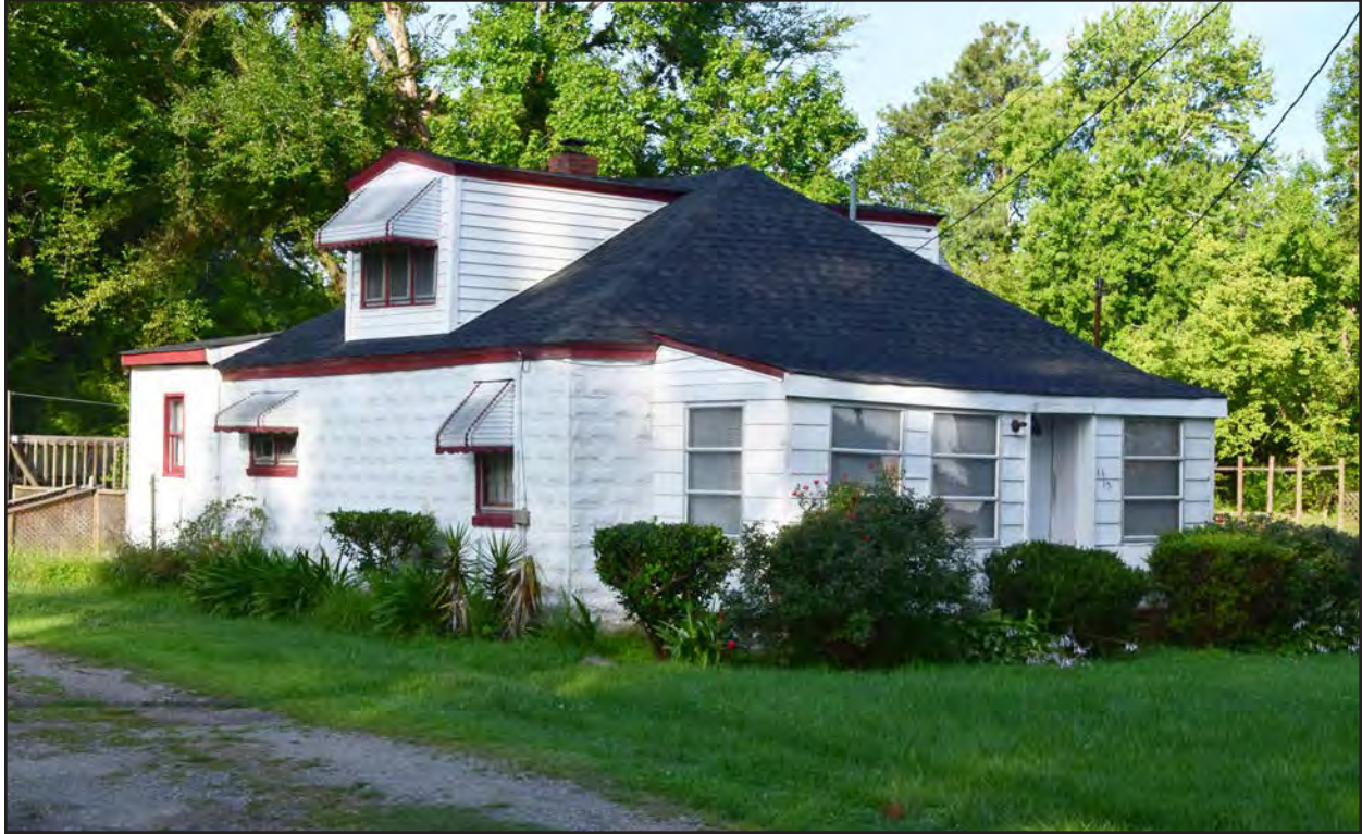
Figure 49. 131-5997, dwelling, northeast and southeast elevations, view to the west.
