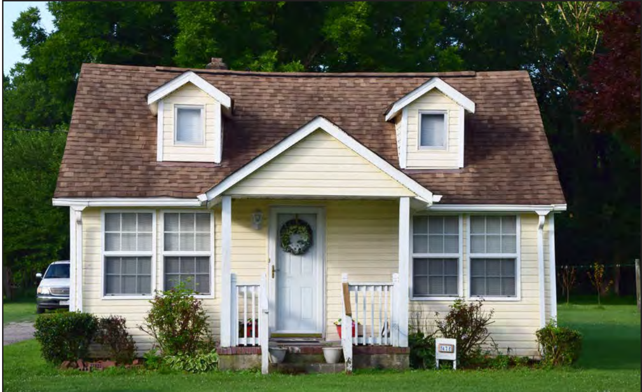
Figure 50. 131-5998, Cape Cod dwelling, northeast elevation, view to the southwest.
