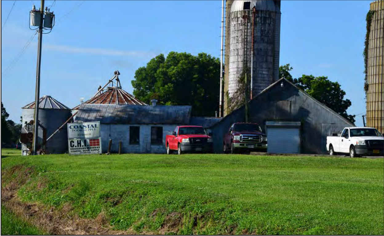
Figure 22. 131-6190, Kurtz Farm, Structure 1, north and west elevations, view to the southeast
