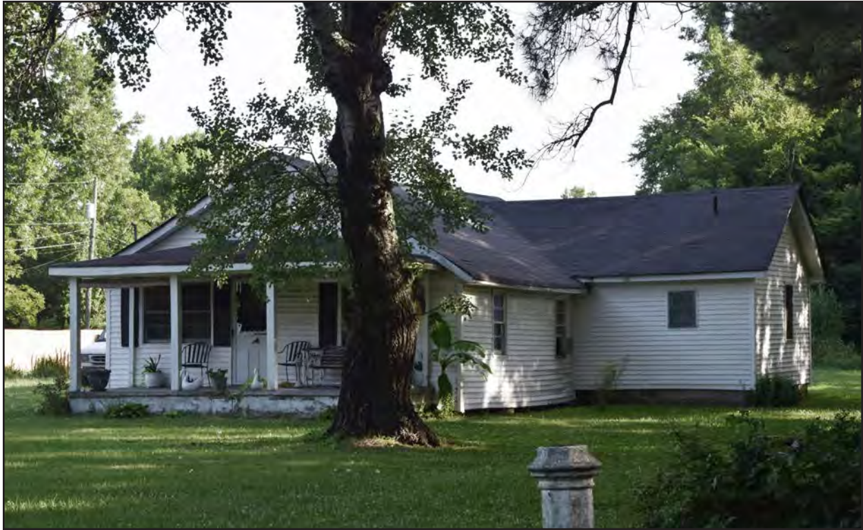
Figure 45. 131-5992, secondary dwelling, southwest and southeast elevations, view to the north.
