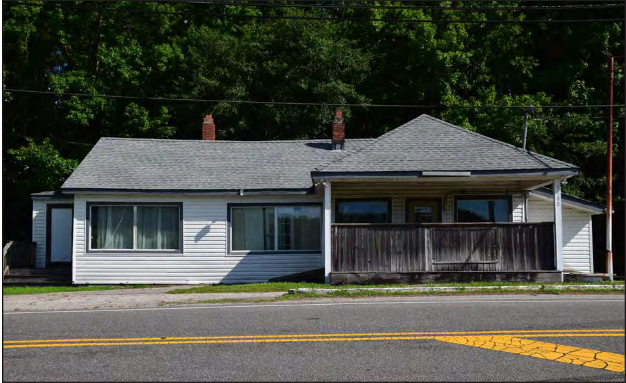
Figure 243. 134-5903, general store, southeast elevation, view to the northwest.
