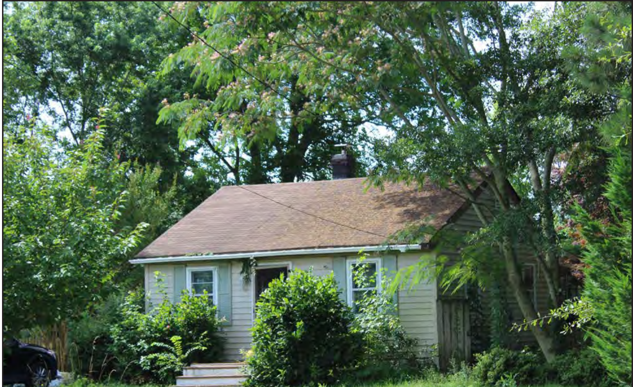
Figure 290. 134-5953, Minimal Traditional dwelling, north elevation, view to the southeast.
