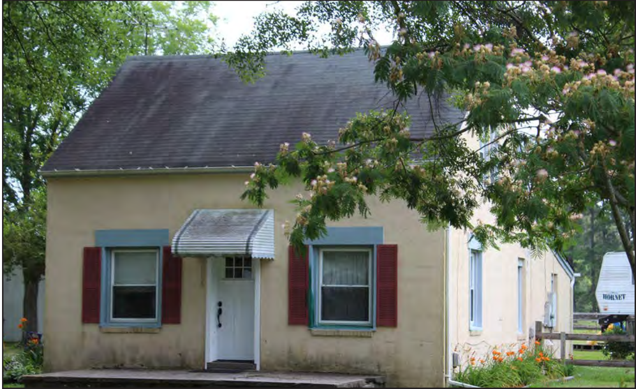
Figure 139. 131-6258, vernacular dwelling, west and south elevations, view to the northeast.
