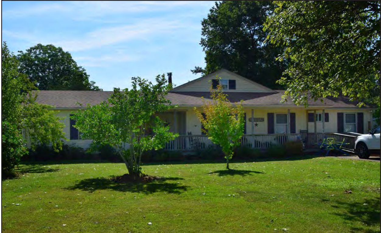
Figure 112. 131-6229, Ranch dwelling, west elevation, view to the east.
