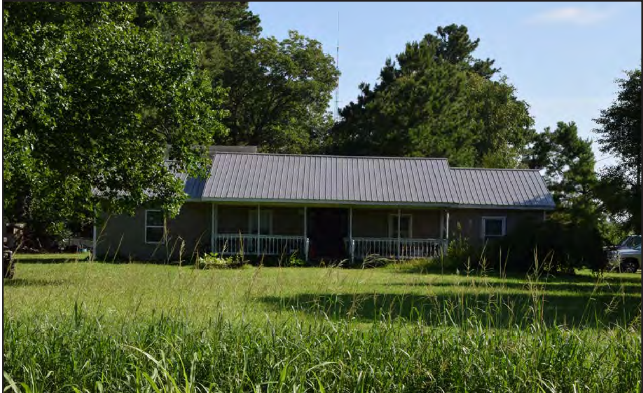
Figure 28. 131-5891, dwelling, south elevation, view to the north.
