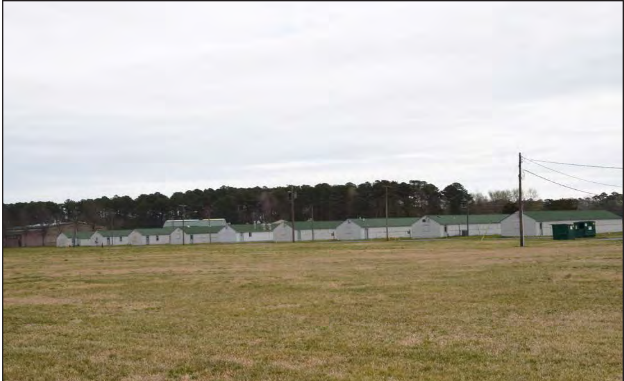
Figure 170. 134-0413, Camp Pendleton/State Military Reservation, overview, view to the northeast.
