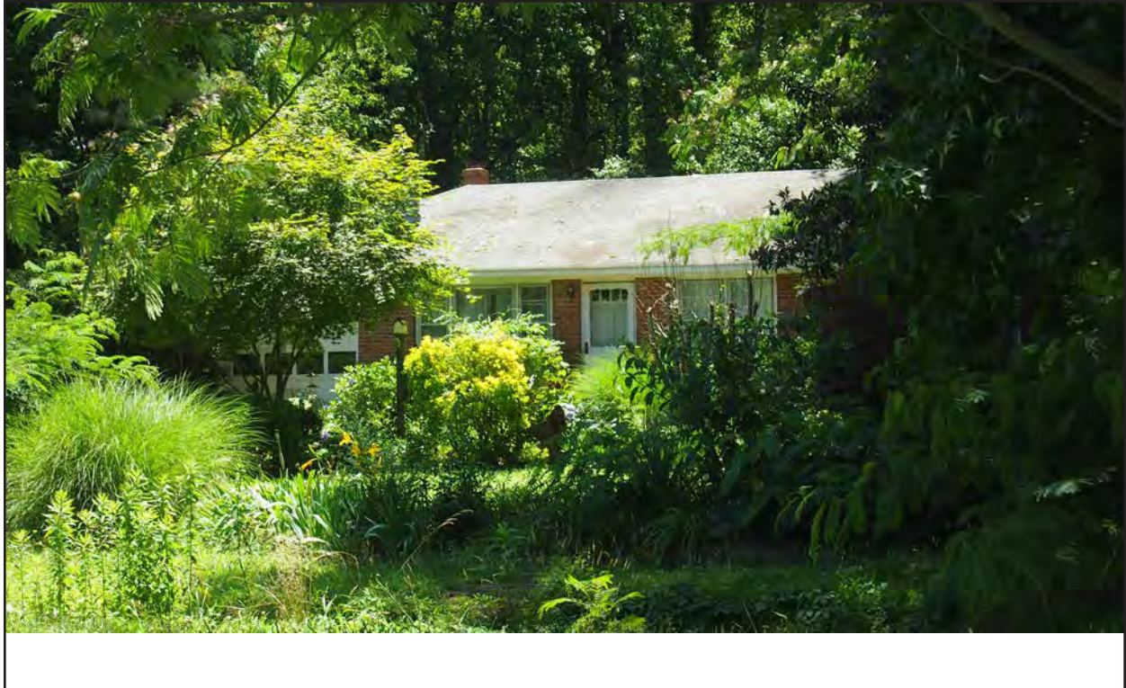
Figure 260. 134-5920, Ranch dwelling, north elevation, view to the south.
