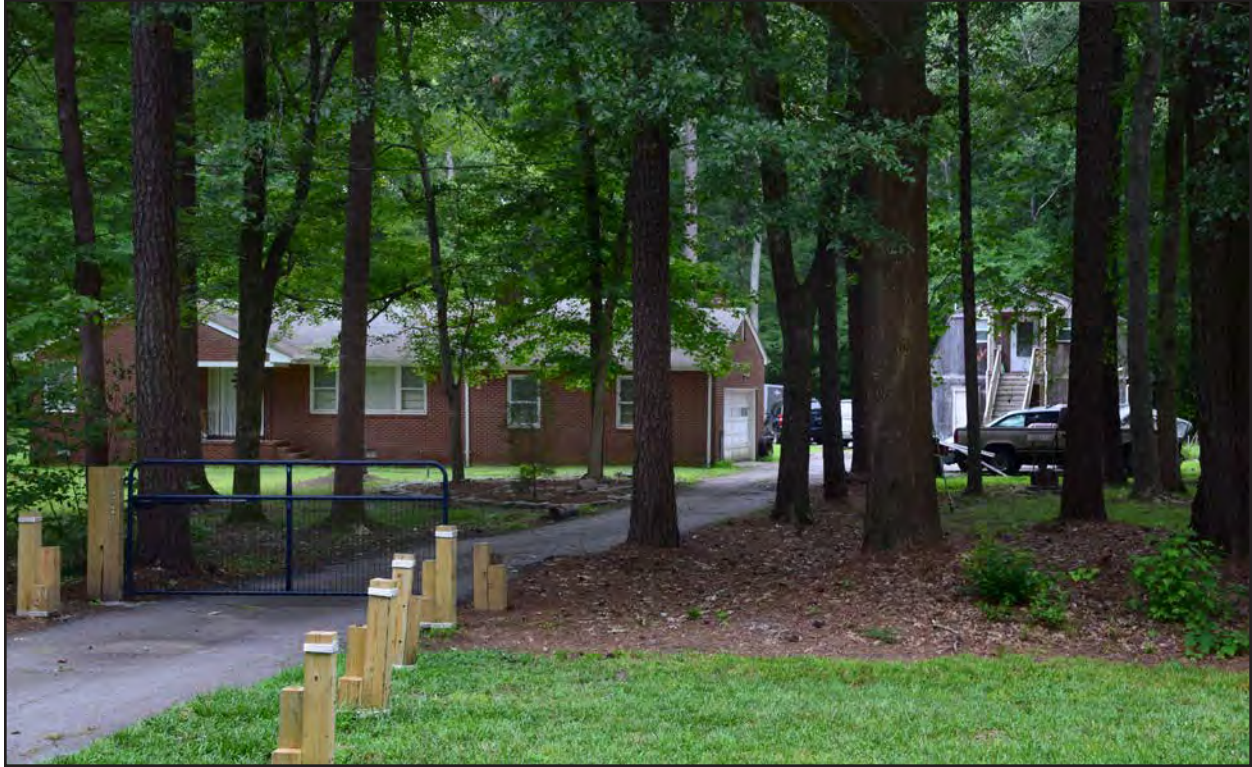
Figure 209. 134-5675, Ranch dwelling, east and north elevations, view to the southwest.
