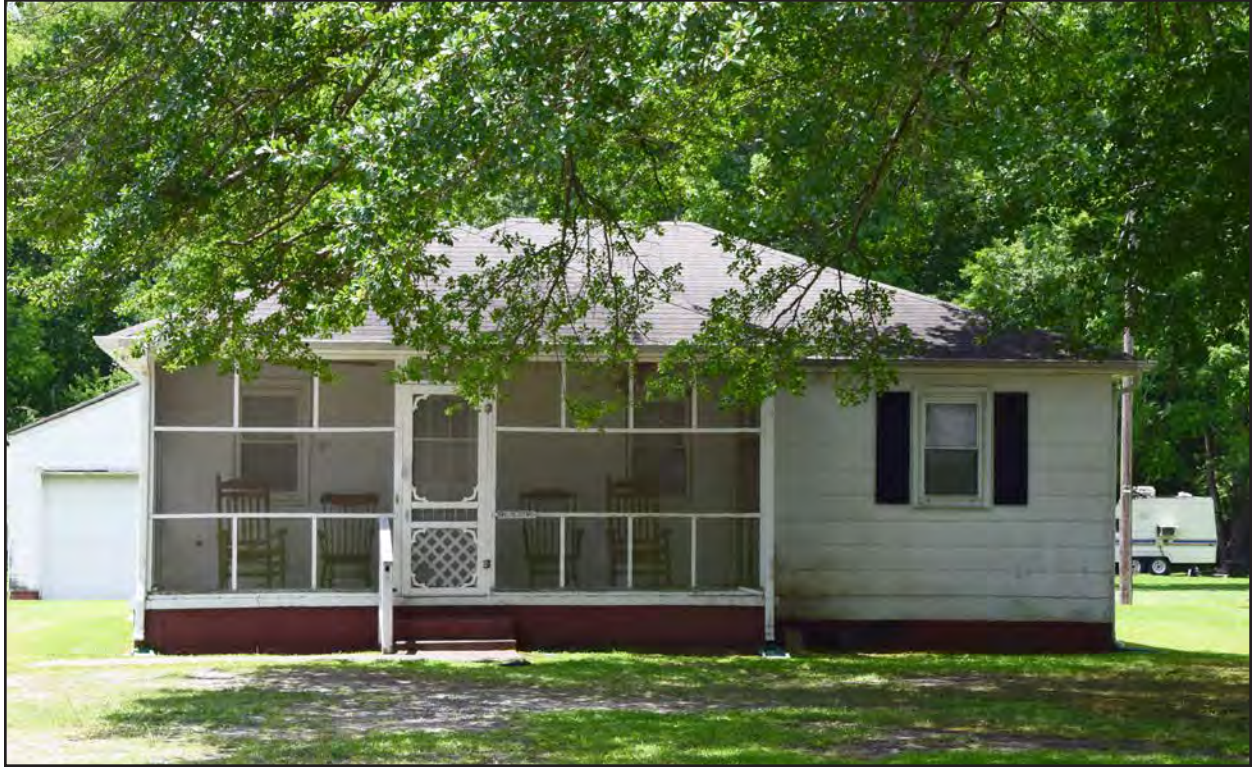
Figure 187. 134-5125, vernacular dwelling, east elevation, view to the west.
