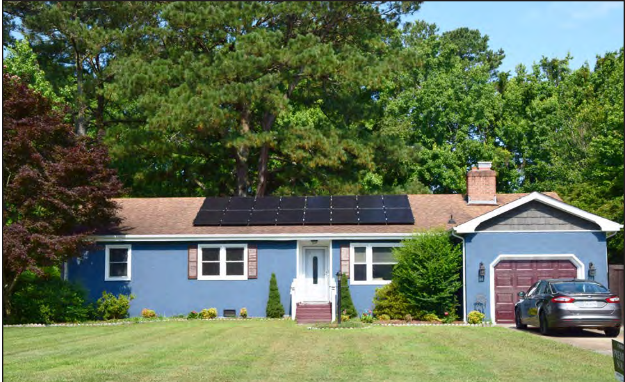
Figure 64. 131-6180, Ranch dwelling, east elevation, view to the west.
