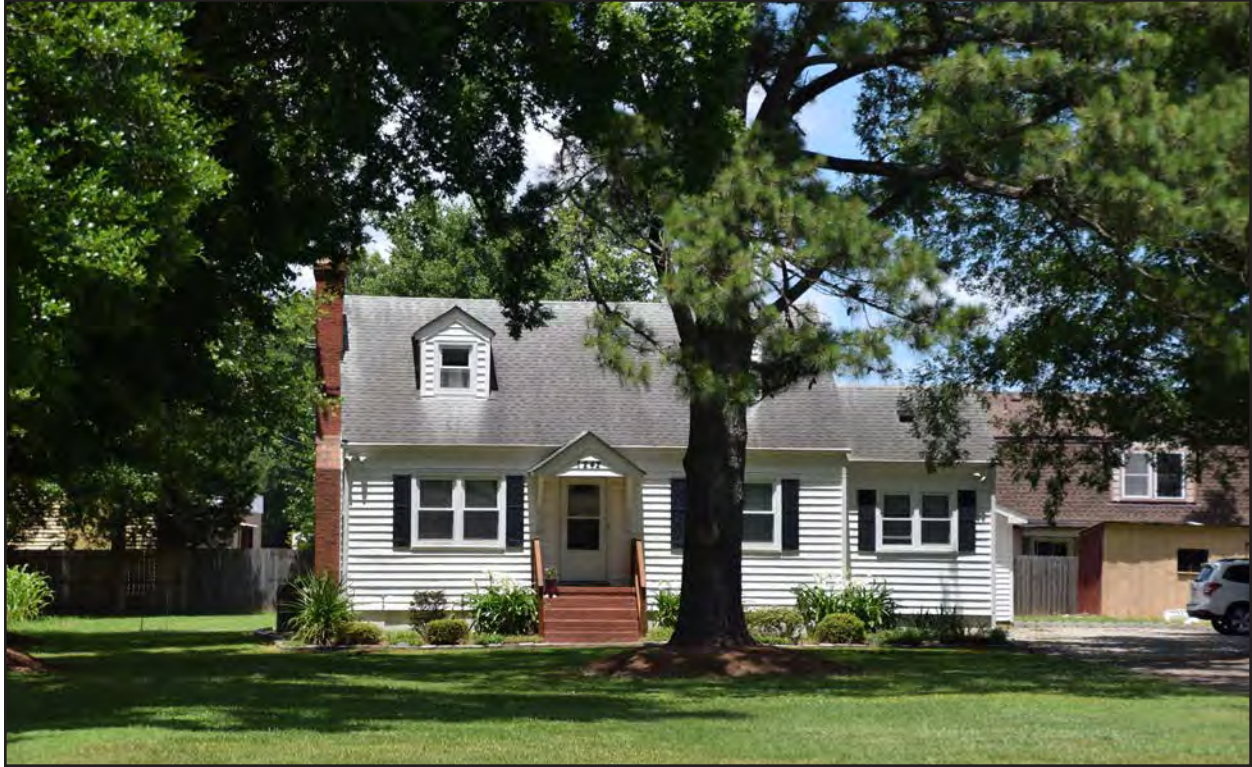
Figure 167. 134-0161, dwelling, south elevation, view to the north
