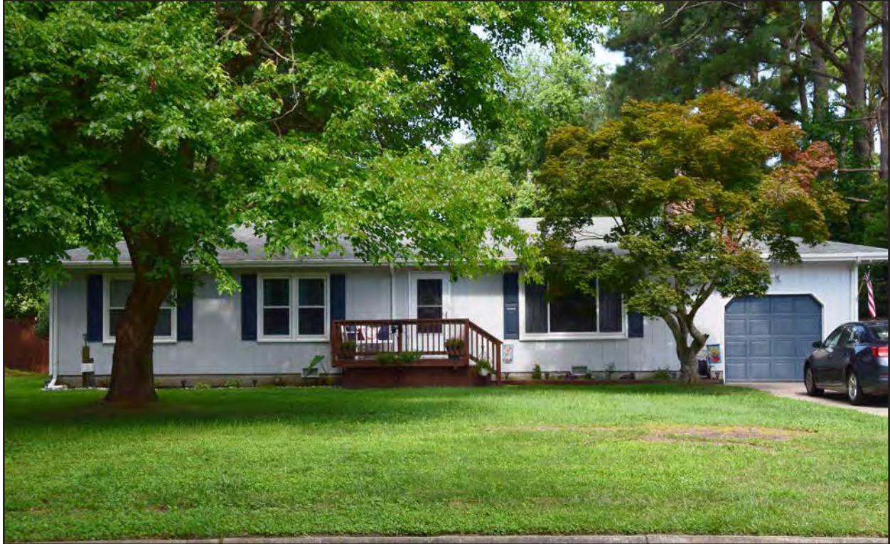
Figure 65. 131-6181, Ranch dwelling, east elevation, view to the west.
