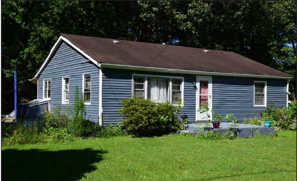
Figure 184. 134-5119, dwelling, northeast and southeast elevations, view to the west.
