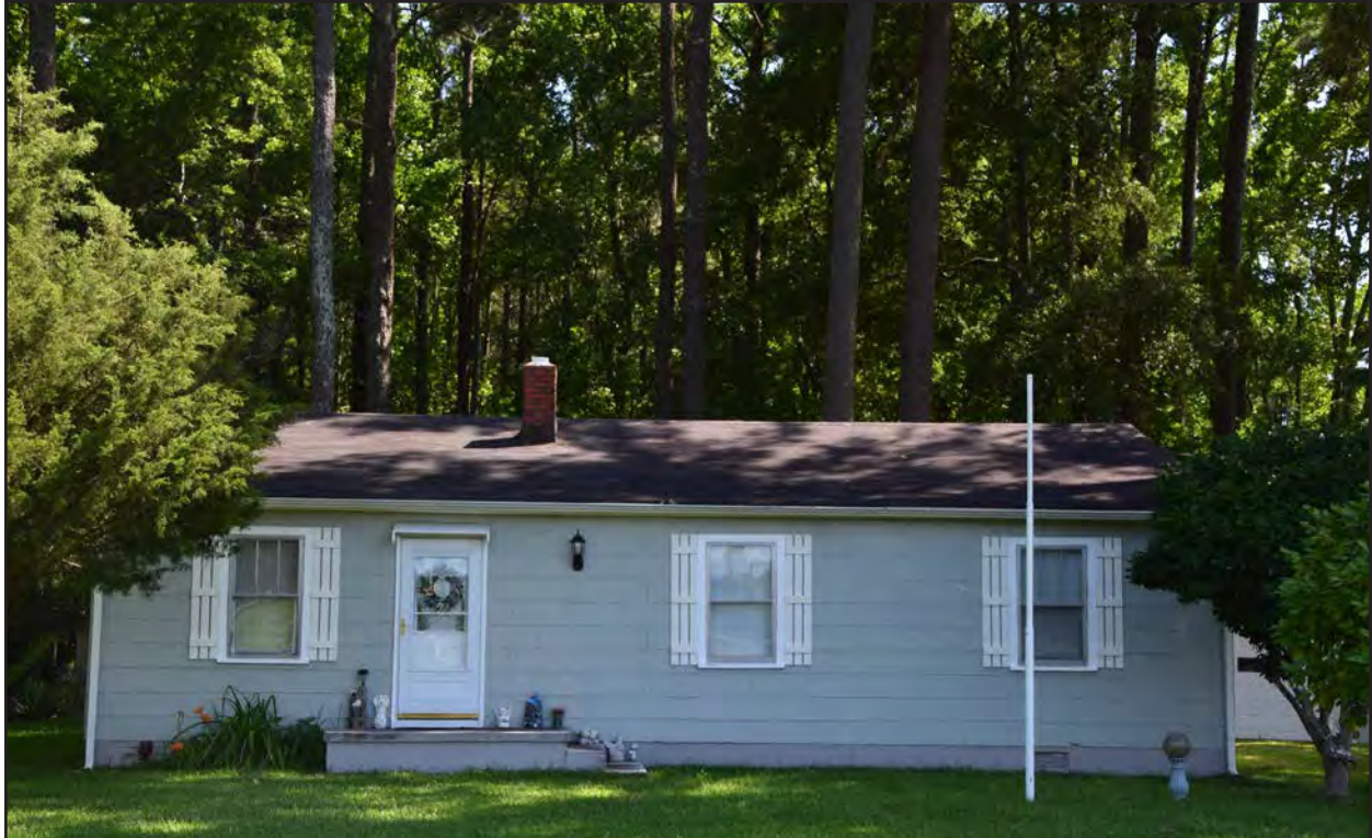
Figure 56. 131-6012, Ranch dwelling, west elevation, view to the east.
