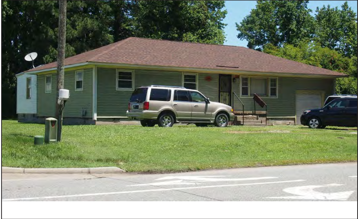
Figure 173. 134-0921, Yoko Wagner House, south and west elevations, view to the northeast.
