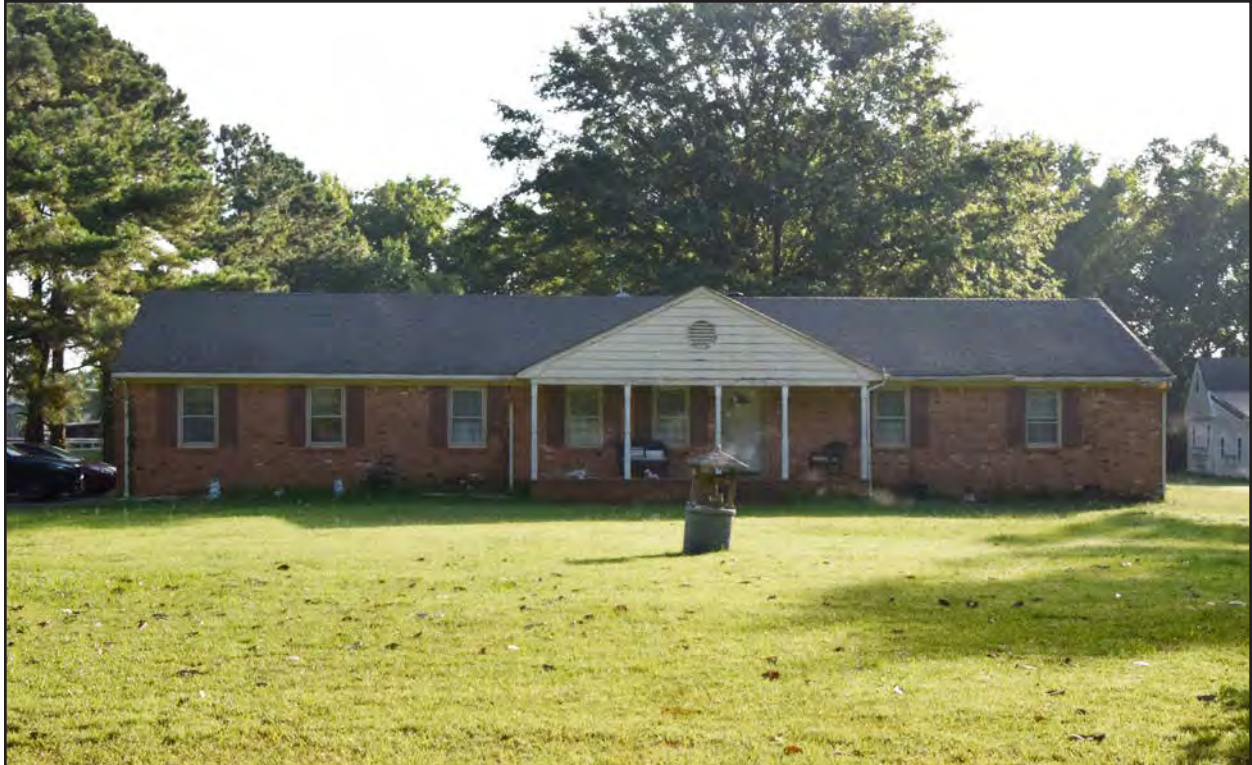
Figure 94. 131-6211, linear Ranch, southwest elevation, view to the northeast.
