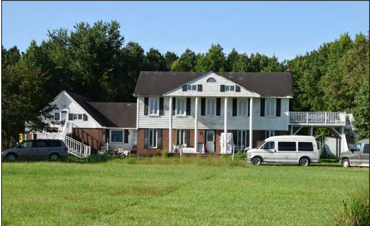
Figure 90. 131-6207, linear Ranch, north elevation, view to the south.
