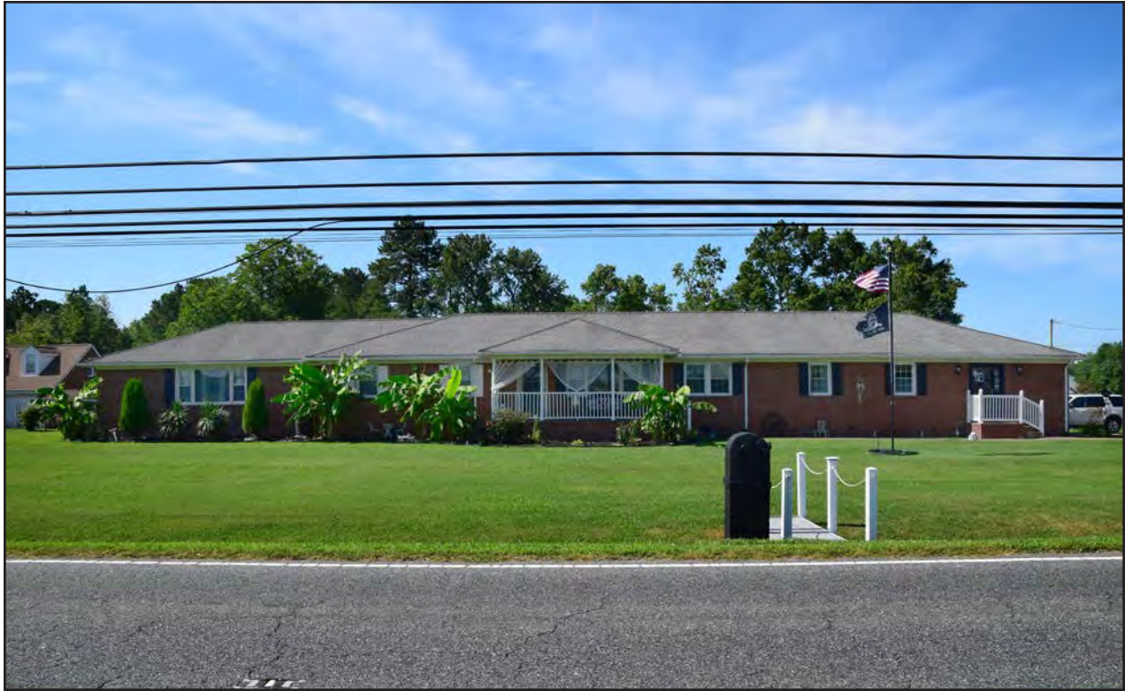
Figure 109. 131-6226, linear Ranch, north elevation, view to the south.
