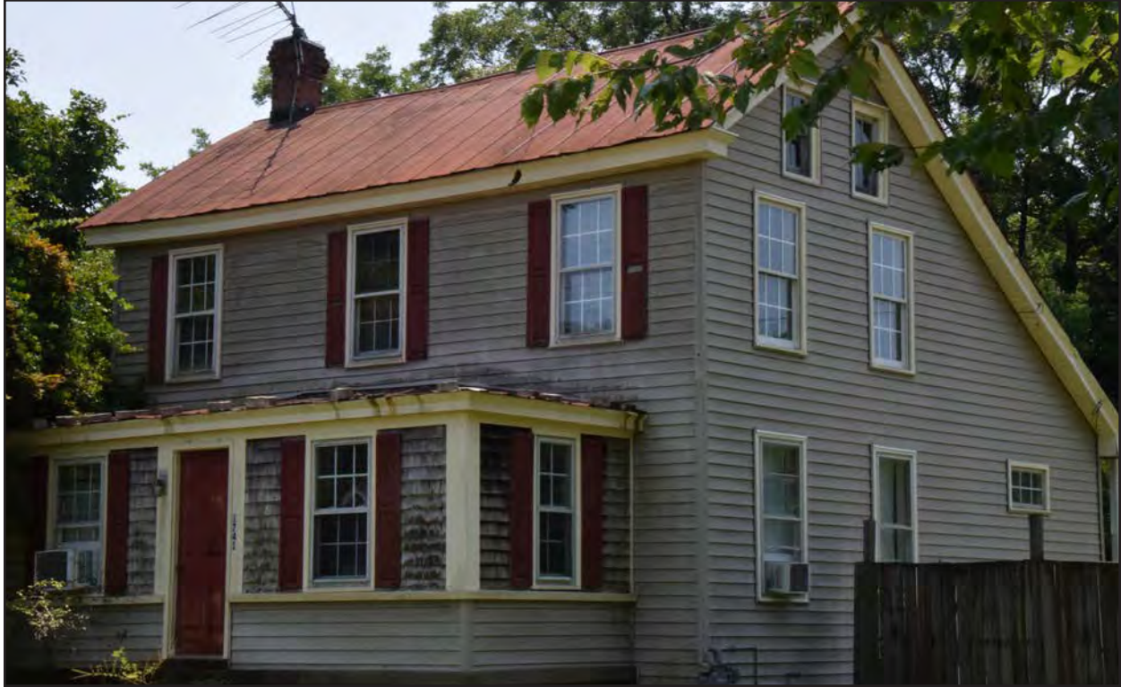
Figure 9: 131-0175, I-House, north and west elevations, view to the southeast.
