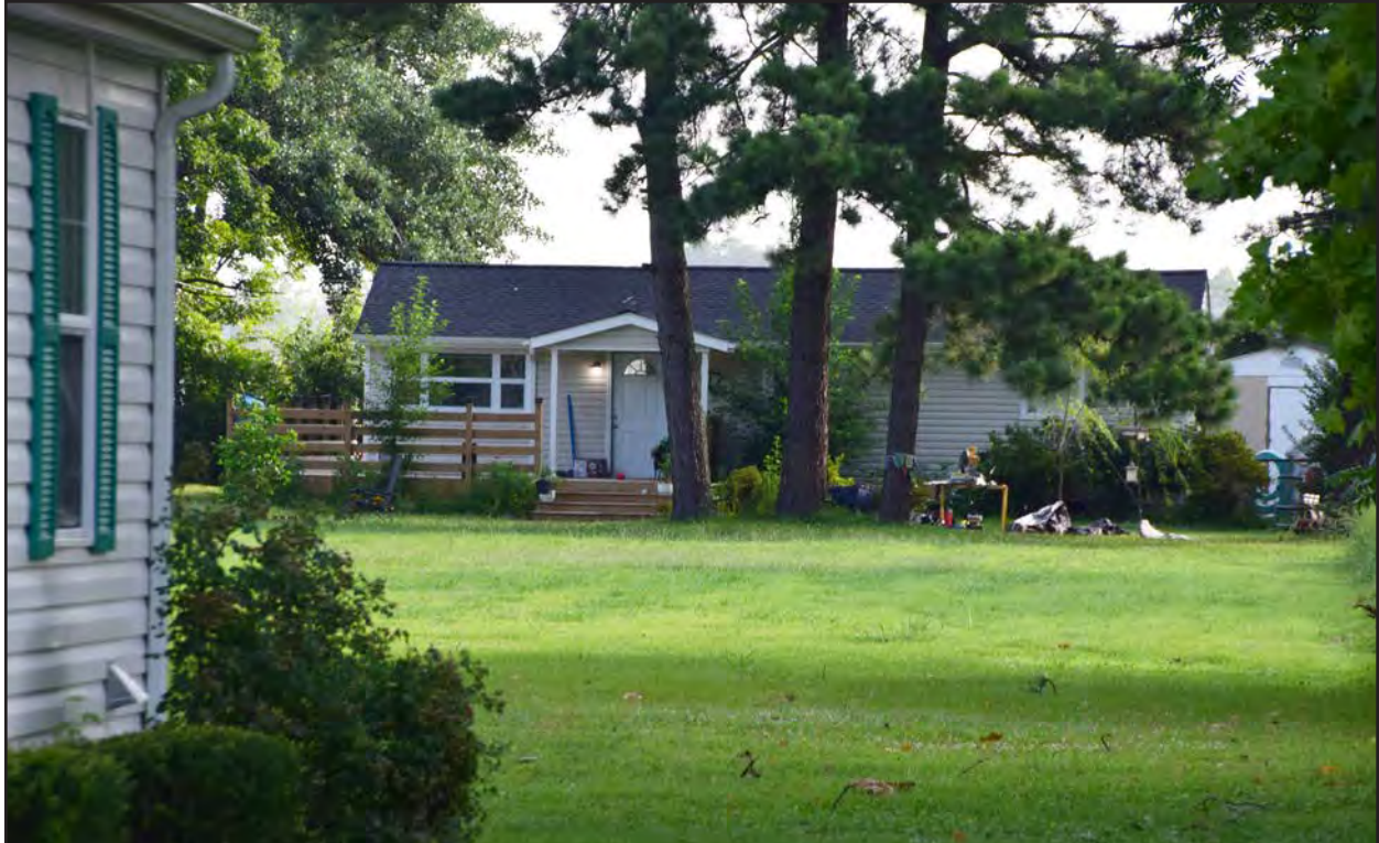
Figure 36. 131-5984, Ranch style dwelling, southwest elevation, view to the northeast.
