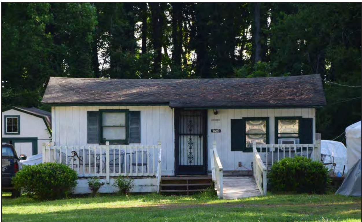
Figure 42. 131-5990, American Small House, southwest elevation, view to the northeast.
