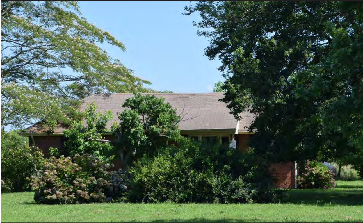
Figure 232. 134-5891, dwelling, south elevation, view to the north.
