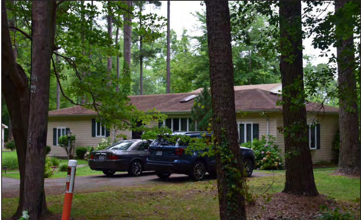
Figure 244. 134-5904, linear Ranch dwelling, west and south elevations, view to the northeast.
