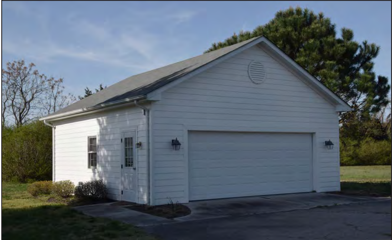
Figure 158. 134-0003, James Bell House, garage, north and east elevations, view to the southwest.
