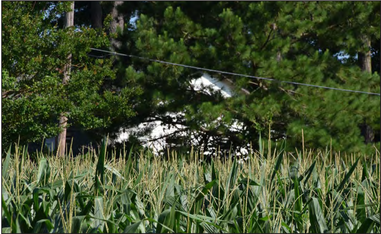
Figure 29. 131-5892, partially visible dwelling, south and east elevations, view to the northwest.
