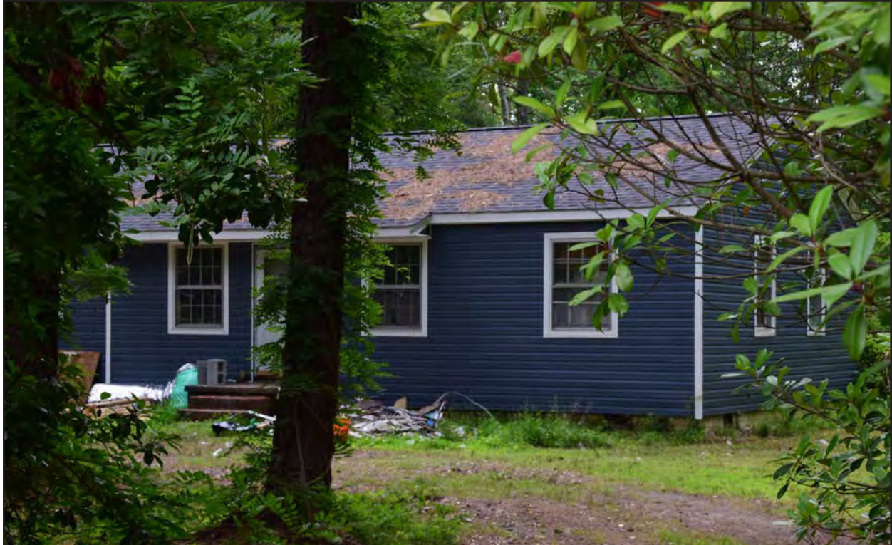
Figure 208. 134-5674, dwelling, west and south elevations, view to the northeast.
