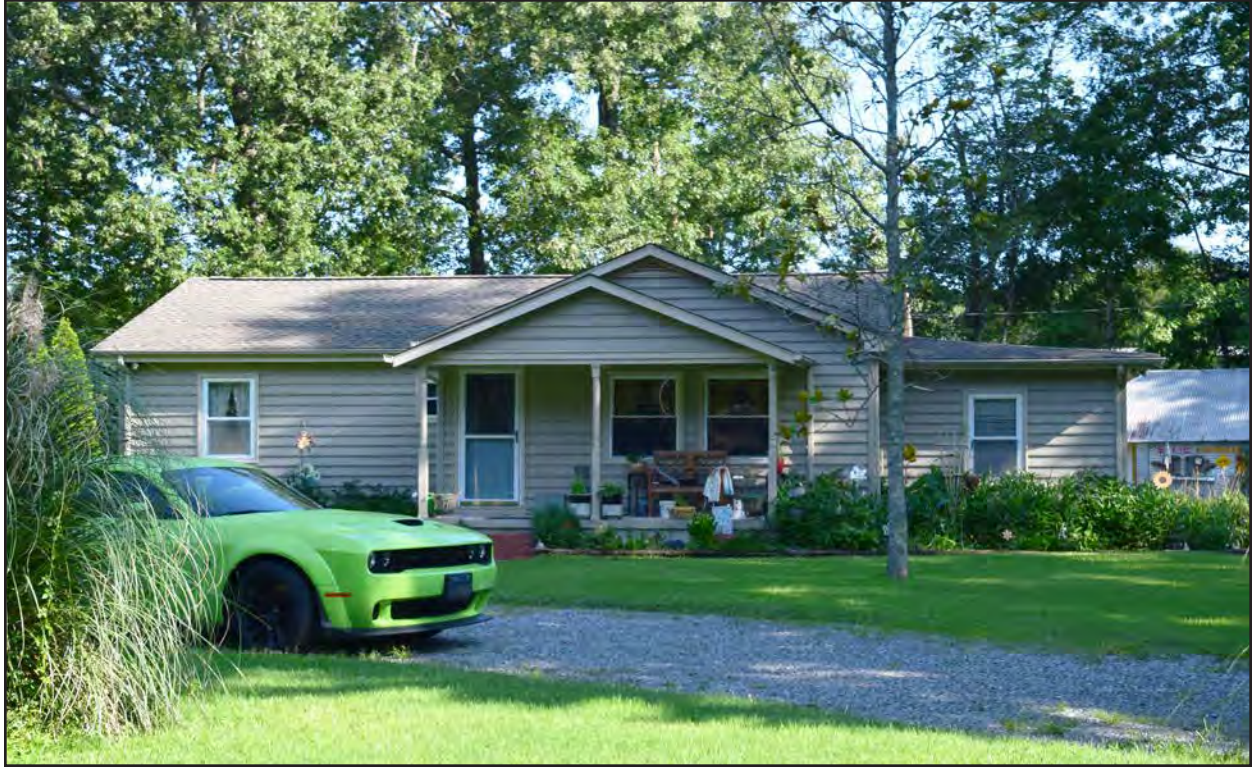
Figure 263. 134-5923, dwelling, south elevation.
