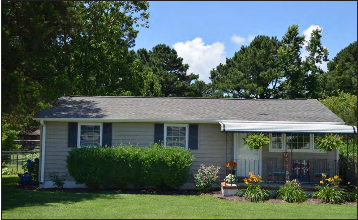
Figure 293. 134-5957, dwelling, northeast elevation.
