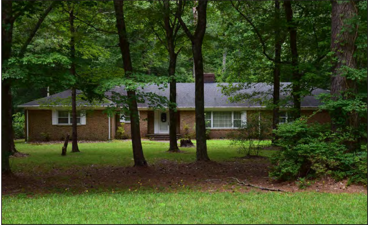
Figure 207. 134-5673, linear-with-clusters Ranch dwelling, east elevation, view to the west.
