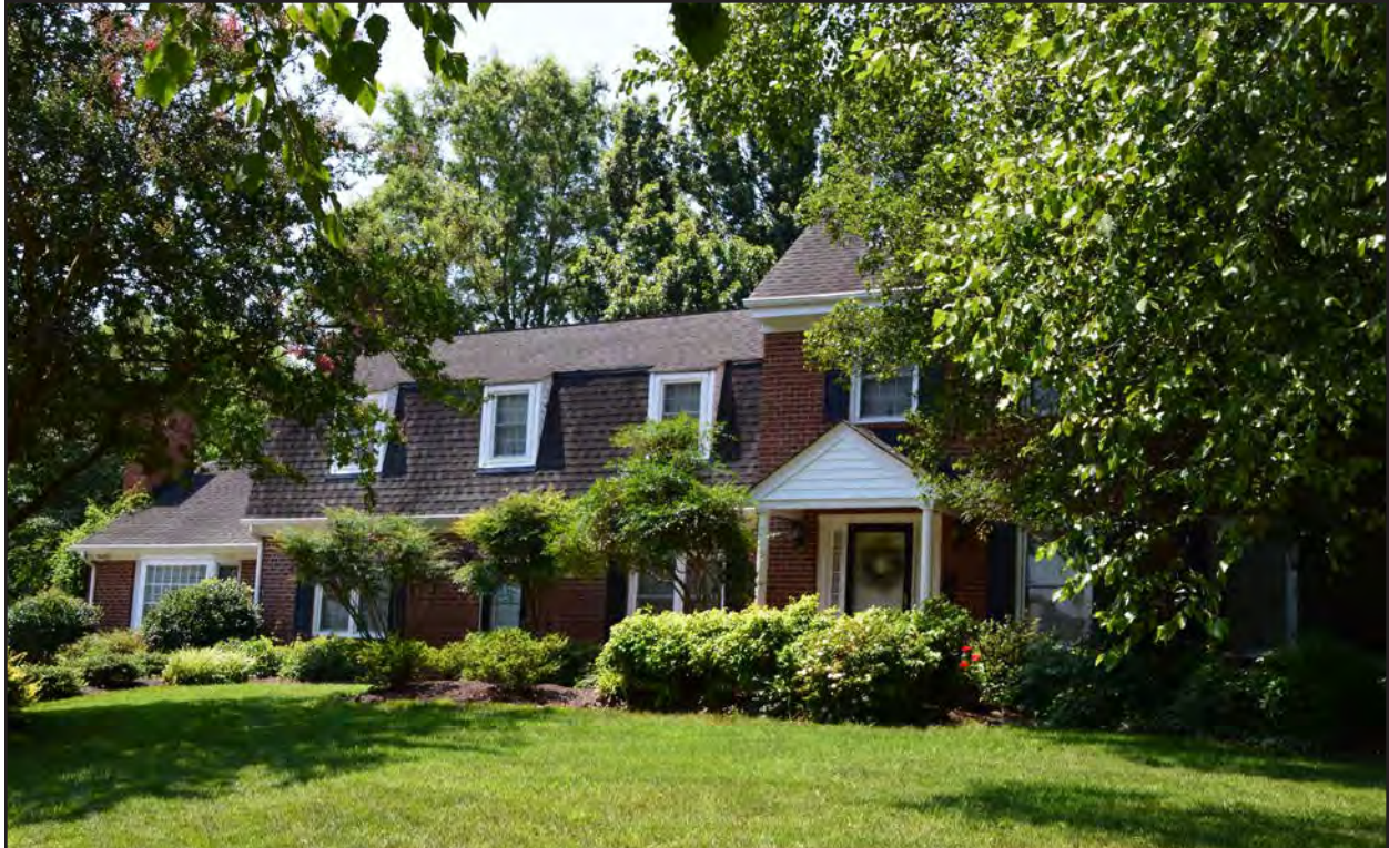
Figure 294. 134-5958, dwelling, northeast elevation.
