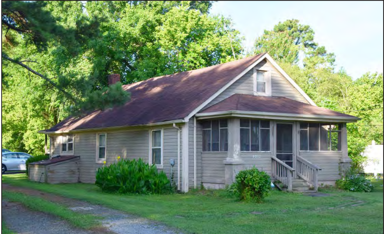
Figure 48. 131-5996, Craftsman dwelling, northeast and southeast elevations, view to the west.
