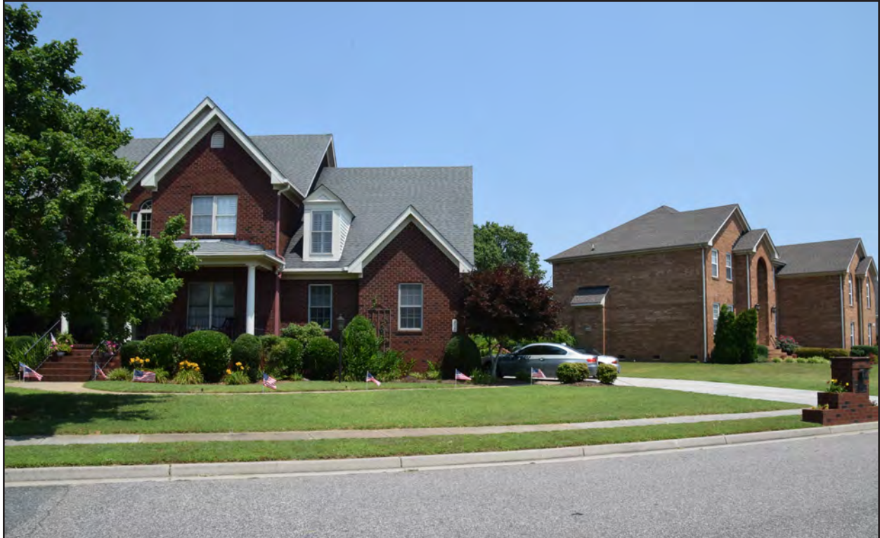
Figure 8. 131-0170, farmhouse, replacement dwelling, view to the north.
