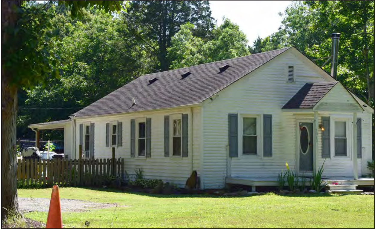
Figure 271. 134-5932, dwelling, southwest elevation, view to the northeast.
