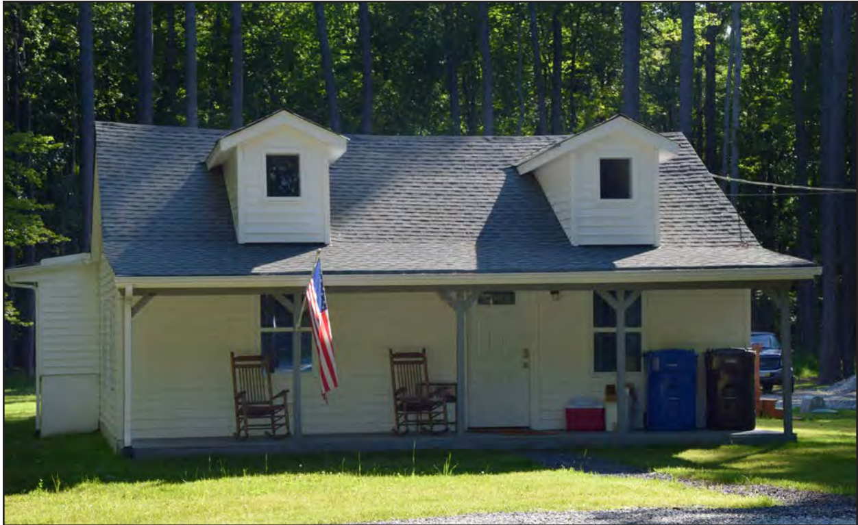
Figure 269. 134-5929, dwelling, southwest elevation, view to the northeast.
