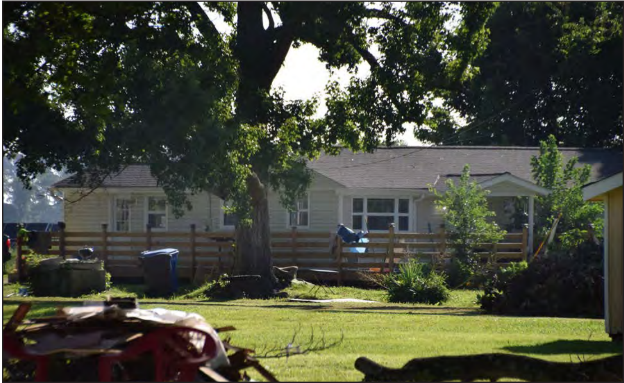
Figure 135. 131-6254, dwelling, southwest and northwest elevations, view to the east.
