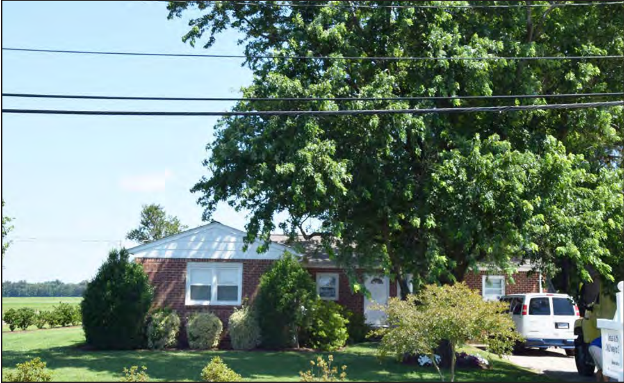
Figure 231. 134-5890, dwelling, south elevation, view to the north.
