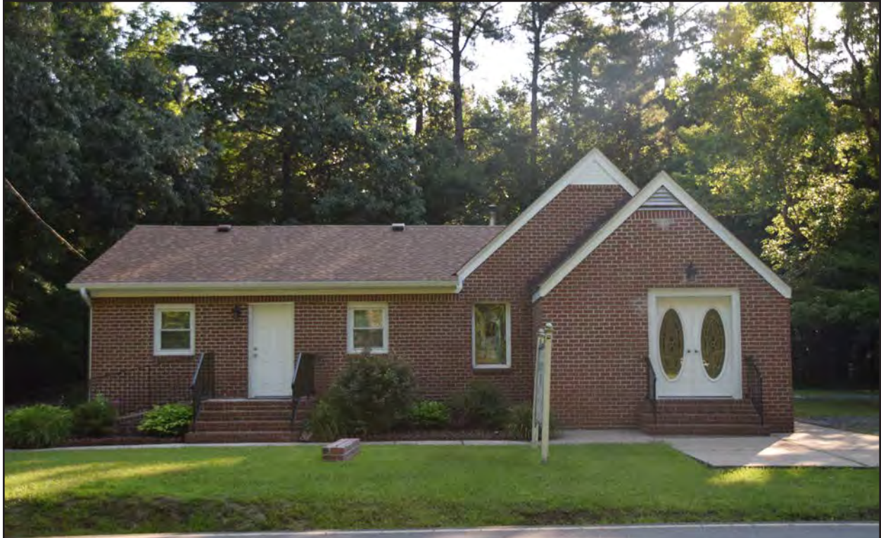
Figure 216. 134-5848, Campbell's Chapel AME Church, southwest elevation, view to the northeast.
