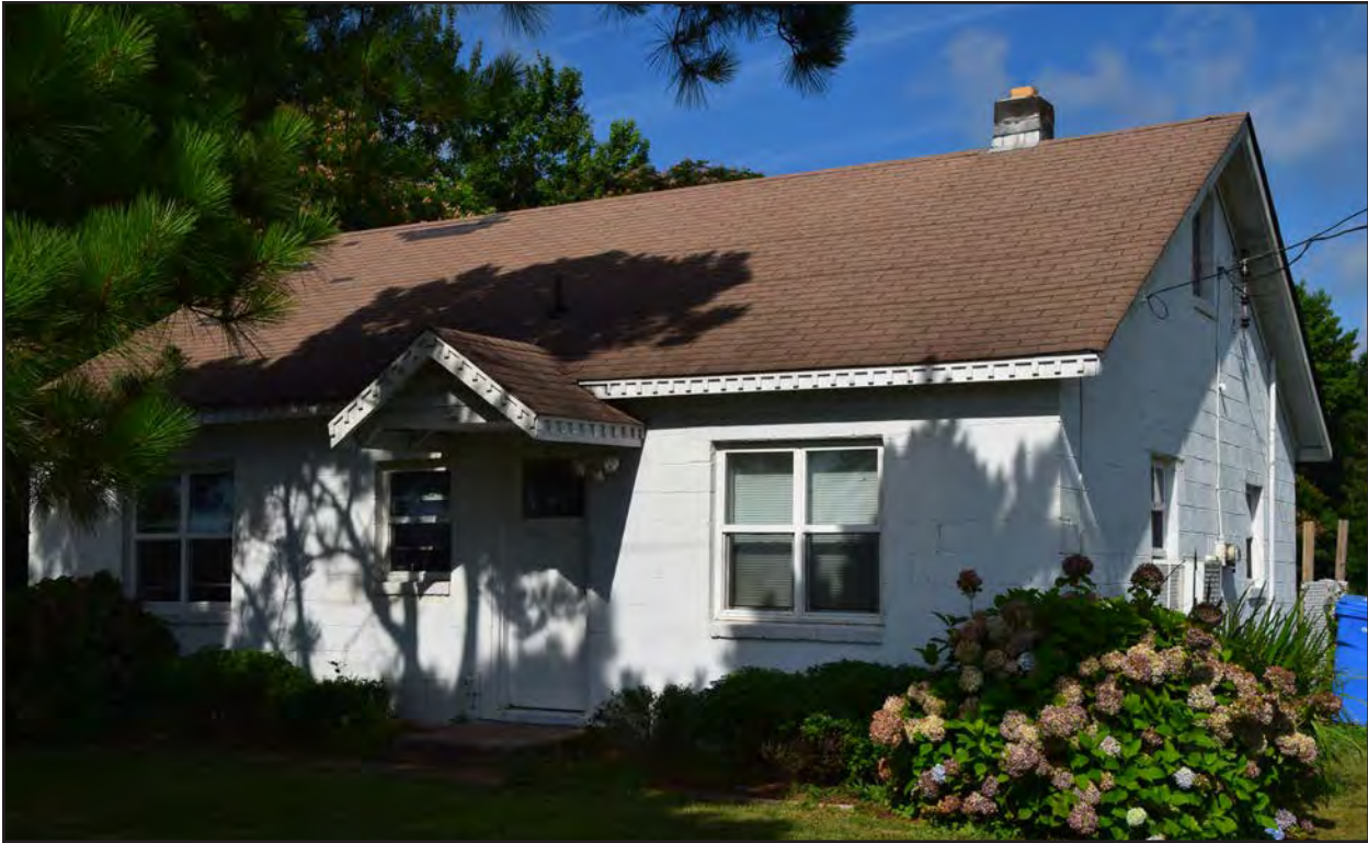
Figure 25. 131-5887, worker house, north and east elevations, view to the southwest.
