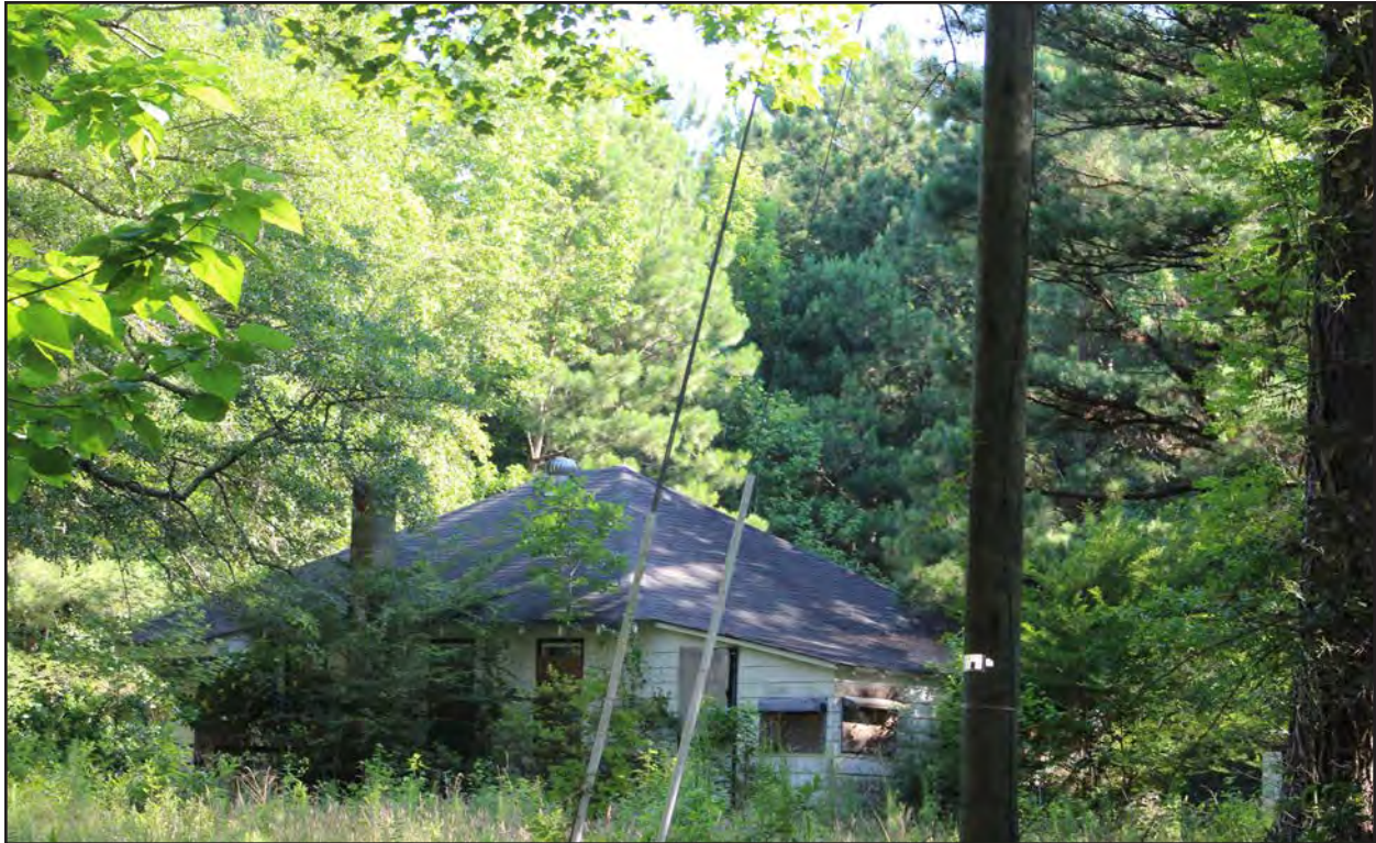
Figure 185. 134-5121, Craftsman dwelling, southwest elevation, view to the northeast.
