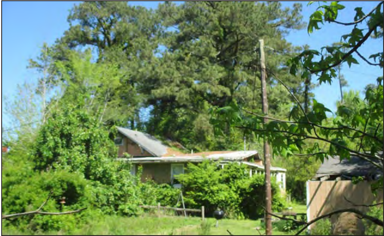
Figure 213. 134-5679, Craftsman dwelling, south and east elevations, view to the northeast
