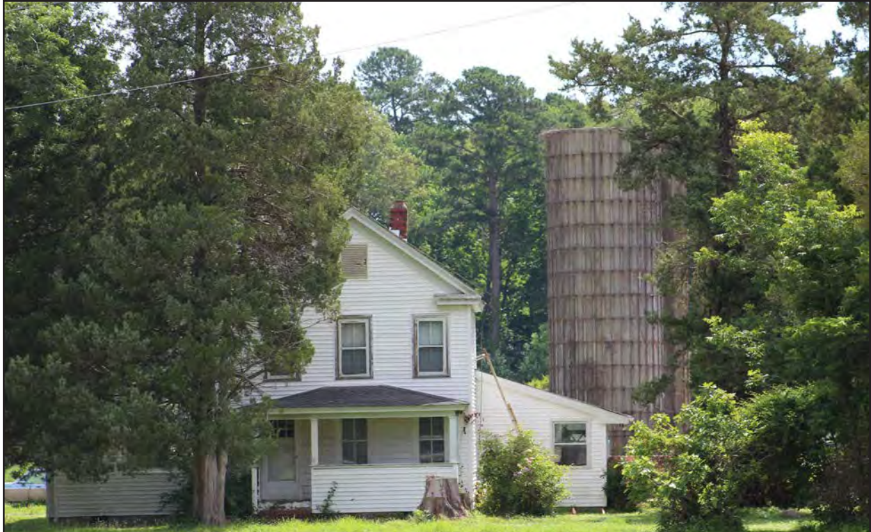
Figure 164. 134-0106, farmhouse, north elevation, view to the south.
