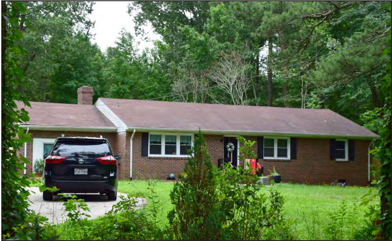
Figure 215. 134-5680, Ranch dwelling, west elevation, view to the east. 134
