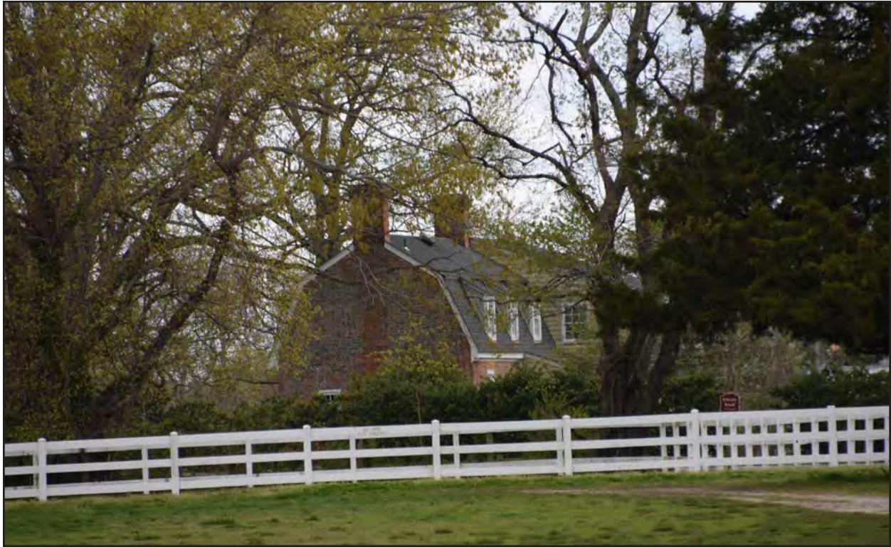
Figure 159. 134-0038, Jonathan Woodhouse House, southwest and southeast elevations, view to the north-northeast.
