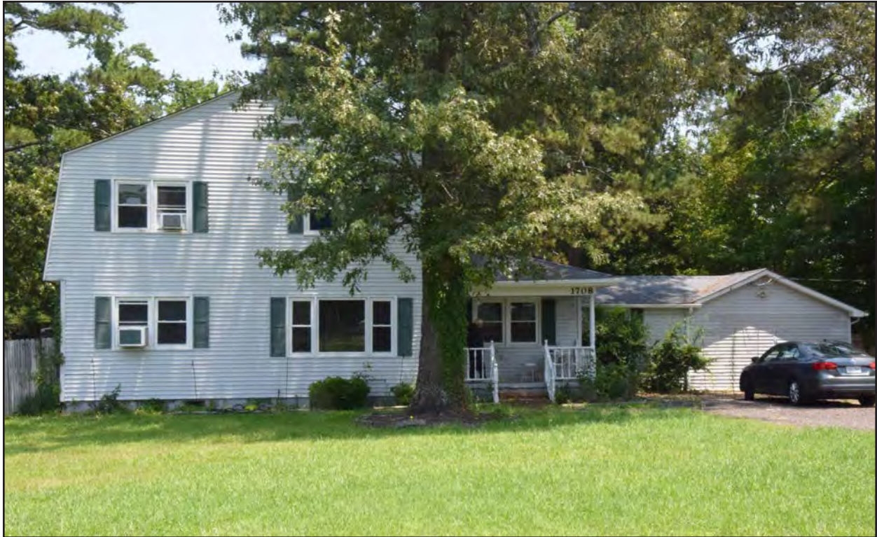
Figure 113. 131-6230, dwelling, south elevation.
