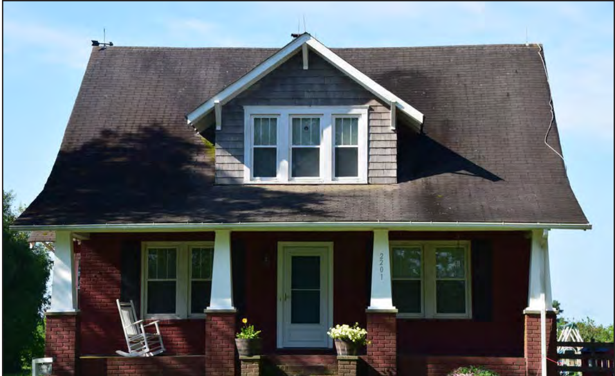
Figure 18. 131-5435, Mount Pleasant Farms, Craftsman Bungalow, northeast elevation, view to the southwest.
