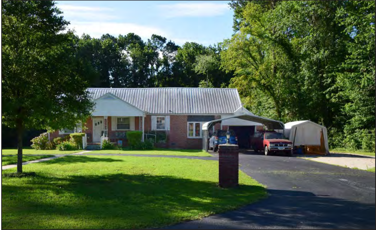
Figure 259. 134-5919, dwelling, northwest elevation.
