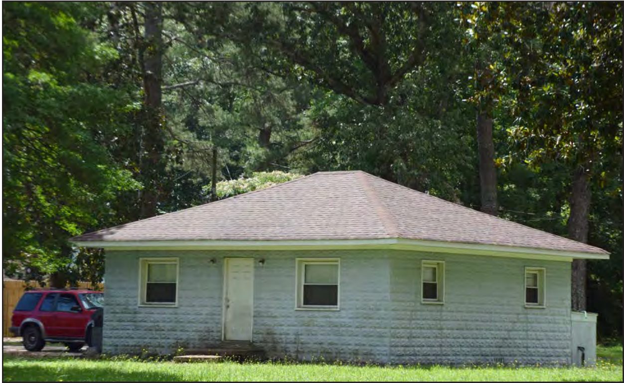
Figure 253. 134-5913, bungalow Ranch, north elevation, view to the south.
