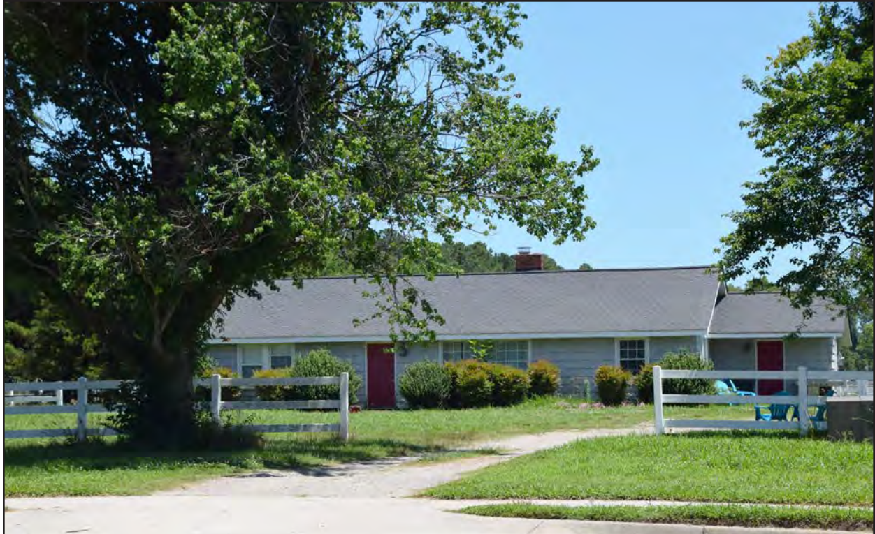
Figure 280. 134-5944, dwelling, southwest elevation, view to the northwest.
