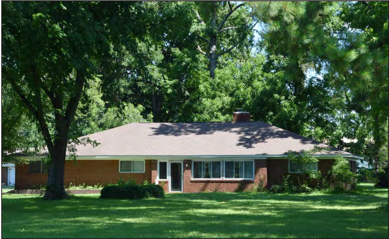
Figure 233. 134-5892, dwelling, south elevation, view to the north.
