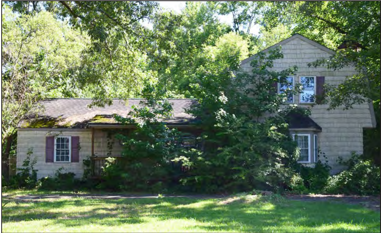
Figure 273. 134-5934, dwelling, southwest elevation, view to the northeast.
