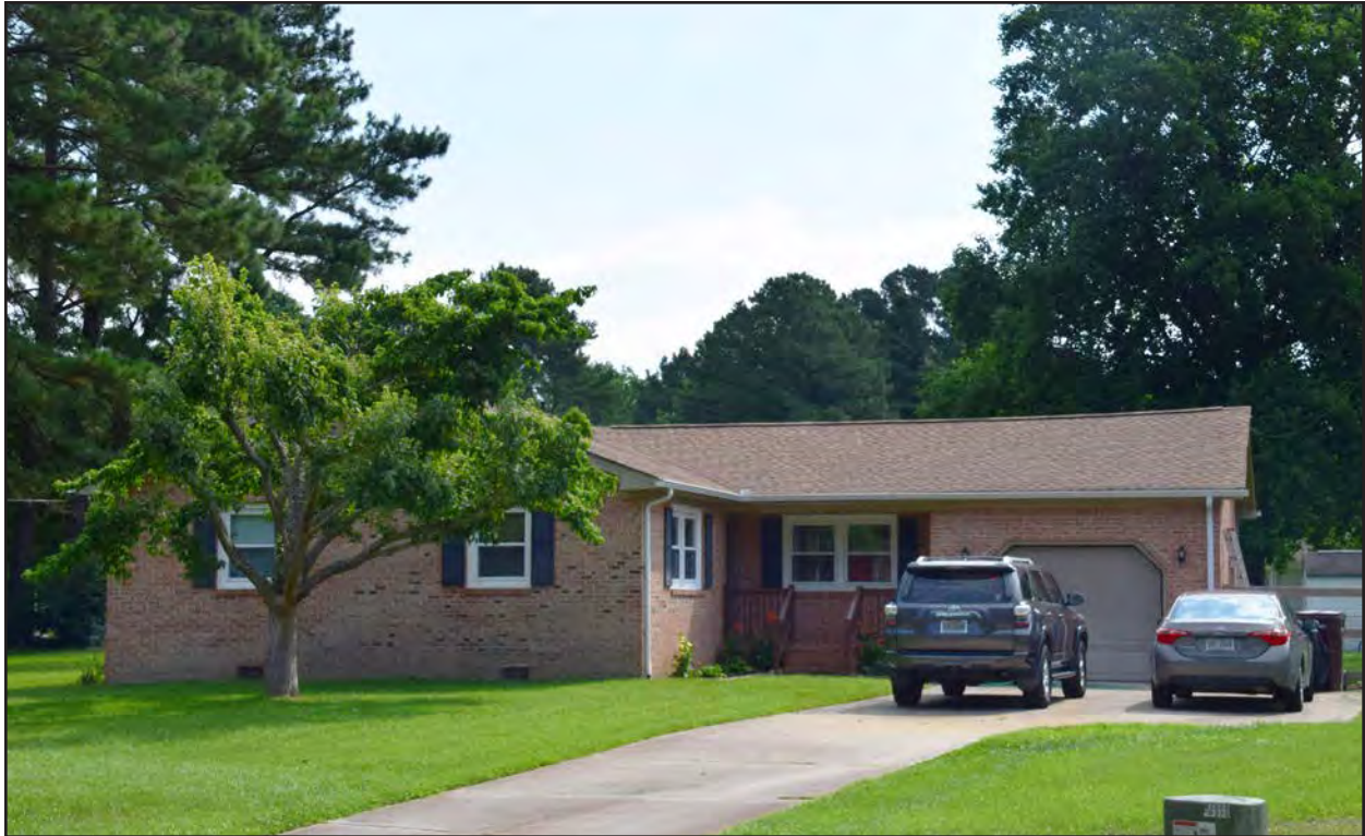
Figure 67: 131-6183, Ranch dwelling, southwest elevation, view to the northeast.
