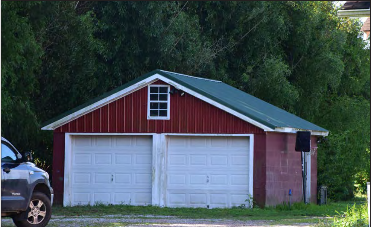
Figure 20. 131-5435, Mount Pleasant Farms, garage, northeast and northwest elevations, view to the
