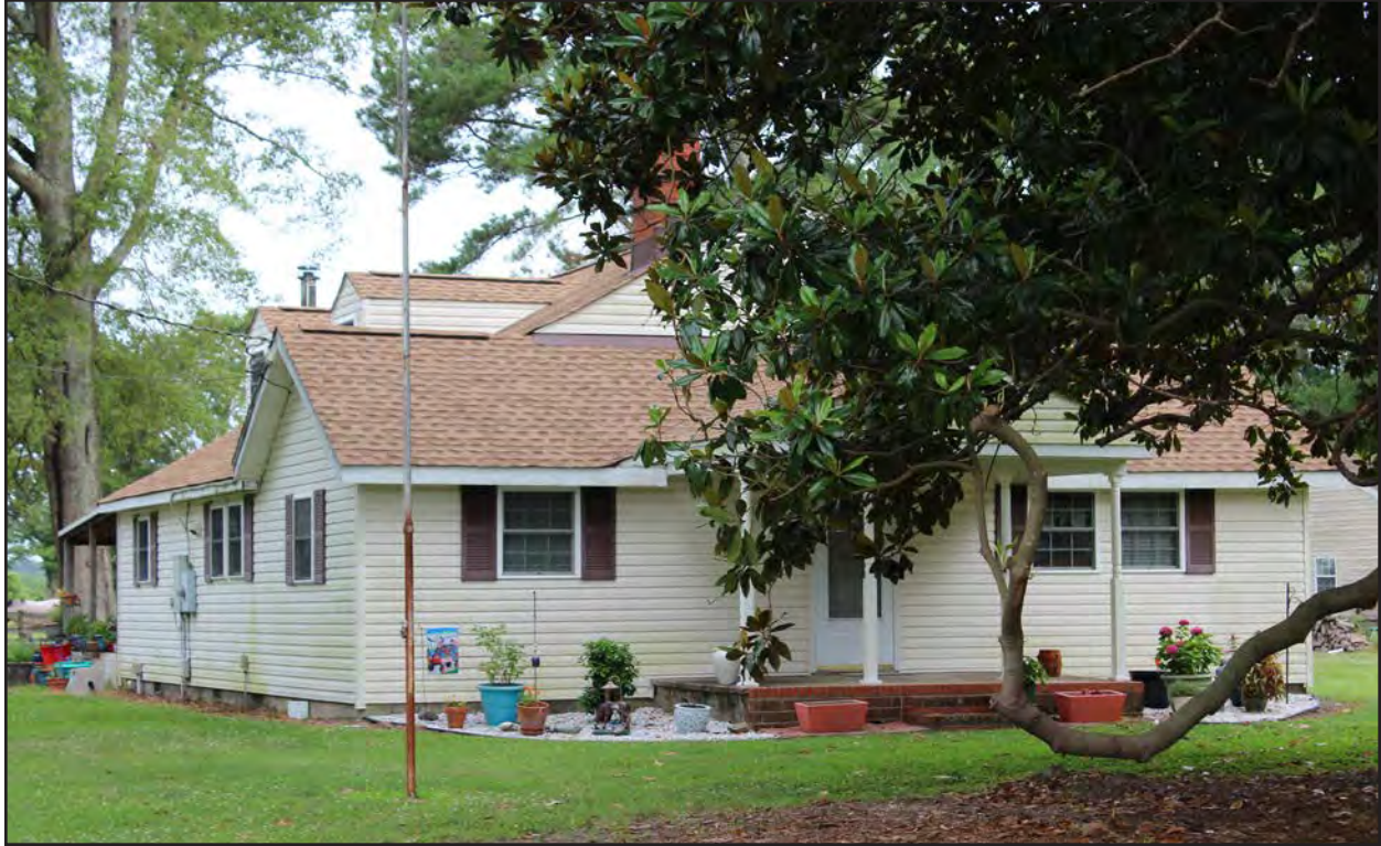
Figure 105. 131-6222, vernacular dwelling, east and south elevations, view to the northwest.
