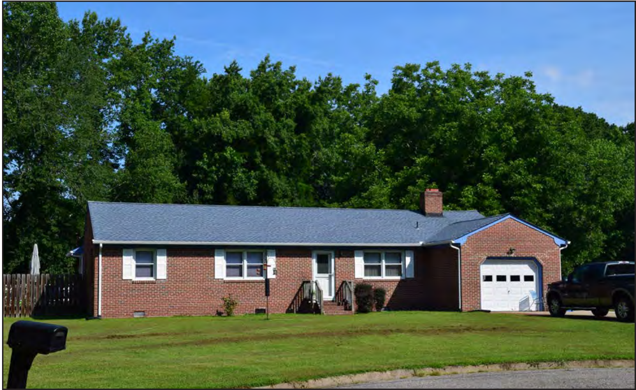
Figure 63. 131-6179, Ranch dwelling, southeast and southwest elevations, view to the north.
