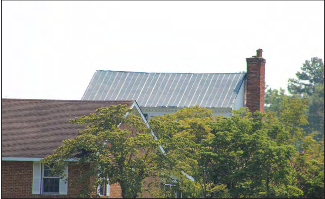
Figure 169. 134-0360, dwelling, west elevation, view to the east.
