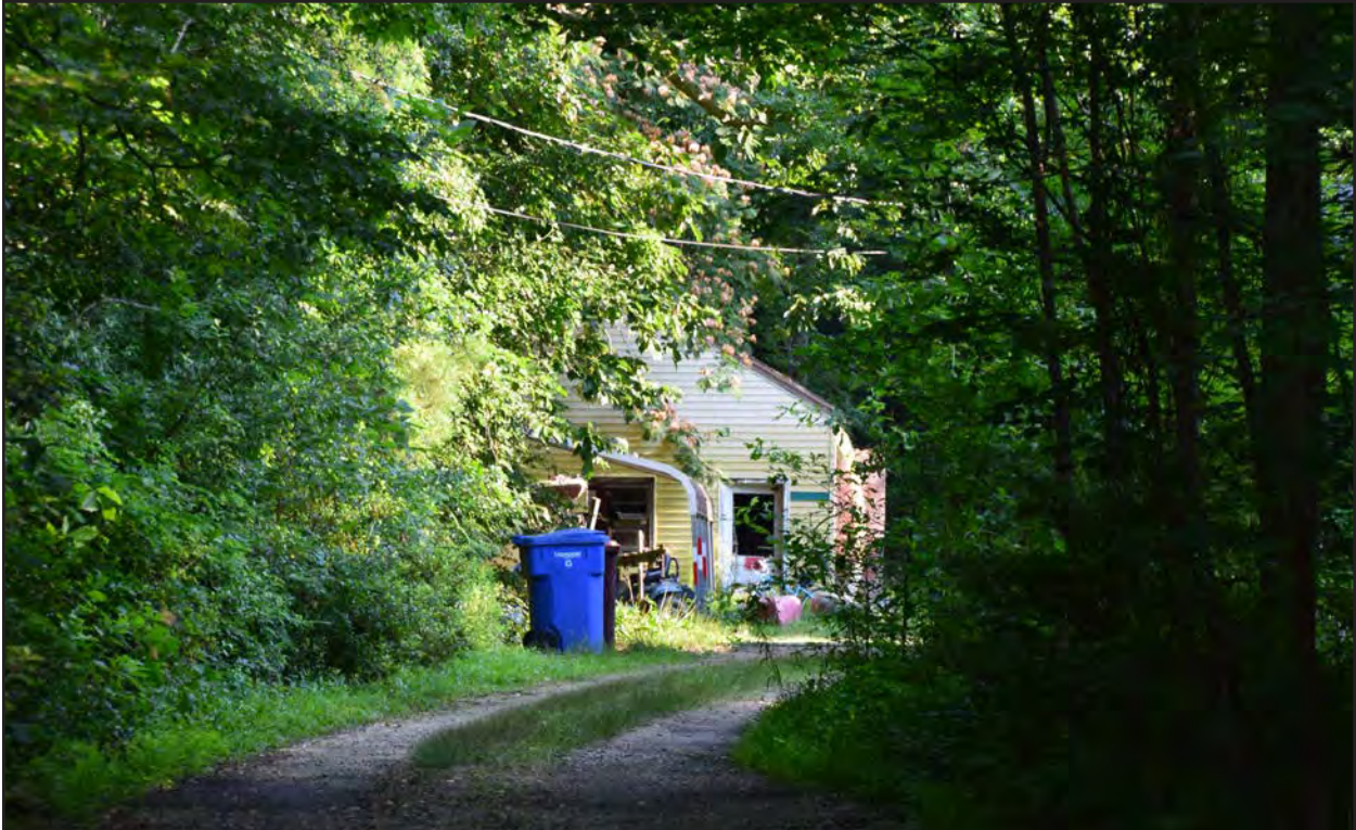
Figure 142. 131-6261, detached garage, south elevation, view to the north.
