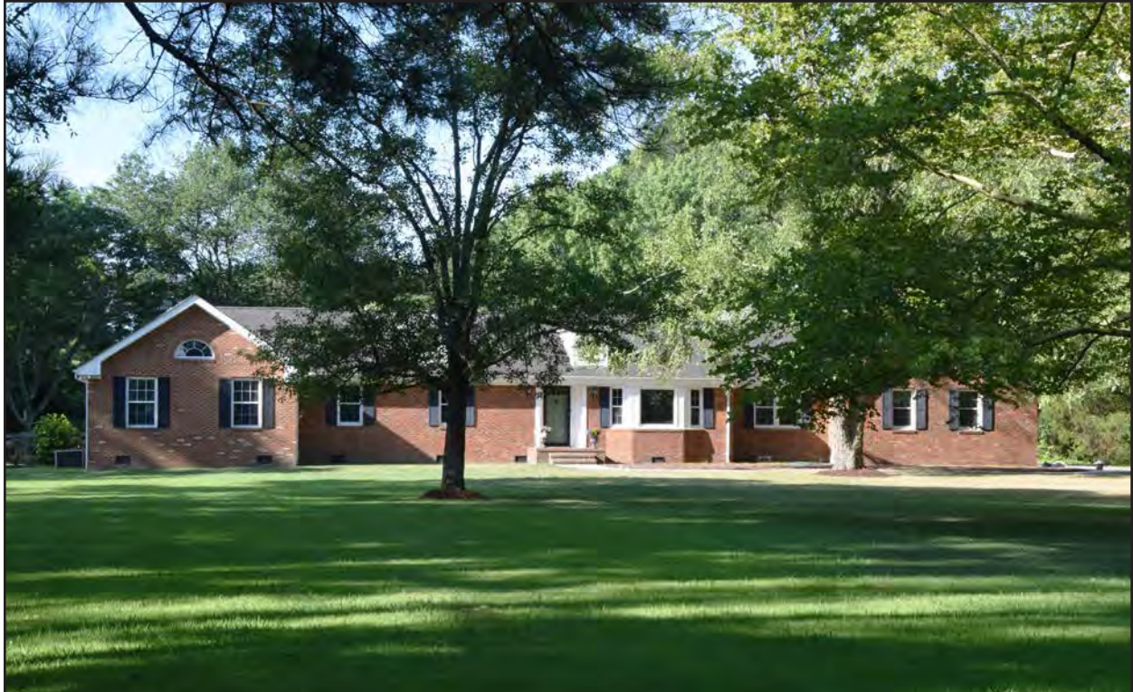
Figure 148. 131-6267, courtyard Ranch, north elevation, view to the south.
