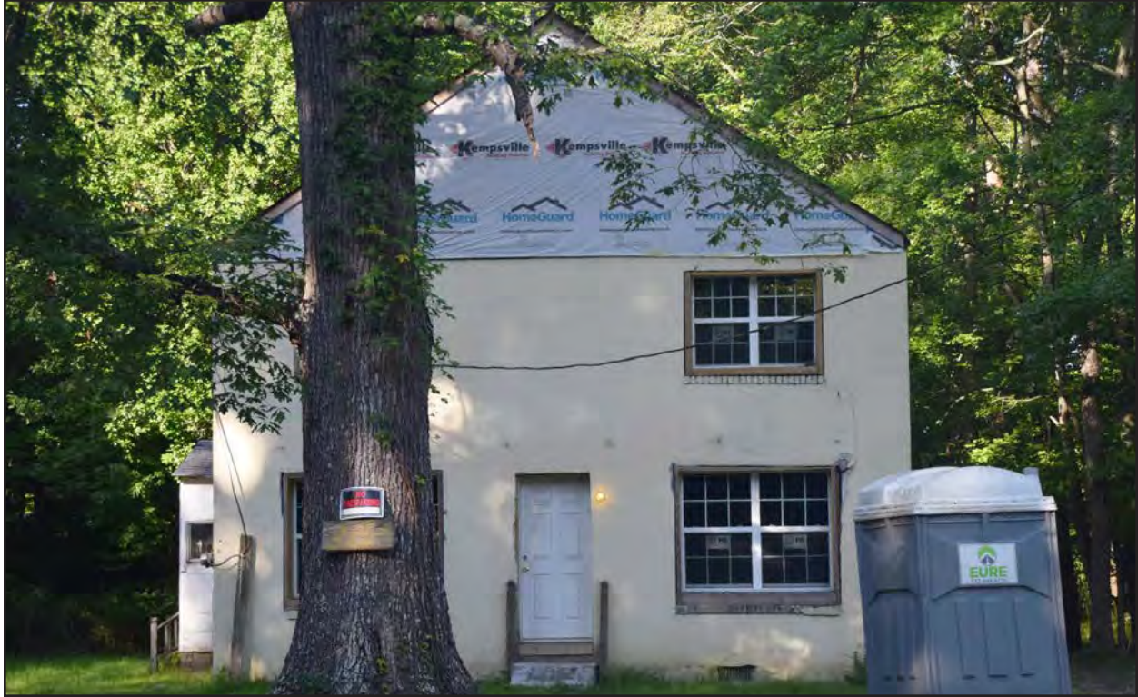
Figure 183. 134-5117, fraternal building, northeast elevation, view to the southwest.
