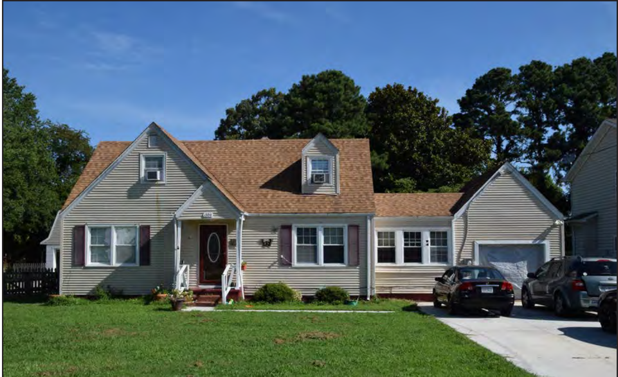
Figure 262. 134-5922, dwelling, south elevation.
