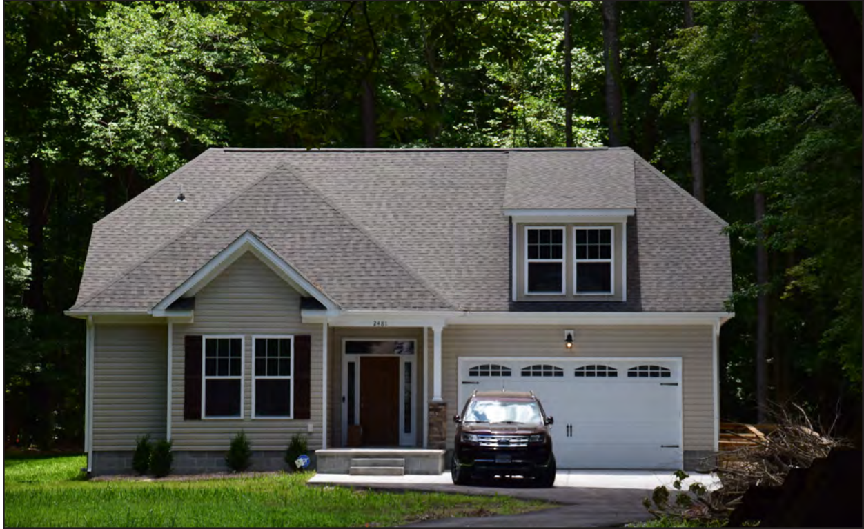
Figure 43. 134-5133, vernacular house, no longer extant, view to the southwest.
