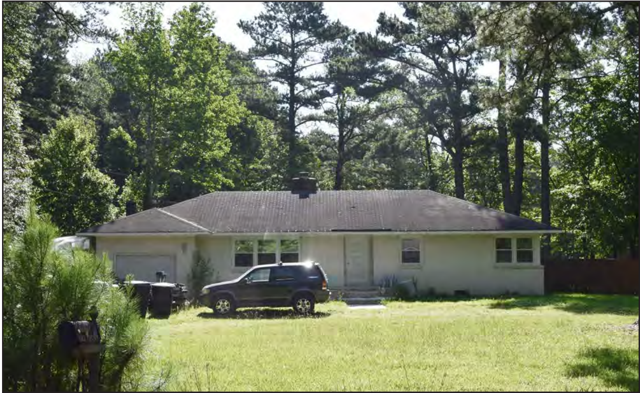
Figure 247. 134-5907, dwelling, west elevation, view to the east.
