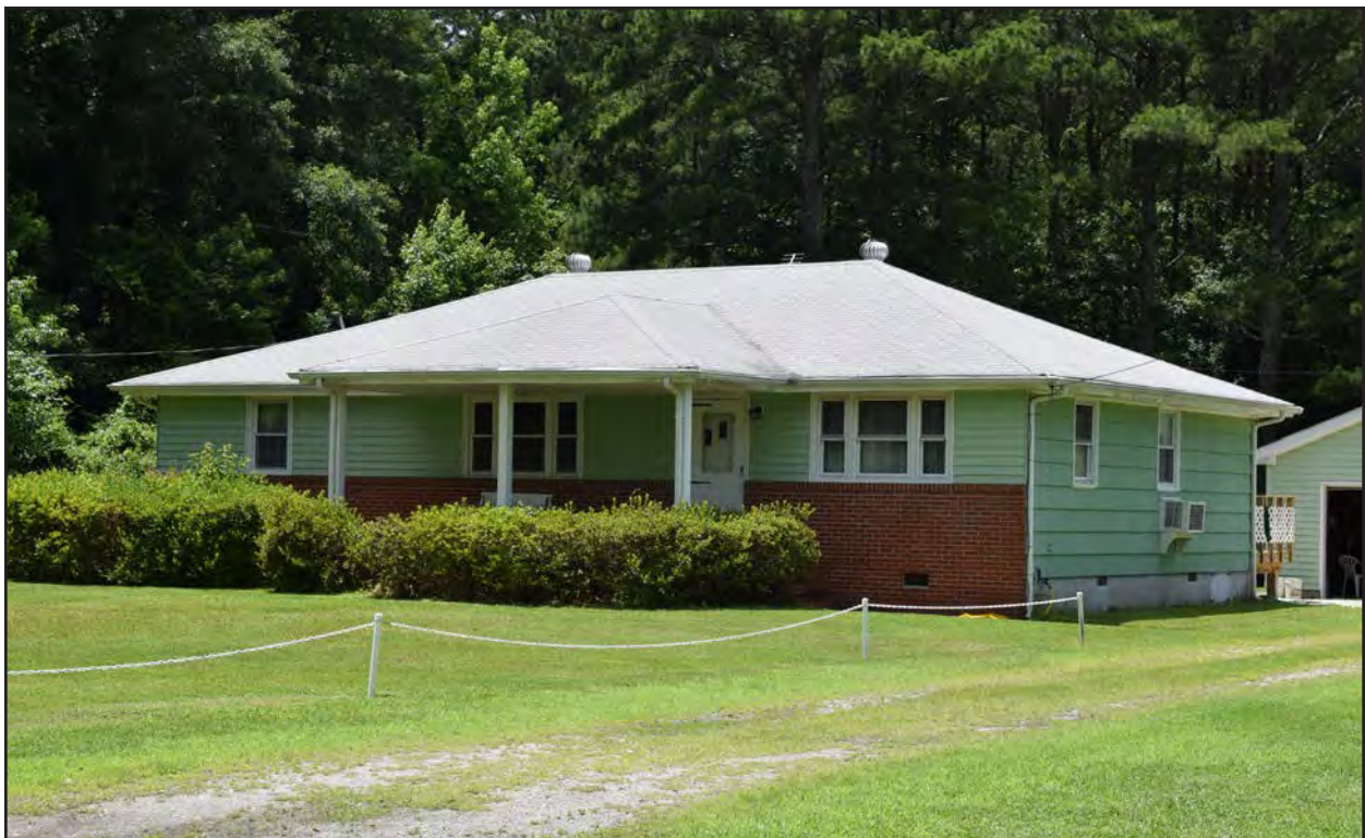
Figure 274. 134-5938, linear Ranch dwelling, east elevation, view to the west.
