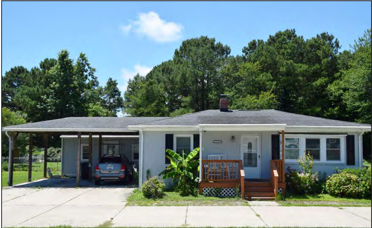
Figure 195. 134-5176, bungalow Ranch, northeast elevation, view to the southwest.
