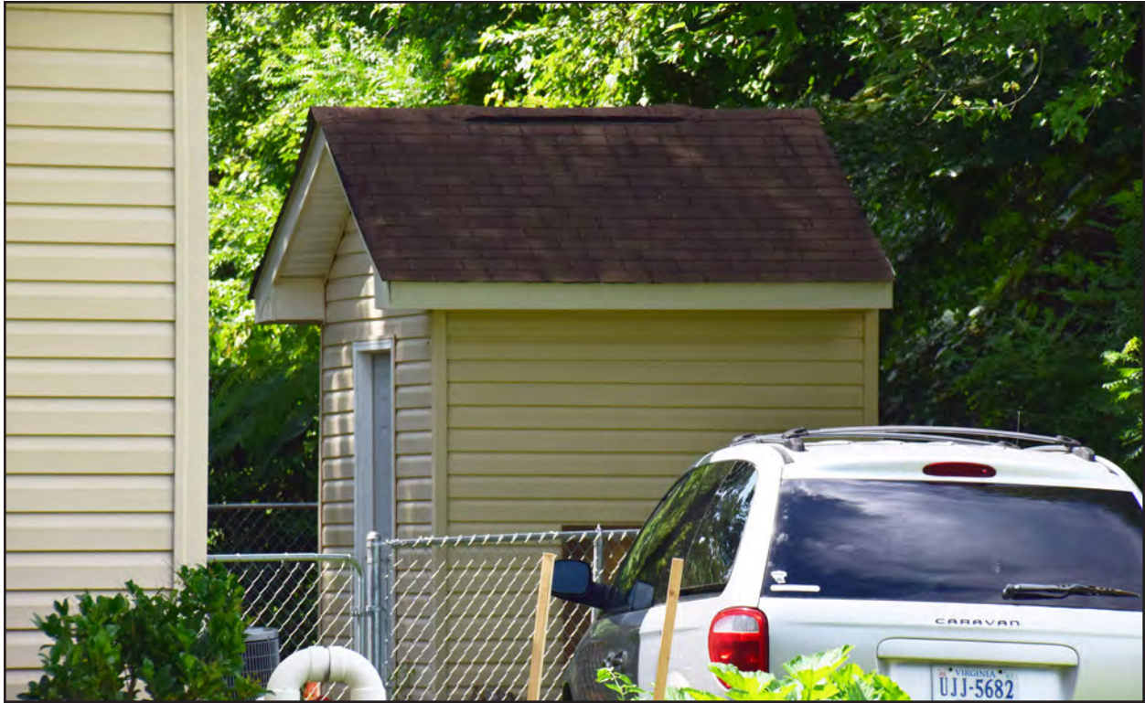
Figure 21. 134-0103, Shotgun house, no longer extant, view to the south.
