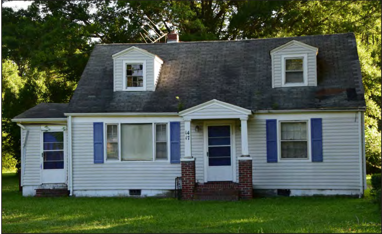
Figure 43. 131-5991, Cape Cod dwelling, southwest elevation, view to the northeast.
