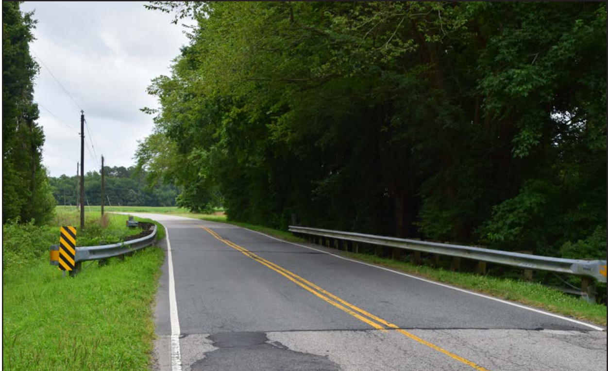
Figure 100. 131-6217 /VDOT #8004, view to the southeast.
