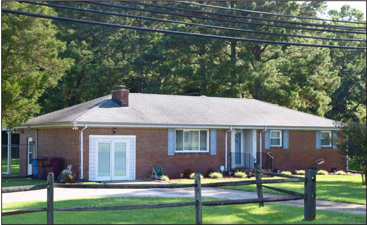
Figure 81. 131-6198, compact ranch dwelling, south and west elevations, view to the northeast.
