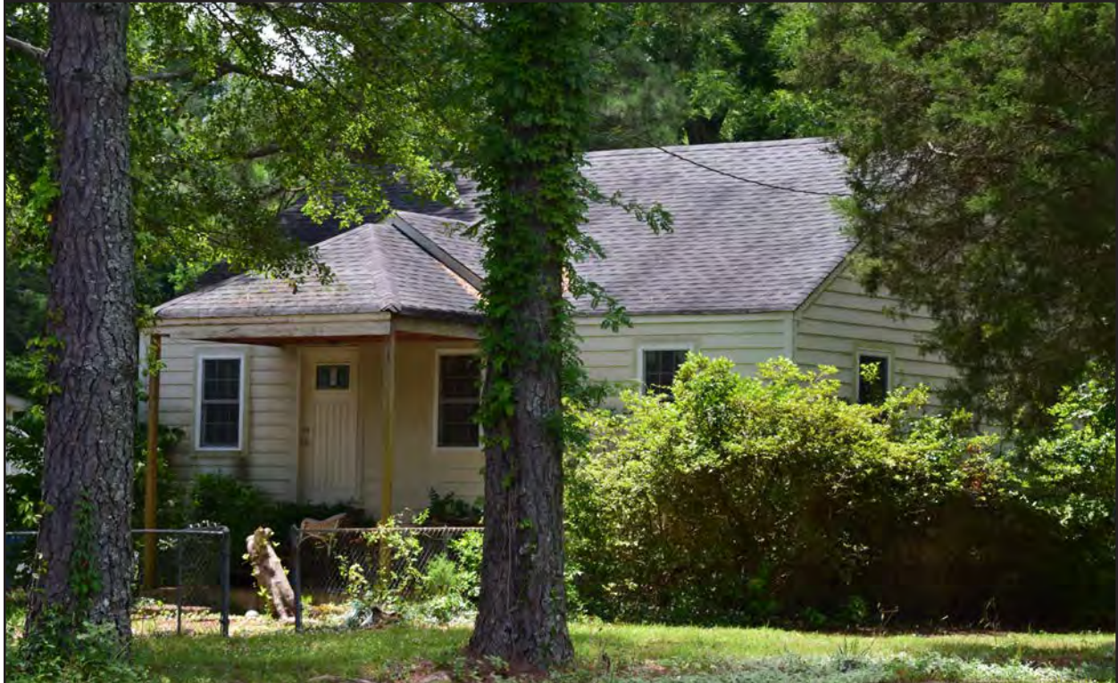
Figure 190. 134-5131, vernacular dwelling, east elevation, view to the west.
