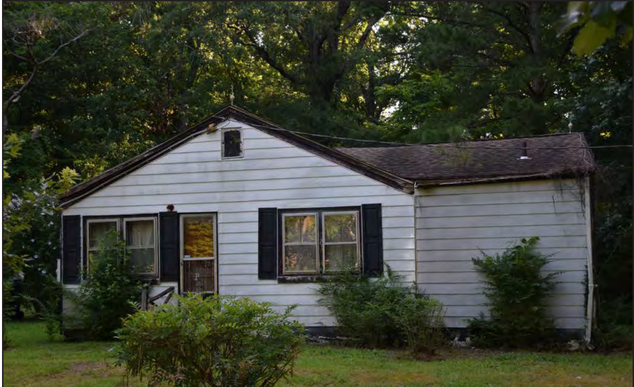
Figure 270. 134-5930, dwelling, southwest elevation, view to the northeast.
