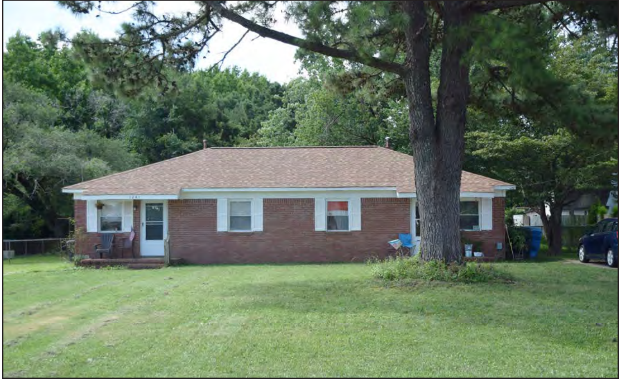
Figure 201. 134-5221, duplex, north elevation, view to the south.
