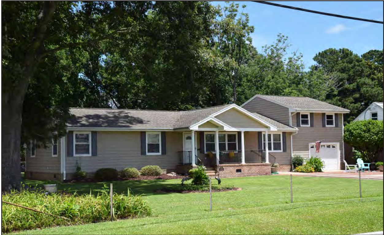
Figure 251. 134-5911, linear Ranch, south and west elevations, view to the northeast.
