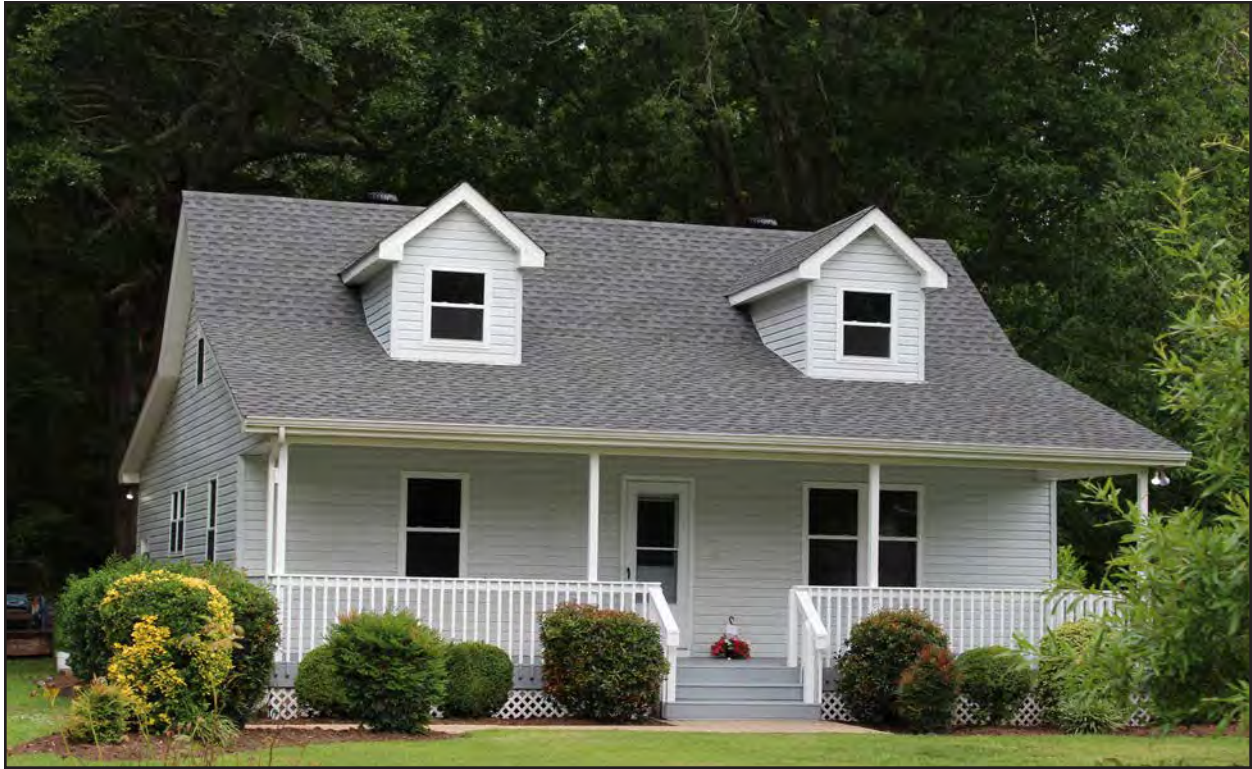
Figure 107. 131-6224, vernacular dwelling, east and south elevations, view to the northwest.
