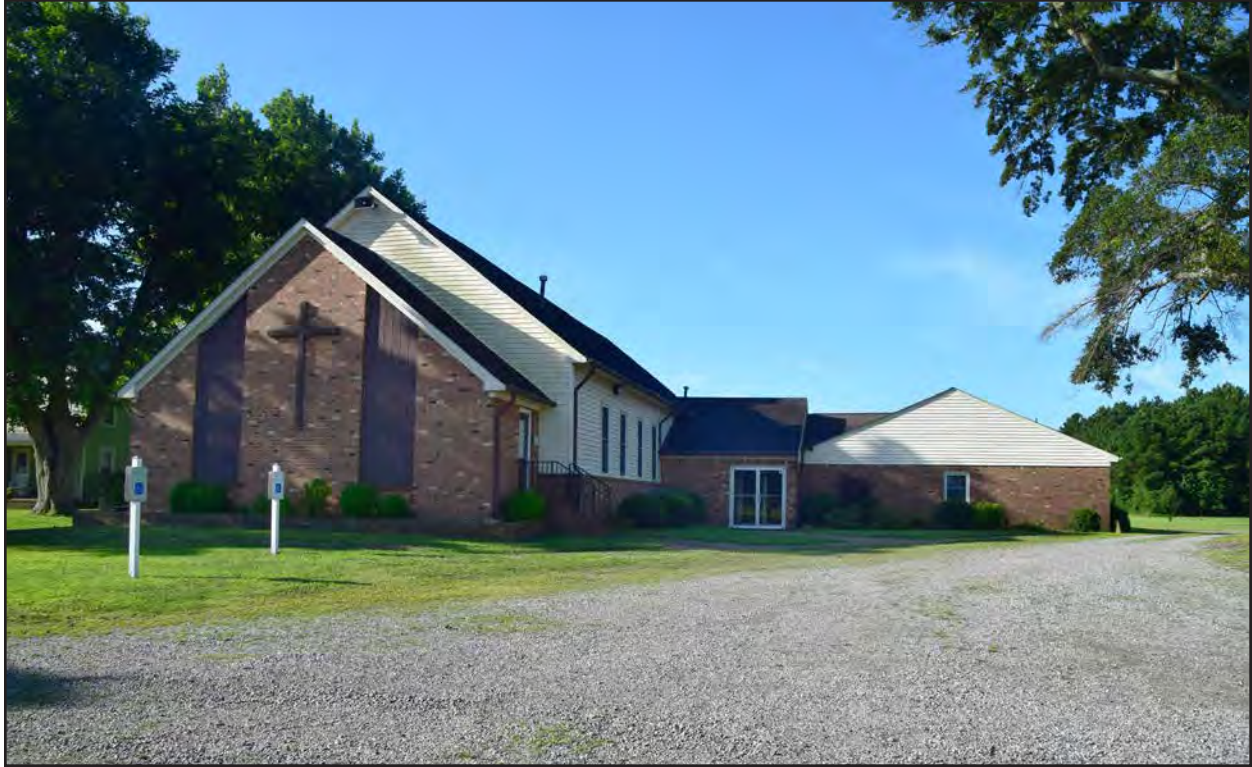
Figure 11. 131-0179, Mount Pleasant Mennonite Church, north and west elevations, view to the south-
