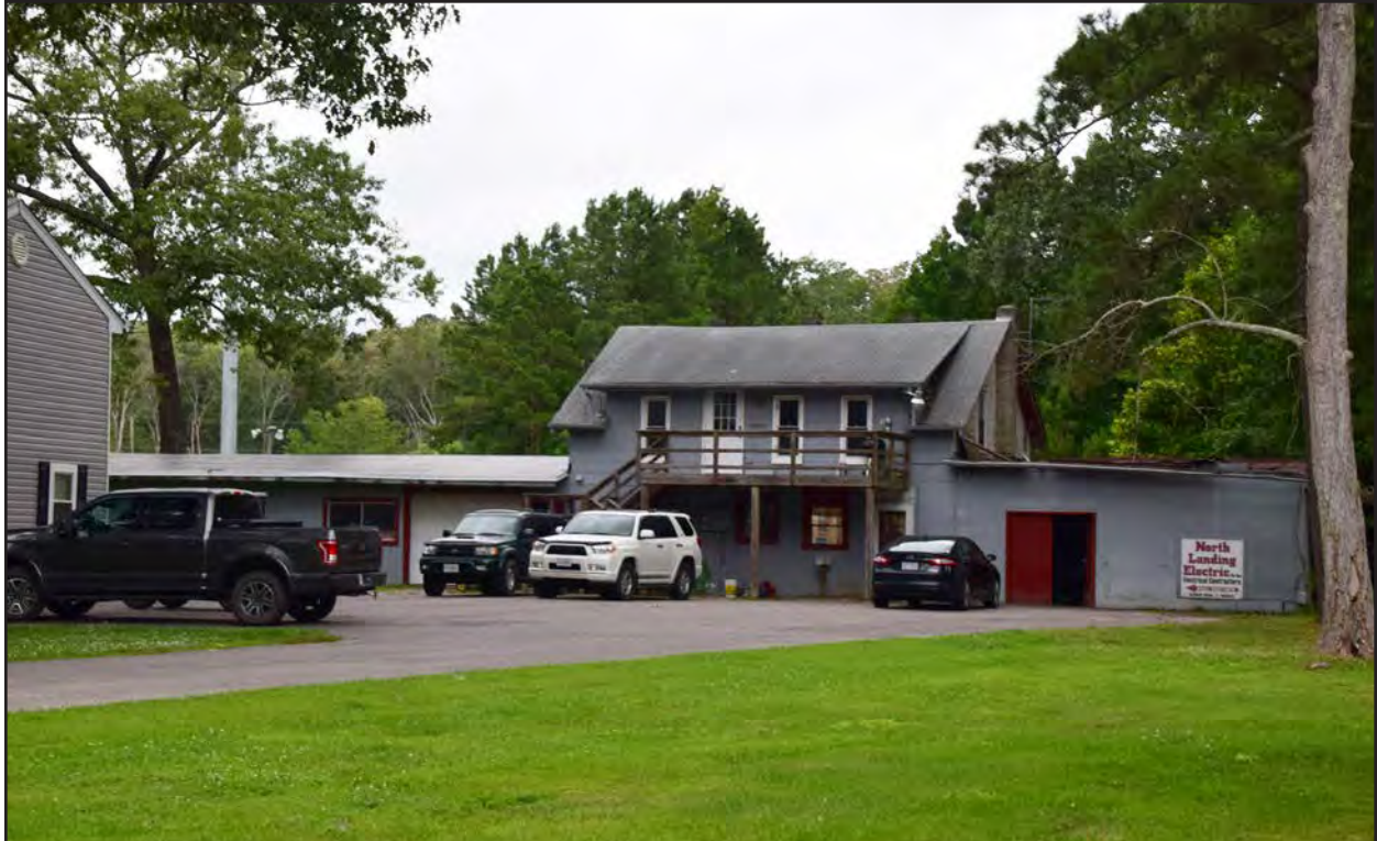
Figure 248. 134-5908, North Landing Electric, vernacular building, south elevation, view to the north.
