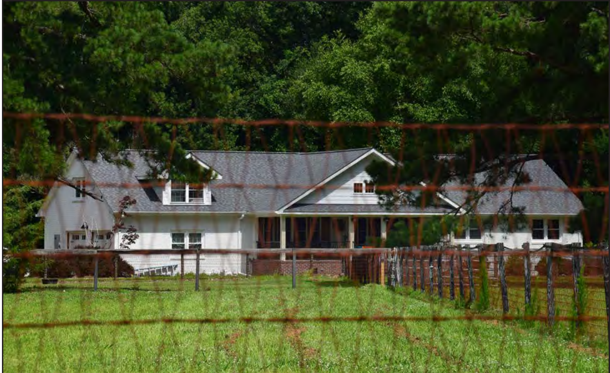
Figure 238. 134-5898, dwelling, southeast elevation, view to the northwest.
