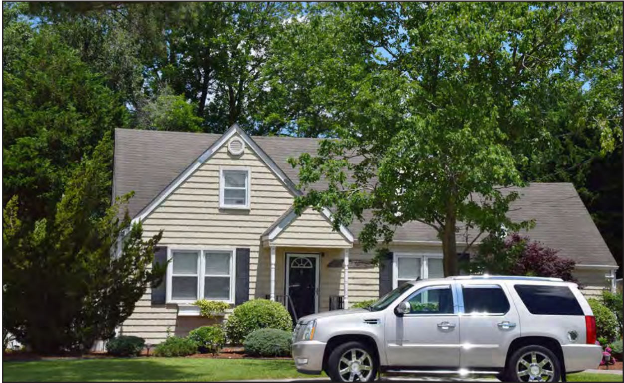
Figure 205. 134-5225, dwelling, south elevation, view to the north.
