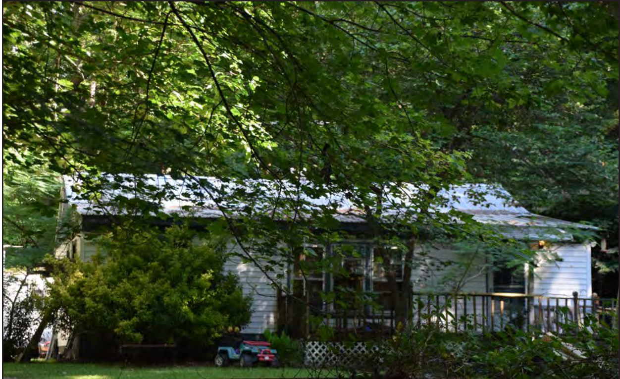
Figure 268. 134-5928, dwelling, southeast elevation, view to the northwest.
