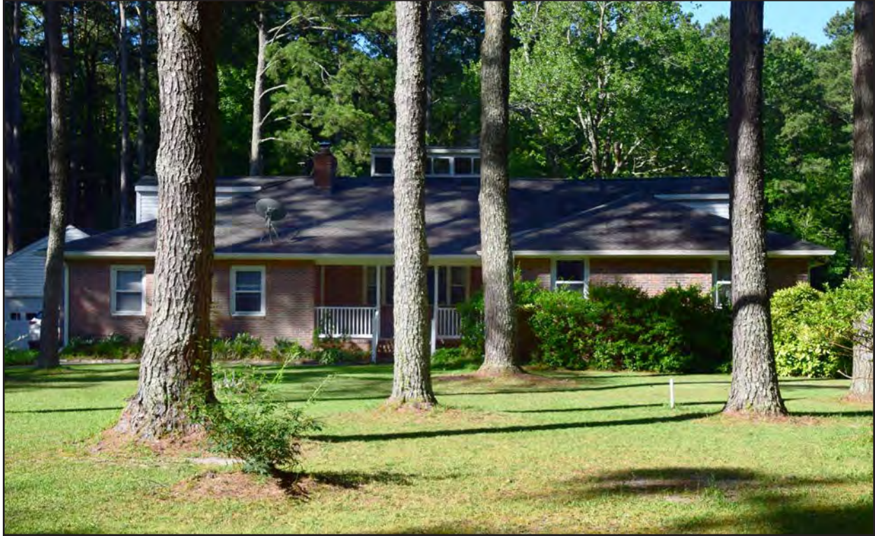
Figure 285. 134-5949, linear with clusters Ranch dwelling, northeast elevation, view to the southwest.
