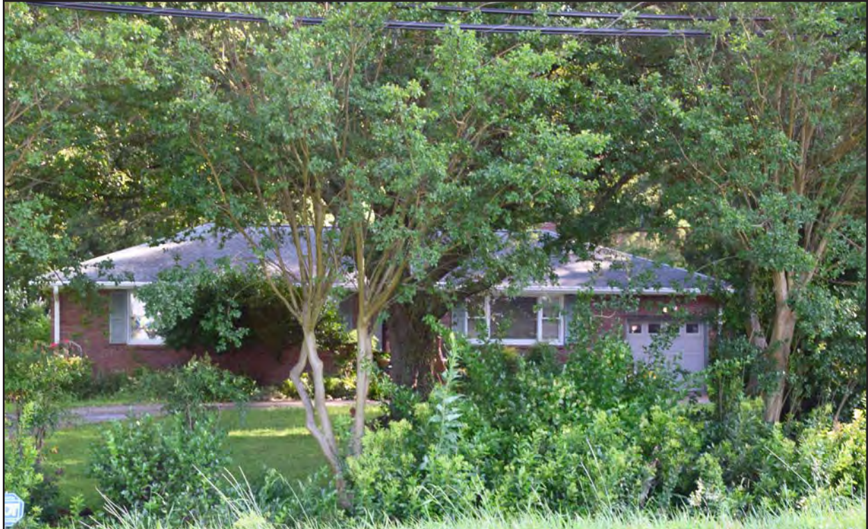
Figure 130. 131-6247, linear Ranch, southwest elevation, view to the northeast.
