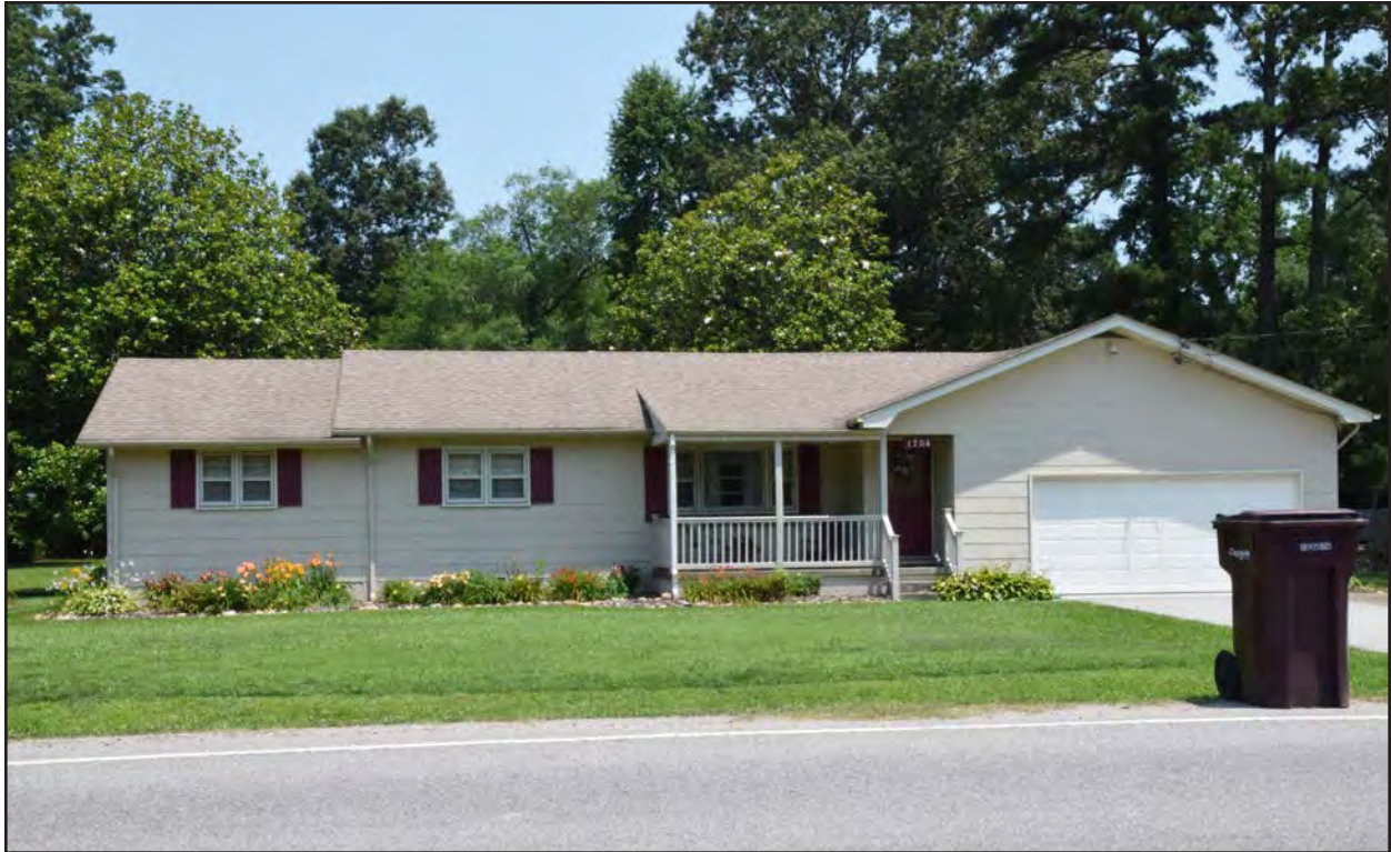
Figure 155. 131-6273, linear Ranch, south elevation, view to the north.
