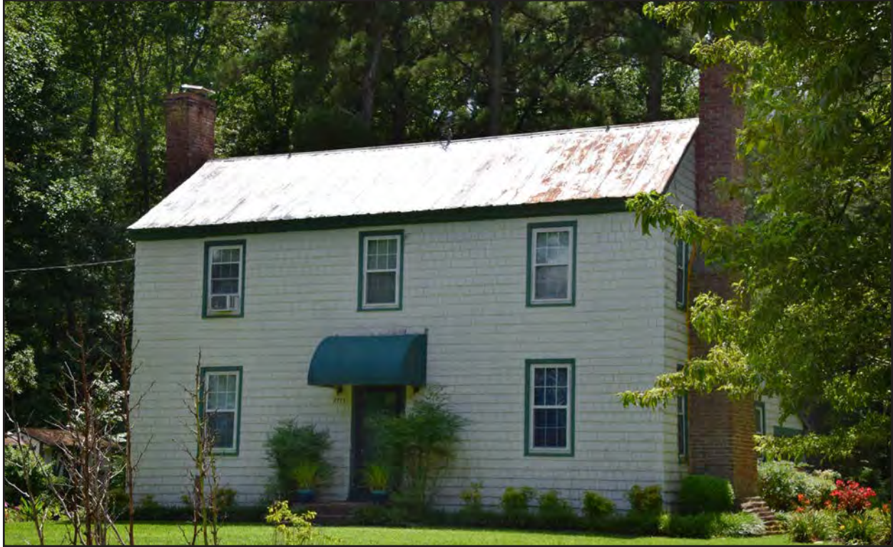
Figure 193. 134-5137, I-House, northeast and northwest elevations, view to the south.
