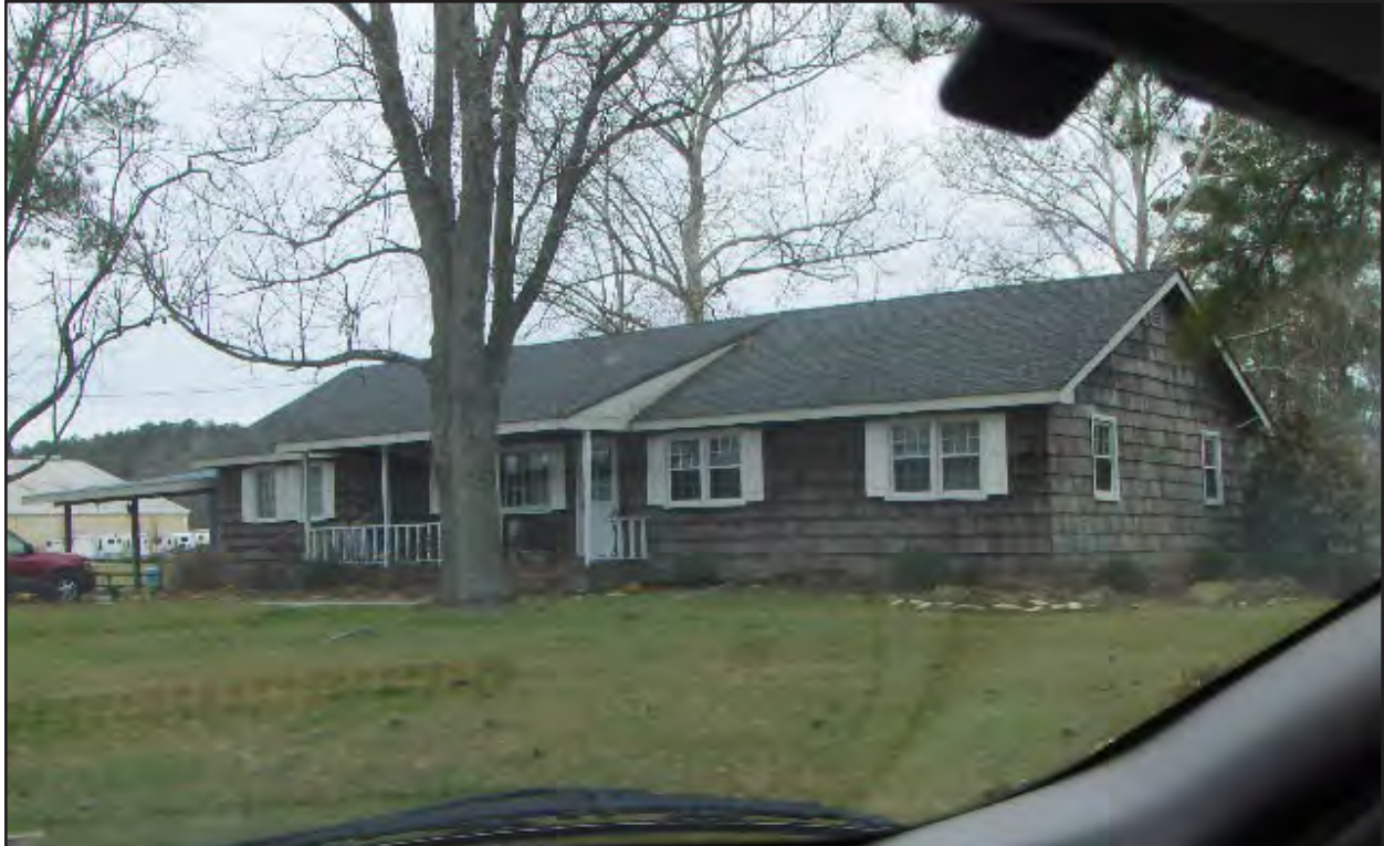
Figure 218. 134-5875, linear Ranch dwelling, southeast and northeast elevations, view to the west (City of Virginia Beach Real Estate Assessor's Office).
