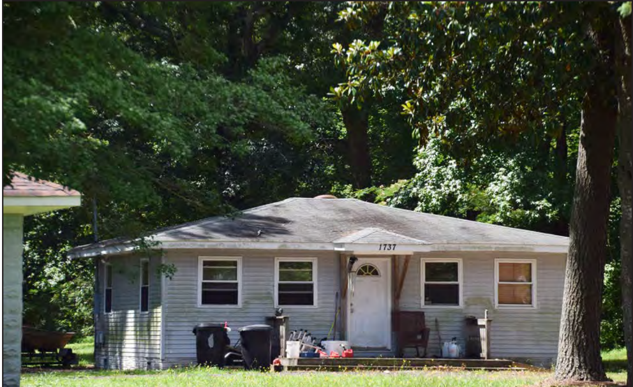
Figure 252. 134-5912, bungalow Ranch, north and east elevations, view to the southwest.
