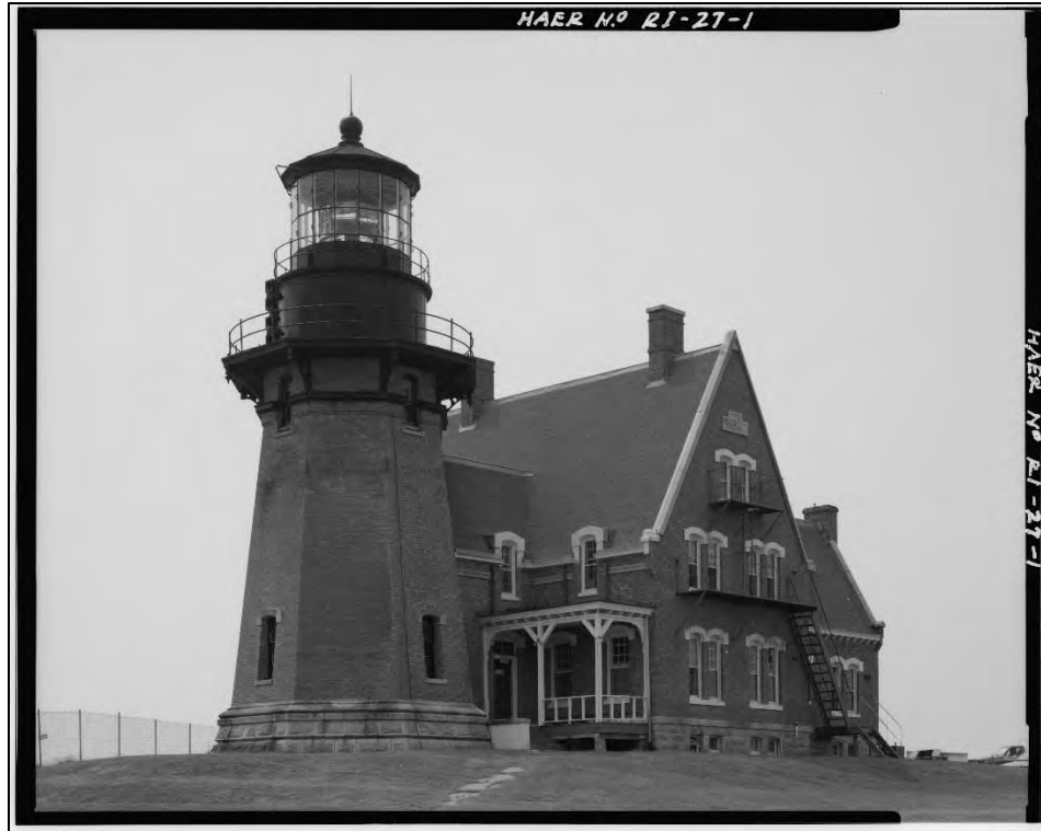
Figure 1. Block Island Southeast Lighthouse before it was offset from the bluff edge (Stupich 1988).
