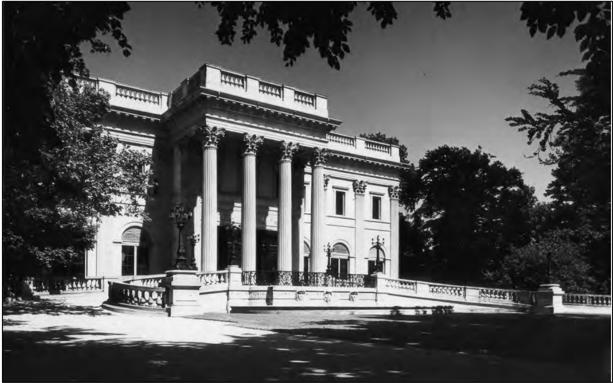
Figure 5. Marble House in the Bellevue Avenue Historic District (NRHP 1971b).
