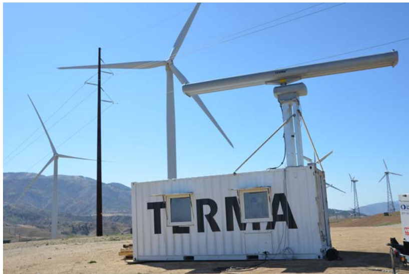
Figure 6. Terma SCANTER 5202 PSR Installed at TWRA
