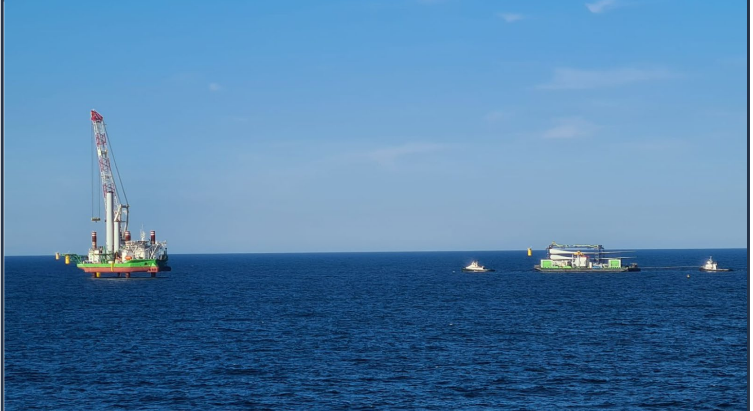
Figure 3.2-2 Wind Turbine Generator Installation
