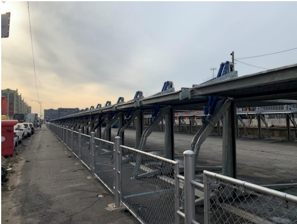
Figure 3.8-11 Viewpoint 8 – Obstructed View of Gowanus Bay Waterfront, Bush Terminal Historic District, and Project Area Looking Southwest from 2nd Avenue north of 2nd Avenue KOP
