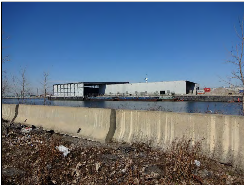
Looking north from 35th Street "Pier" at SBMT toward contemporary recycling facility at 29th Street "Pier." 35th Street "Pier" will be repaved, a wharf installed into the "interpier" basin, and the basin will be dredged, as will the area to the west of the 35th Street "Pier."
