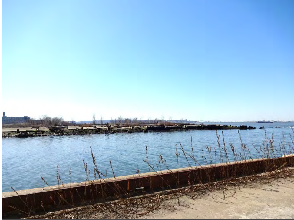
Looking west toward Pier 7 in National Register-eligible Bush Terminal Historic District from SBMT 39 th Street "Pier." Dredging would occur in the "interpier" basin between remnants of Pier 7 and 39 th Street "Pier." Improvements would be made to the 39 th Street "Pier."
