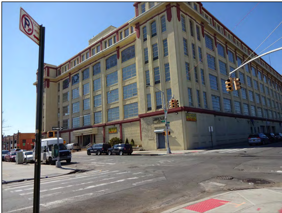
Looking toward east façade of American Can Company; façade faces Second Avenue.
