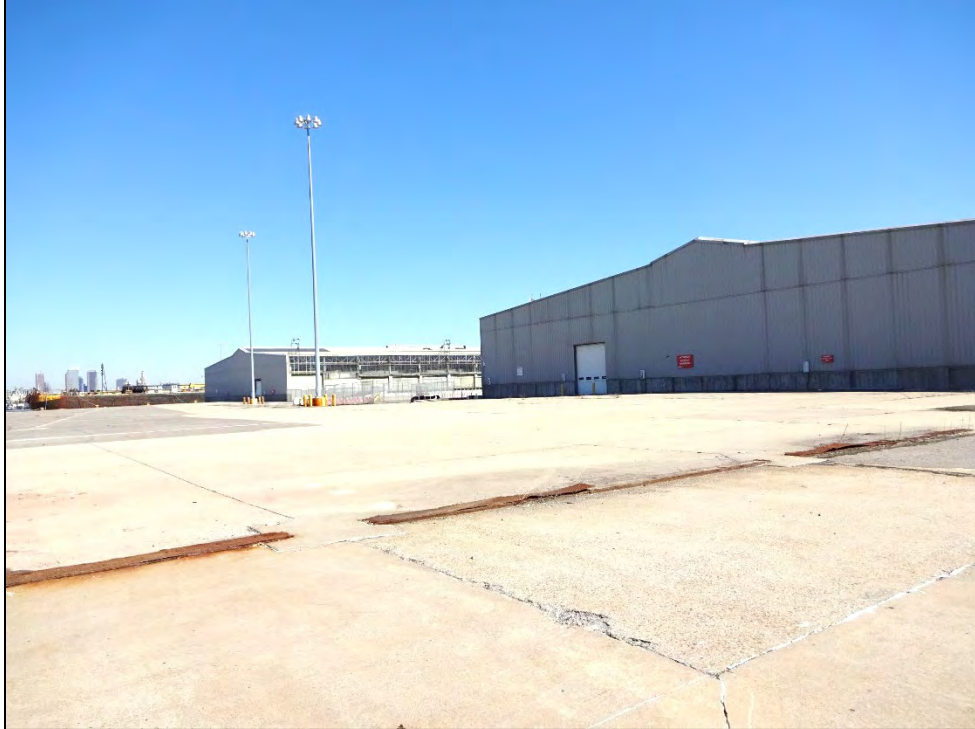
Looking southwest toward existing building structures at SBMT (39th Street "Pier"). SBMT has been determined not eligible for listing in the National Register. Structures and paving will be removed, and the area will be repaved.
