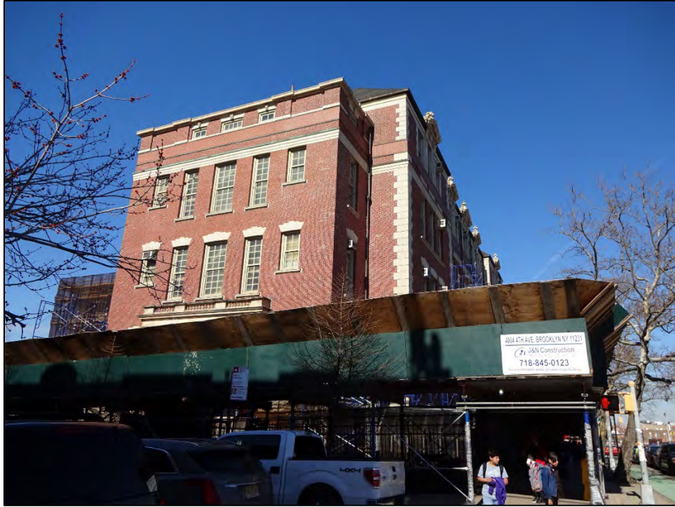
National Register-eligible I.S. 136 at the corner of Fourth Avenue and 41st Street. Building is approximately 1,600 ft removed from SBMT. Looking northward from the south sidewalk of 41st Street
