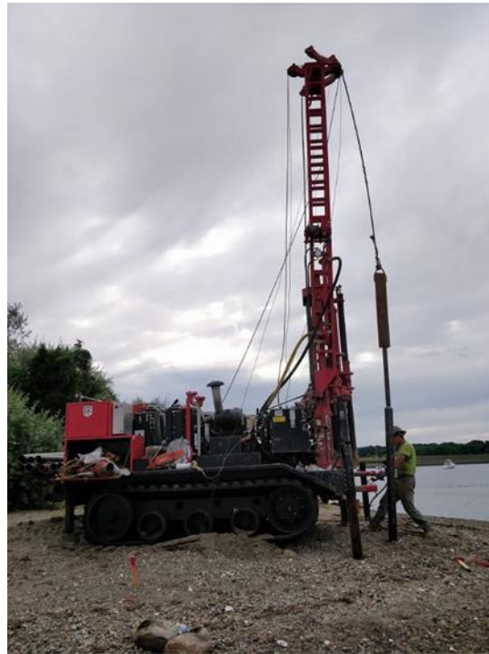
Figure 2-6 Pile driving at Davisville, URI
