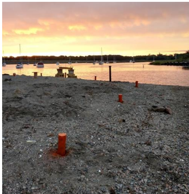
Figure 2-7 Driven piles at Davisville, URI
