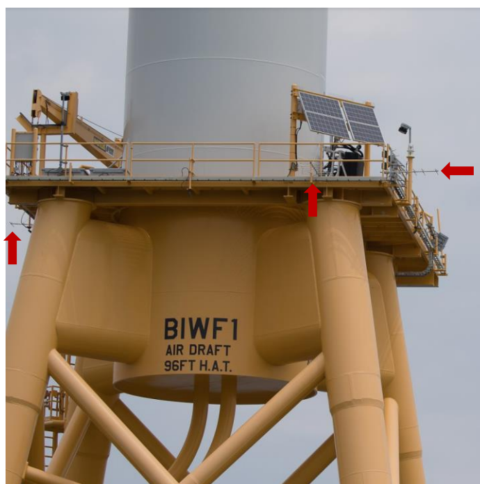
Figure 1.18. Block Island Wind Farm Turbine #1 (eastern most turbine) showing 3 of 4 6-element (7.1-dB) antennas (red arrows) mounted on railings ~ 33 m above ocean.
