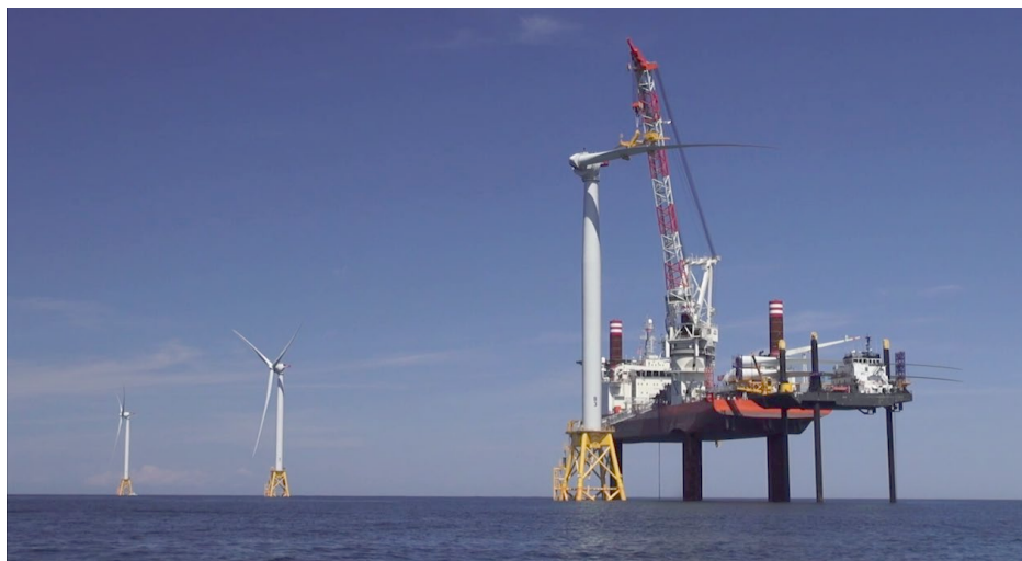
Photos: All 3 images depict the decommissioning phase of offshore wind turbines.
