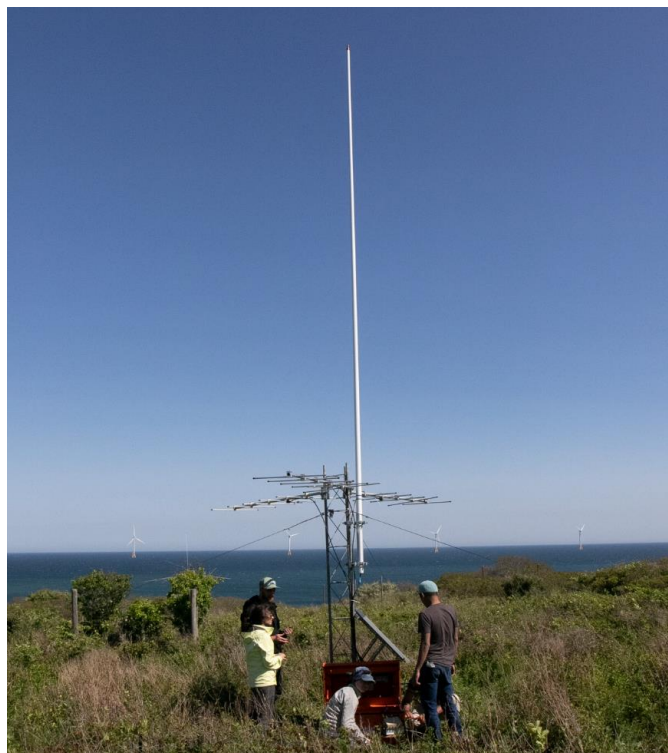
Figure 1.13. Tower array (3 m tall tower) at Southeast Lighthouse in June 2019, showing 3 5-element Yagi 8-dB antennas, a 6.m tall, 10-dB omnidirectional antenna, with Lotek SRX800 receiver.
