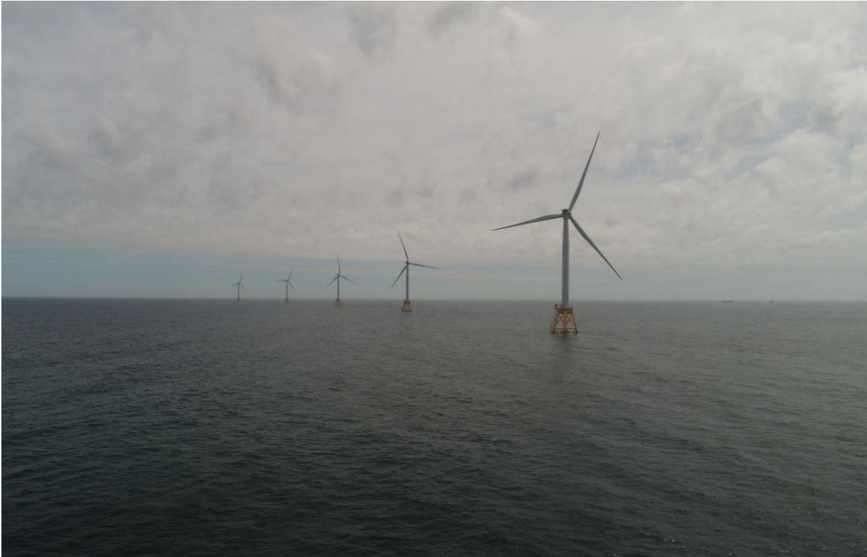
Endpiece – Block Island Wind Farm taken by drone during calibration survey
