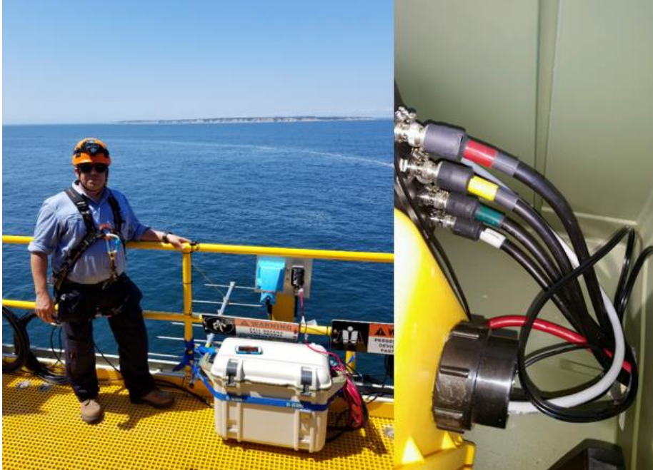
Figure 1.16. VHF telemetry station on Turbine #1, Block Island Wind Farm, installed on 3 August 2017 by Deepwater Wind with 4 6-element 7.1-dB Yagi antennas installed. Block Island can be seen in background. Photo by J. O’Keefe DWW.
