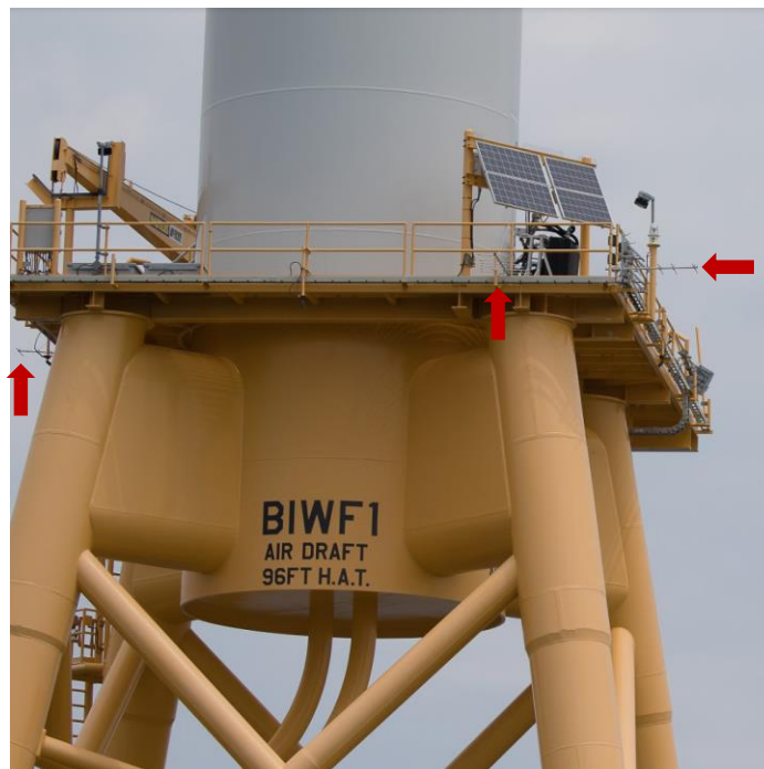
Figure 1.18. Block Island Wind Farm Turbine #1 (eastern most turbine) showing 3 of 4 6-element (7.1-dB) antennas (red arrows) mounted on railings ~ 33 m above ocean.
