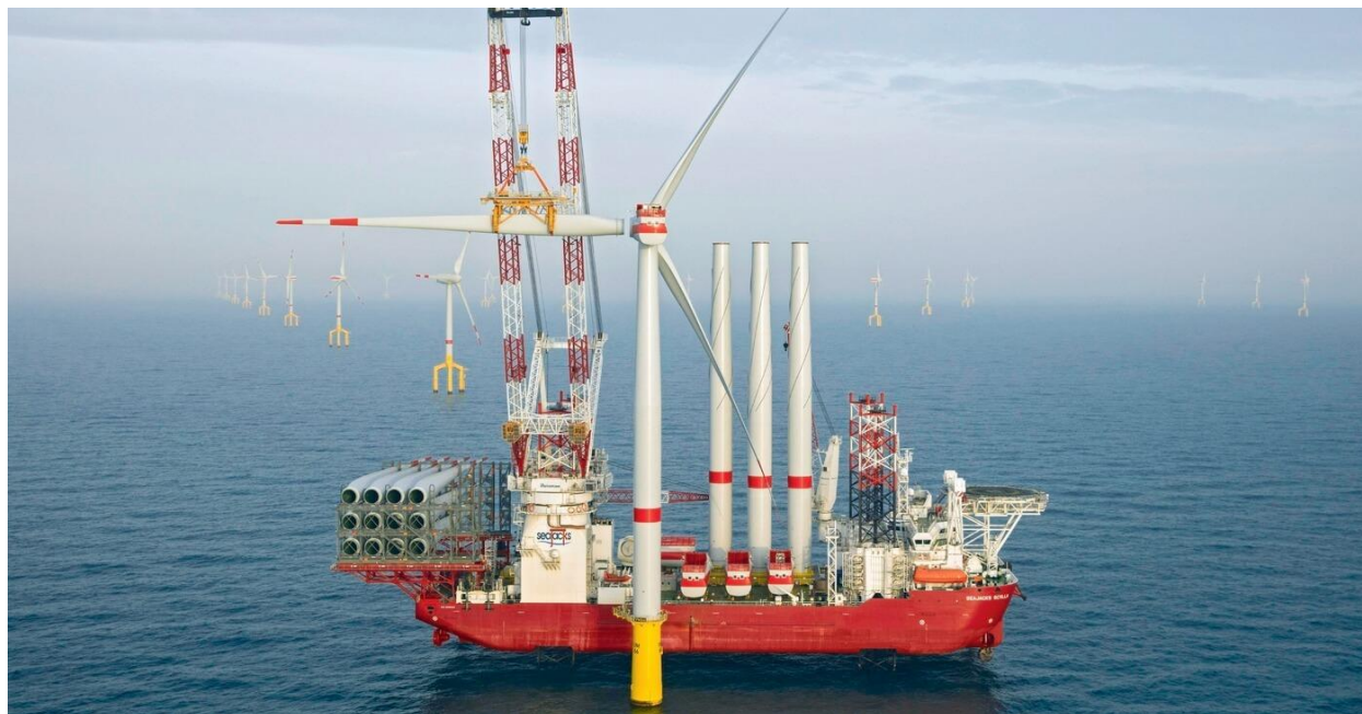
Figure 1 - WTGs transported in vertical position
