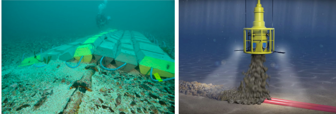
Figure 3-2. Examples of potential cable protection systems: (left) placement of prefabricated concrete mattresses; (b) deposition of rocks along the cable route.
