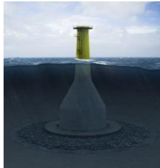
Gravity Base Structure
