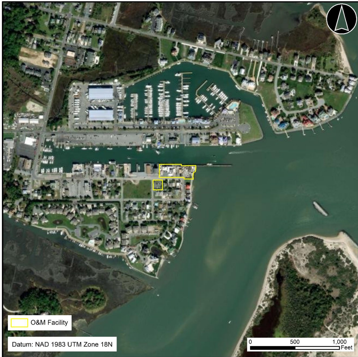
Figure 2-6. Potential Ocean City Harbor Quayside Operations Site
