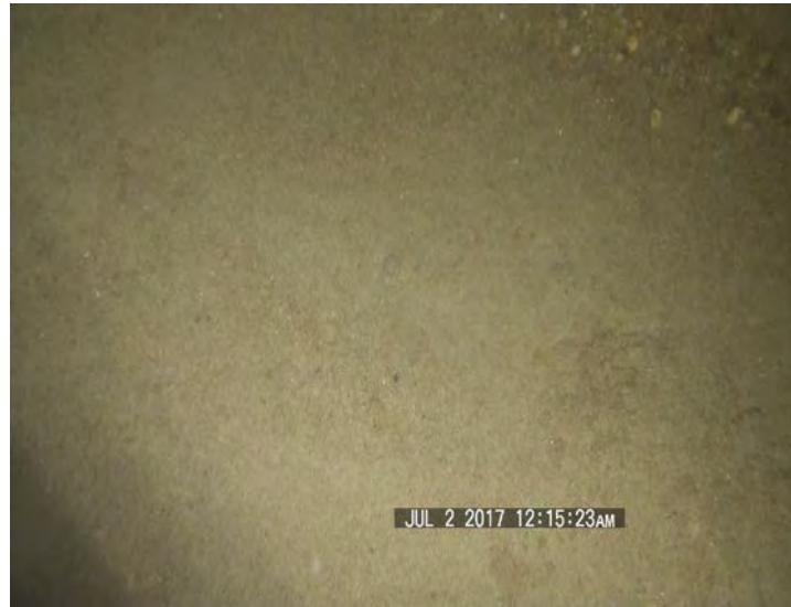
Station Target: E: 548022 N: 4324687 Depth: 22m
