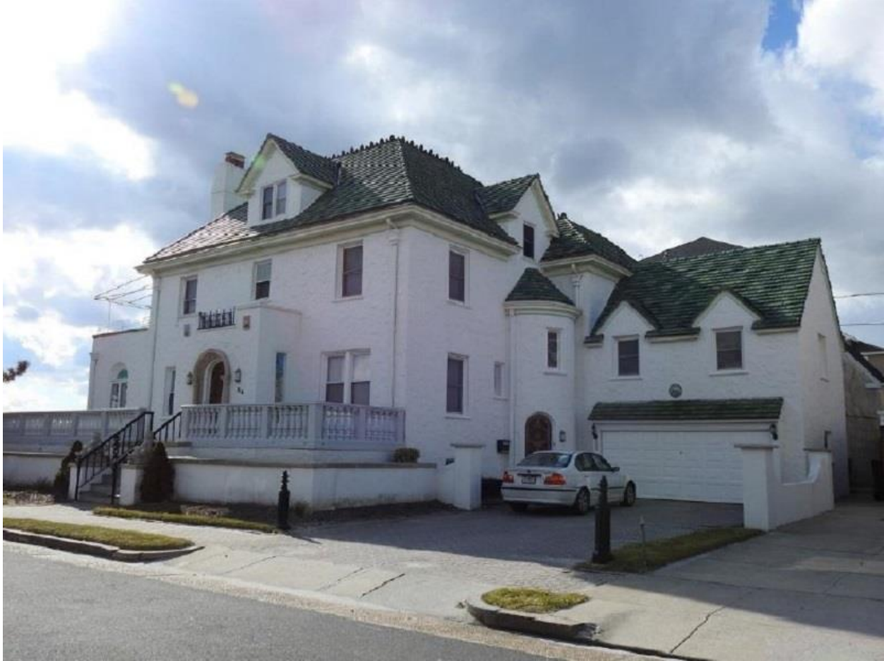
Figure A-3 House at 114 South Harvard Avenue, Ventnor City
