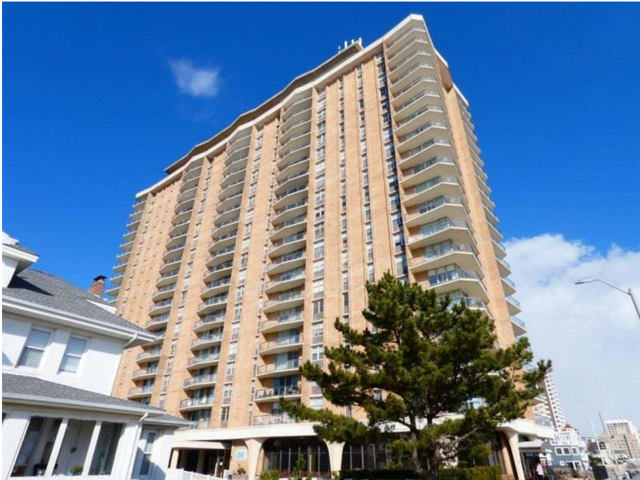
Figure A-2 Vassar Square Condominiums, 4800 Boardwalk, Ventnor City
