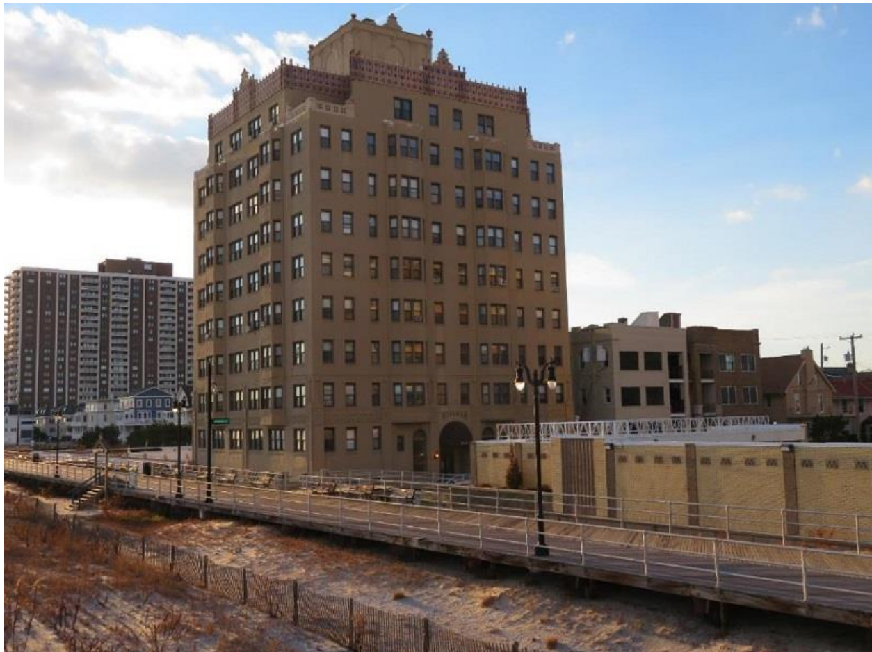
Figure A-1 Riviera Apartment, 116 South Raleigh Avenue, Atlantic City
