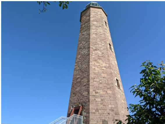
1: Exterior View of Old Cape Henry Lighthouse
