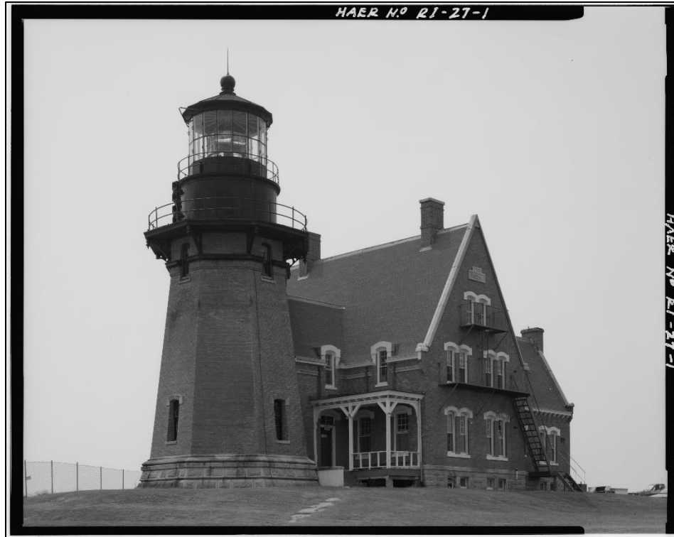
Figure 1. Block Island Southeast Lighthouse before it was offset from the bluff edge (Stupich 1988).
