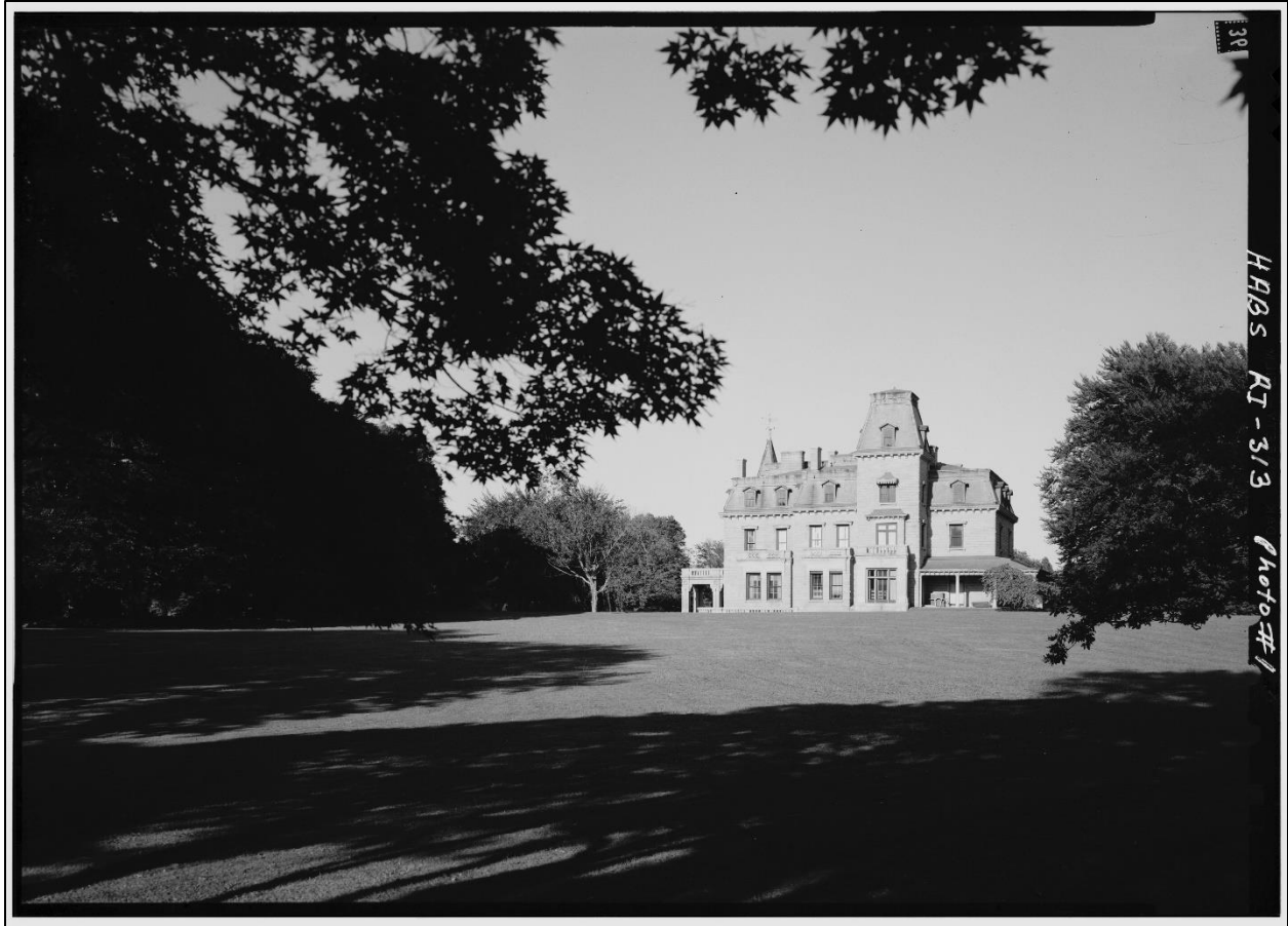
Figure 3. Chateau-sur-mer in the Bellevue Avenue Historic District (Boucher 1969; NRHP 1972).
