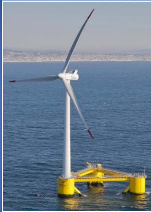
Principle Power 2.0 MW Turbine Portugal 2011 - 2016 17 m waves / 60 knot winds
