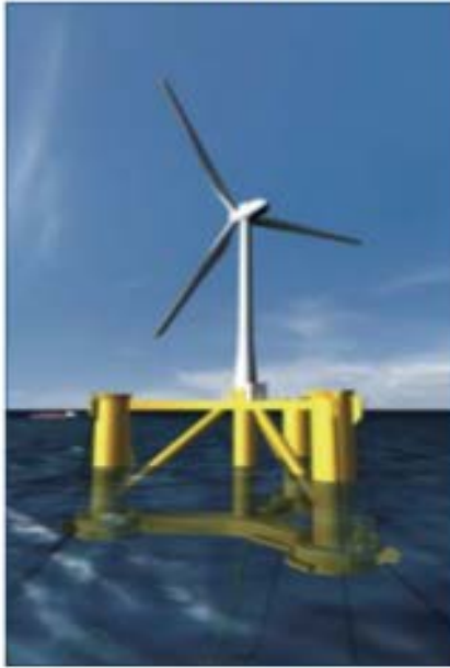
Compact Semi-Sub (2MW)
